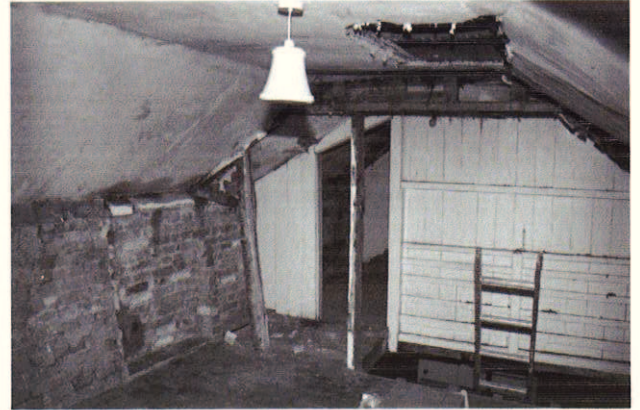
Plate 22: As Plate 21 after plaster stripped
