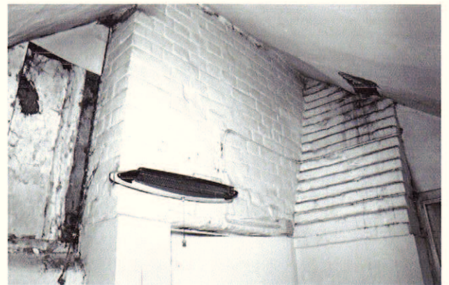
Plate 12: Previously external north-west corner with brick chimney stack
