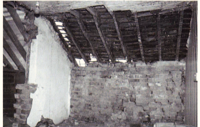
Plate 28: First floor, back room, west wall with roof structure exposed
