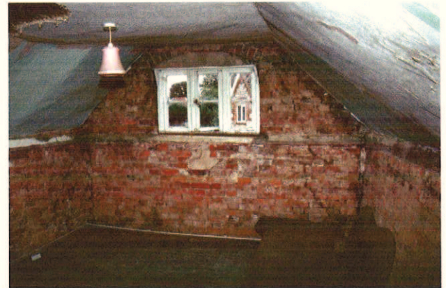
Plate 24: As Plate 23 after plaster stripped
