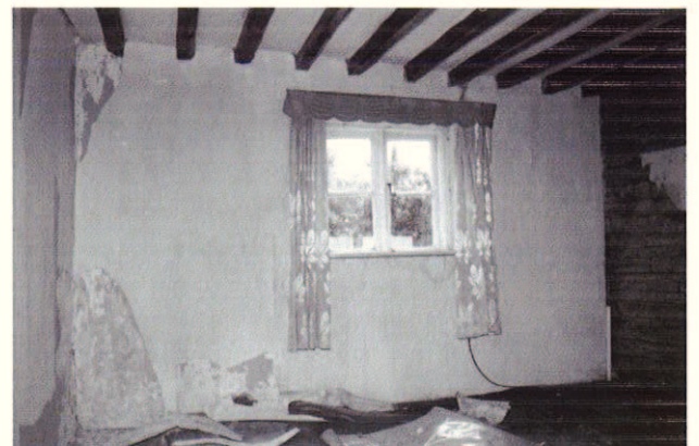
Plate 13: Blocked opening seen in SW extension
