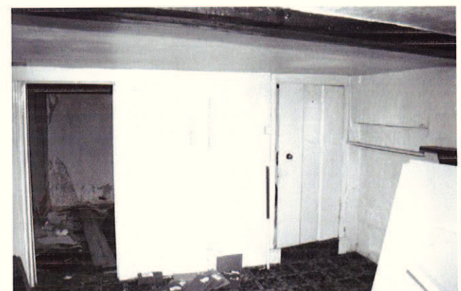
Plate 8: Ground floor, front room, south wall
