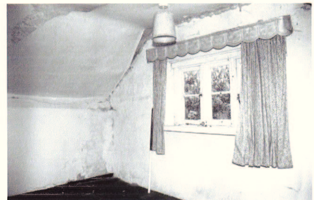
Plate 26: First floor, back room, south-east corner
