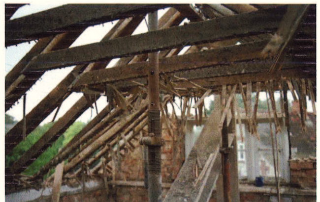
Plate 32: Detail of roof construction – front room, looking north (C A Cheal)
