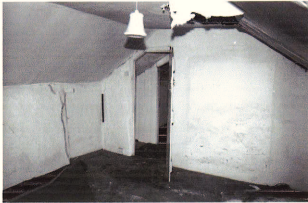
Plate 21: First floor, front room, south-east corner Showing offset in the east wall
