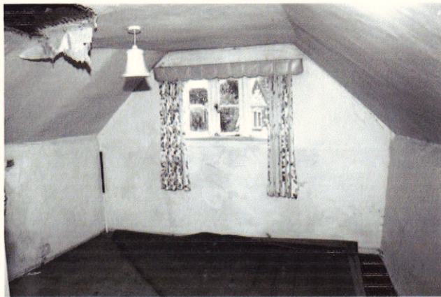
Plate 23: First floor, front room, north wall
