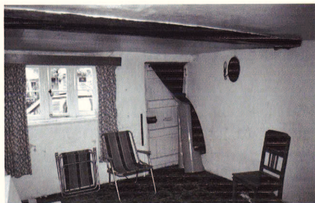
Plate 7: Ground floor, front room, north wall
