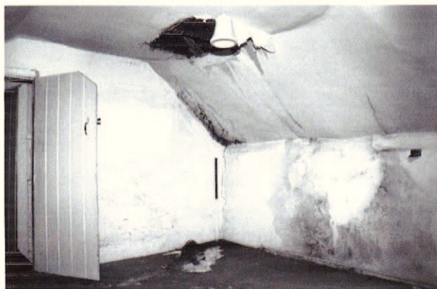
Plate 25: First floor, front room, south-west corner
