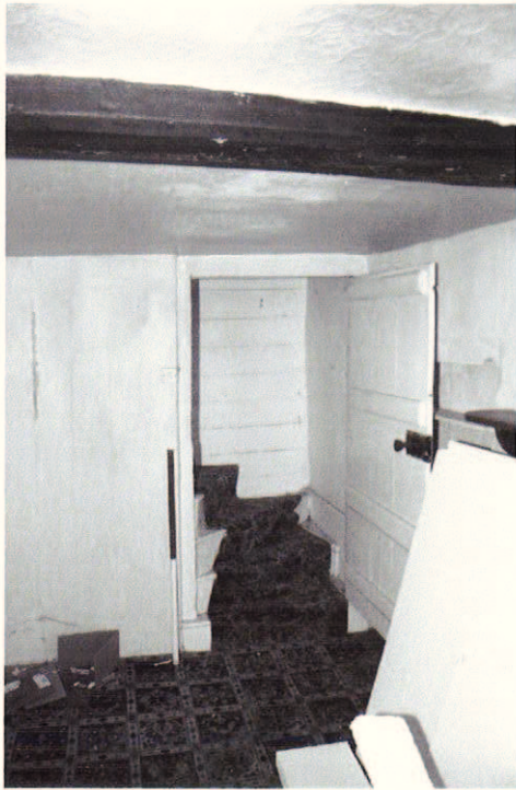
Plate 9: Ground floor, front room, stairs
