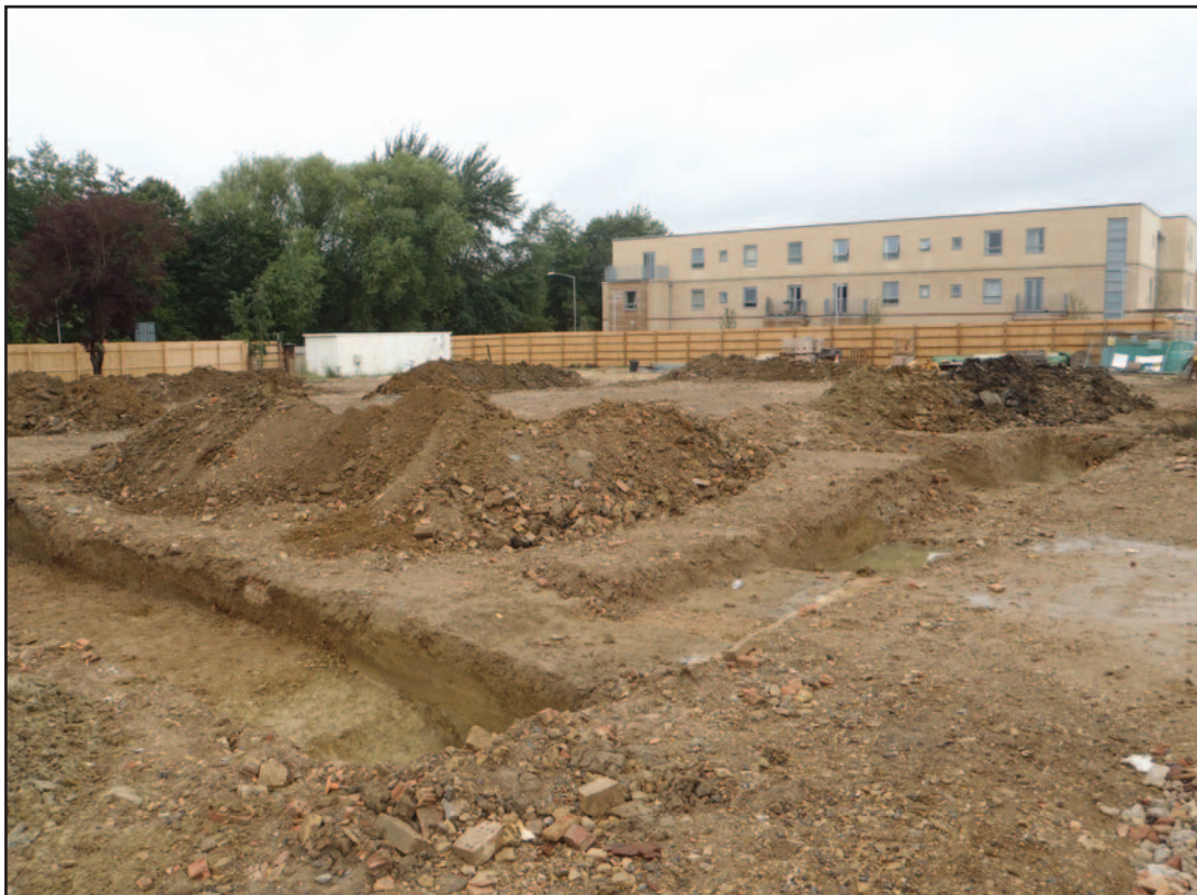
Plate 8: General shot of site showing development on 2007 excavation area, taken from north west
