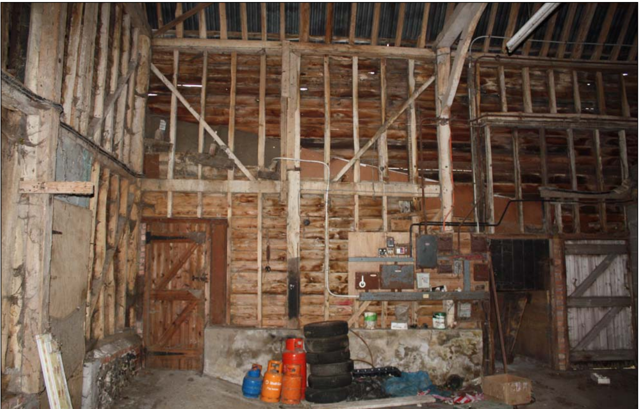
Plate 30: Building 5, internal view, southern elevation
