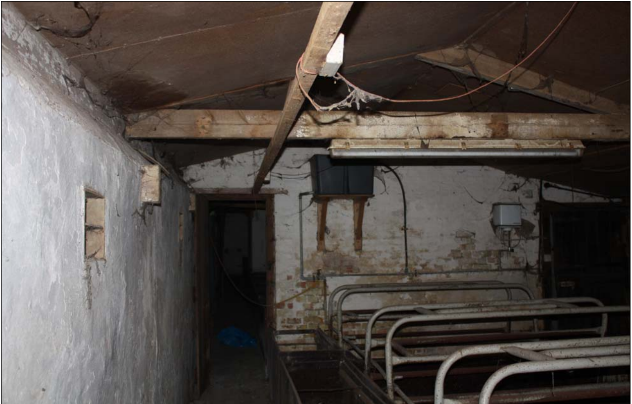
Plate 35: Building 6, internal view
