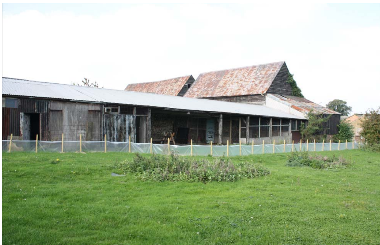
Plate 31: Building 6, viewed from east
