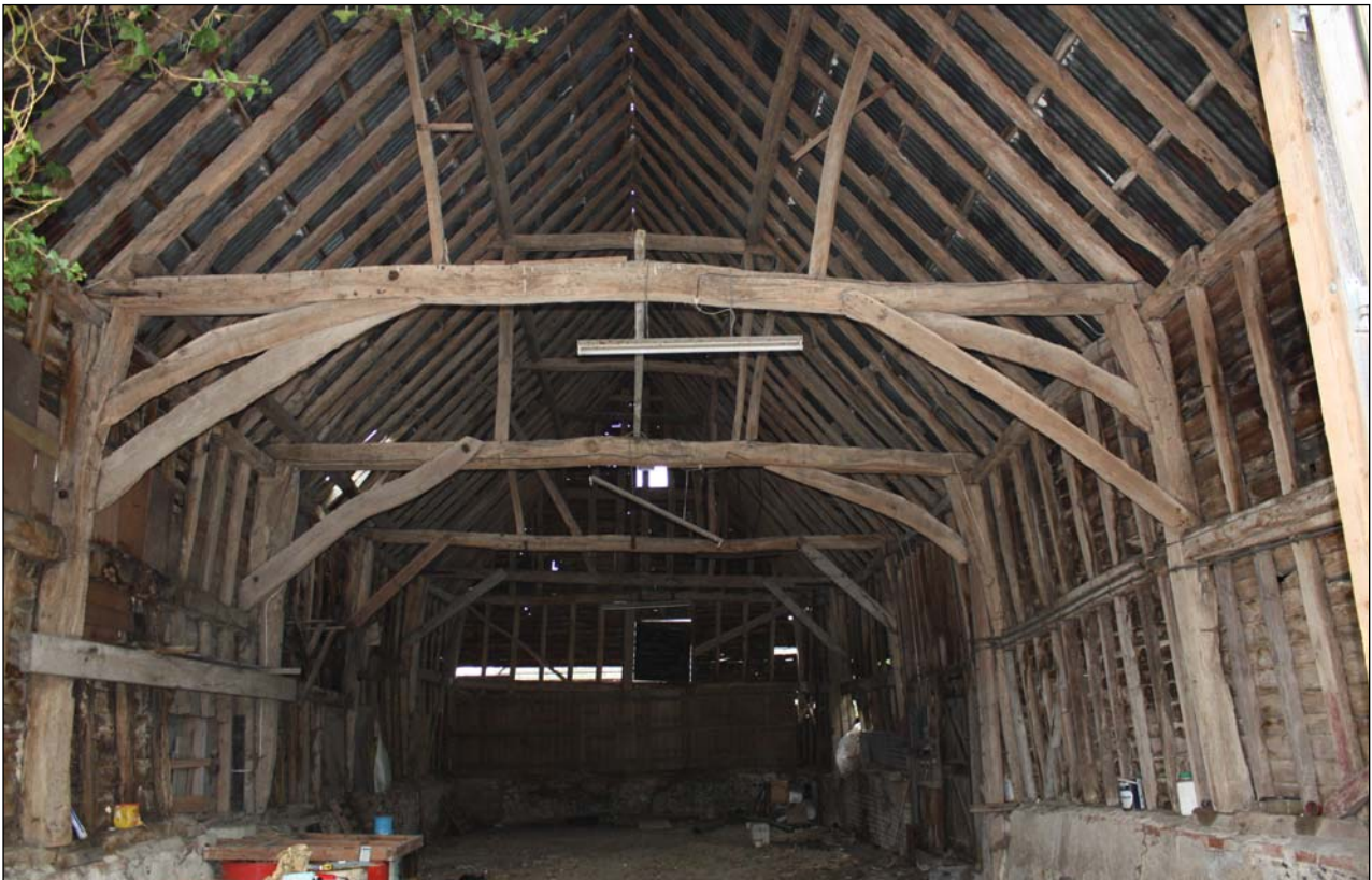
Plate 21: Building 4, Internal view
