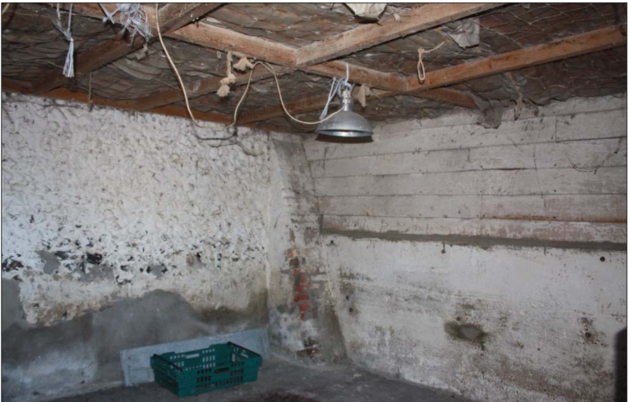
Plate 18: Building 3, Detail of flint wall, viewed from inside
