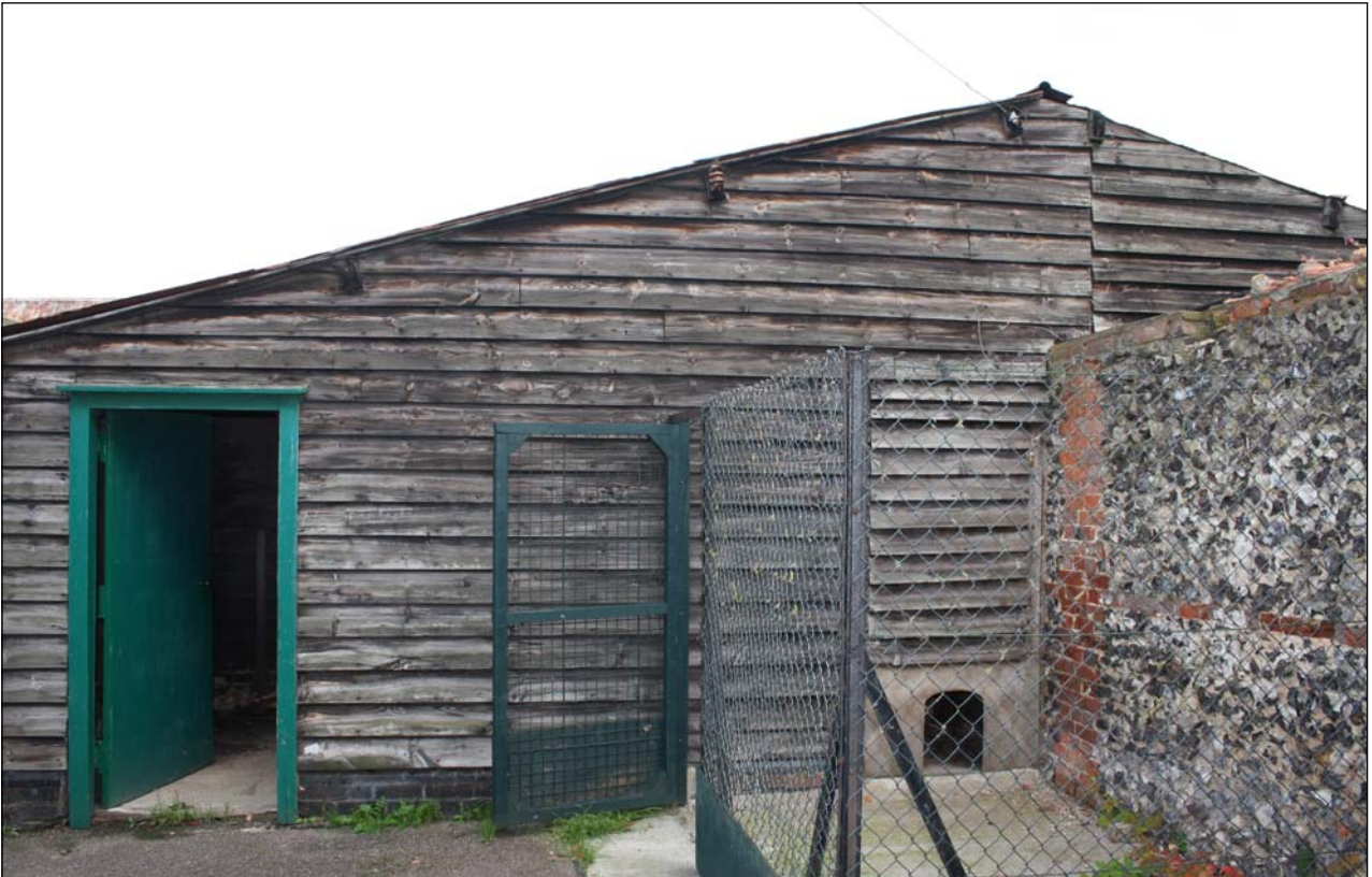
Plate 33: Building 6, southern gable end
