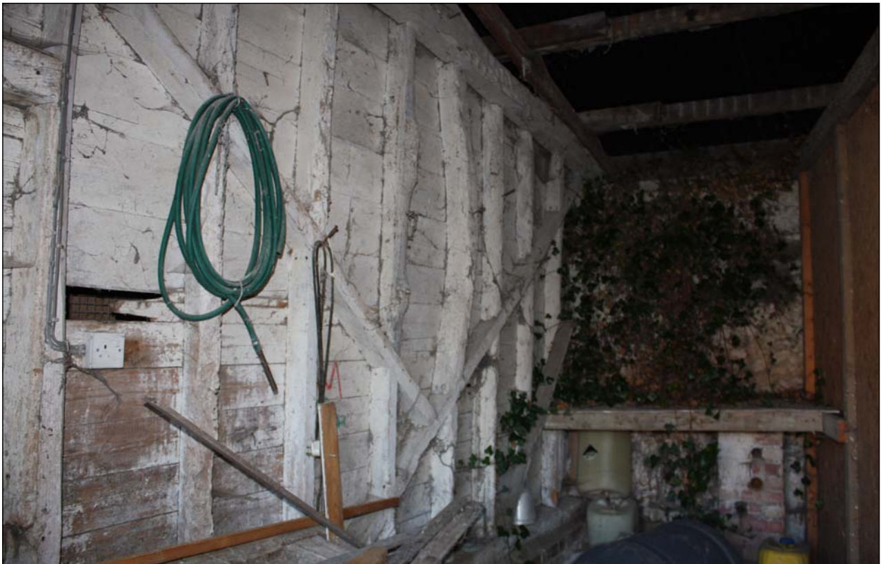
Plate 15: Building 2, Internal view of re-used partition
