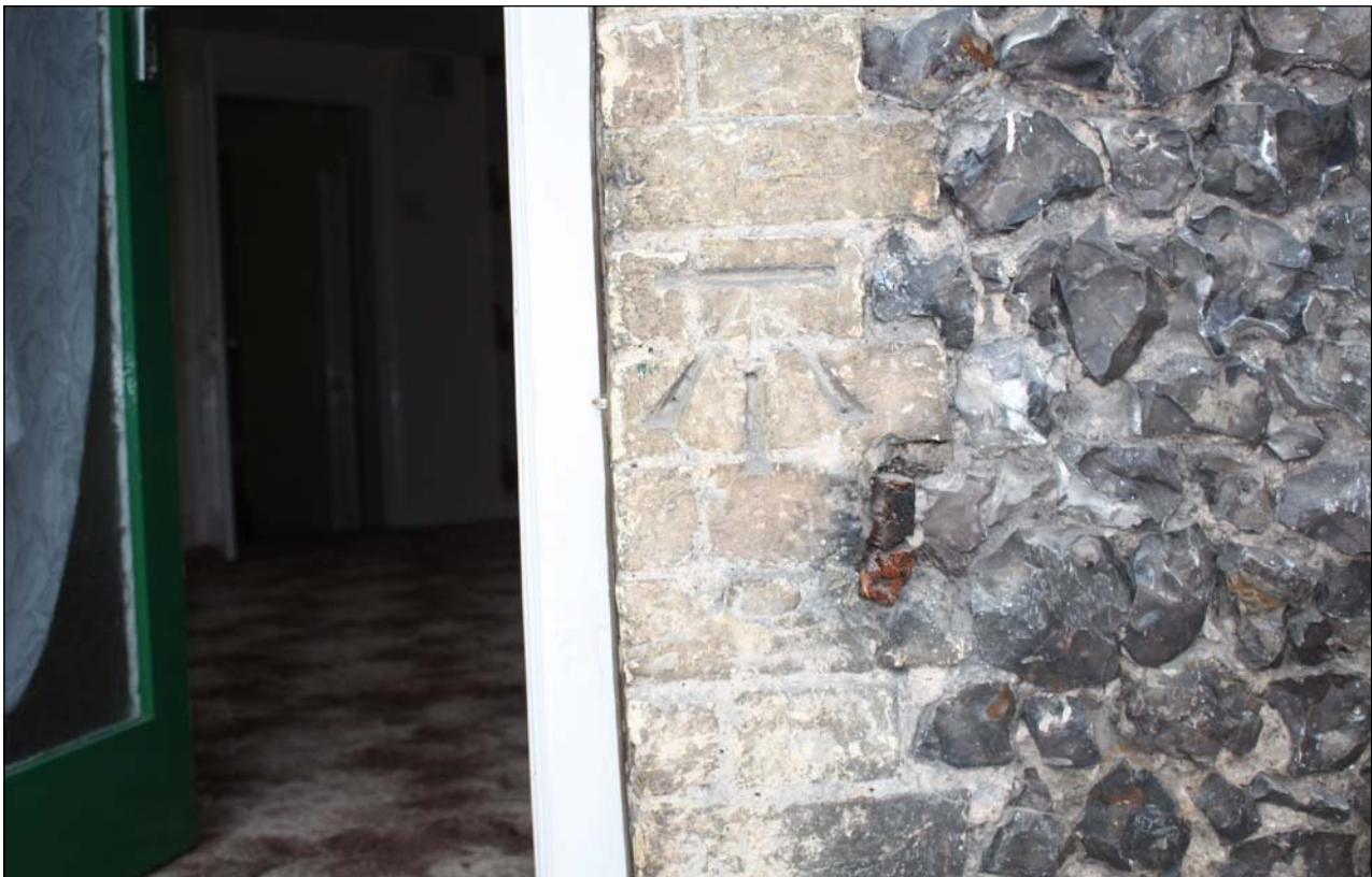
Plate 2: OS Benchmark on right of front door
