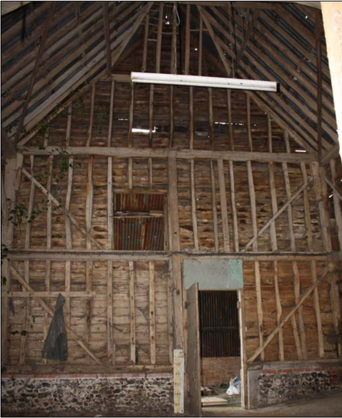
Plate 29: Building 5, internal view, eastern gable end
