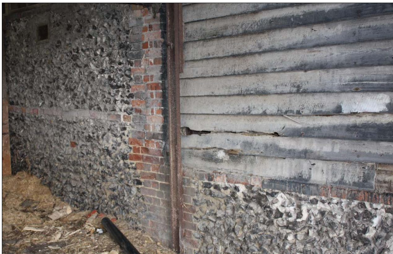
Plate 32: Detail of flint wall where Building 5 joins flint wall of Building 6
