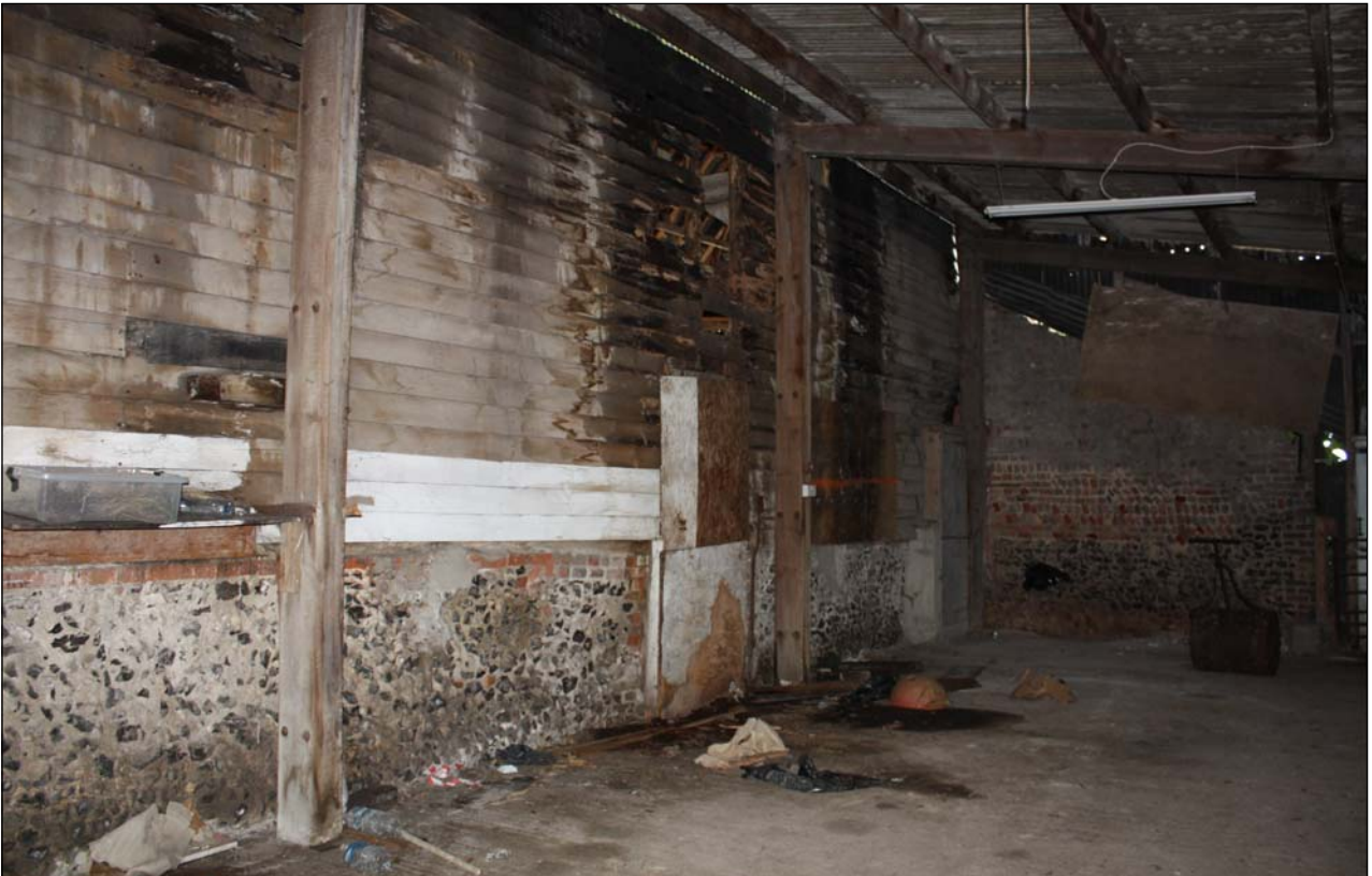
Plate 40: Detail of flint wall and northern elevation of Building 4, viewed from inside Building 11
