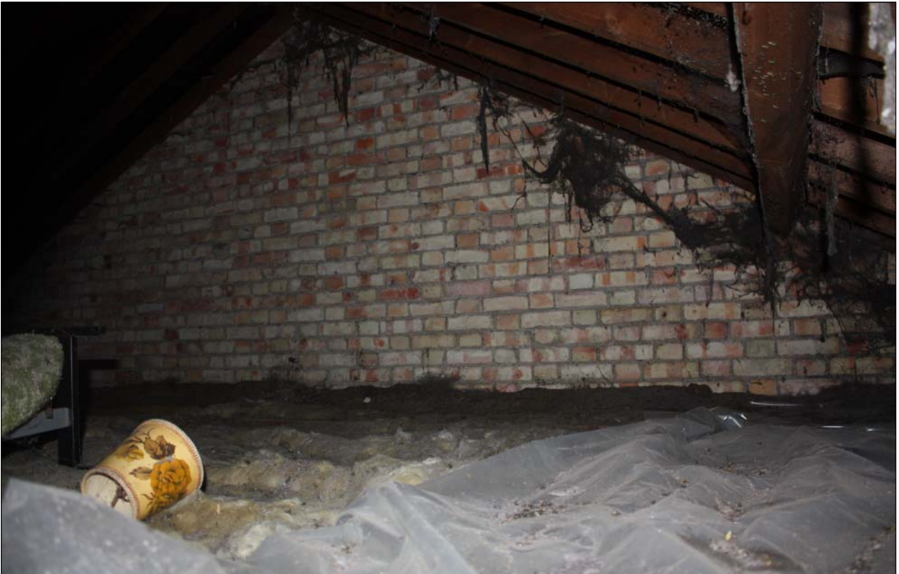
Plate 11: Building 1, Northern gable-end wall of farmhouse, viewed from attic
