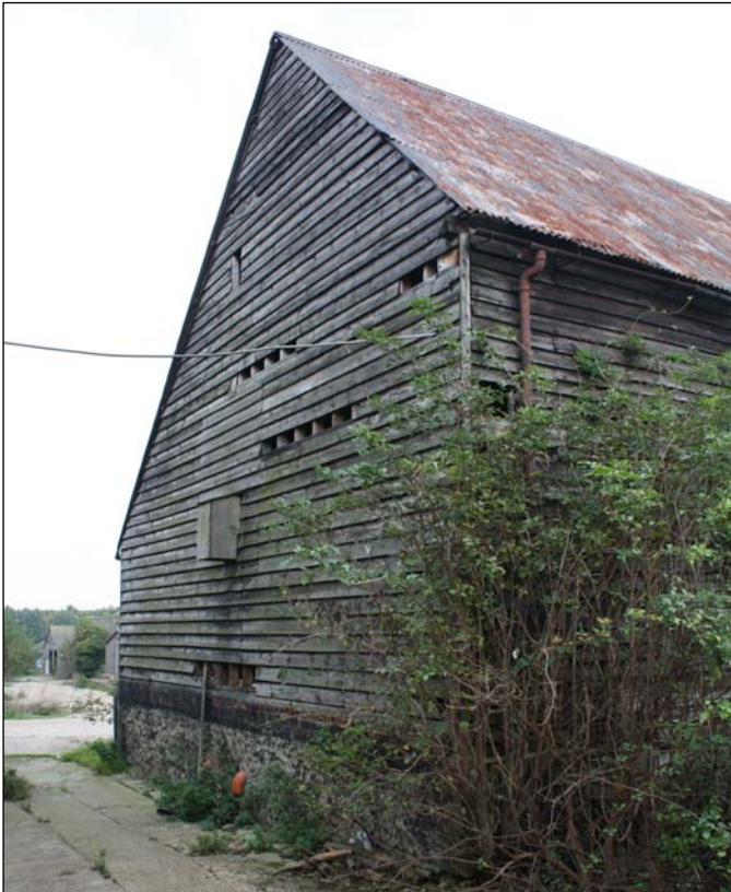
Plate 25: Building 5, gable-end, viewed from south
