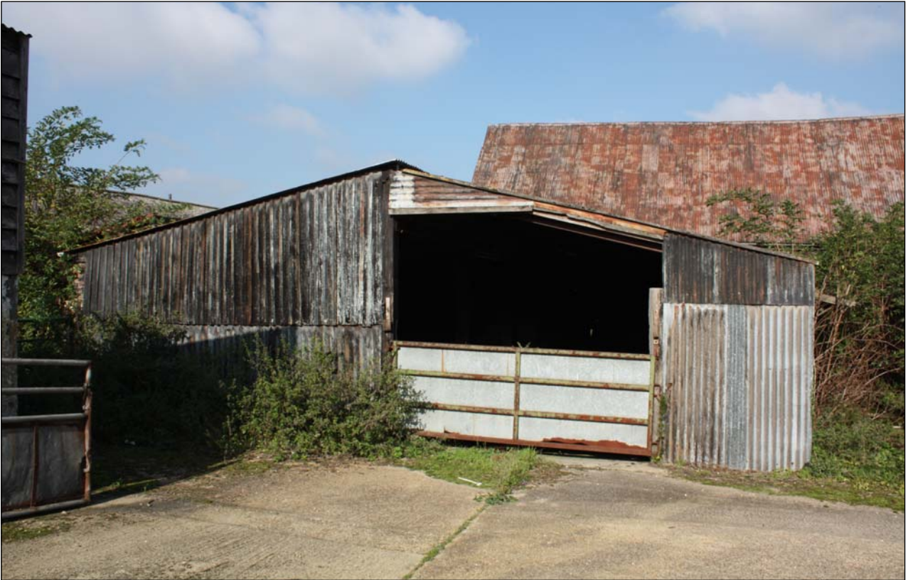
Plate 37: Building 9, viewed from south-east
