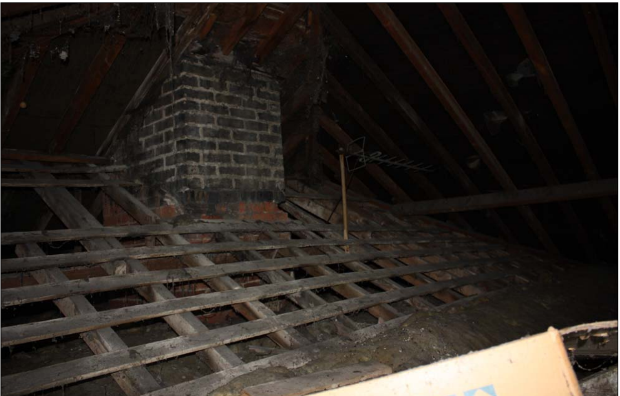
Plate 12: Building 1, Detail of early roof, viewed from inside attic
