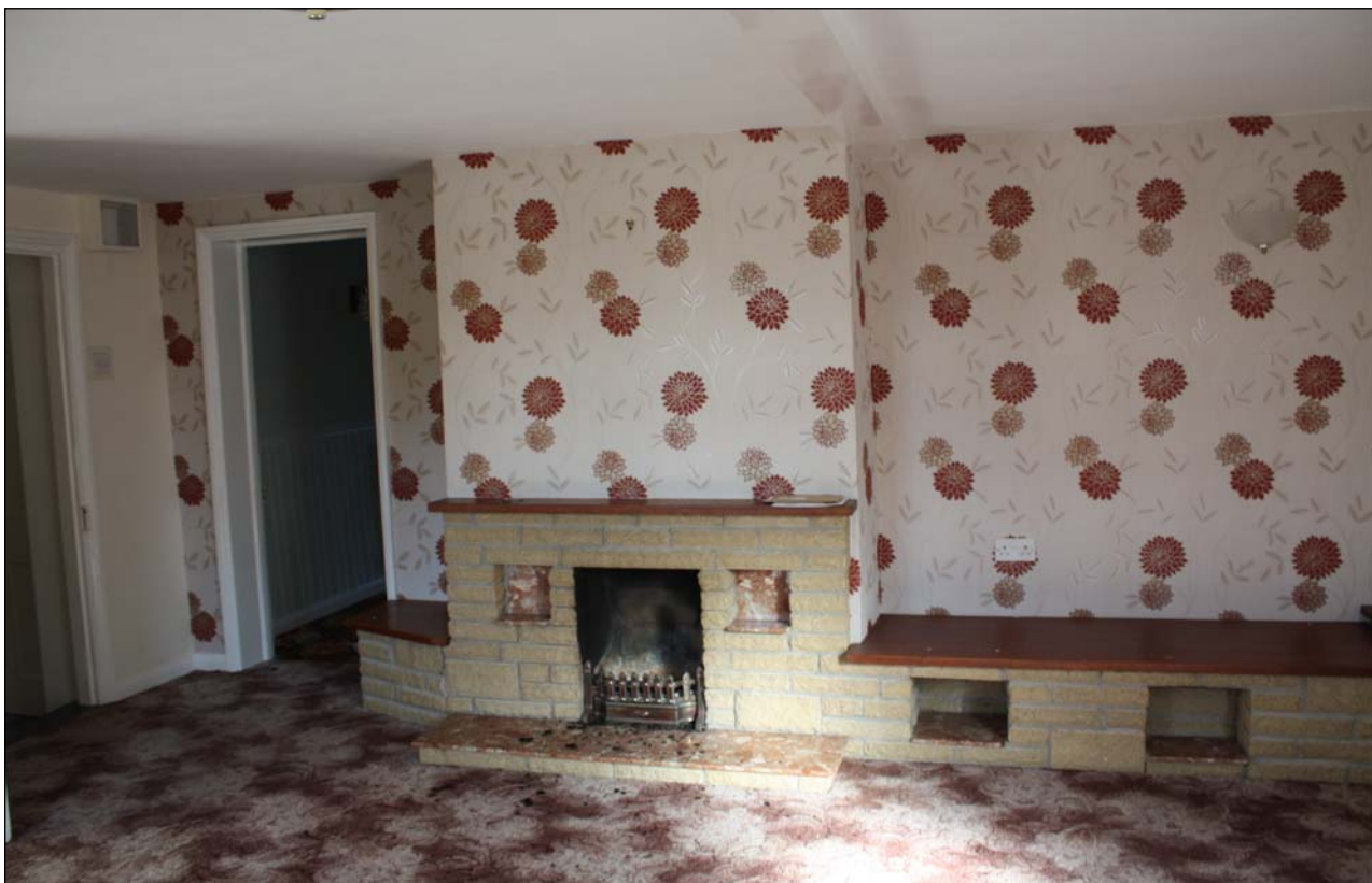
Plate 7: Building 1, Living room; G1
