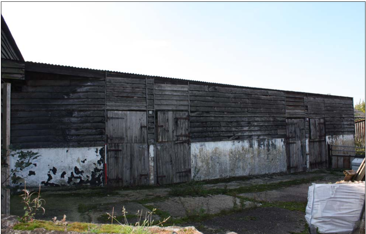
Plate 16: Building 3, viewed from east
