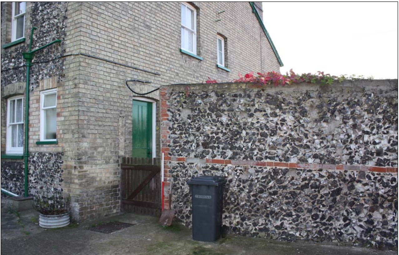
Plate 36: Flint wall and Building 1, viewed from east
