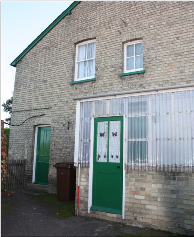
Plate 5: Building 1, Farmhouse, viewed from north-west
