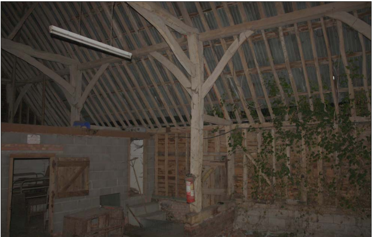
Plate 26: Building 5, Internal view of aisled posts and modern structure
