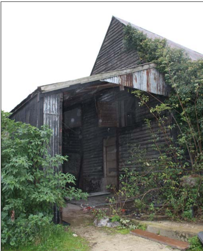
Plate 24: Building 5, gable end, viewed from north-east
