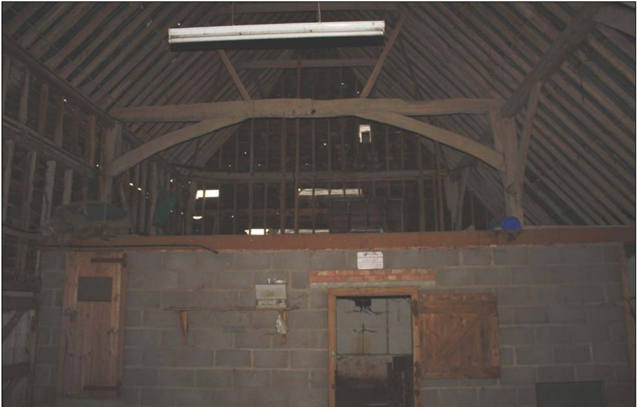
Plate 27: Building 5, Internal view showing roof structure and modern structure
