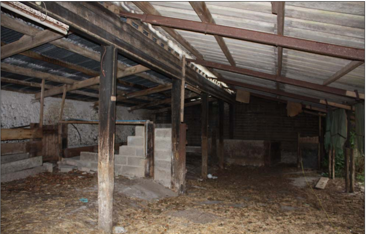
Plate 38: Building 9, internal view
