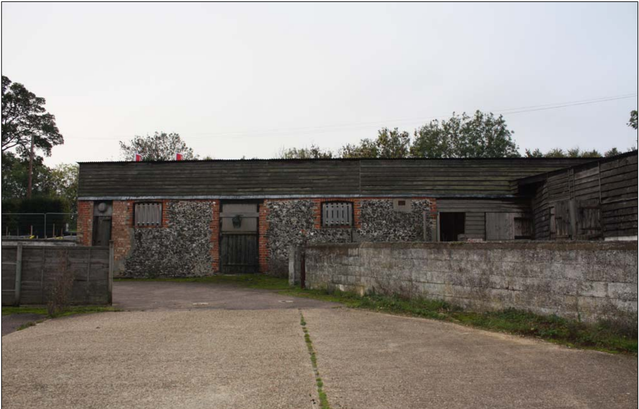
Plate 13: Building 2, Viewed from north
