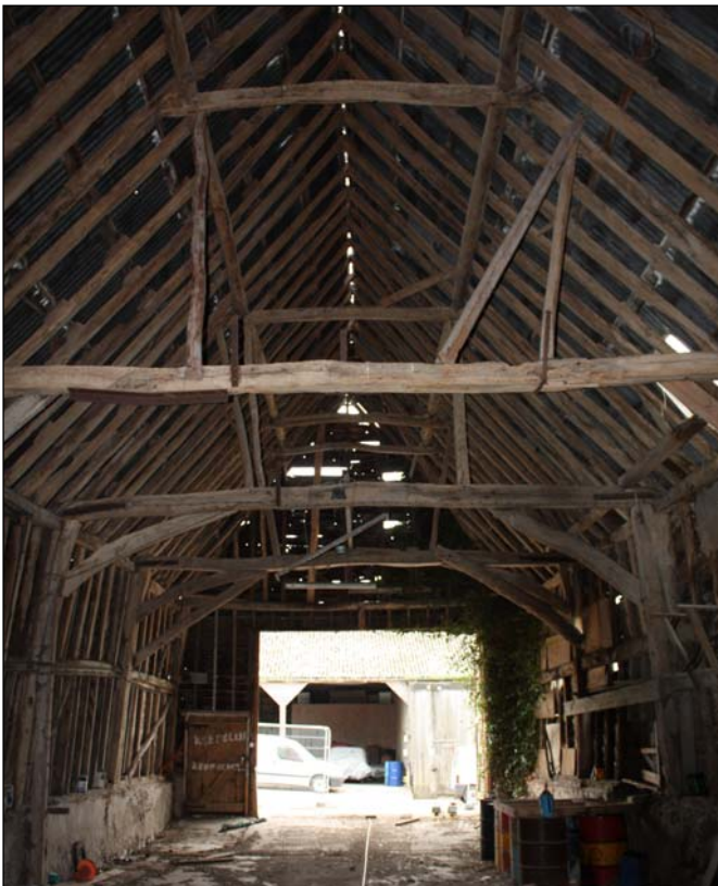
Plate 22: Building 4, Internal view
