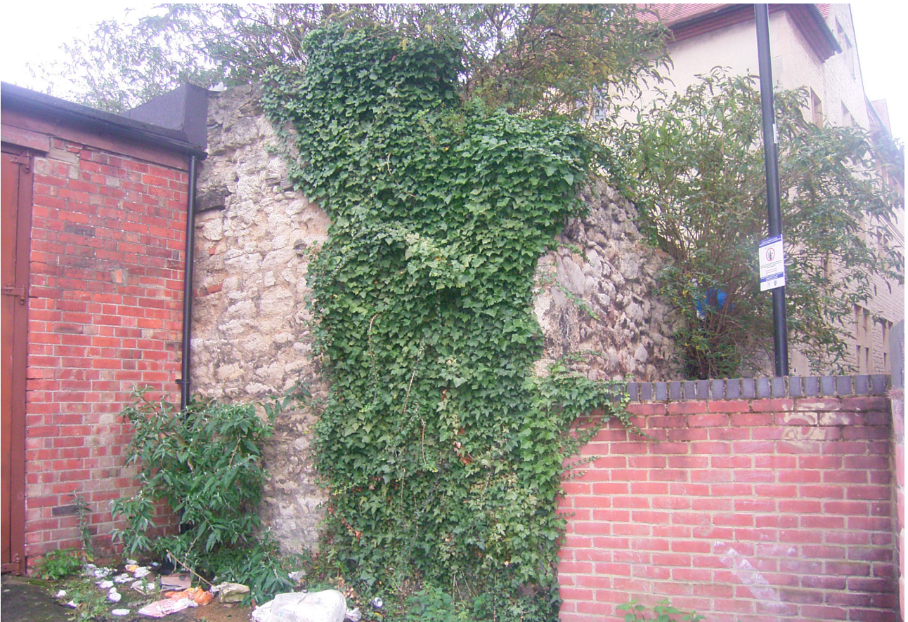
Plate 8: Surviving south-west corner from Malthouse on Rose Place (Wall 19)
