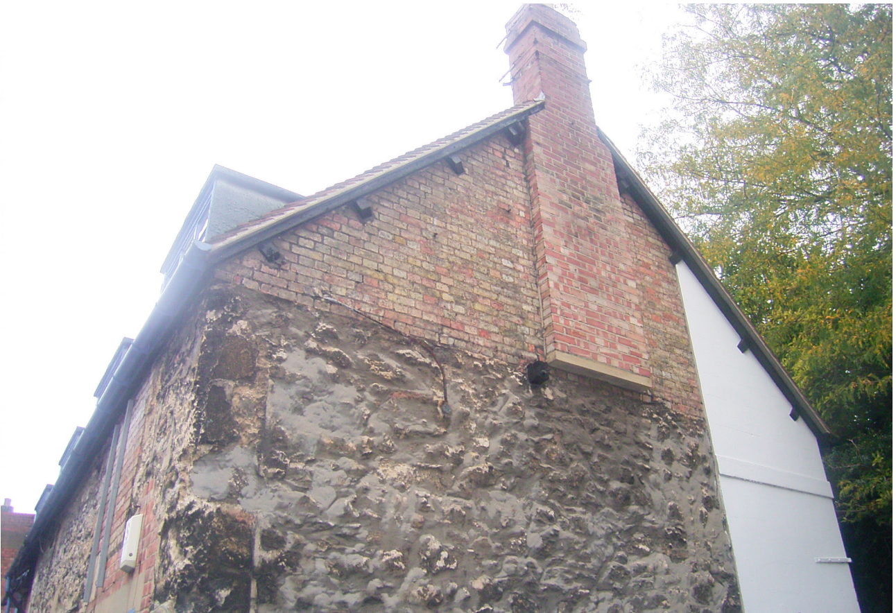
Plate 4: East gable of 6 Brewer Street (Wall 7)
