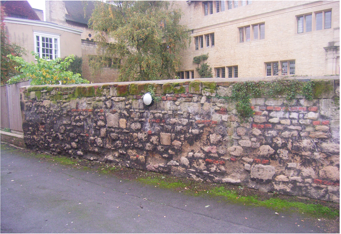
Plate 1: West side of Wall 1
