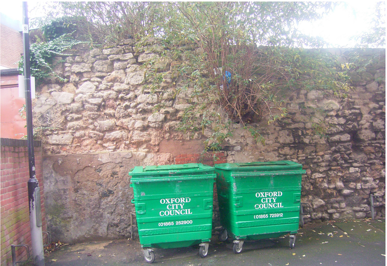
Plate 7: Surviving west end from south wall of former Malthouse on Rose Place (Wall 19)
