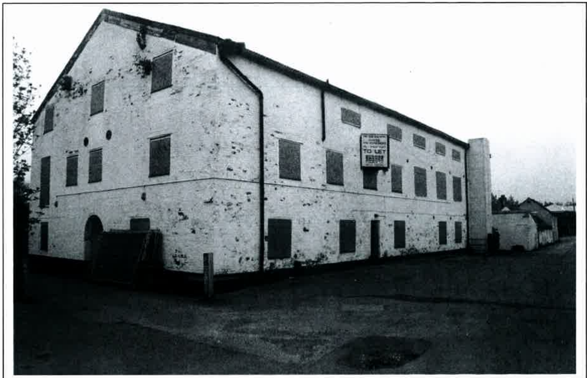
Plate 8. Block B: general view from south-west
