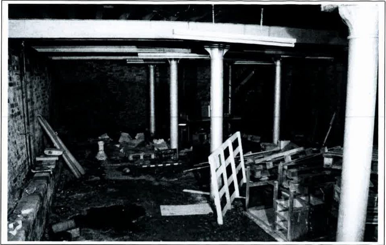
Plate 13. Block B: general view of cellar from west
