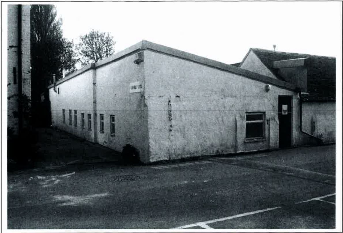
Plate 7. Block E: general view from north-west
