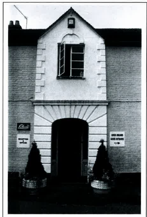
Plate 6. Block D: portico to east elevation
