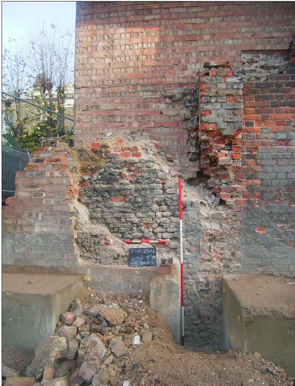
Plate 8: Wall 47 looking east
