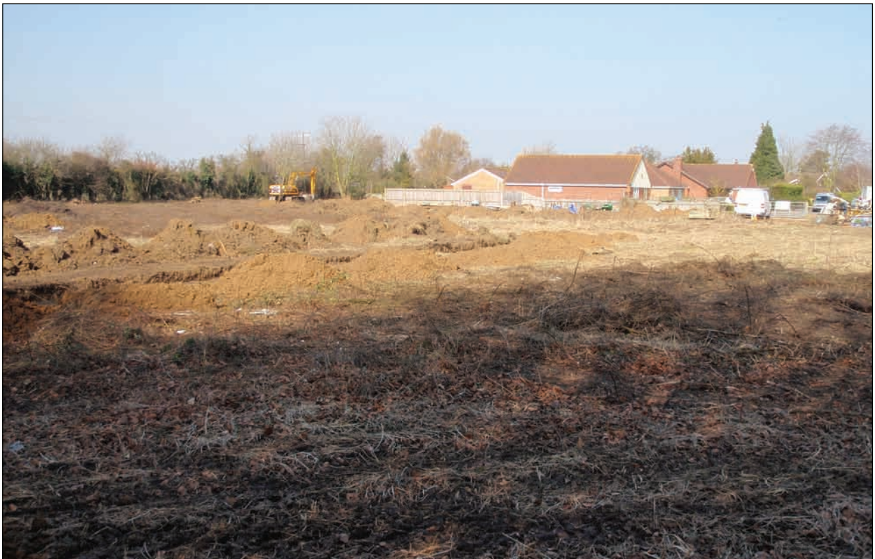
Plate 2: Working shot of site, looking northwest
