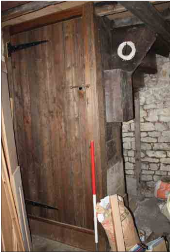
Plate 70: Access stairs to first floor, Building 1
