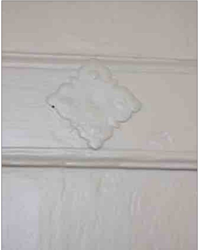
Plate 40: Backplate of a drop handle on F4 door as viewed from F5a
