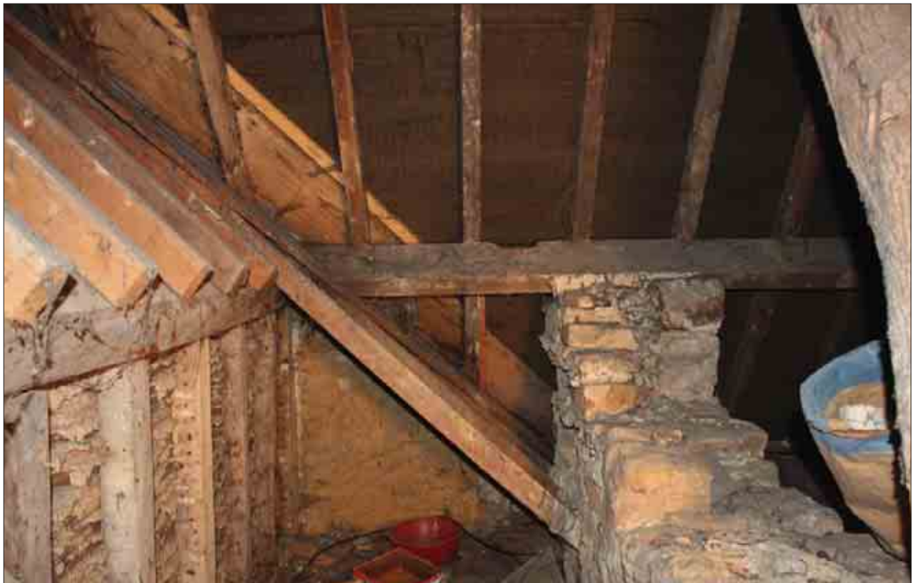
Plate 53: Original end wall as viewed from S4
