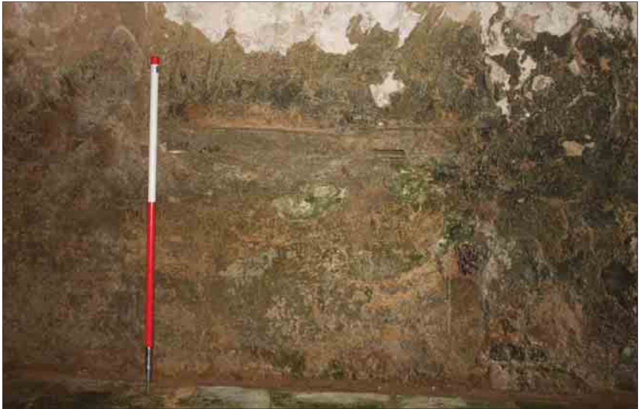
Plate 58: Blocked-up opening, C1
