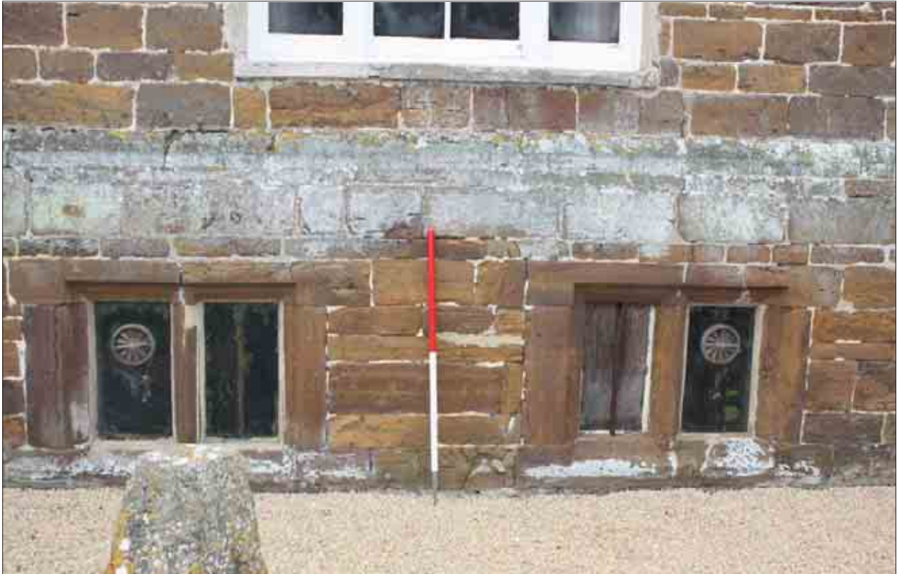
Plate 7: Detail of cellar windows on north-west facing elevation of farmhouse
