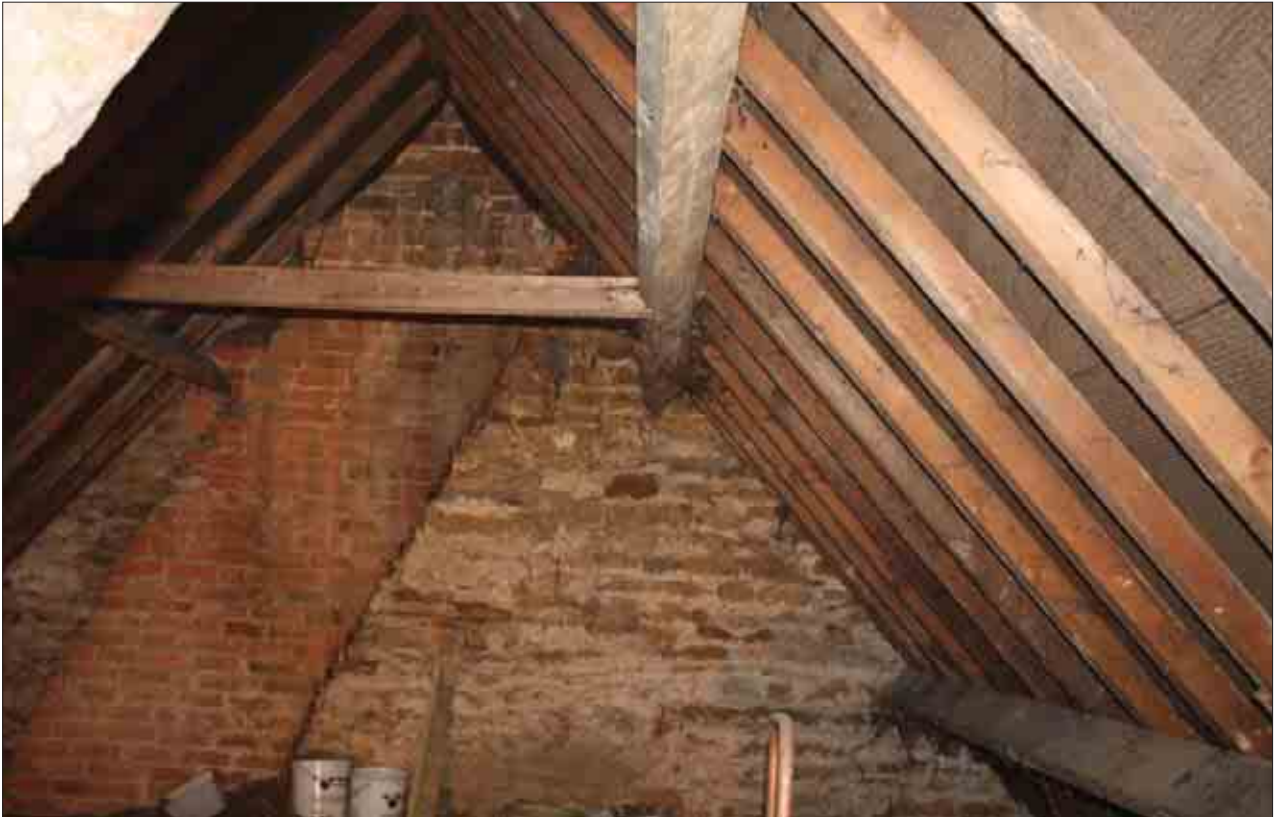
Plate 52: Detail of chimney within S4
