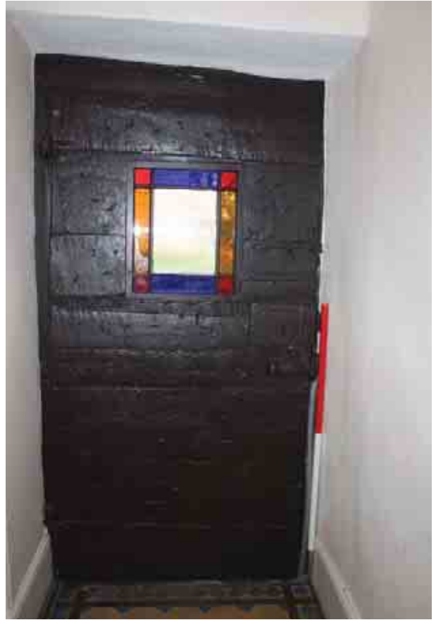
Plate 29: Internal view of north-west entrance door as viewed from corridor G6
