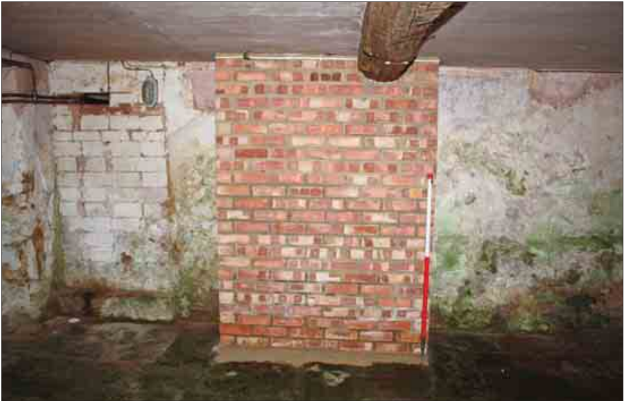
Plate 60: Blocked opening and 20th century structural support, C1
