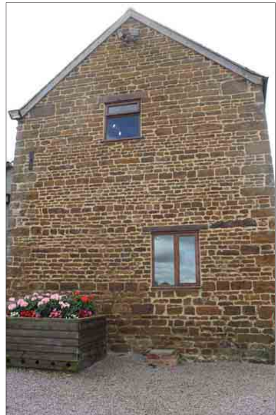
Plate 87: North-facing elevation, Building 3
