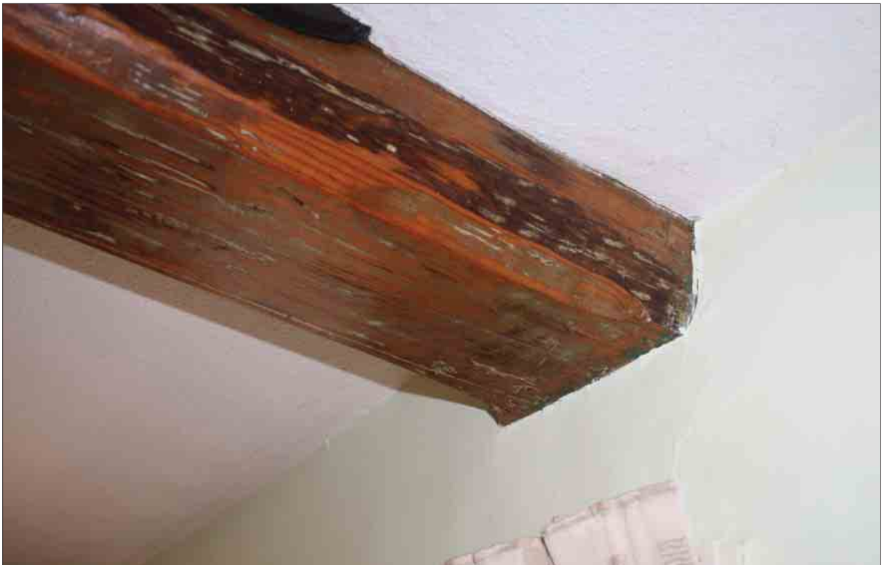
Plate 34: Detail of chamfered beam, F1
