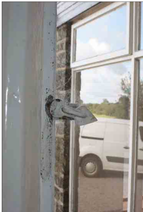
Plate 12: Late 17th century turnbuckle catch on window, G1
