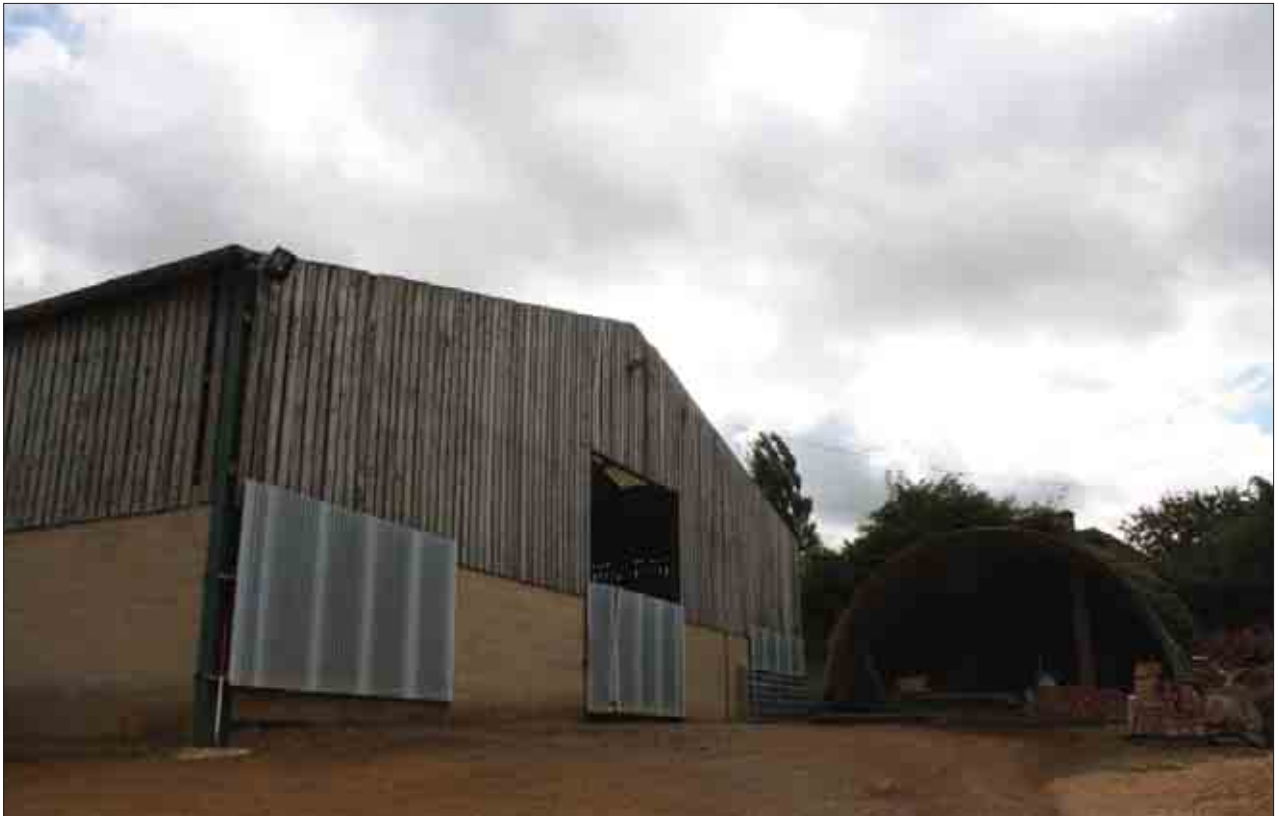
Plate 103: Buildings 8 and 9 as viewed from north
