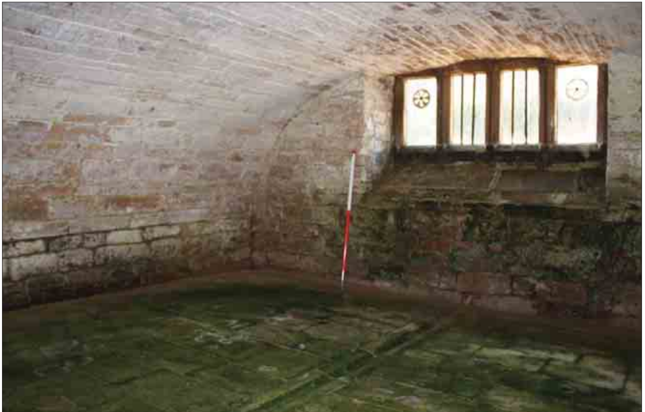
Plate 62: General room view, C2
