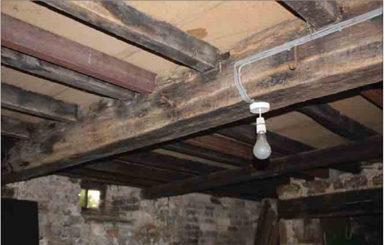
Plate 68: Ceiling beam and ceiling joists, G3, Building 1
