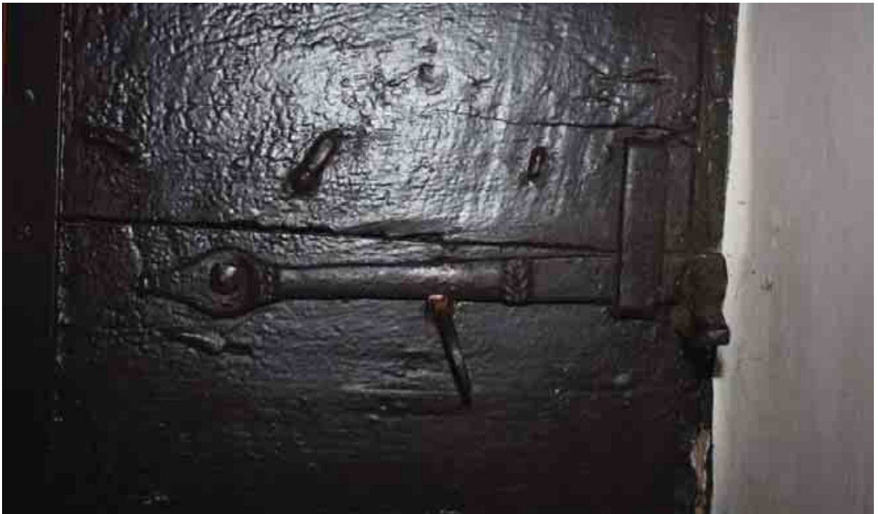
Plate 30: Detail of latch on inside of entrance door
