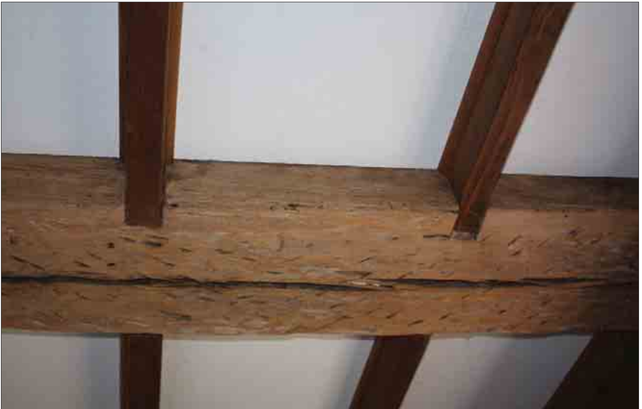
Plate 18: Detail of ceiling beam and replacement joists, G3
