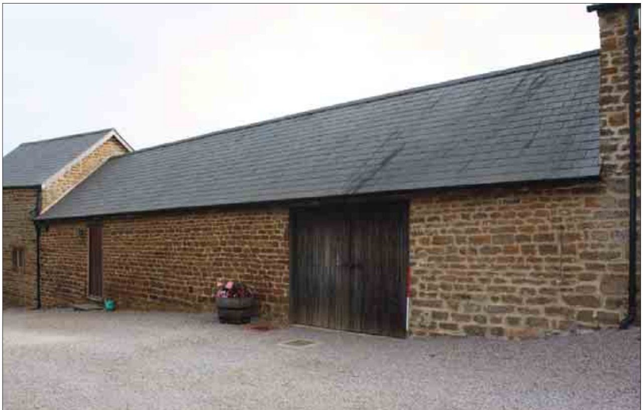
Plate 76: West-facing elevation, Building 2
