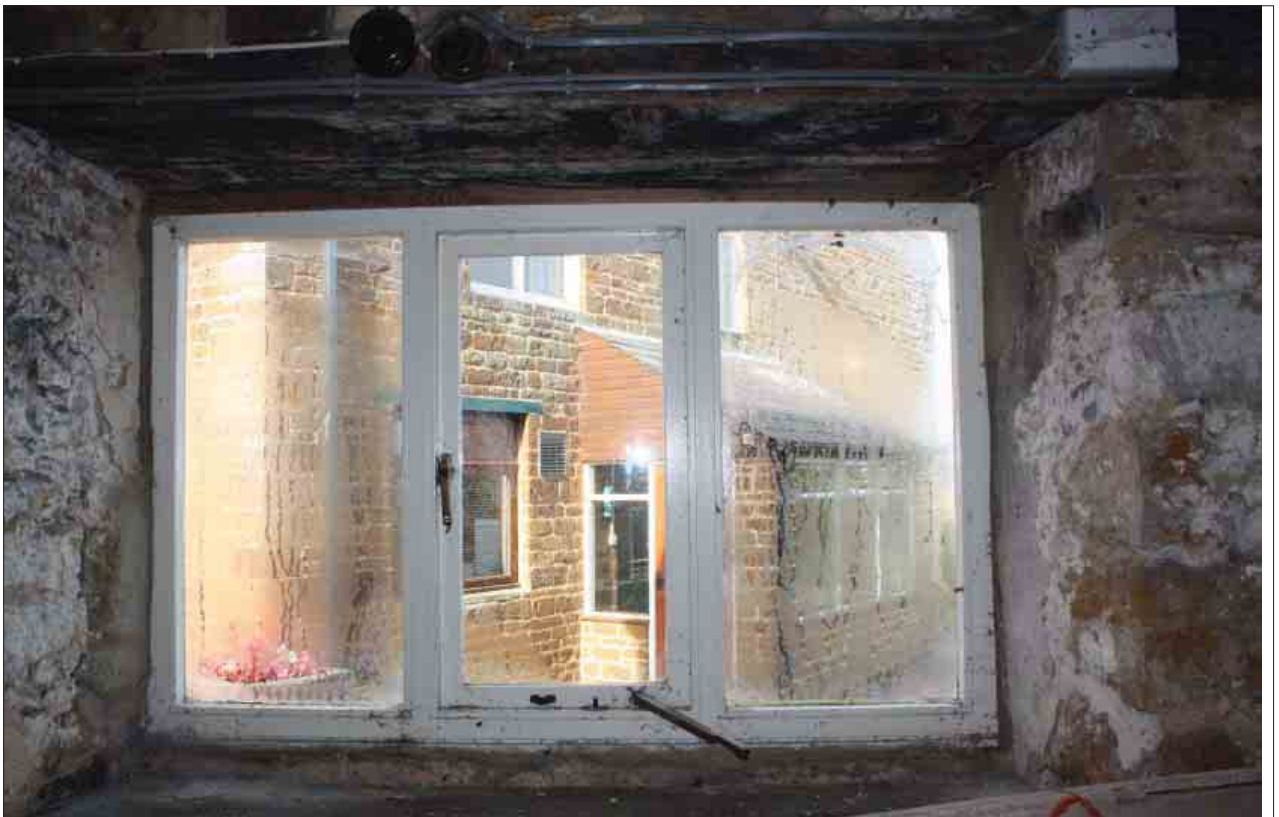
Plate 69: 20th century window, G3, Building 1
