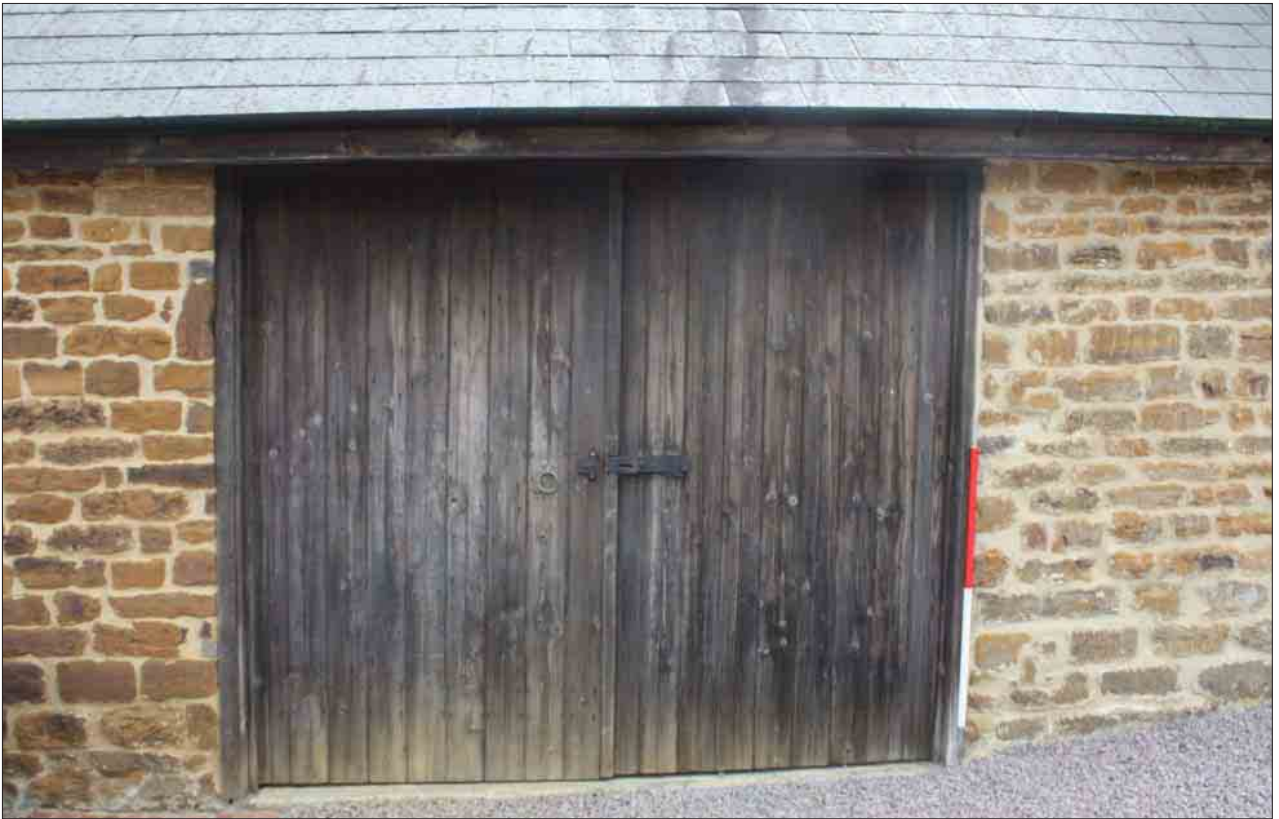
Plate 77: “Cart-door” entrance, west-facing elevation, Building 2
