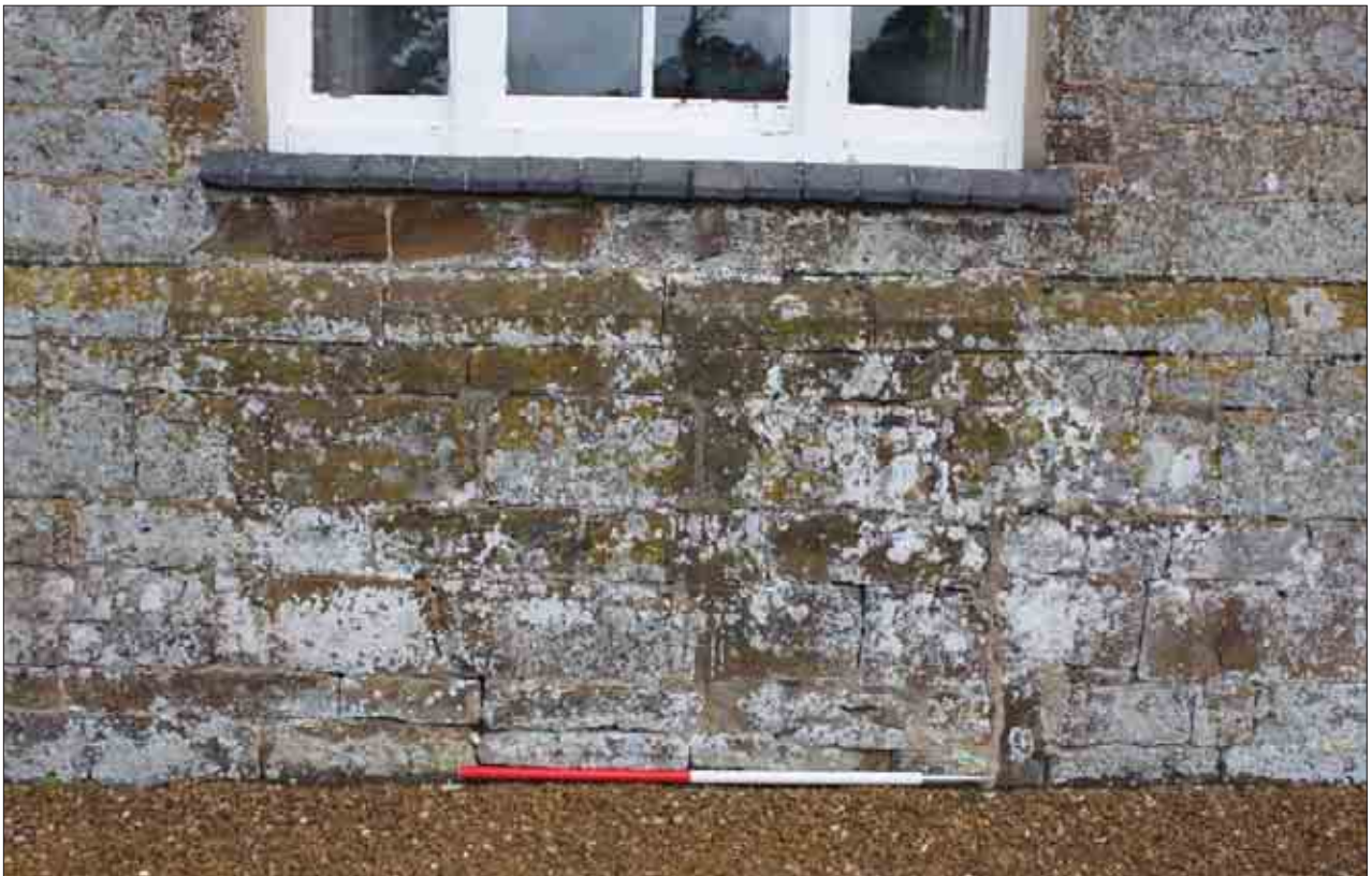
Plate 2: Blocked-up opening beneath window on south-west facing elevation of farmhouse
