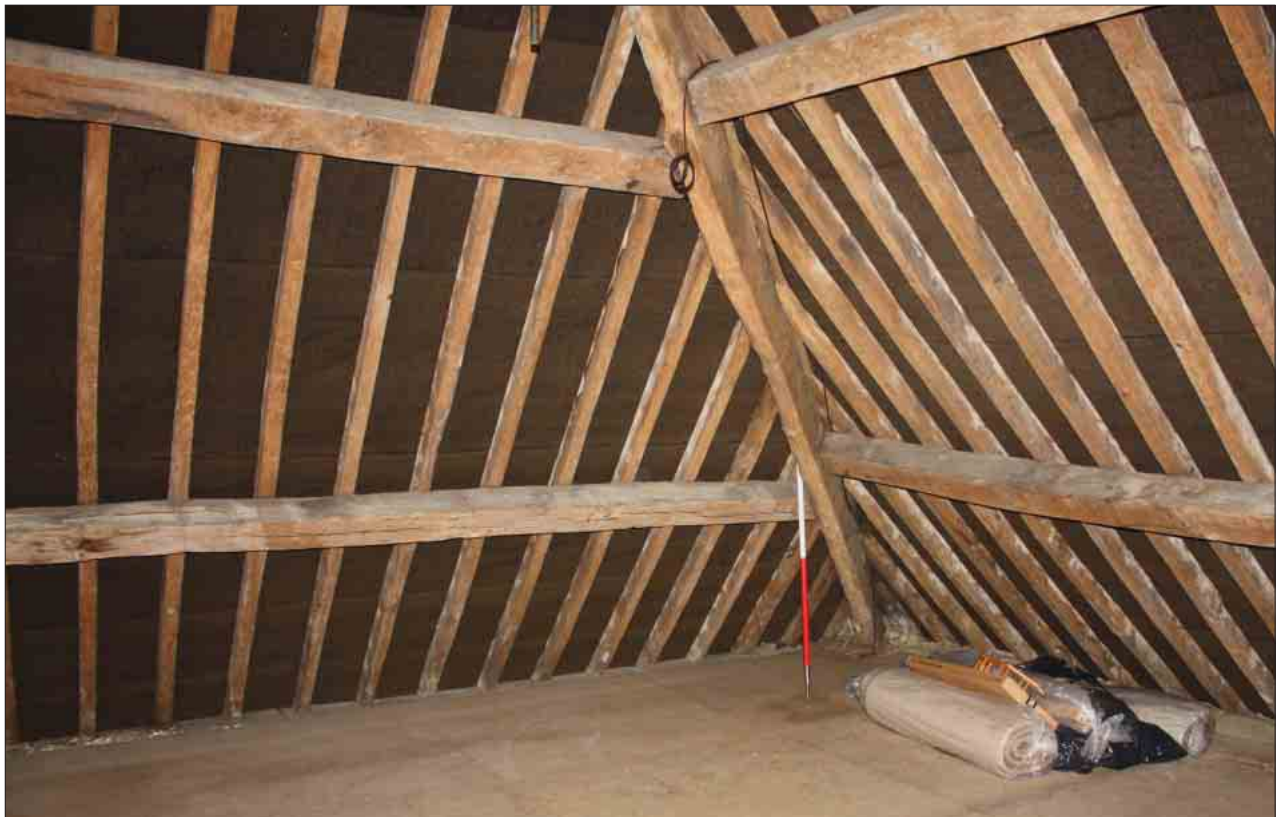
Plate 49: Purlins and common rafters, S2
