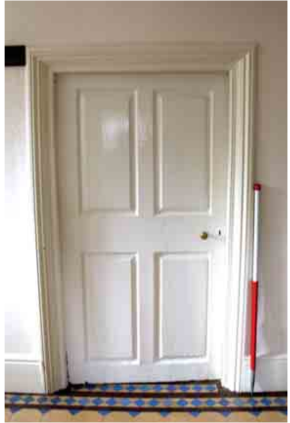
Plate 22: Internal access door into G4 as viewed from corridor G6
