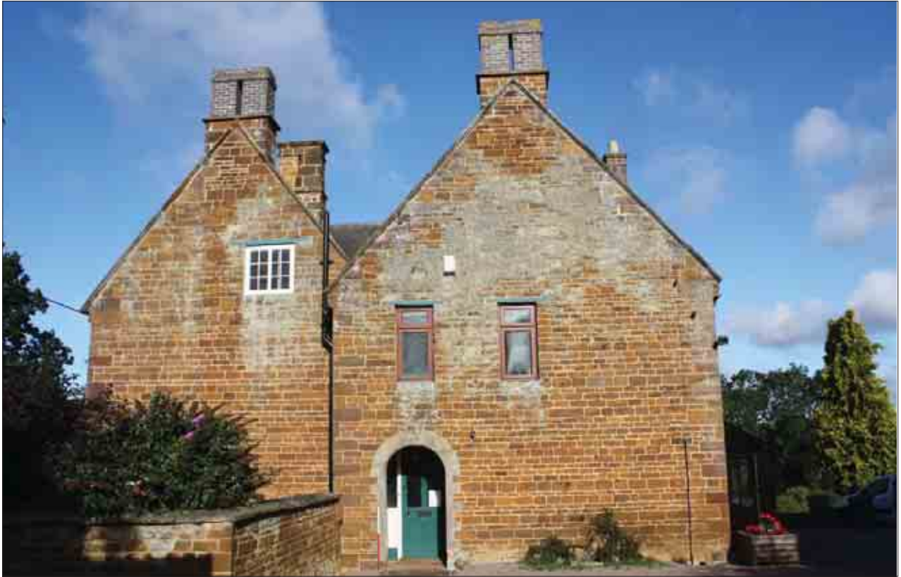
Plate 3: South-east facing elevation of farmhouse
