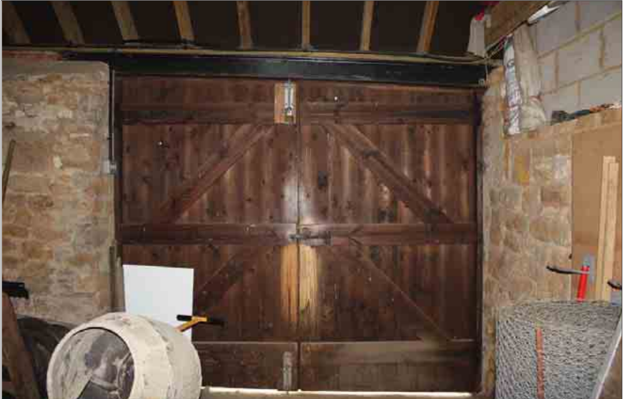
Plate 81: Interior view, G3, Building 2
