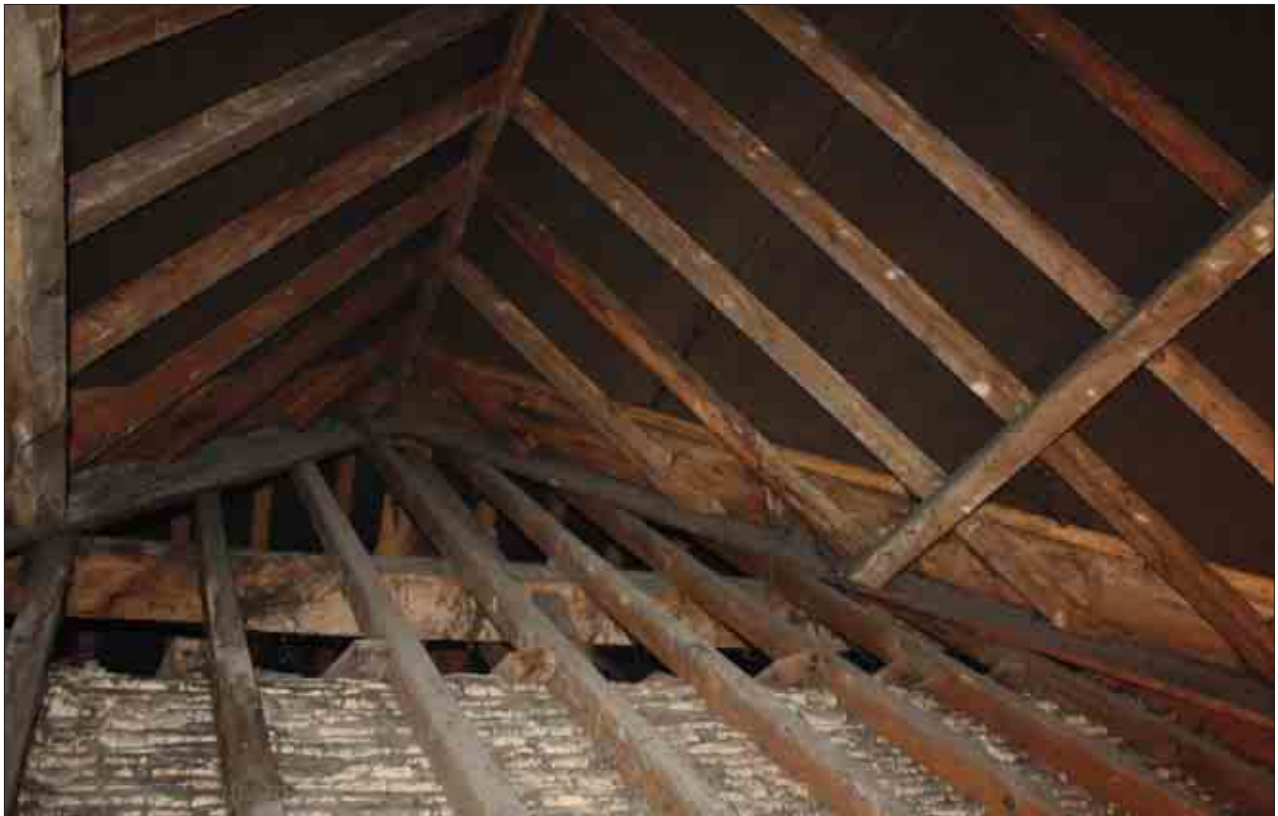
Plate 55: Remnants of original roof structure above S3 as viewed from S4
