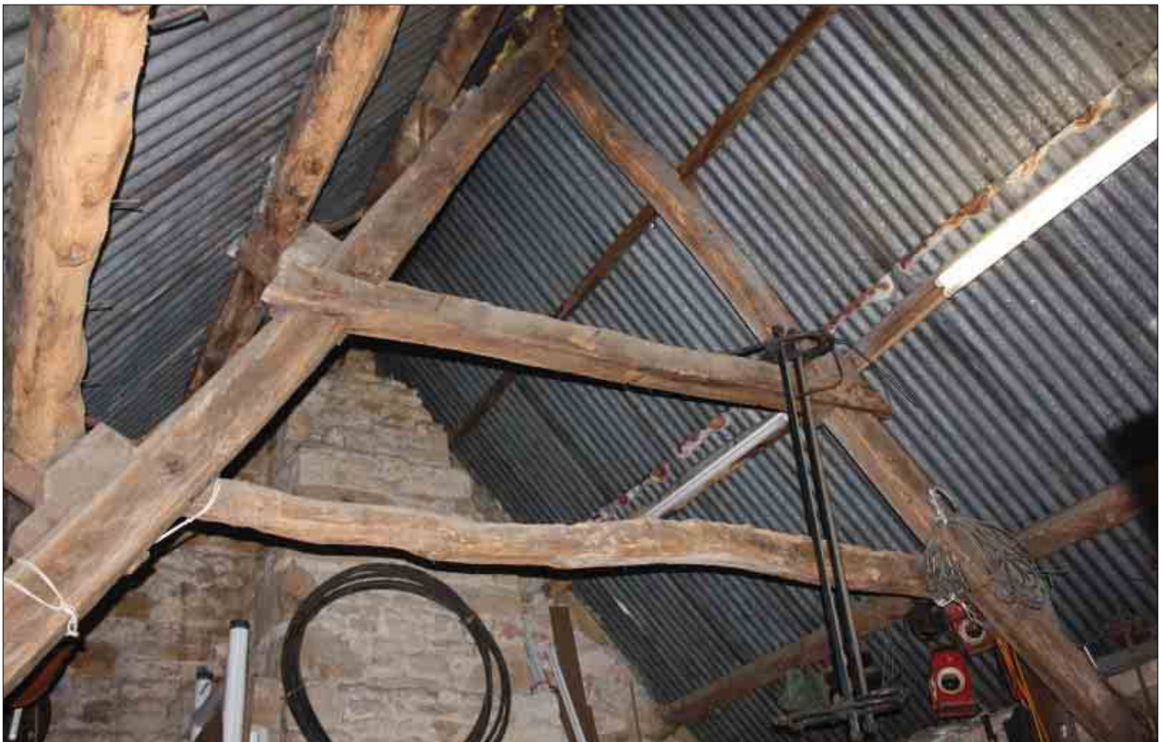
Plate 73: Roof structure and stone chimney, F1, Building 1
