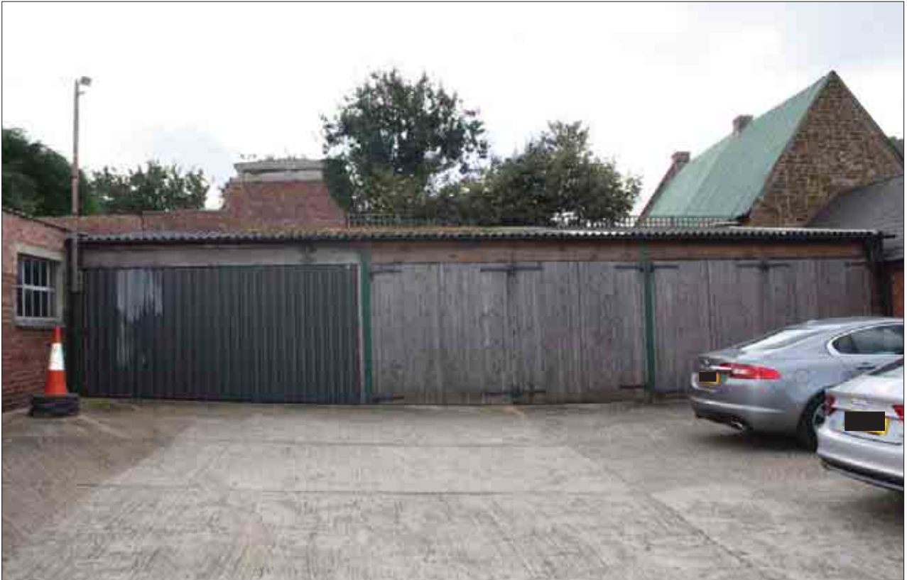
Plate 92: North-facing elevation, Building 4
