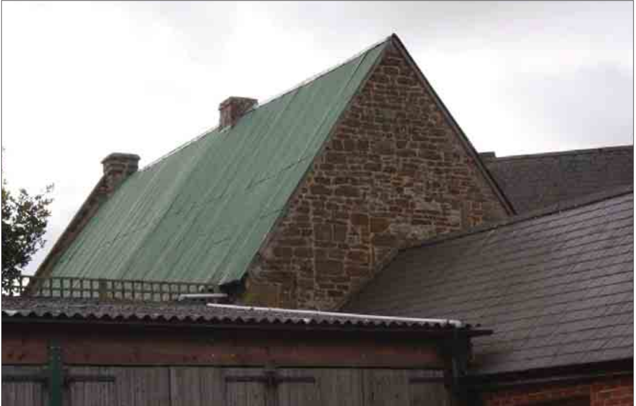
Plate 66: North-facing elevation, Building 1
