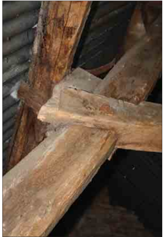
Plate 74: Carpenters mark on roof truss F2, Building 1
