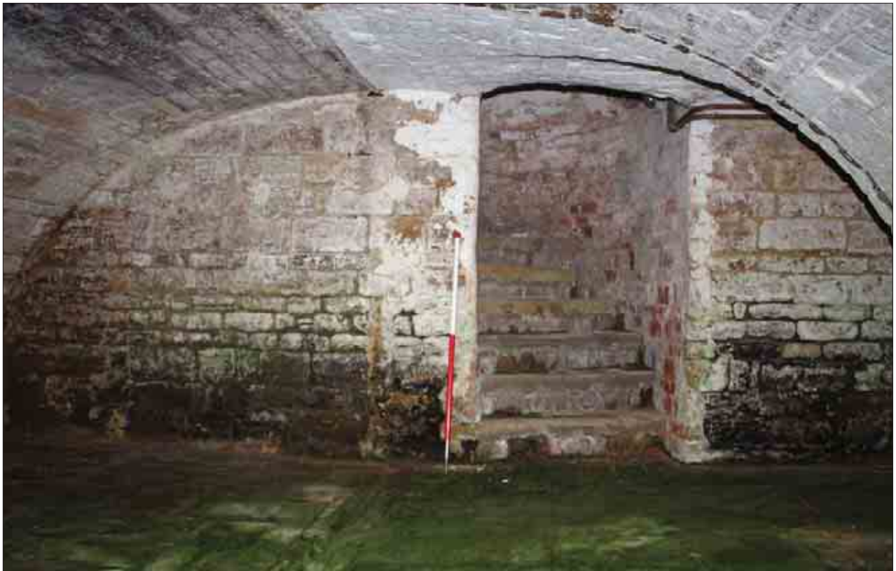
Plate 61: General room view, C2
