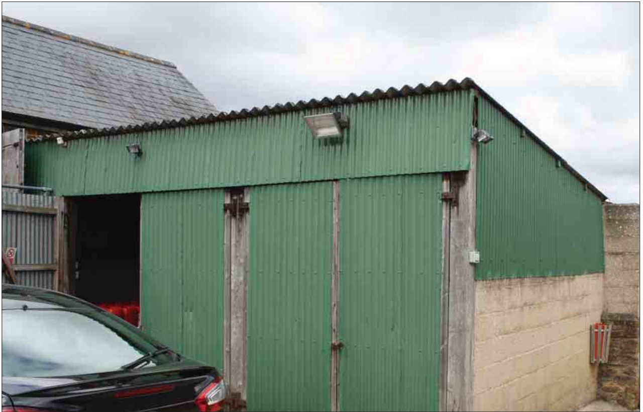
Plate 100: South-facing view, Building 6
