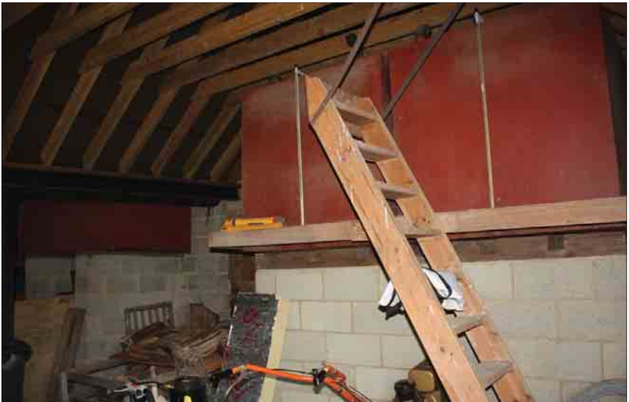
Plate 82: Modern breeze-block structure, walls and replacement roof, G3, Building 2
