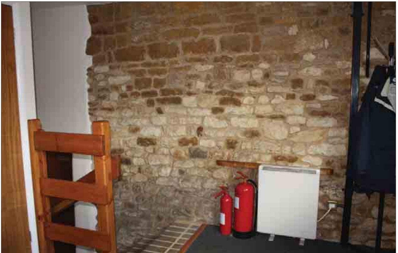
Plate 84: Exposed stone wall on northern wall, G7, Building 2
