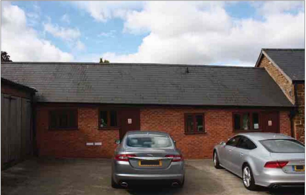
Plate 79: East-facing elevation, Building 2
