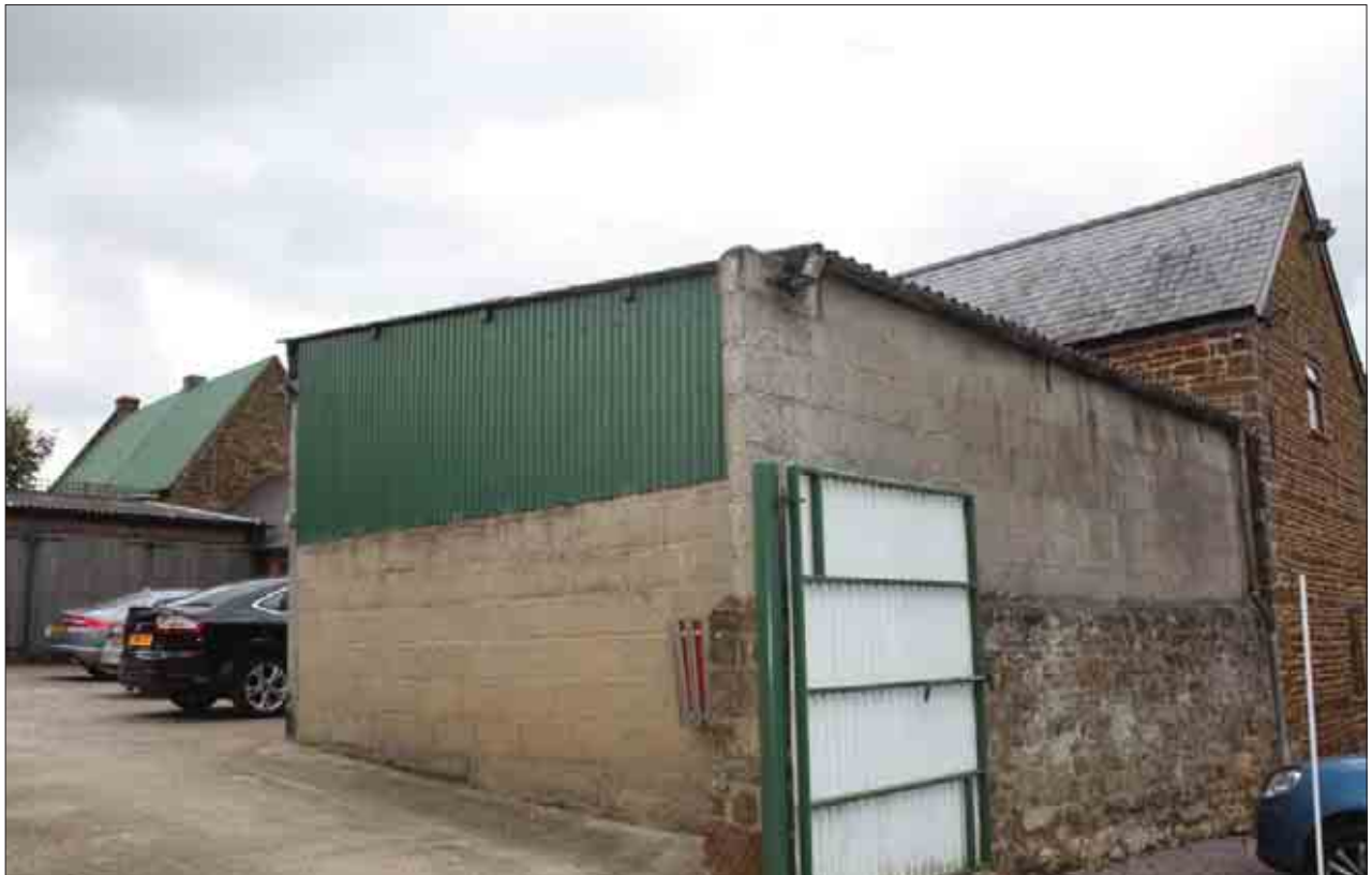
Plate 101: Building 6 as viewed from north-east
