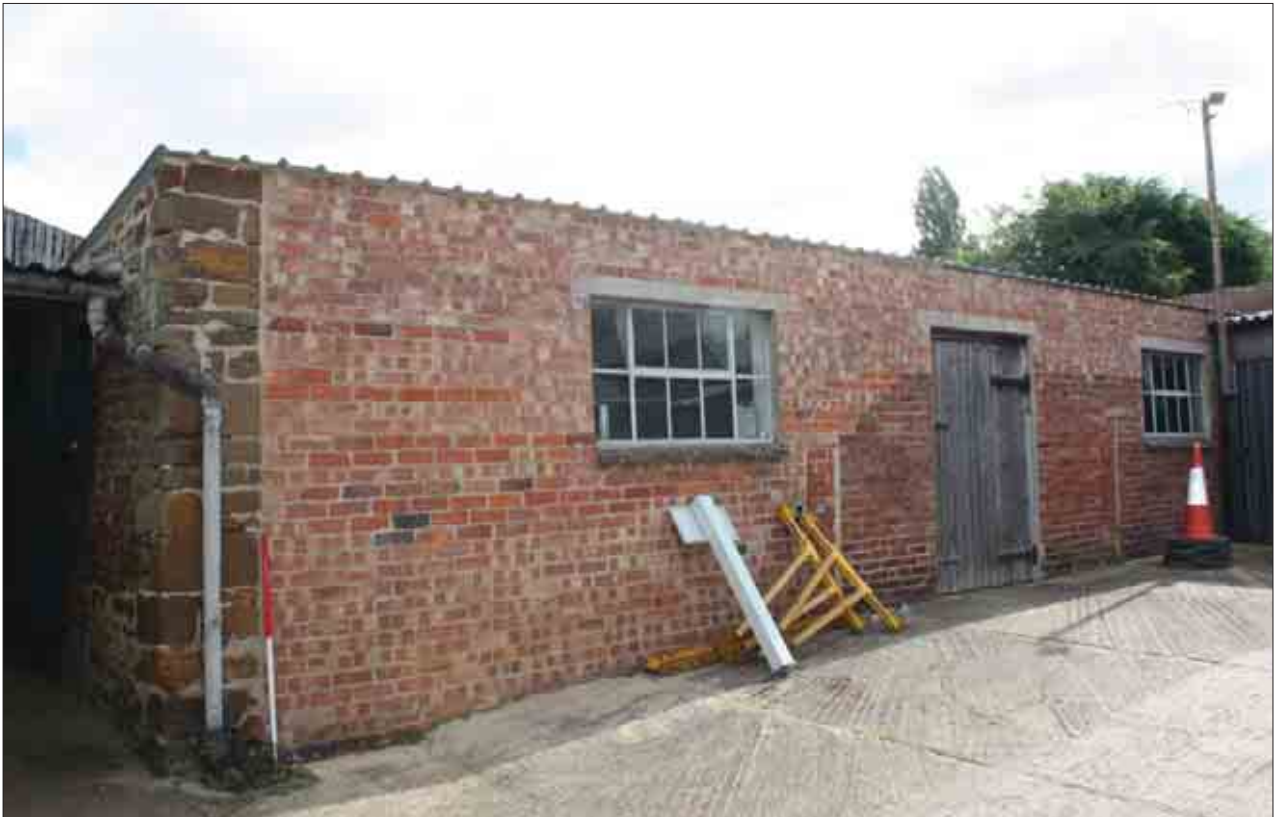
Plate 94: West-facing elevation, Building 5
