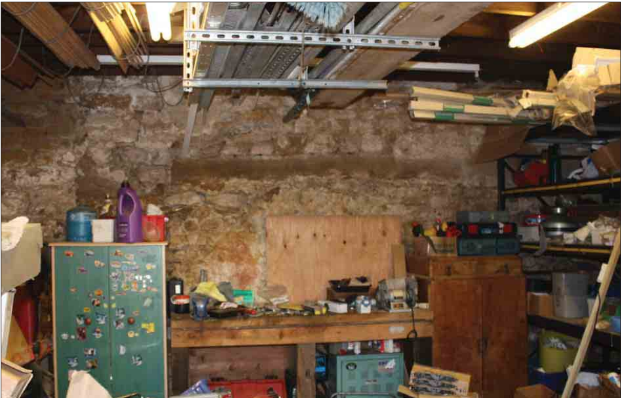
Plate 70: Lintel on rear wall, G4, Building 1
