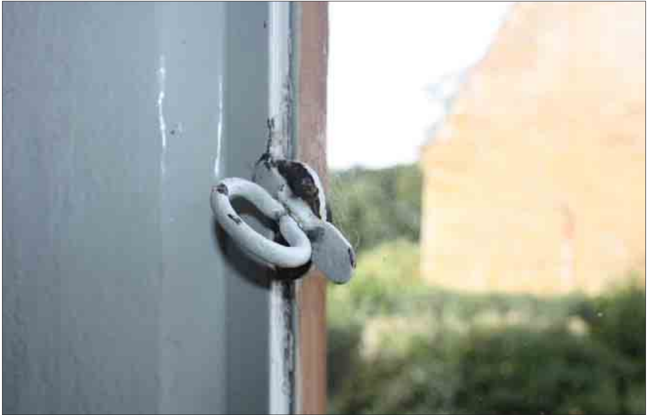
Plate 11: Late 17th century turnbuckle catch on window, G1
