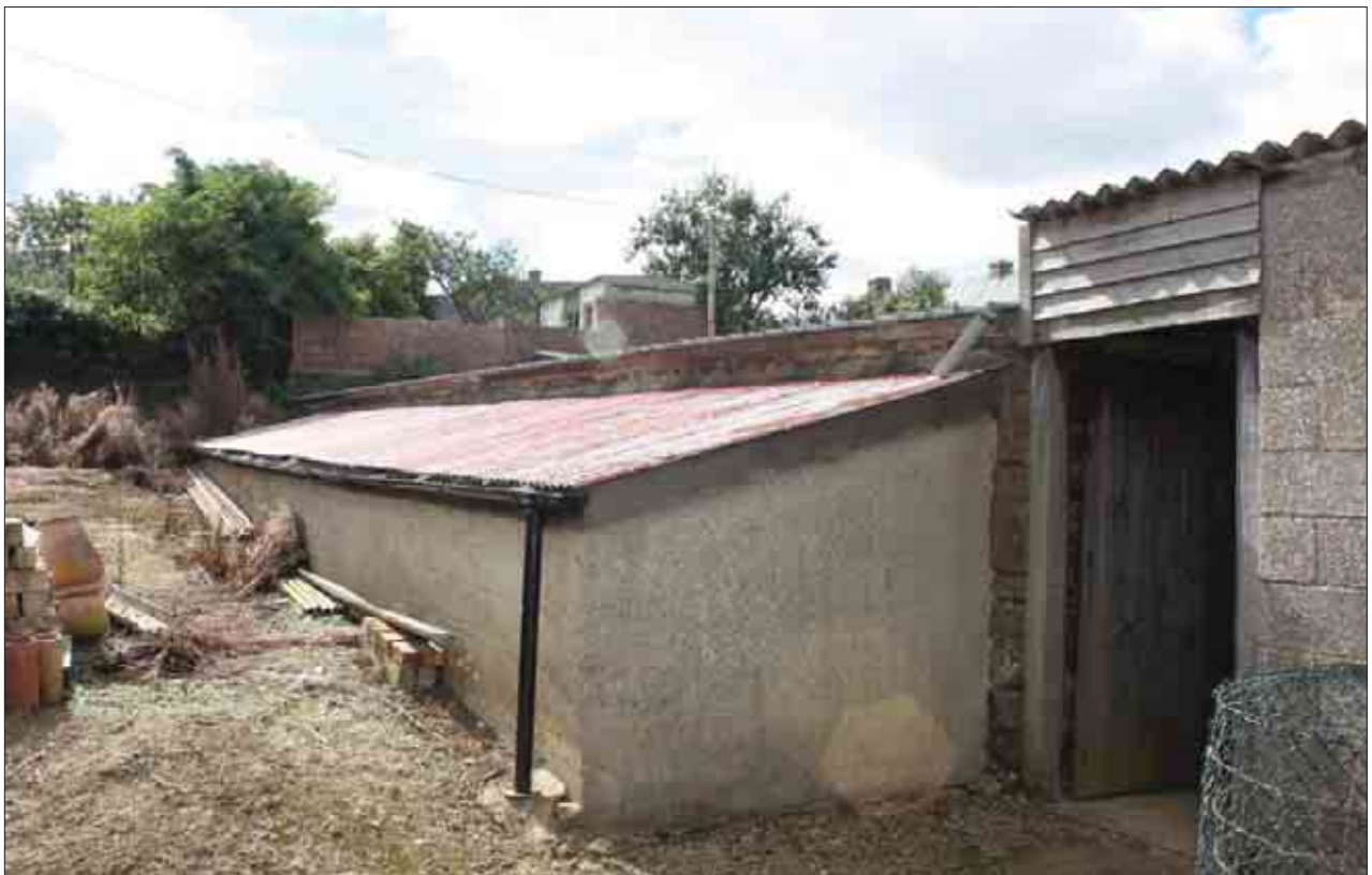
Plate 95: East-facing elevation, Building 5
