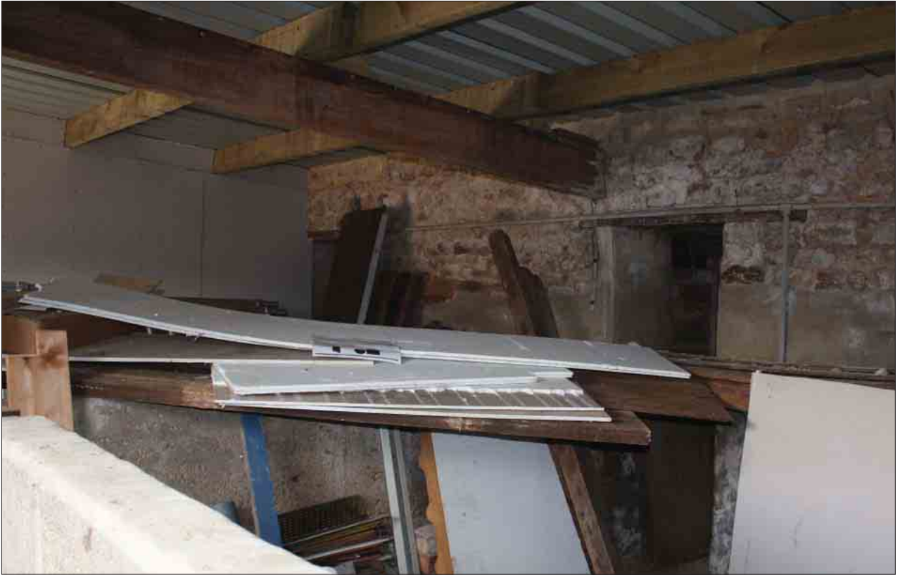
Plate 98: Detail of opening on rear wall, Building 5
