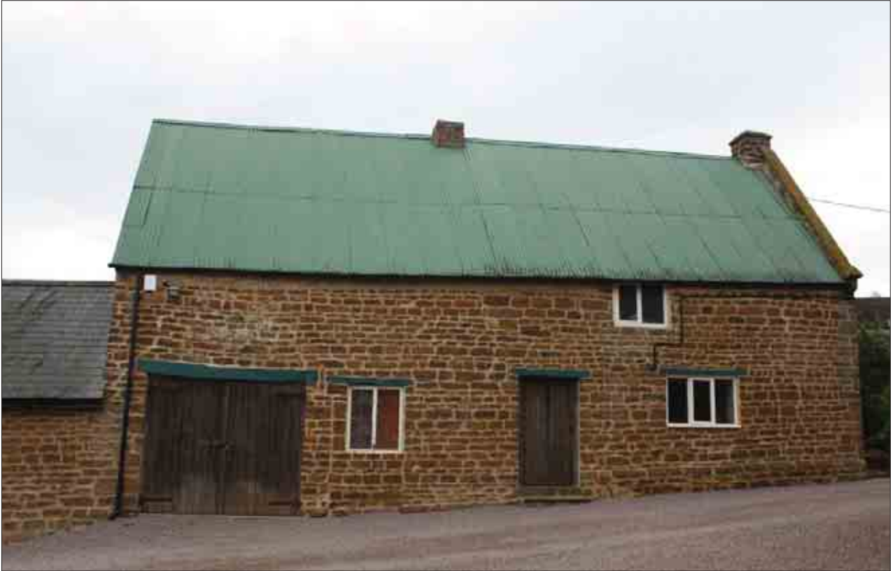
Plate 64: West-facing elevation, Building 1
