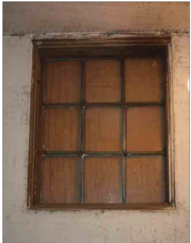
Plate 42: Interior "window" between F4 and F5b as viewed from F5b
