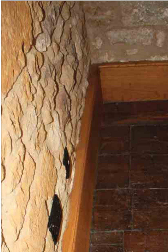
Plate 19: Floorboards in front of possible blocked opening, G3
