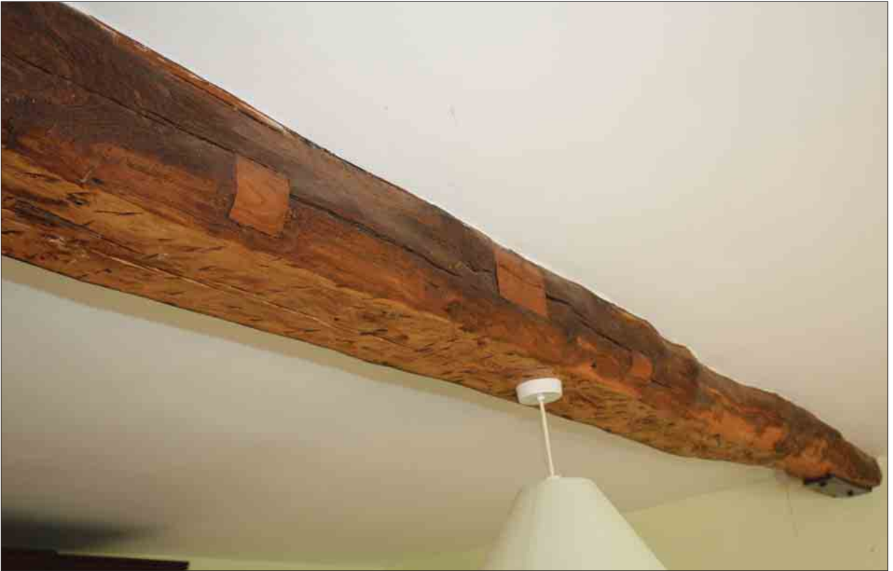
Plate 37: Detail of ceiling beam, F3
