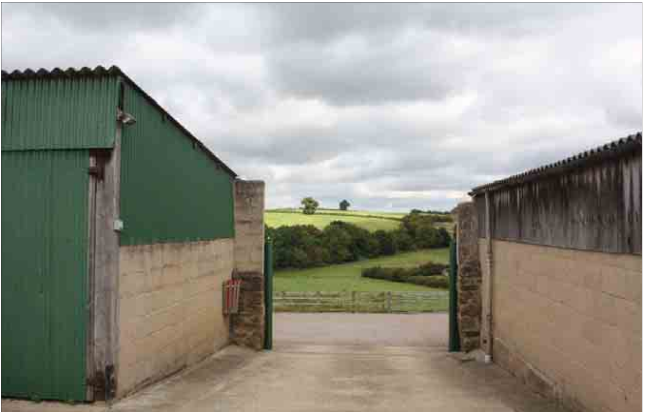
Plate 99: Entrance to courtyard looking northwards with Building 6 (left) and Building 7 (right)
