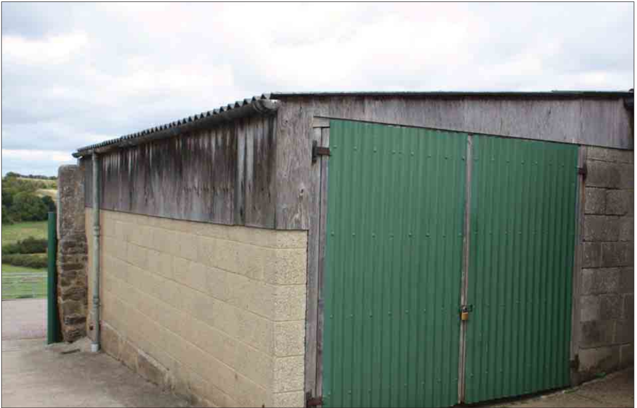
Plate 102: South-facing elevation, Building 7
