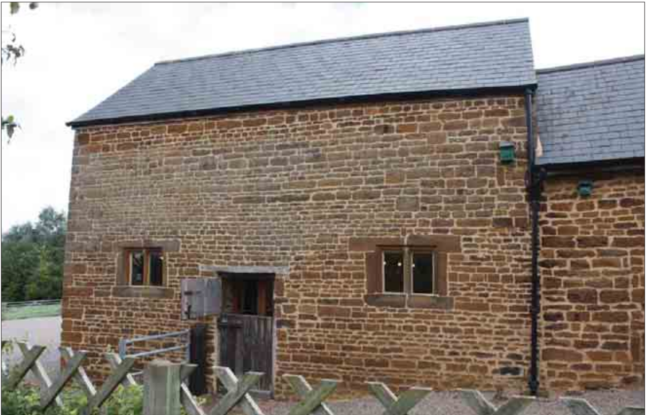
Plate 85: West-facing elevation, Building 3
