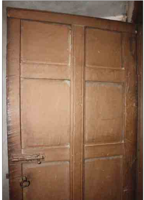
Plate 44: Door leading from F5b to attic
