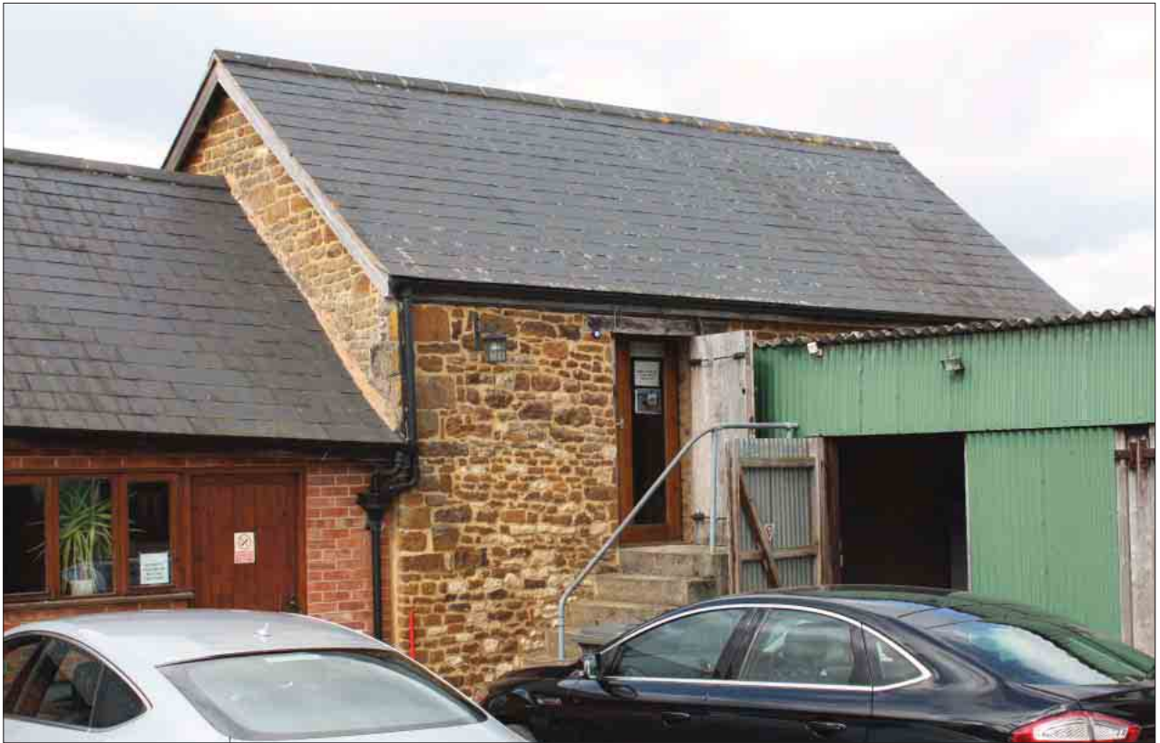
Plate 88: East-facing elevation, Building 3
