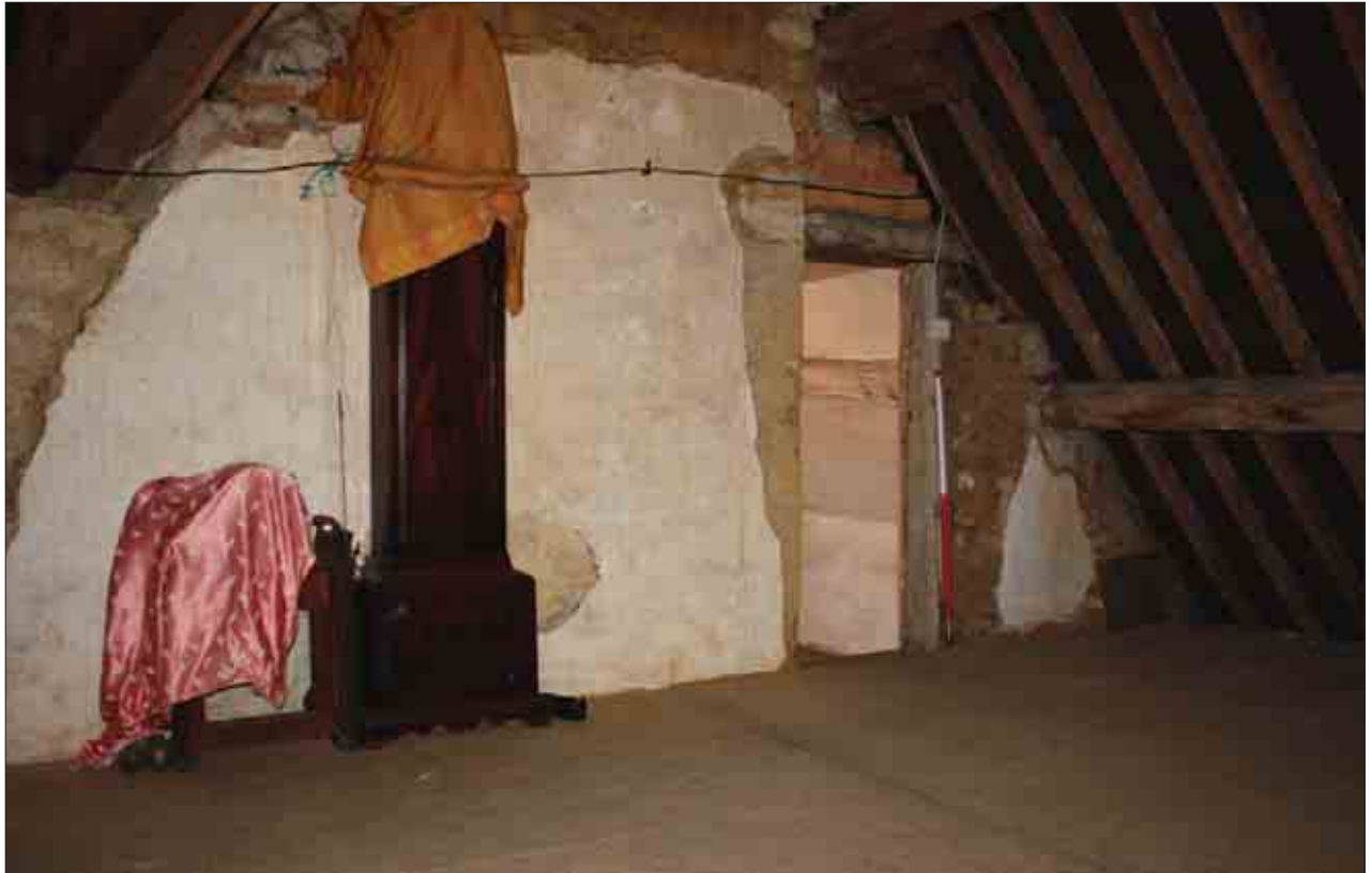
Plate 50: Rendered stone wall in S2
