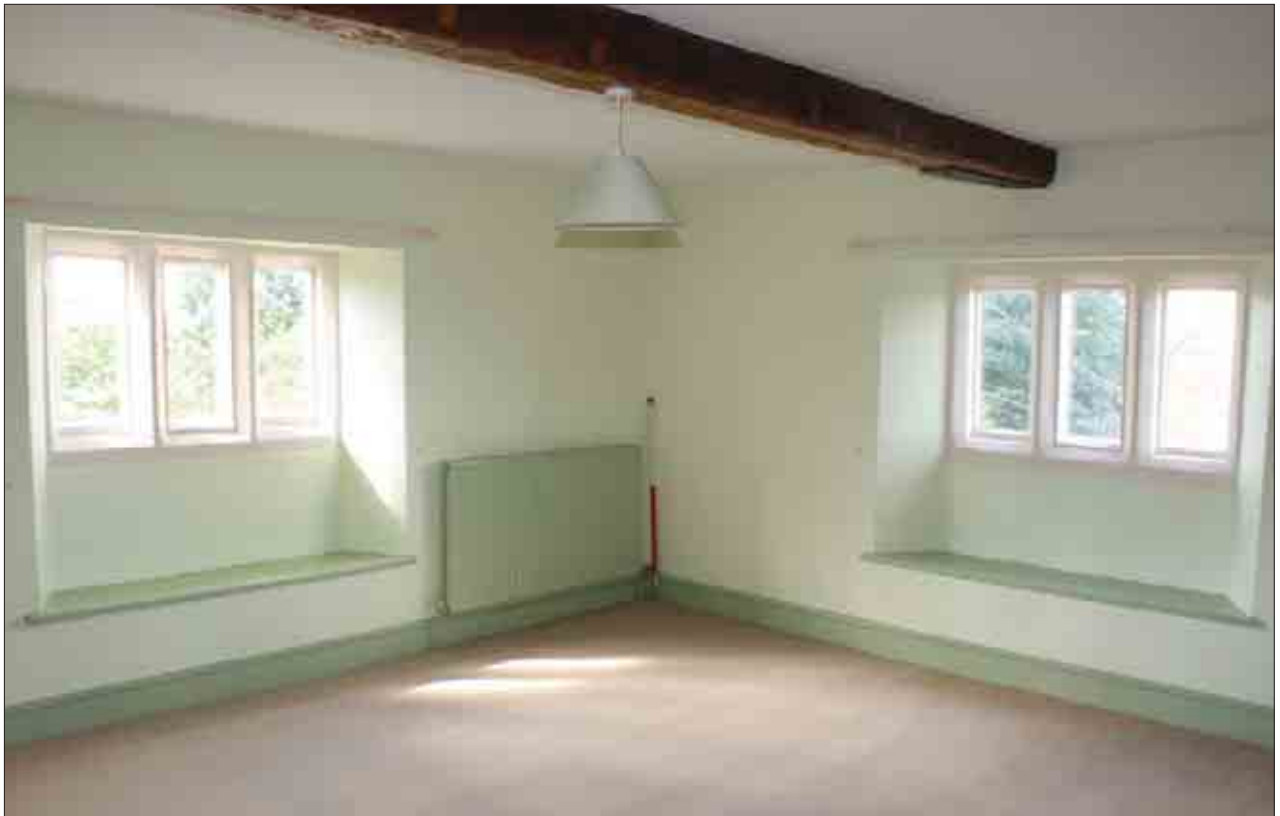
Plate 36: General room view, F3
