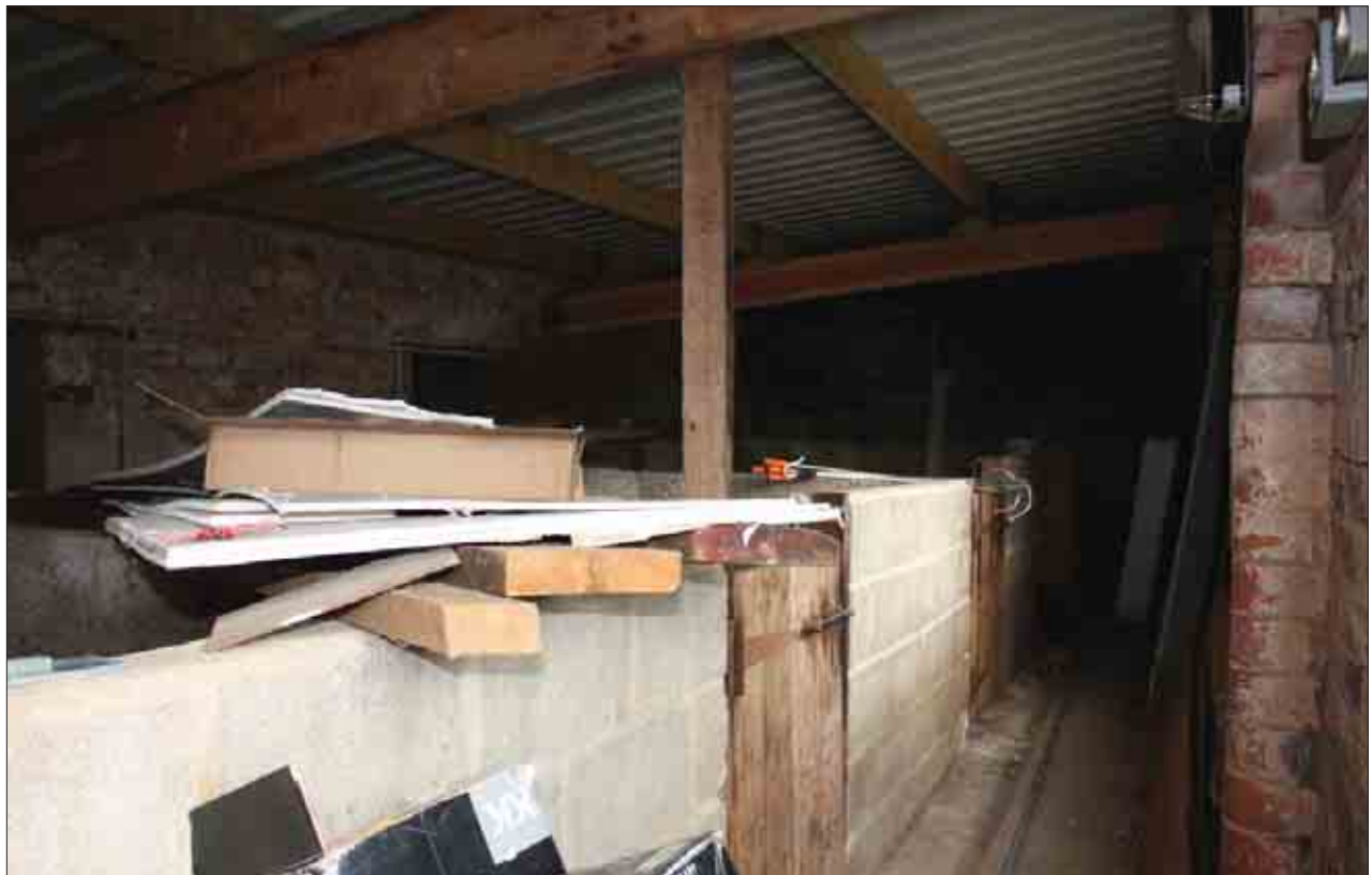
Plate 97: Internal view, Building 5
