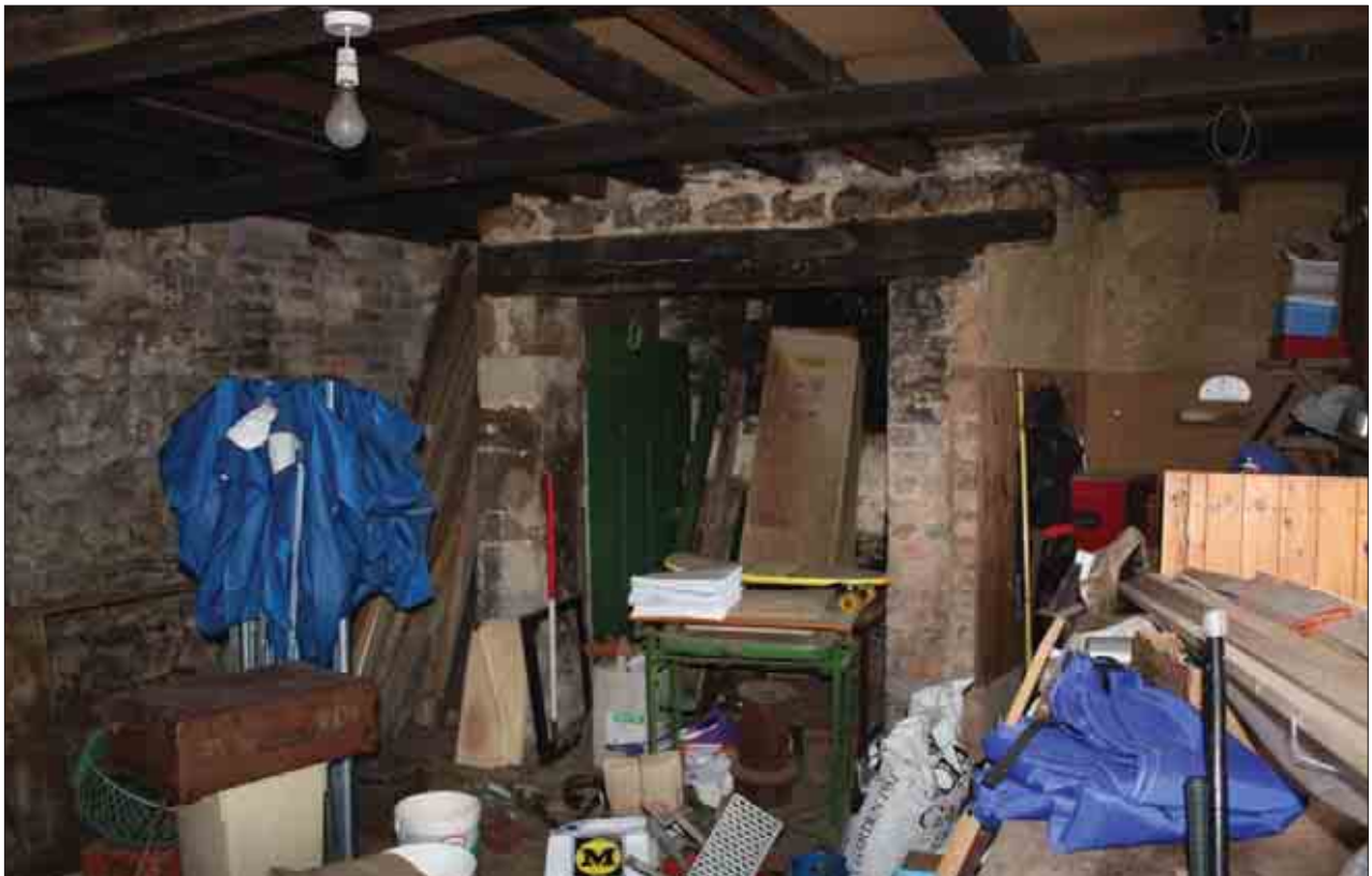
Plate 67: Internal view, G3, Building 1
