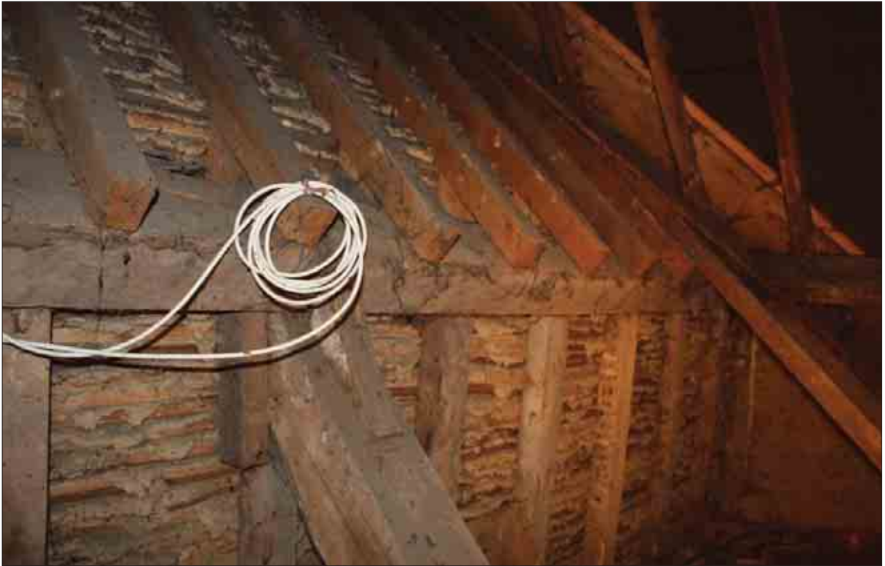
Plate 54: Detail of lath and plaster on outside of S3 as viewed from S4
