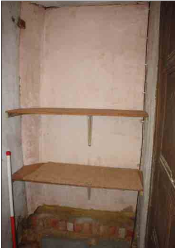
Plate 43: Position of blocked-up door, F5b
