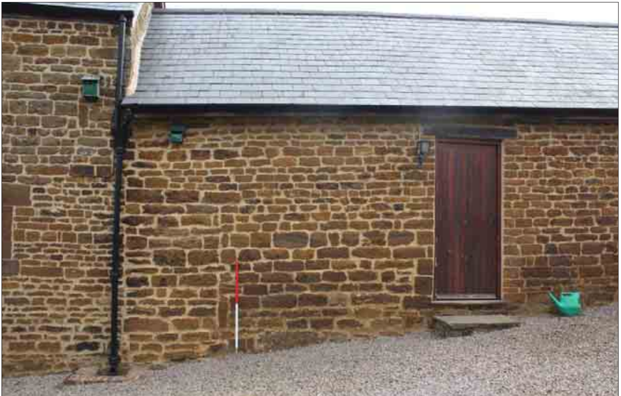
Plate 78: Blocked-up and modern doors, west-facing elevation, Building 2
