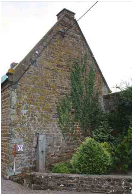
Plate 65: South-facing elevation, Building 1
