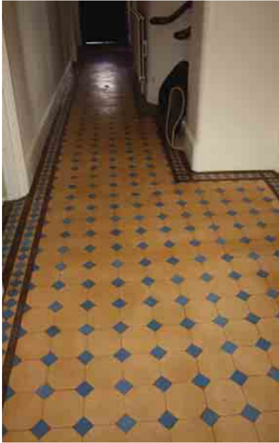
Plate 28: Tiled floor of corridor G6
