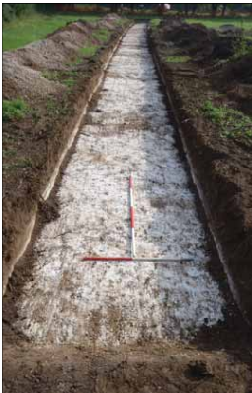
Plate 9: Trench 9 looking north east
