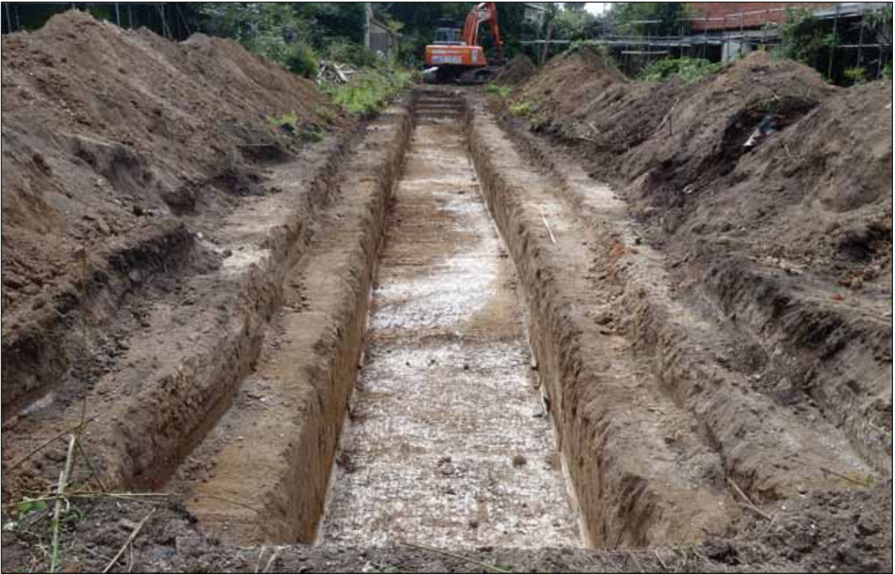
Plate 1: Trench 1 looking south west
