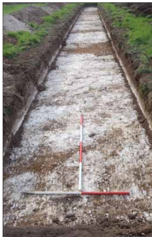
Plate 6: Trench 2 looking south east
