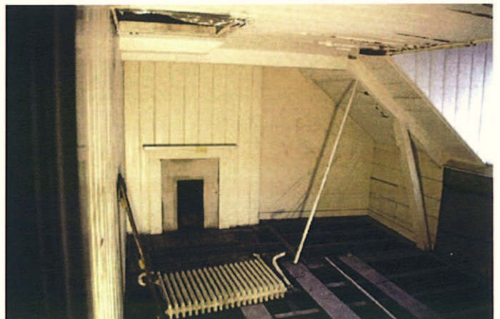
Plate 14: Typical internal partition wall construction, E414
