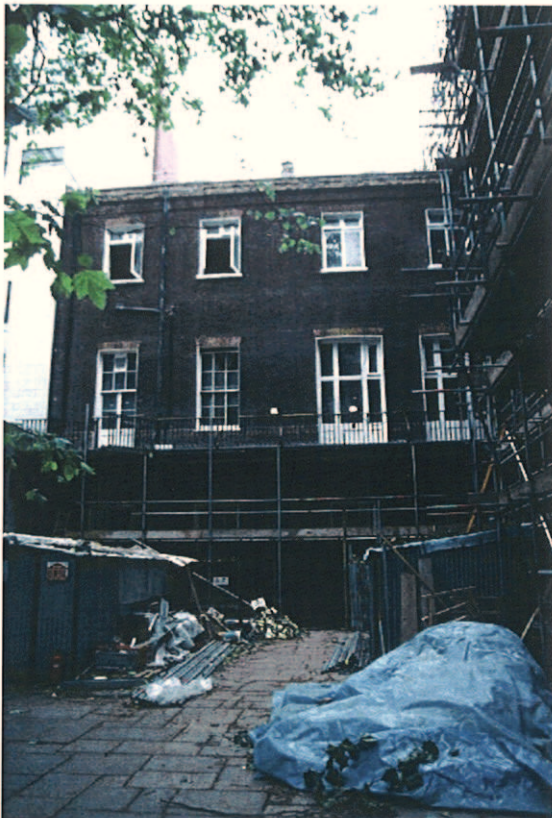
Plate 3: Courtyard, looking west
