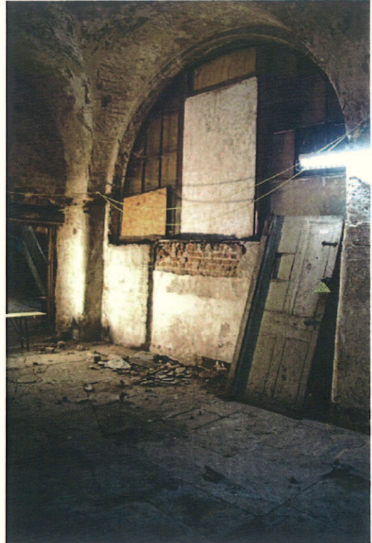
Plate 11: Lunnette window in west wall of E133 replacement window
