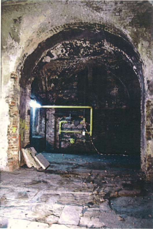
Plate 10: Basement of the Babmaes Building, E132&3, view north
