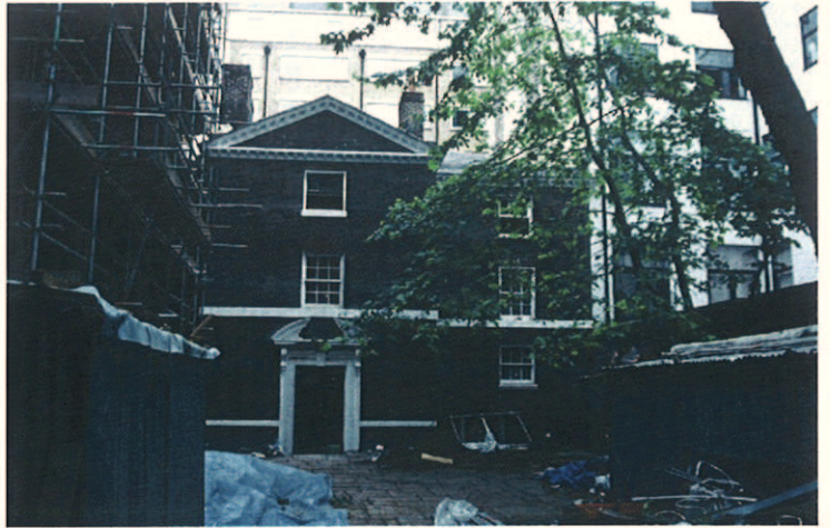
Plate 2: Front elevation of the Babmaes building
