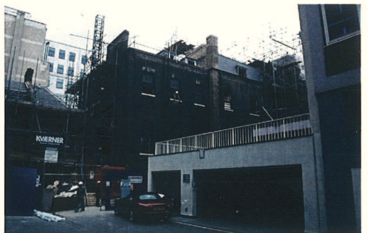
Plate 5: Earl de Grey 1830's rebuild and projecting 1790's Byfield Stair
