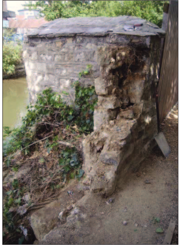
Plate 7: Core of wall during dismantling (north side)
