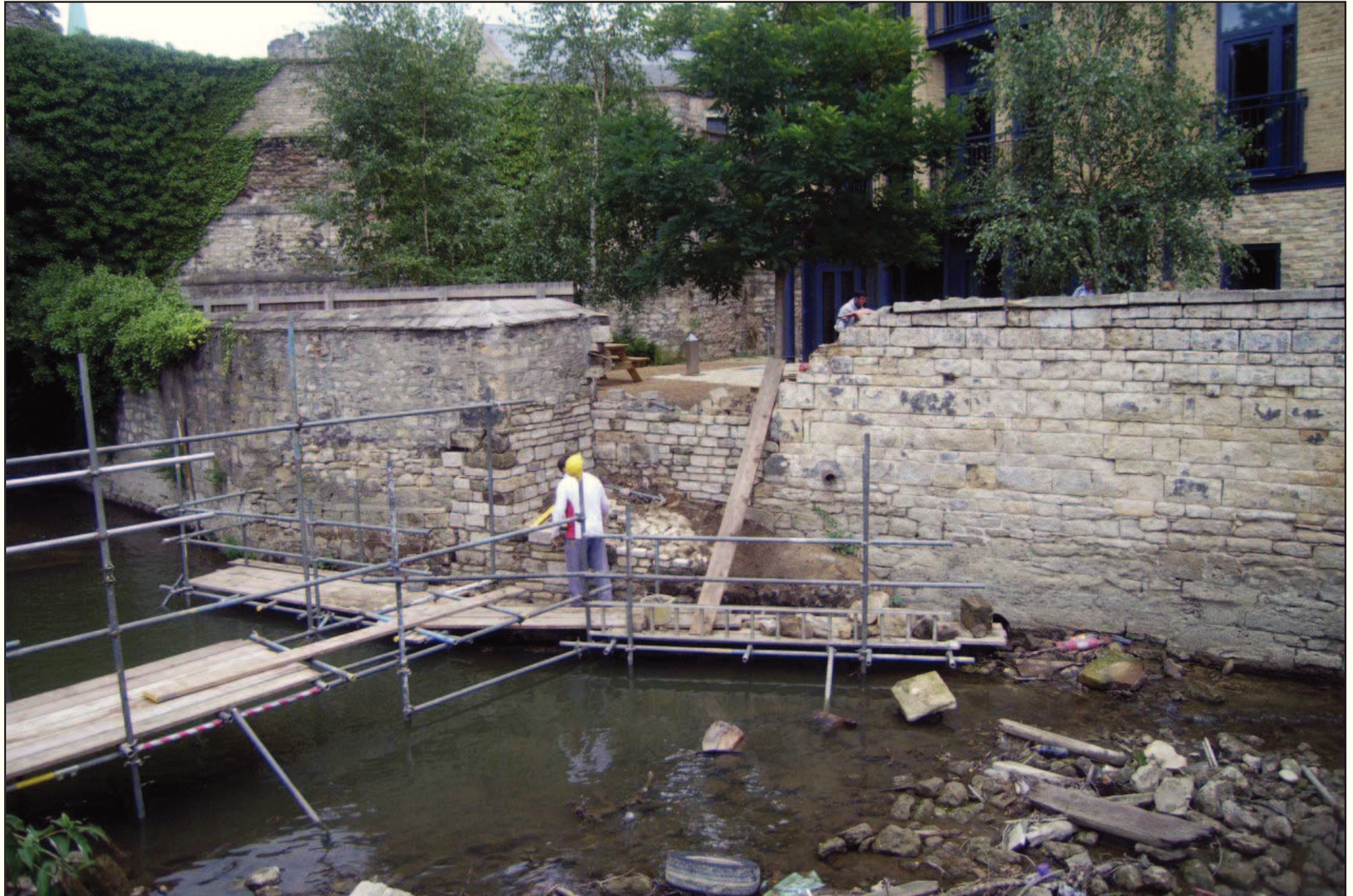
Plate 1: Repair work underway
