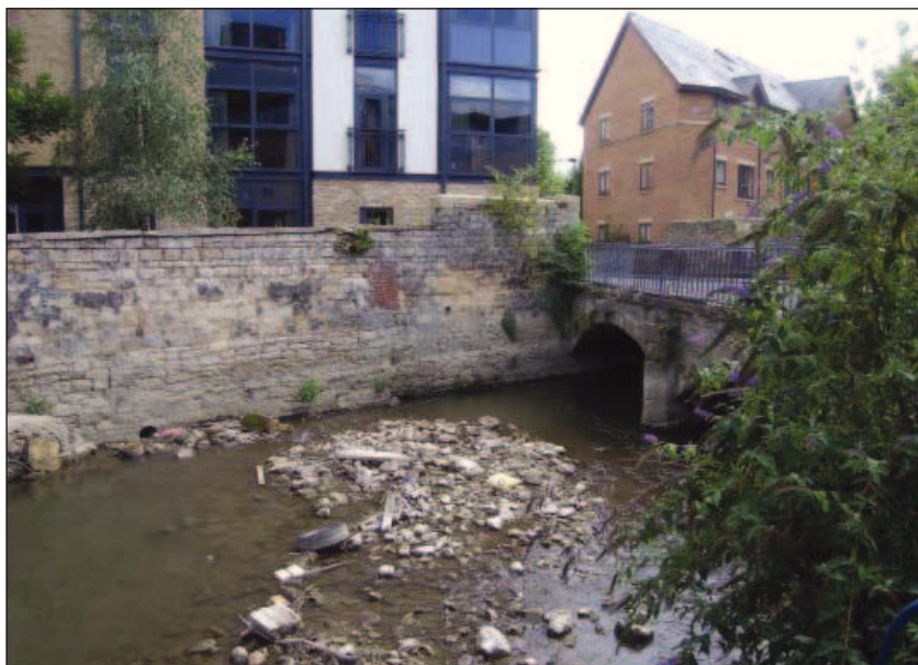
Plate 5: Revetment wall to south of current area
