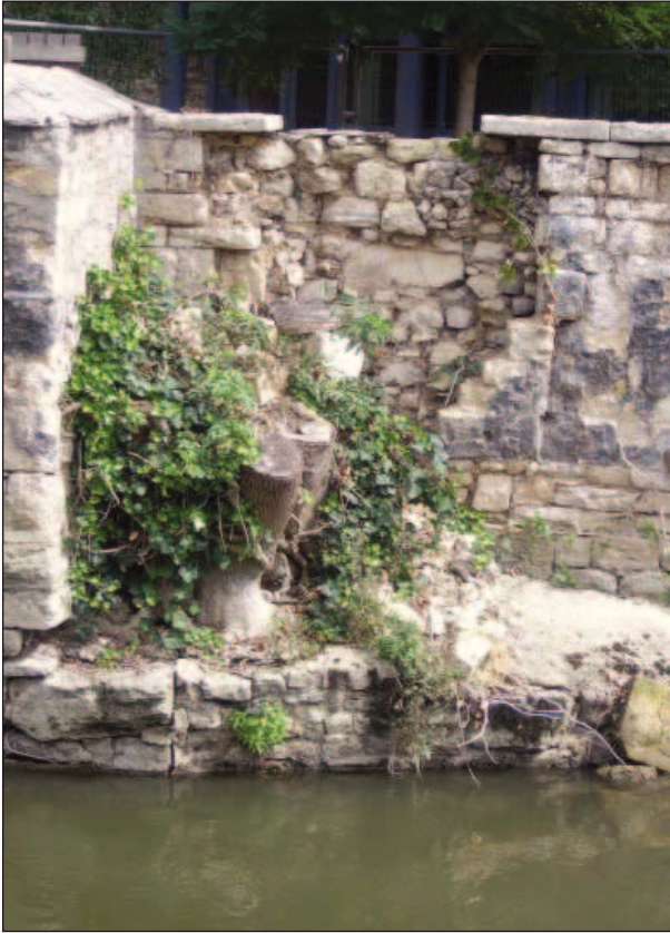
Plate 6: View of area collapse prior to conservation
