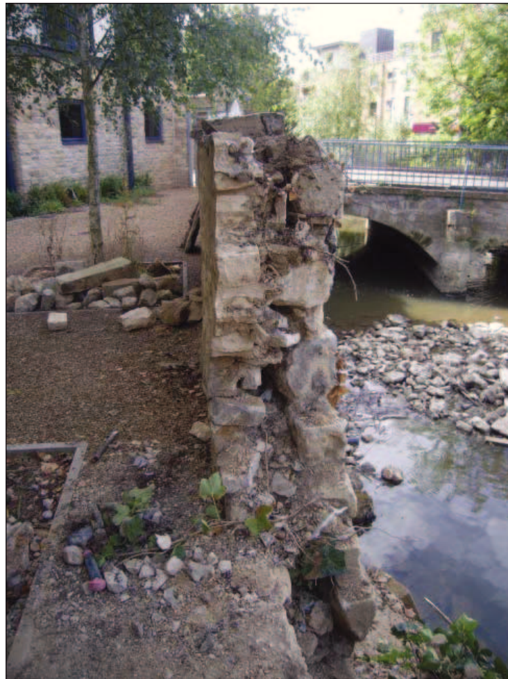
Plate 8: Core of wall during dismantling (south side)
