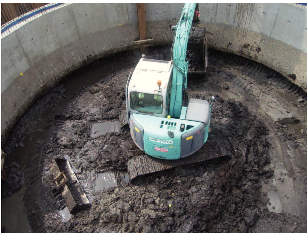
Plate 4: Excavation of the organic deposits.
