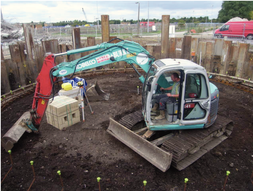
Plate 1: Excavation of the pump shaft
