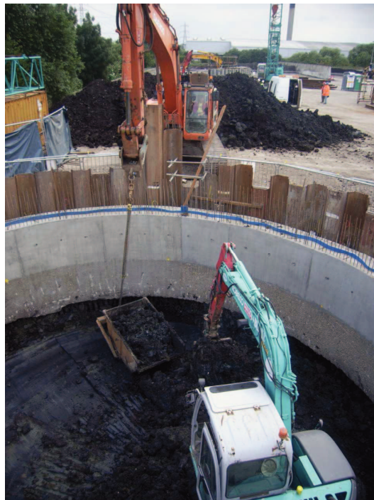
Plate 2: Removal of spoil from the excavation
