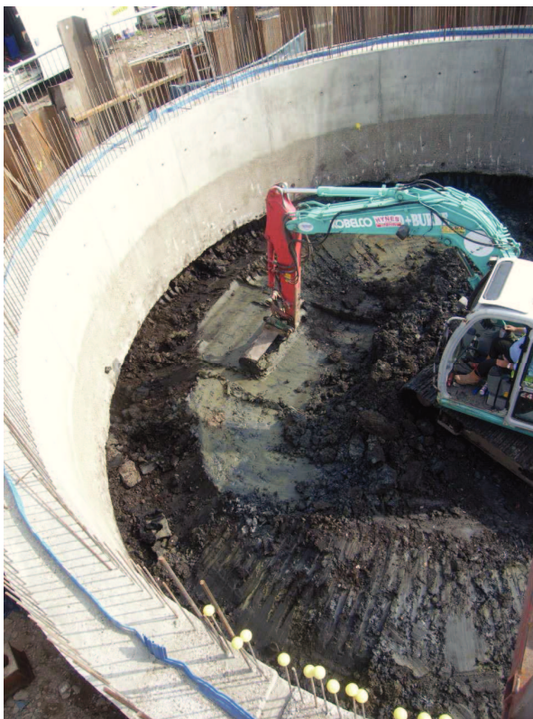
Plate 3: Excavation of the alluvium
