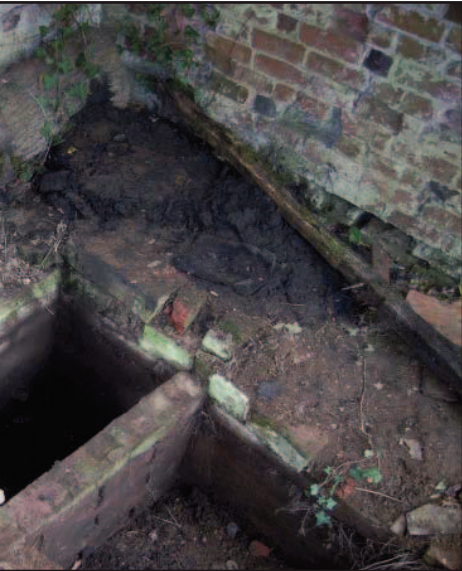
Plate 19: Small pits within bath house
