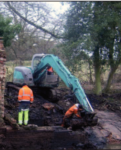
house from west during clearance works
