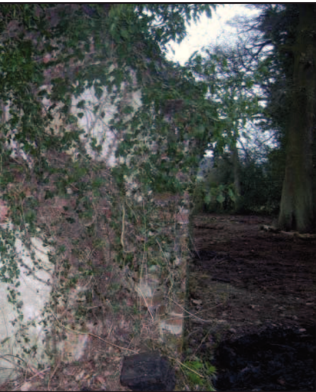
south end of surviving part of bath house
