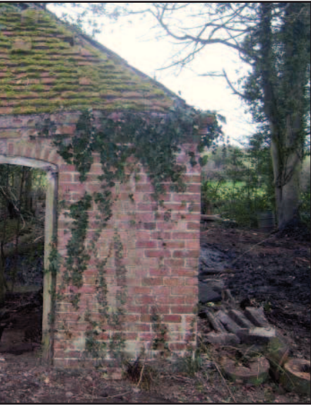
vation of surviving part of bath house
