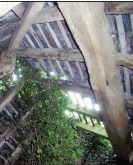
Roof within surviving part of bath house
