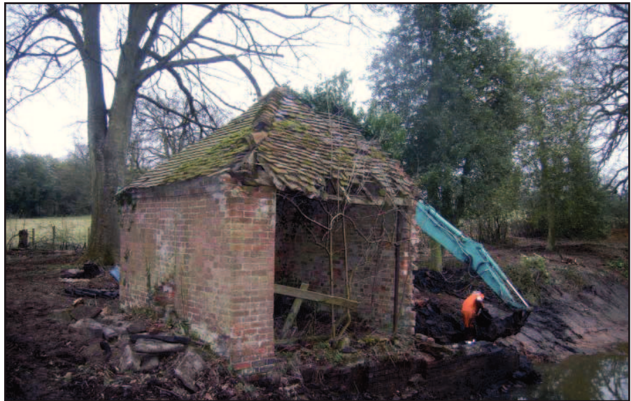
Plate 4: Bath House from north-west during clearance
