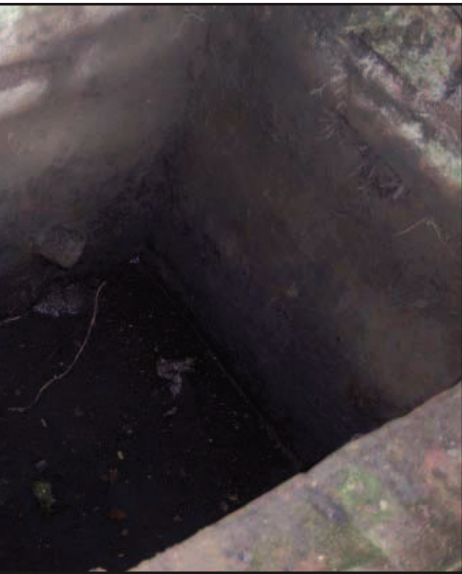
pit in bath house with pipe towards base
