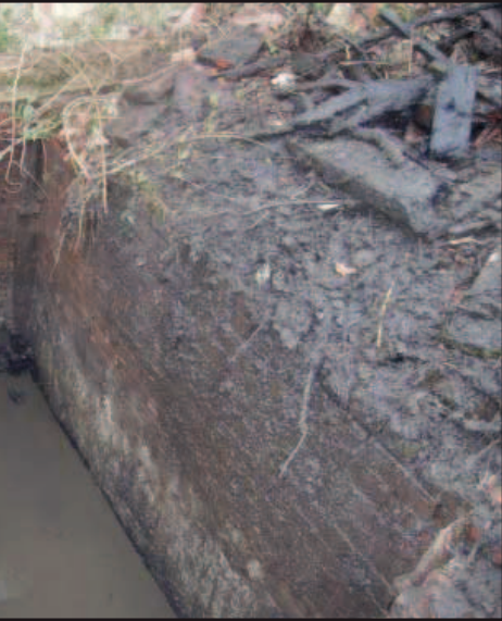
Former bath house after removal of infill
