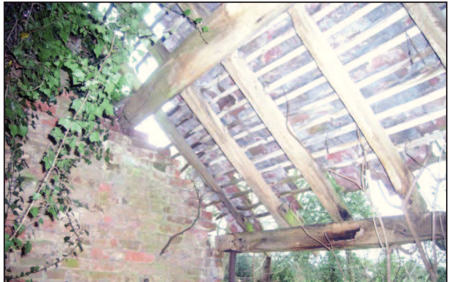
Plate 12: Roof within bath house looking south-west
