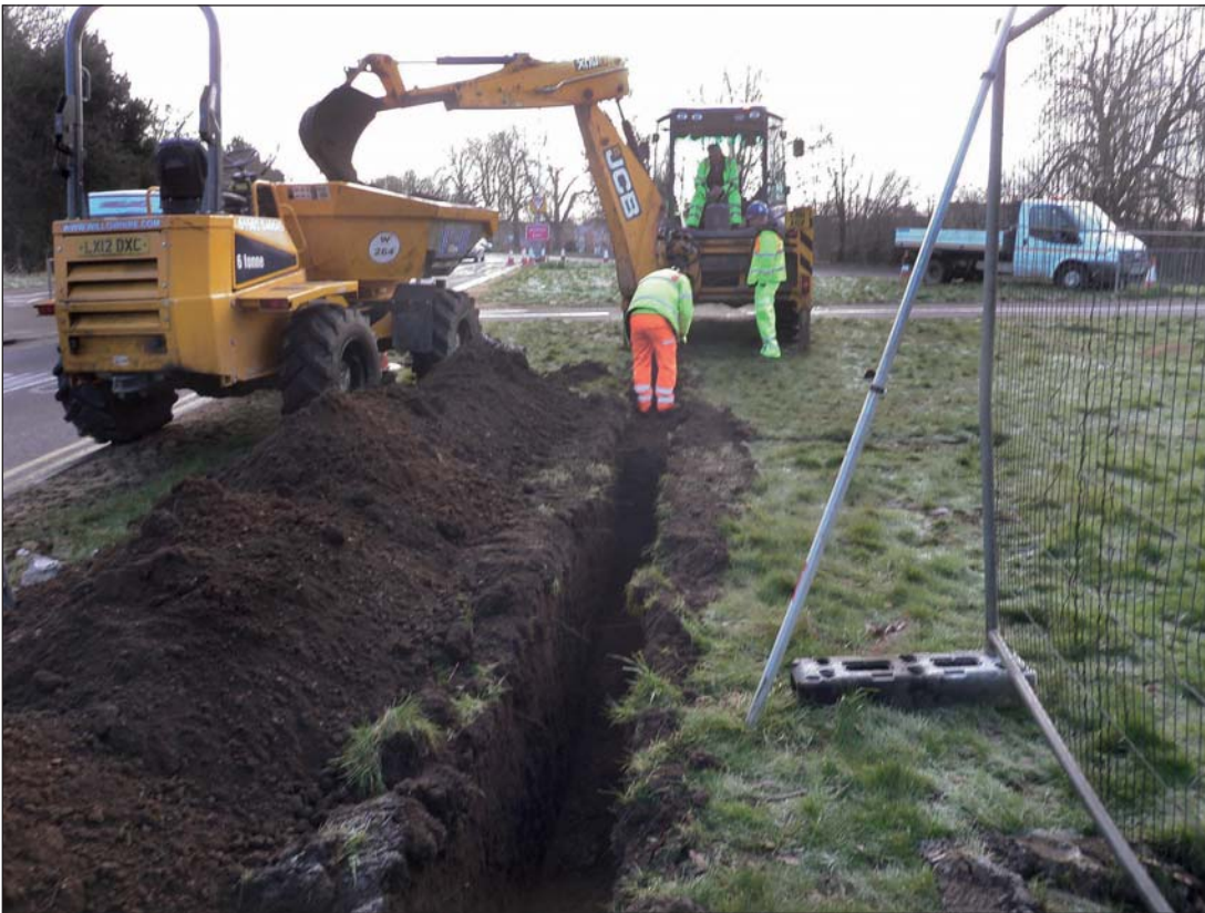
Plate 1: Drain trench at Brampton Road Interchange, taken from the west
