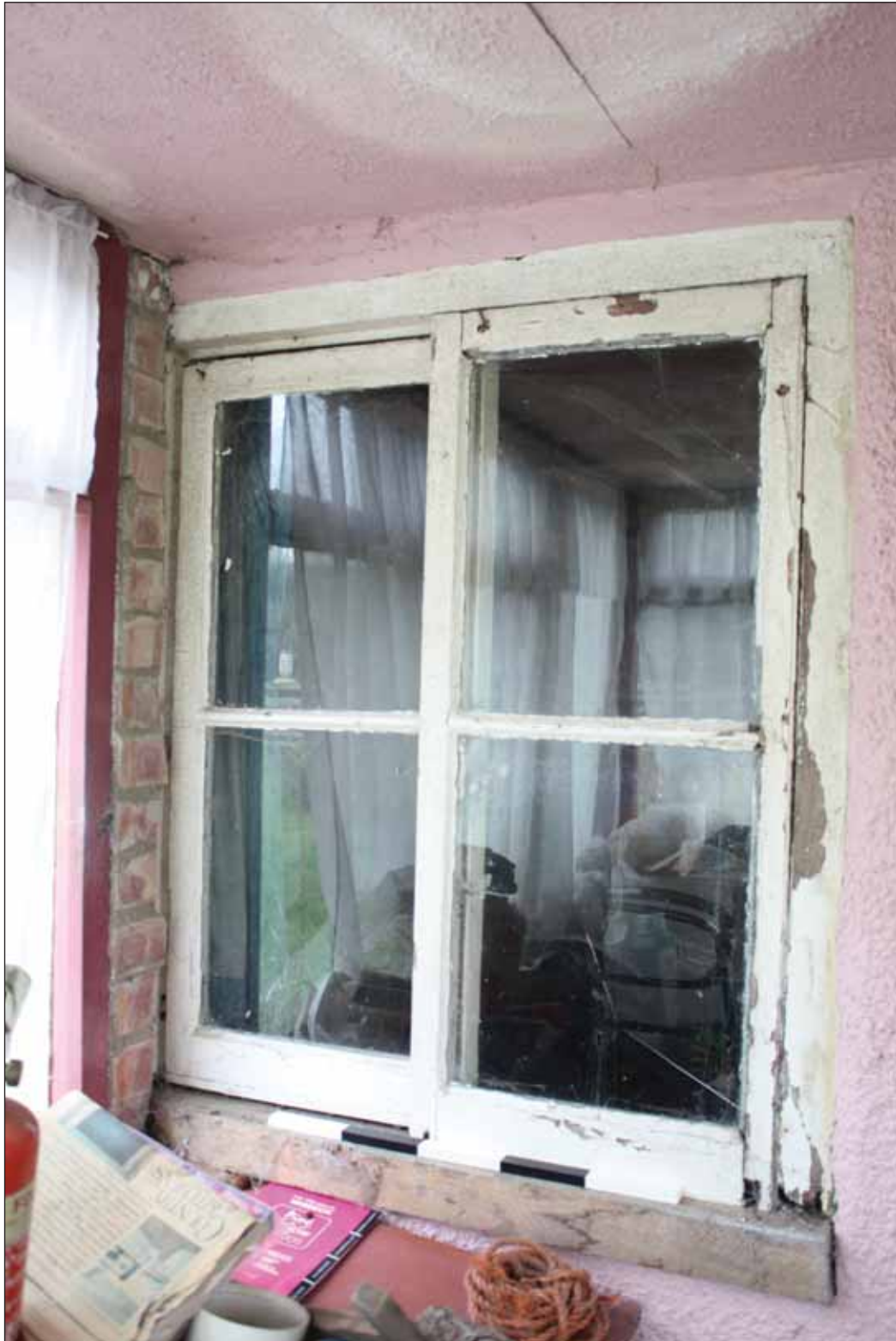
Plate 14. Detail of window (from G3)
