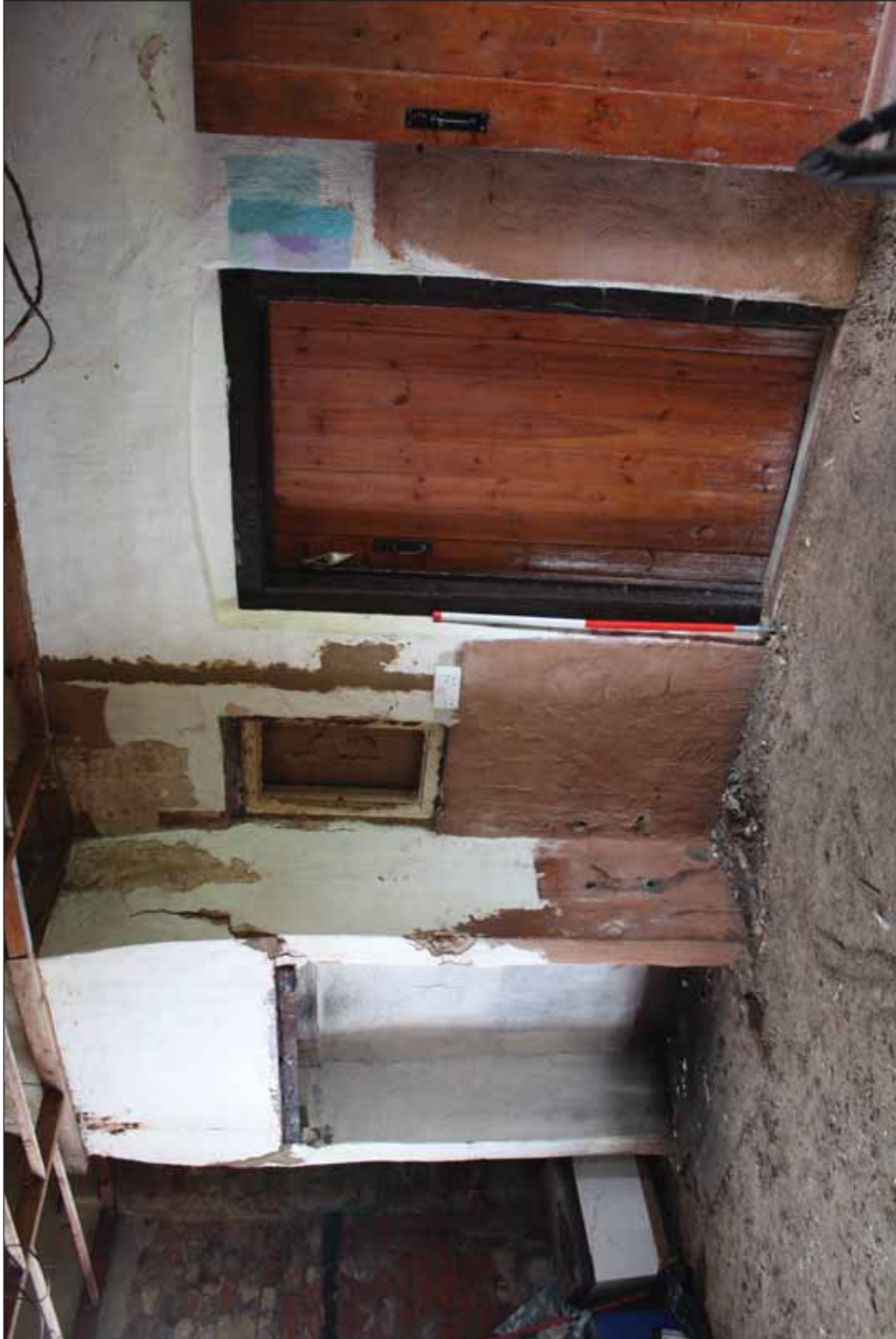
Plate 13. Interior wall, G2
