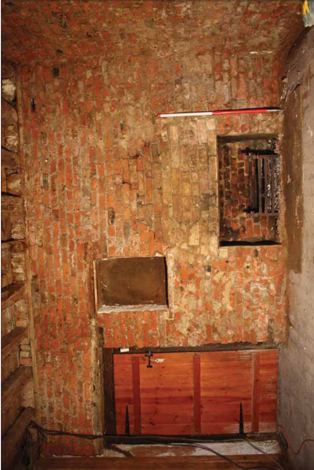
Plate 10. Interior wall, G1
