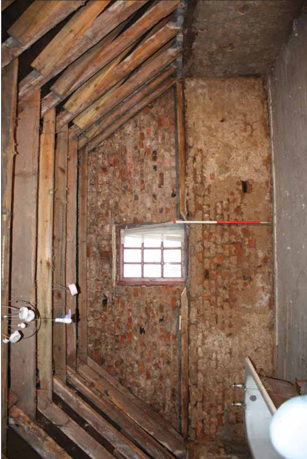
Plate 17. Internal shot of southern gable end (F1)
