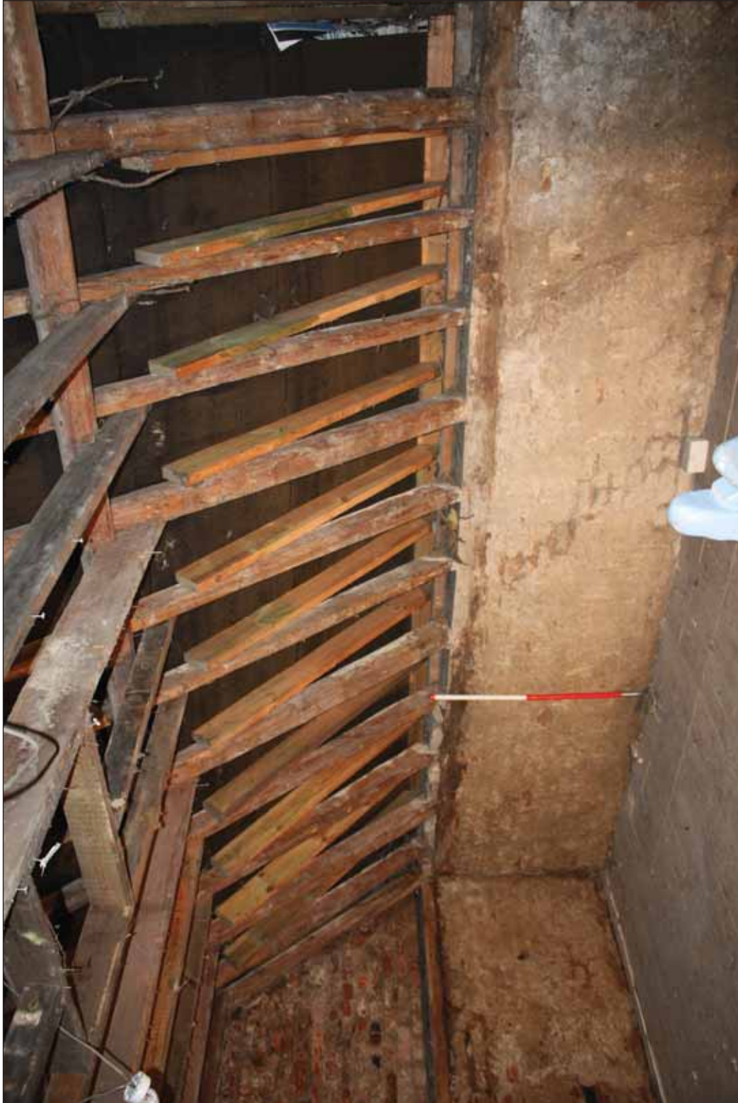
Plate 18. Room shot showing rafters, wall plates and collars, F1
