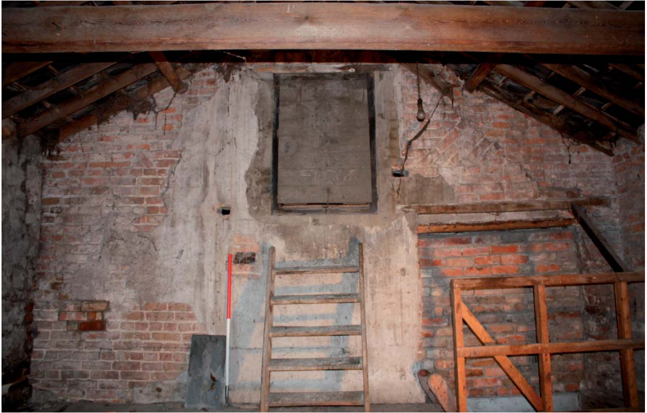
Plate 33: Interior detail, Building 6, first floor
