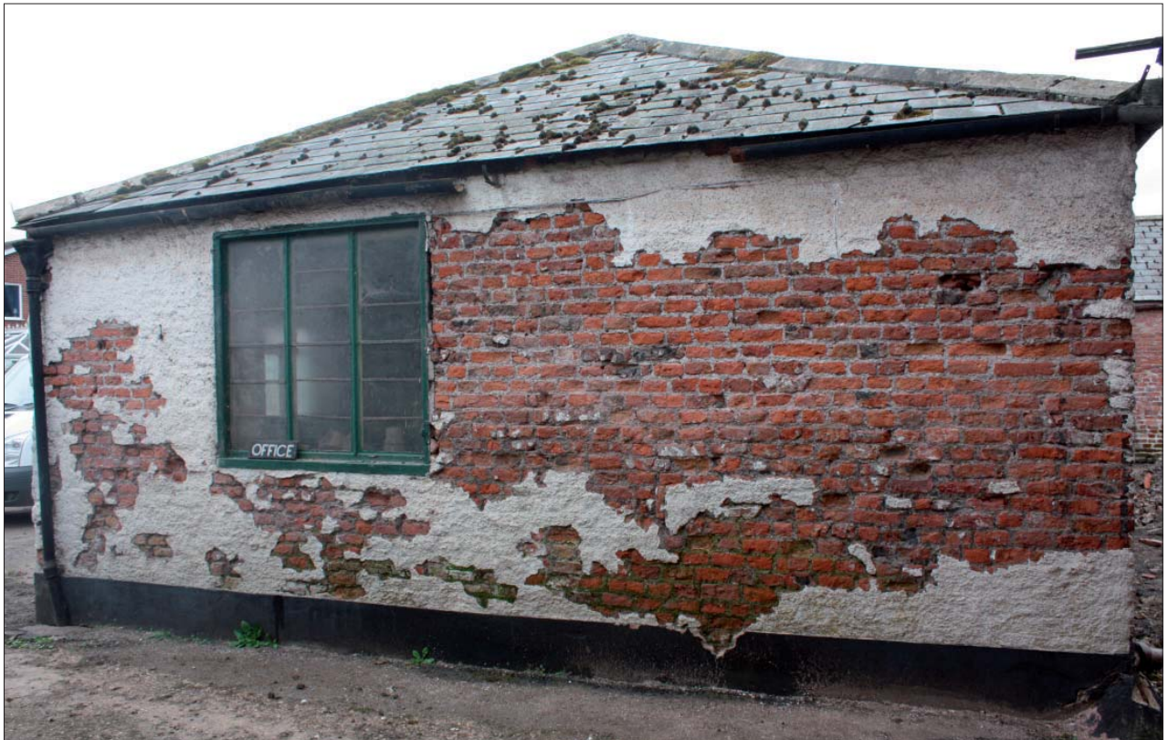
Plate 10: Building 3 from north
