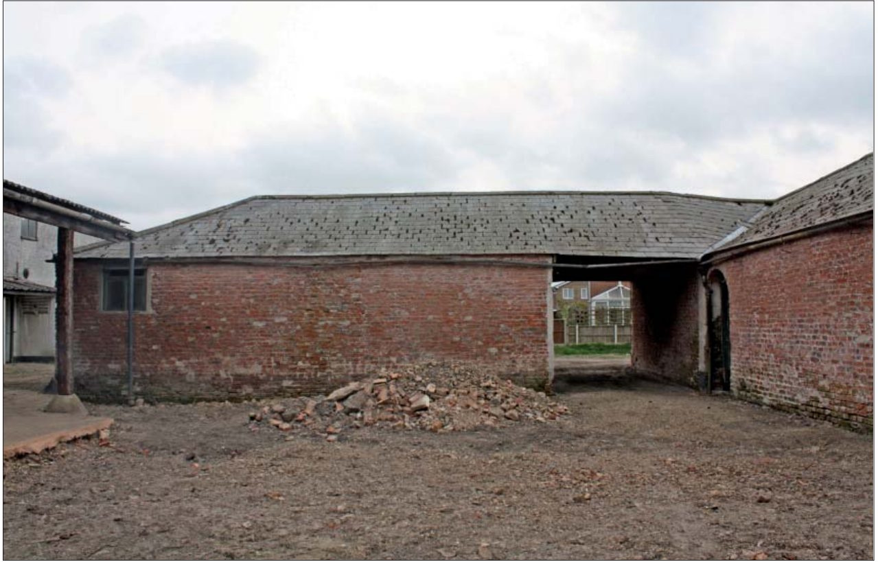
Plate 9: Building 3 from northwest
