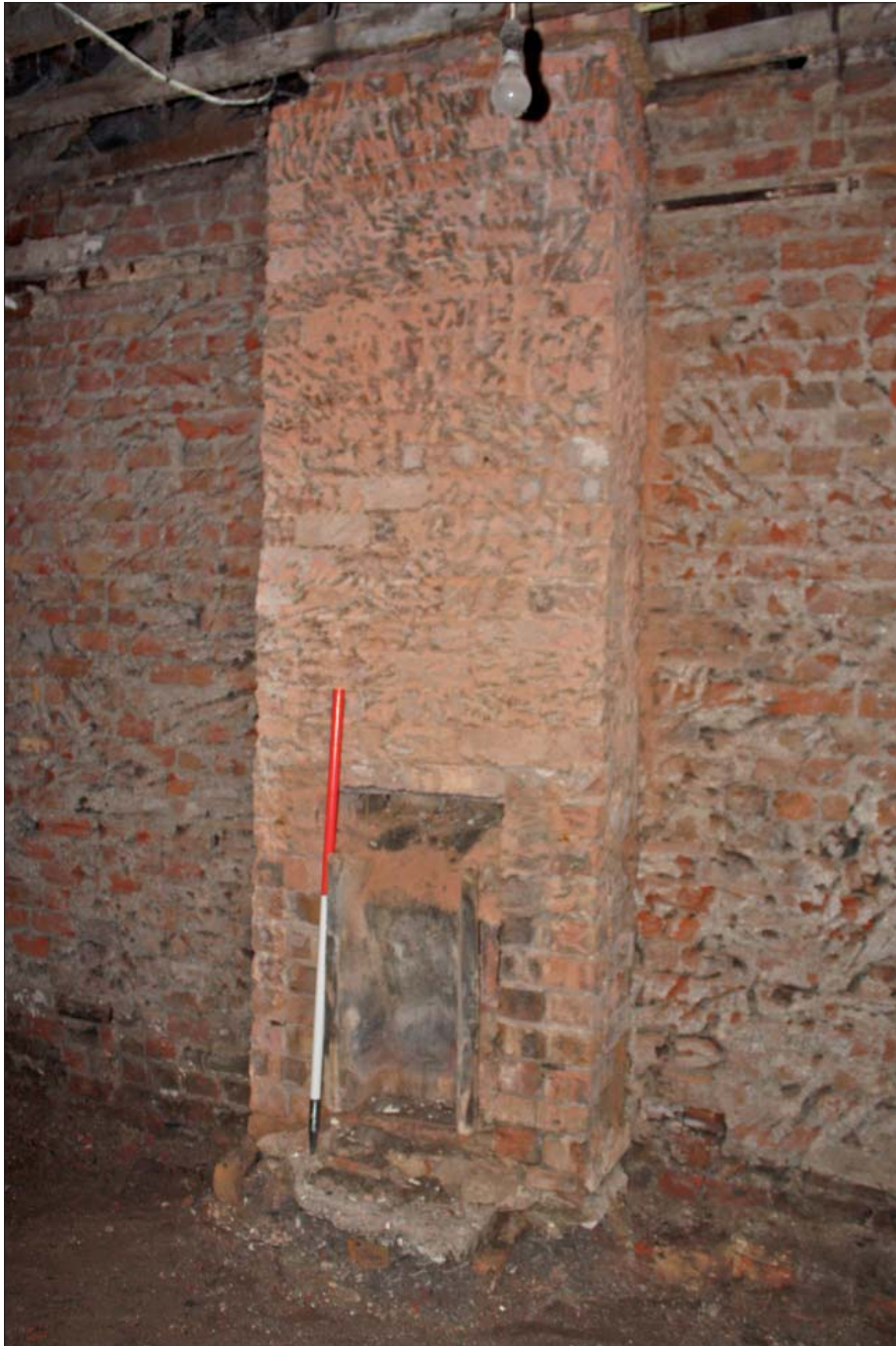
Plate 19: Building 4 showing interior detail of fireplace/chimney-breast
