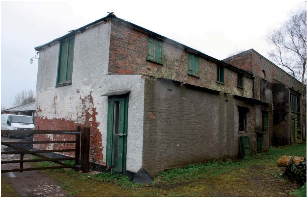
Plate 30: Building 6 from east
