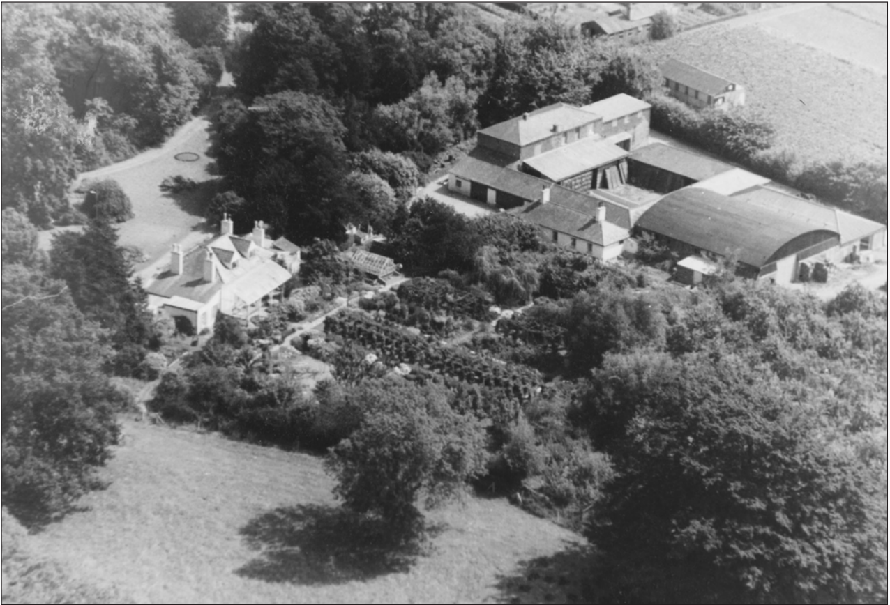
Figure 7: Aerial photograph (undated).
