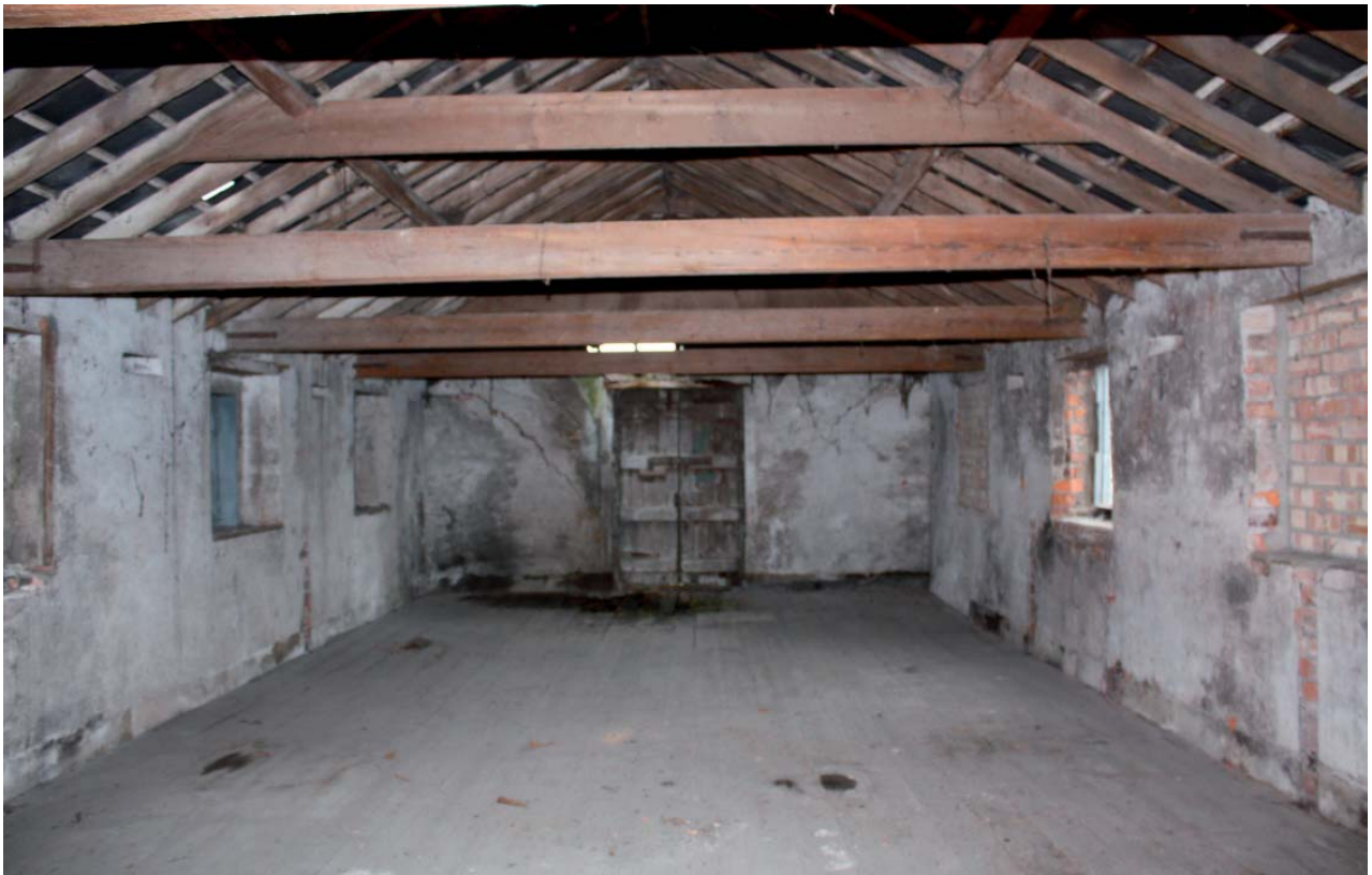
Plate 34: Interior detail, Building 6, first floor
