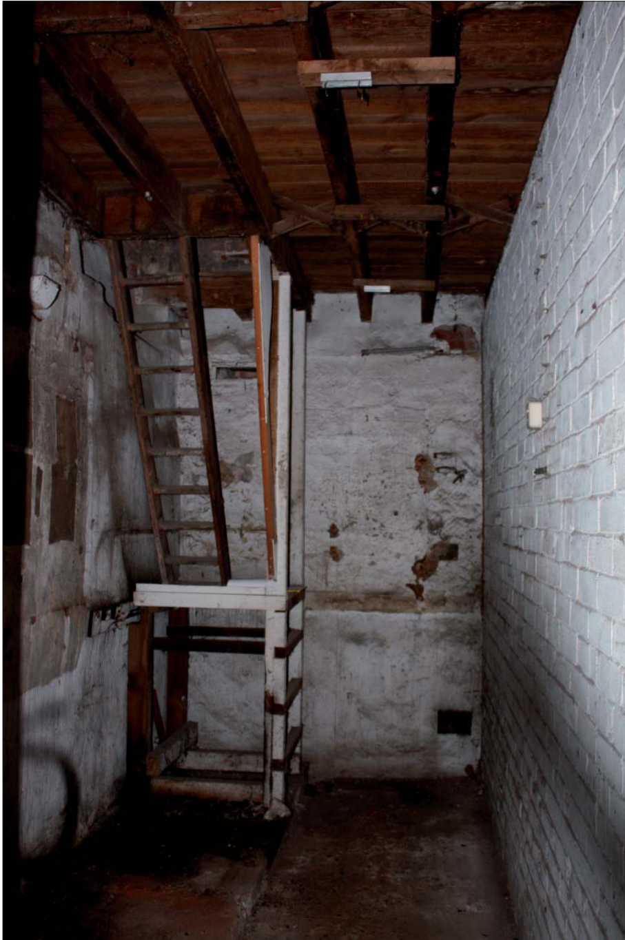
Plate 32: Interior detail, Building 6, ground floor
