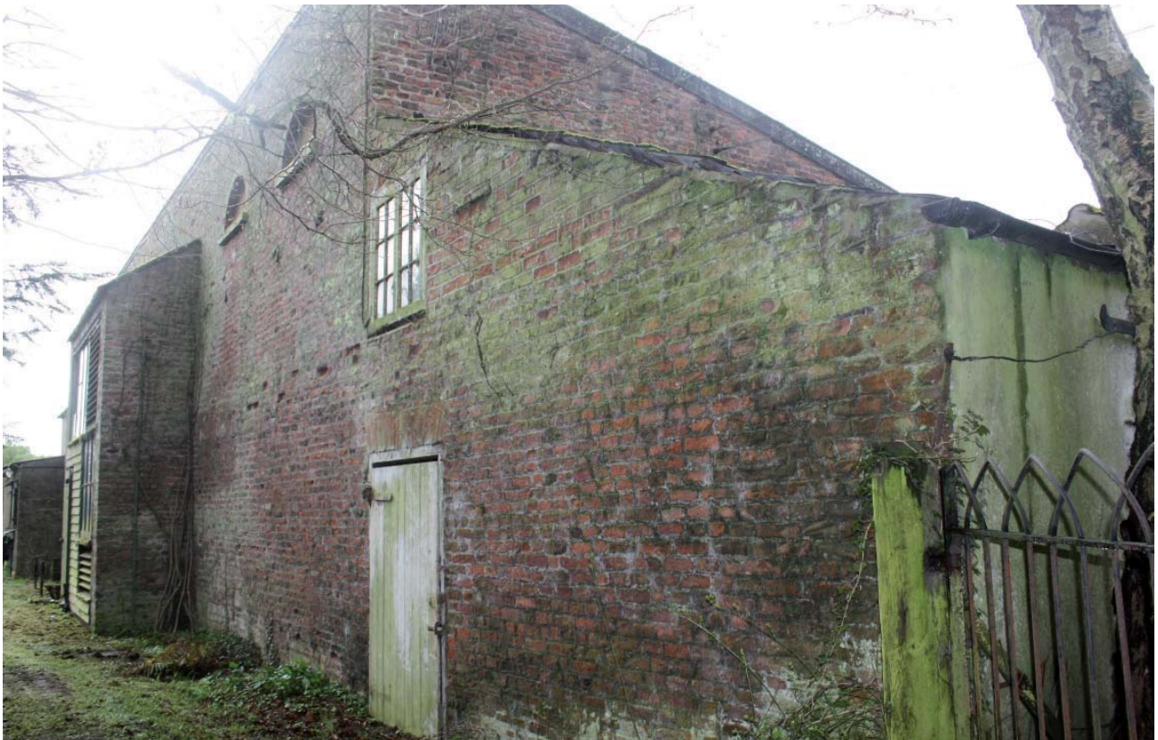
Plate 23: Building 5 from north
