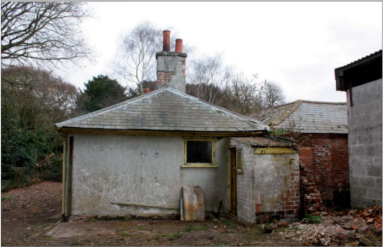
Plate 15: Building 4 from southwest
