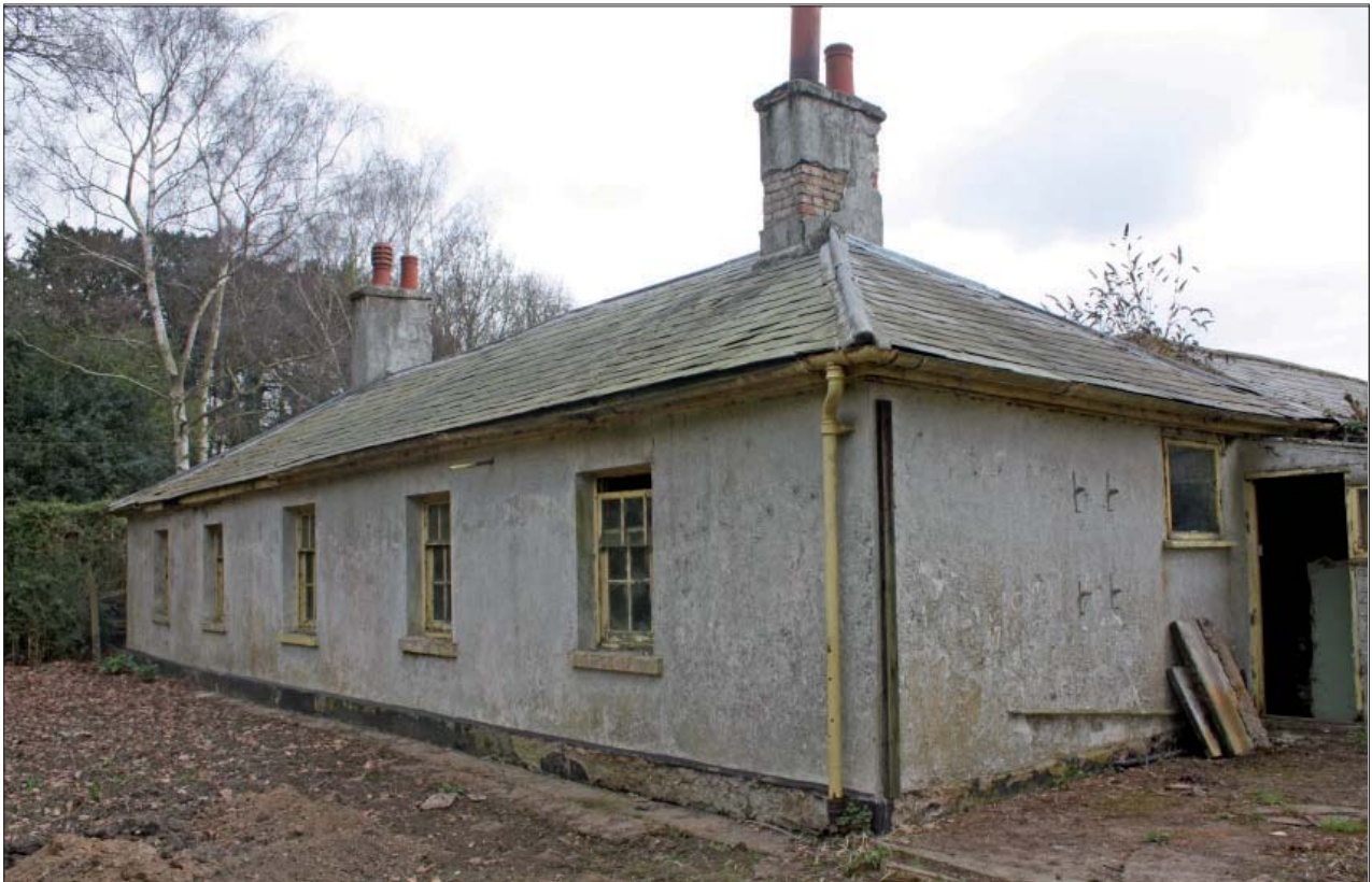
Plate 14: Building 4 from west
