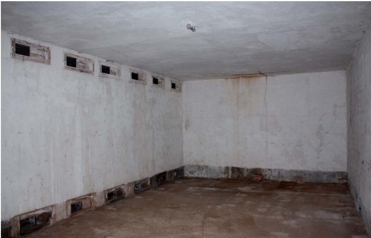
Plate 31: Interior detail, Building 6, ground floor
