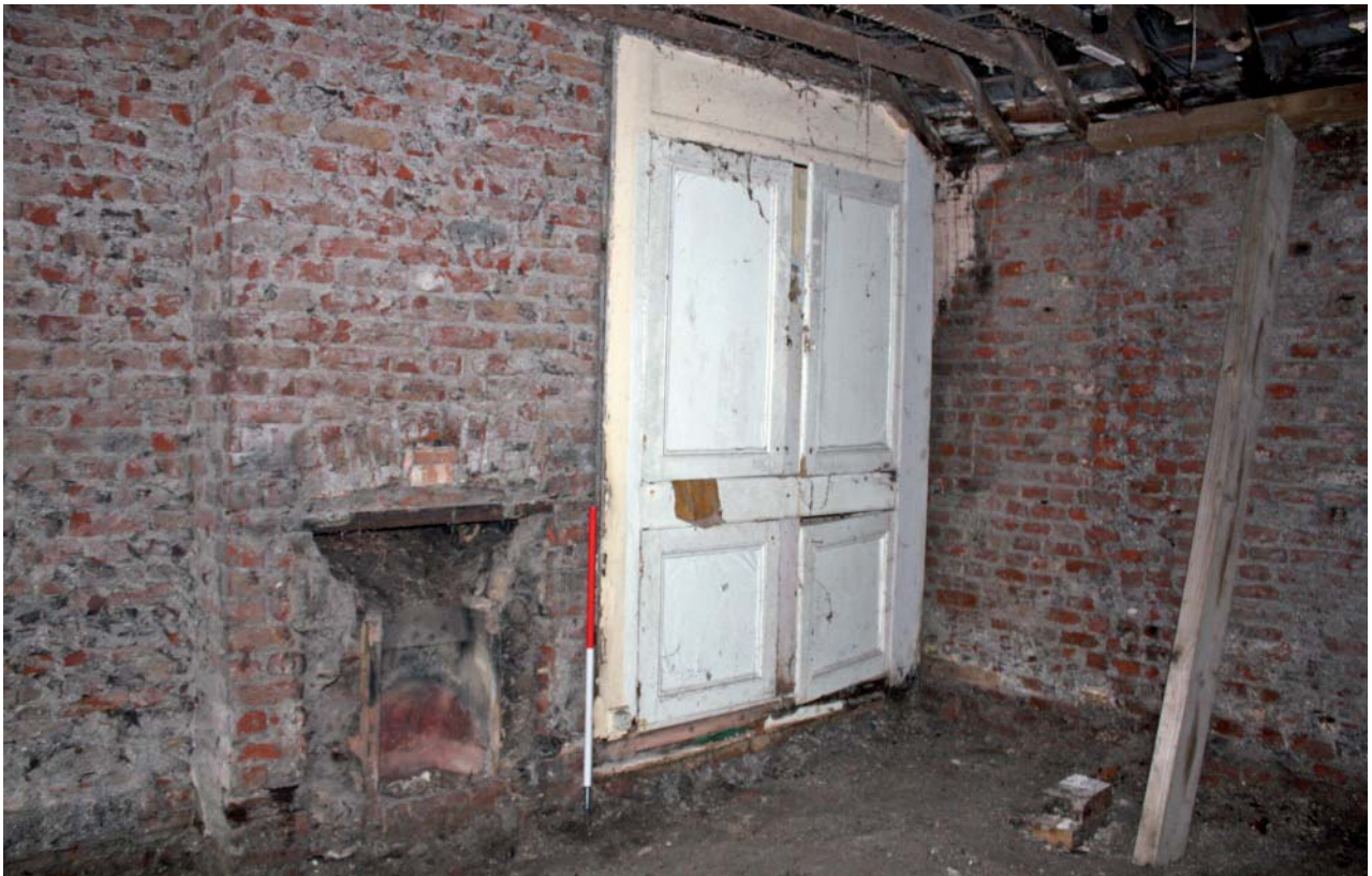
Plate 18: Building 4 showing interior detail of fireplace/chimney-breast and re-used paneling
