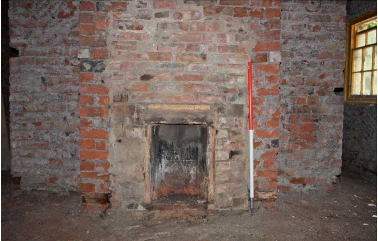
Plate 17: Building 4 showing interior detail of fireplace/chimney-breast
