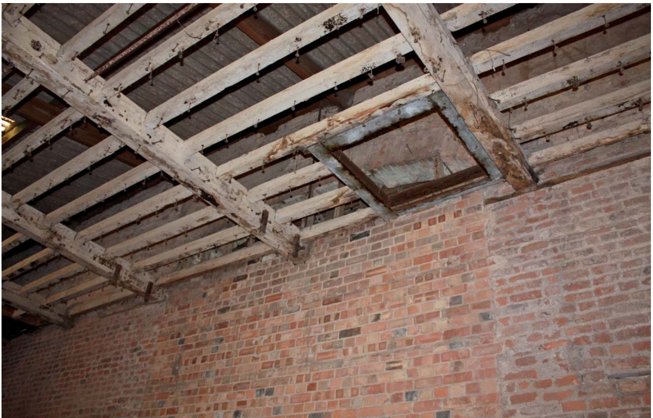
Plate 26: Detail of blocked former entrance, Building 5
