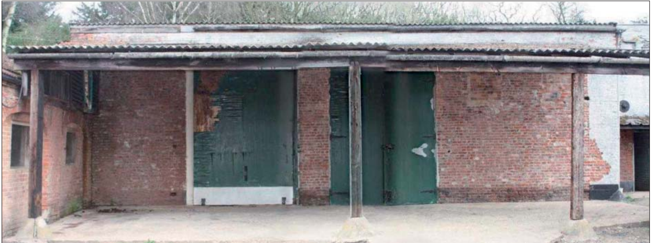
Plate 20: Building 5 from southwest (images "stitched" using Autostitch)
