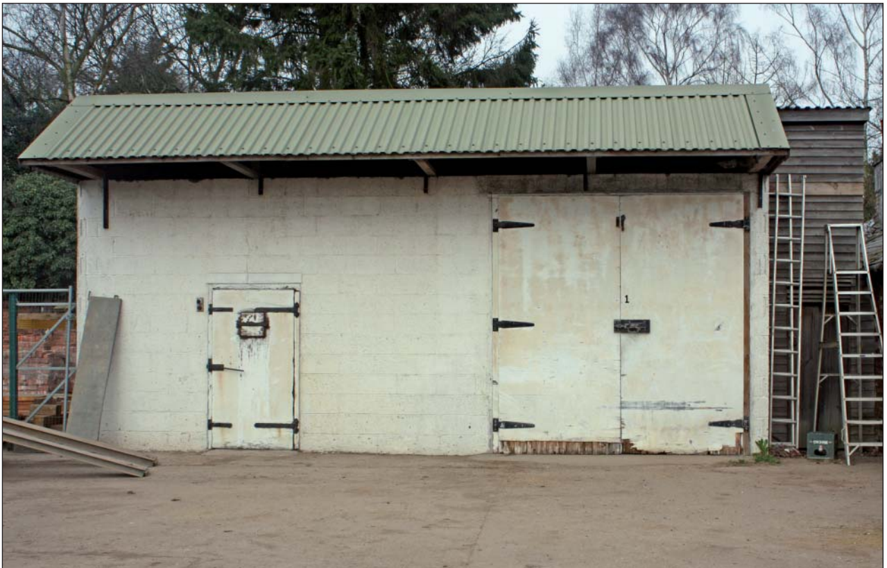
Plate 2: Building 1 from southeast
