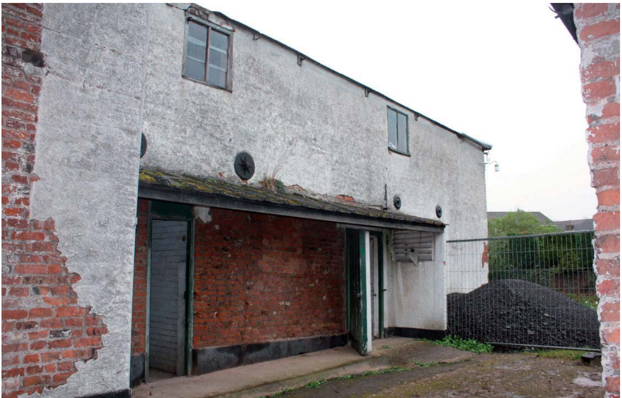
Plate 29: Building 6 from west
