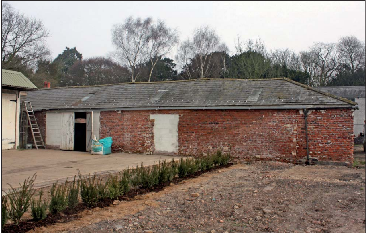
Plate 3: Building 2 from southwest
