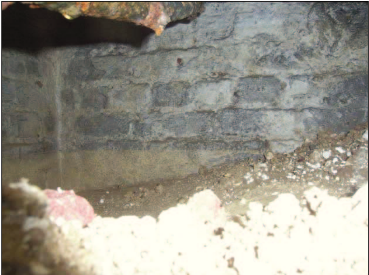
Plate 14: Trench 2. Walls within void
