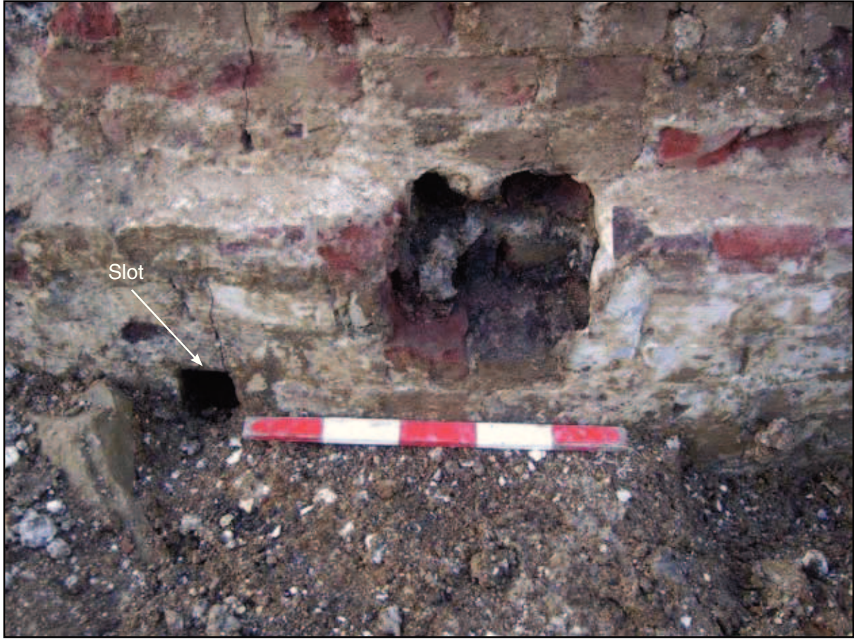
Plate 4: Trench 2. Elevation view of recess for horizontal support in wall 3001, and window slot visible, looking north-west
