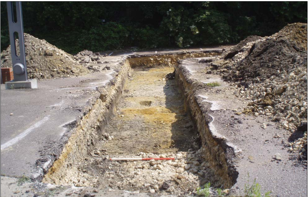
Plate 2: Trench 2, looking south-east
