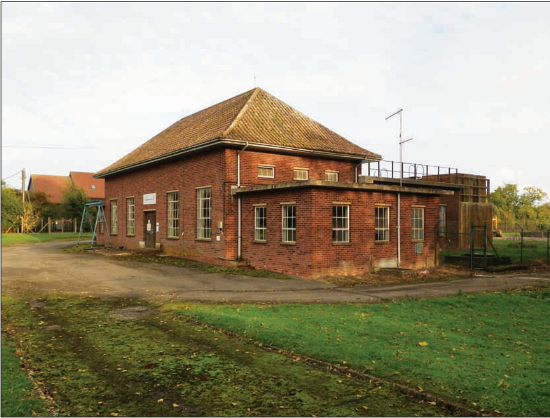
Plate 1: The water treatment works building HER16307 (facing east)
