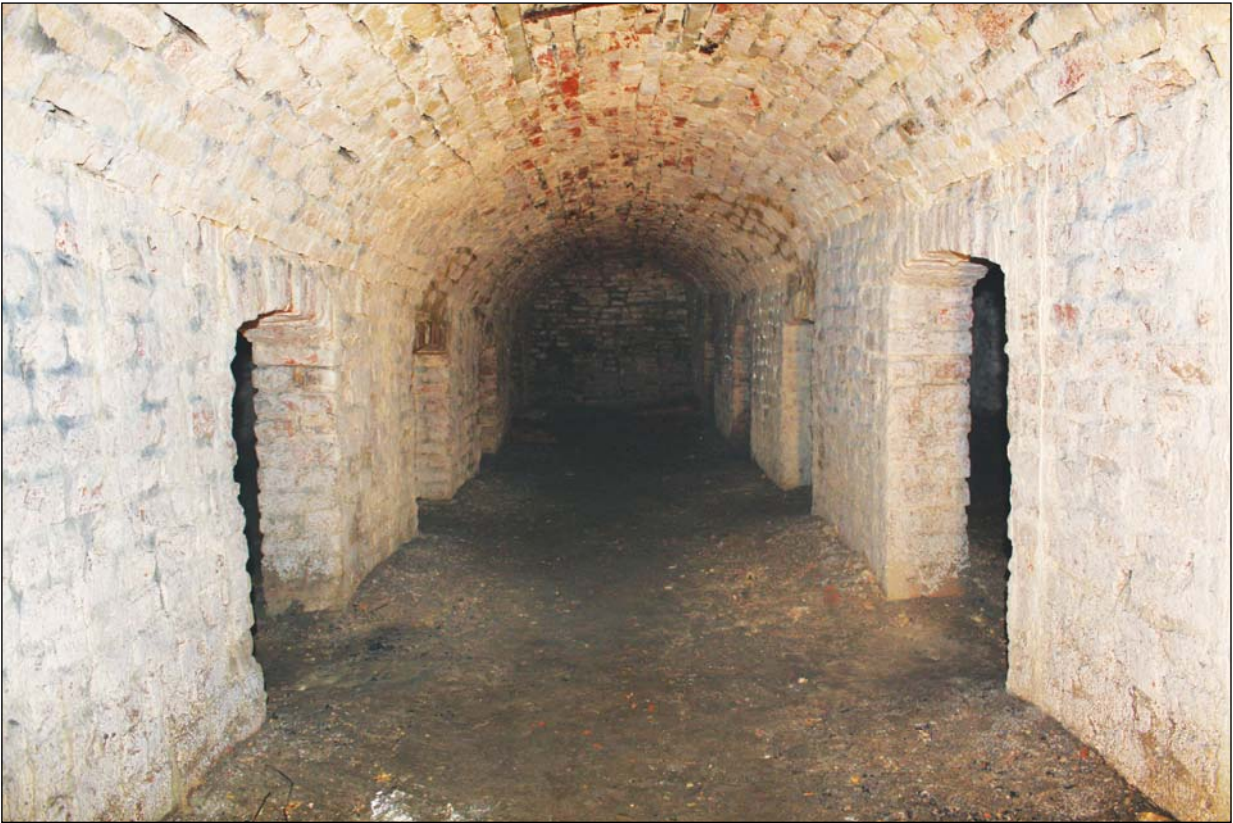
Plate 27: The vaults, R6
