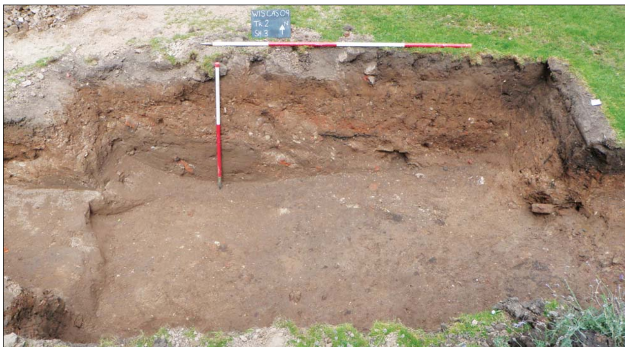
Plate 5: Pre-excavation shot of south-facing section, Trench 2, lower garden
