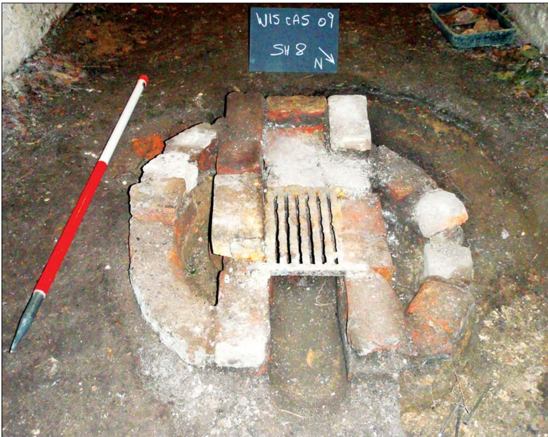
Plate 22: Base of brick "oven" recorded in the vaults
