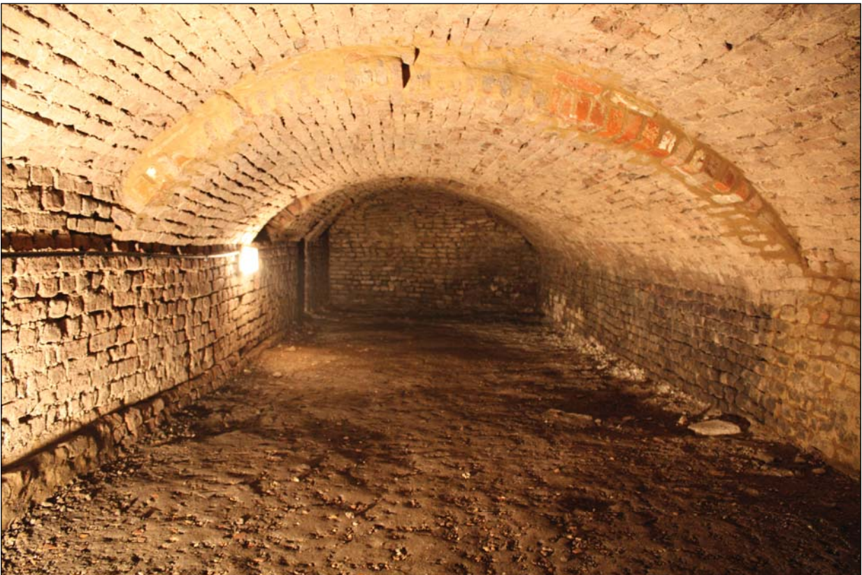
Plate 28: End tunnel L9, the vaults
