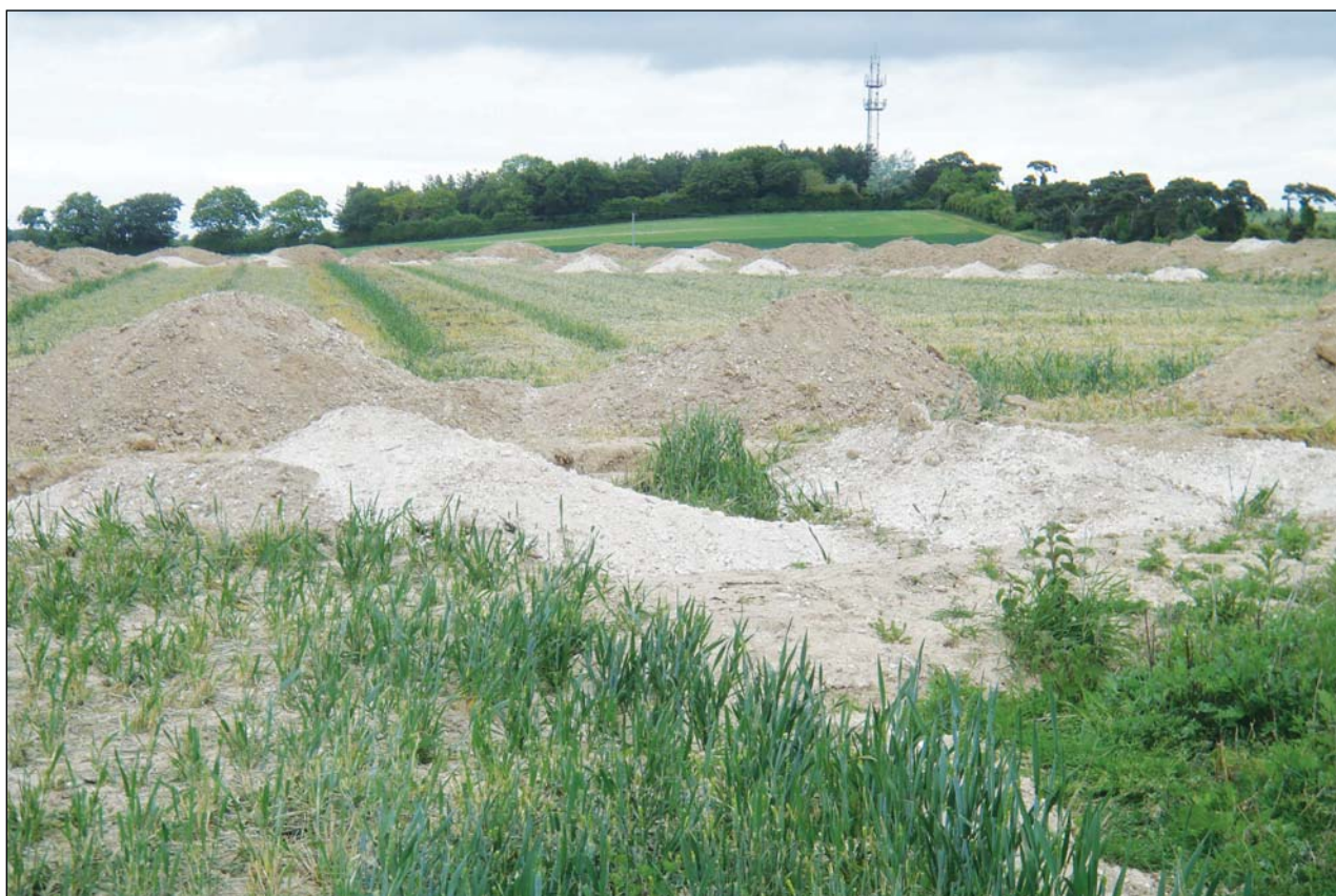
Plate 5: Working shot of site looking north towards radio mast on summit of Chalk Hill
