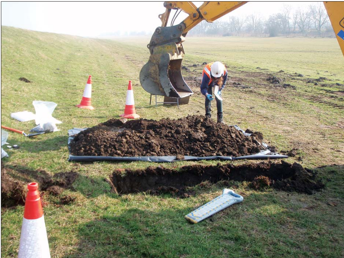
Plate 4: Test pit under excavation
