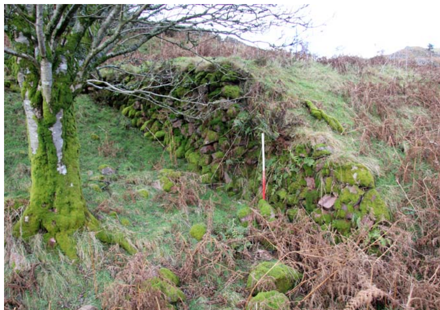
Plate 17: The retaining wall supporting the upper section of the inclined plane (Site BG36 )
