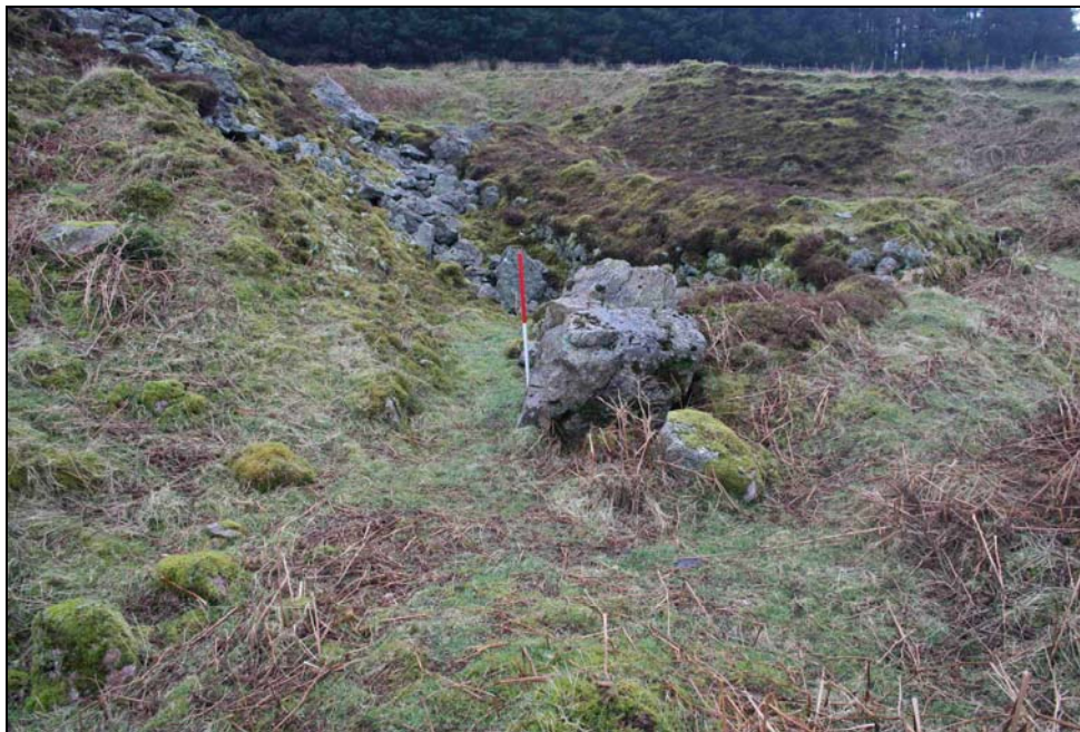
Plate 15: The truncated entrance to an adit (Site BG10e ) overlain by a later revetted spoil bank (Site 10d )
