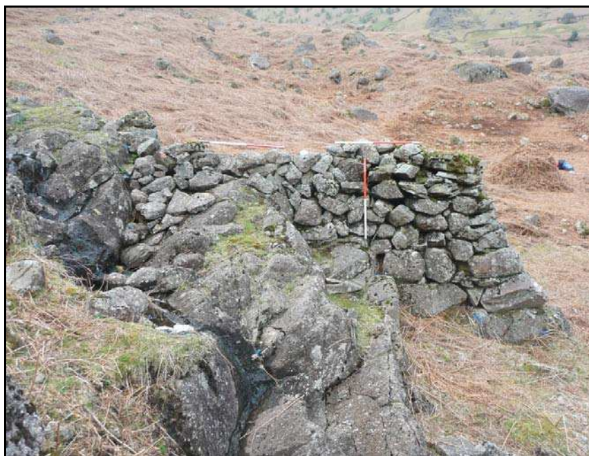
Plate 25: South wall elevation of the eastern end of the extant launder platform (Site SMG08.1 )
