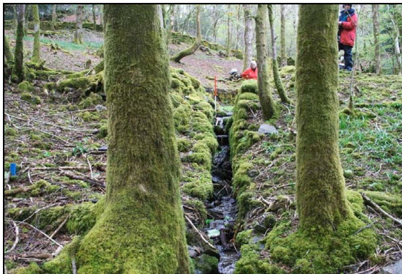
Plate 40: Outflow from the wheel pit into the linear tail race (Sites LW02 and LW04.1 )
