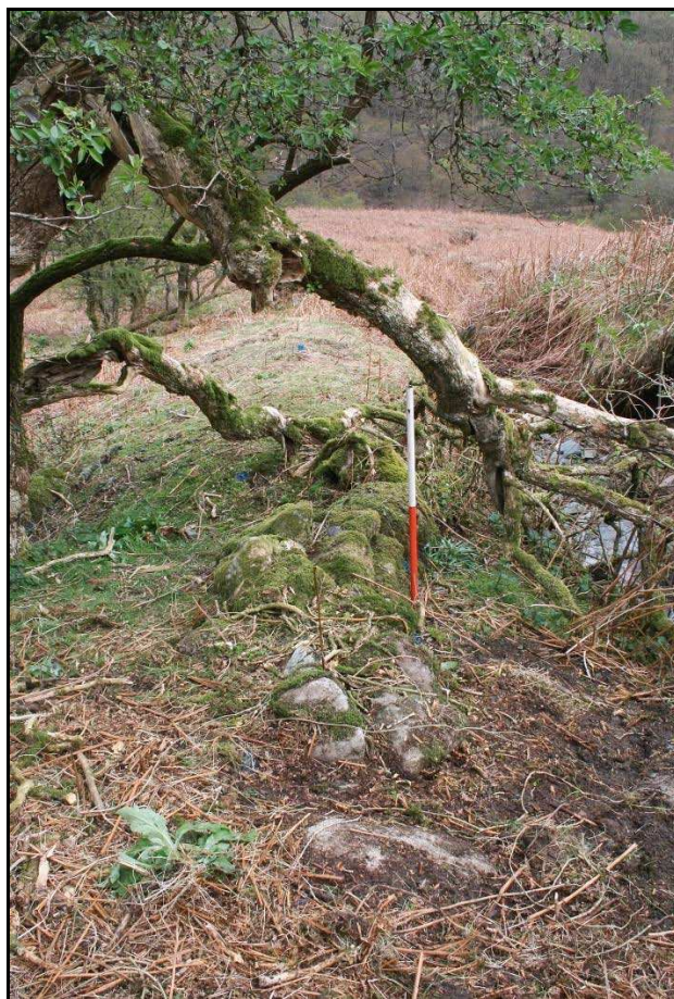
Plate 32: Linear blocking dam wall located at the take-off point at the beginning of the head race (Site LT09 )
