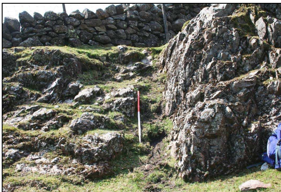
Plate 45: A narrow rock-cut channel carrying the head race/secondary divert channel down the rocky outcrop (Site SG01.2 )
