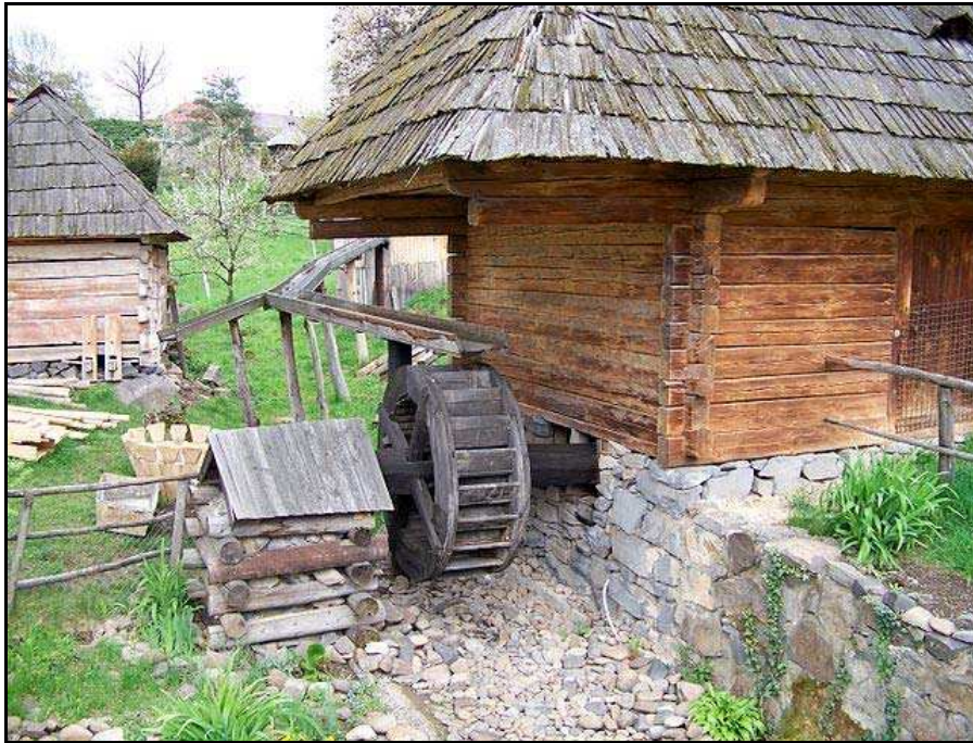
Plate 4: Launder and waterwheel on a small village mill at the Museum of Folk Architecture and Life, Uzhhorod, Ukraine
