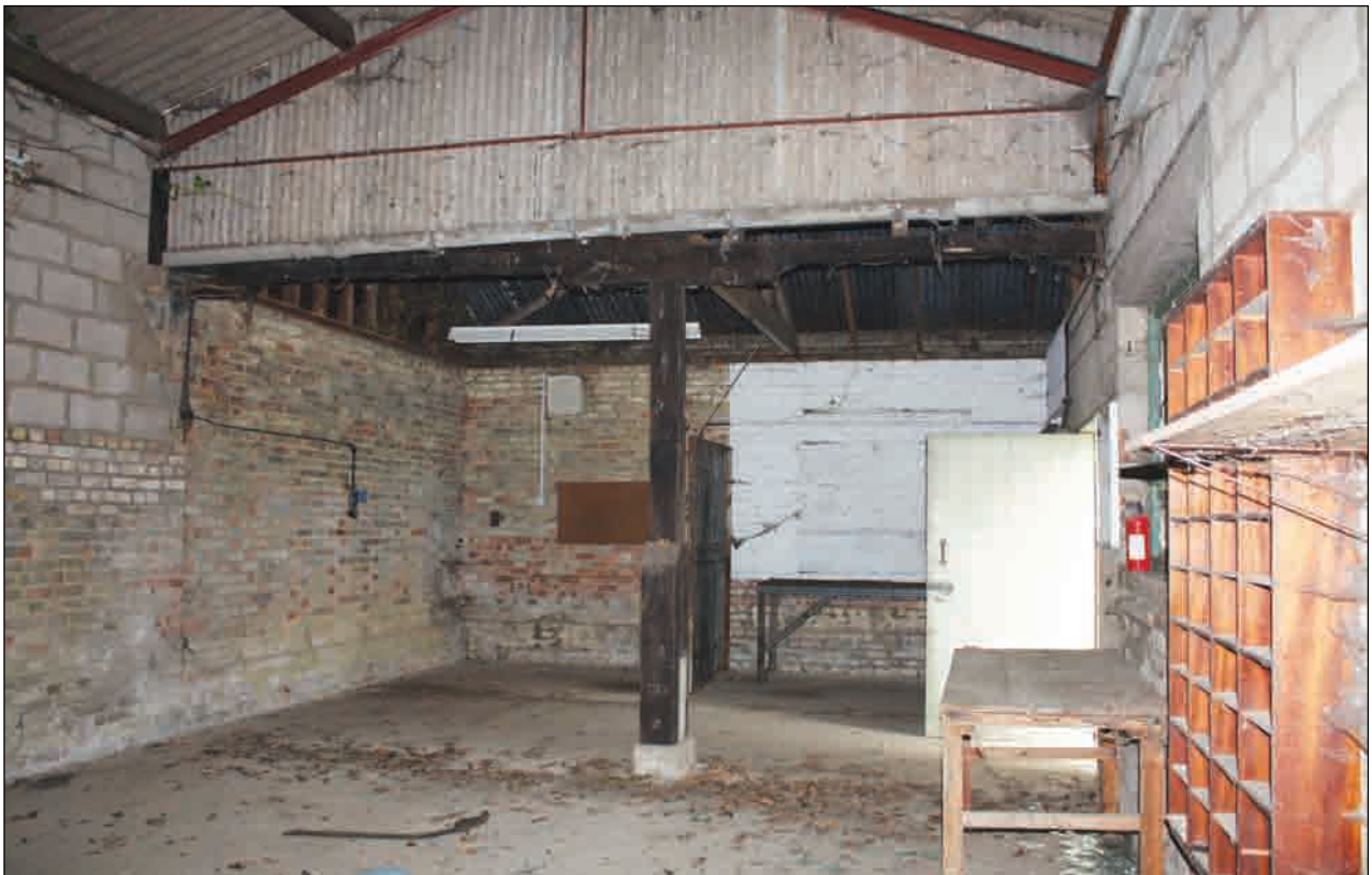
Plate 66: Interior view, Building 4
