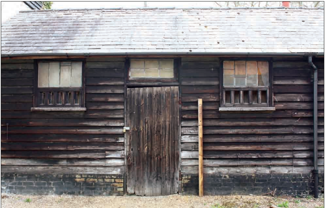
Plate 17: Entrance on west-facing elevation, Building 2
