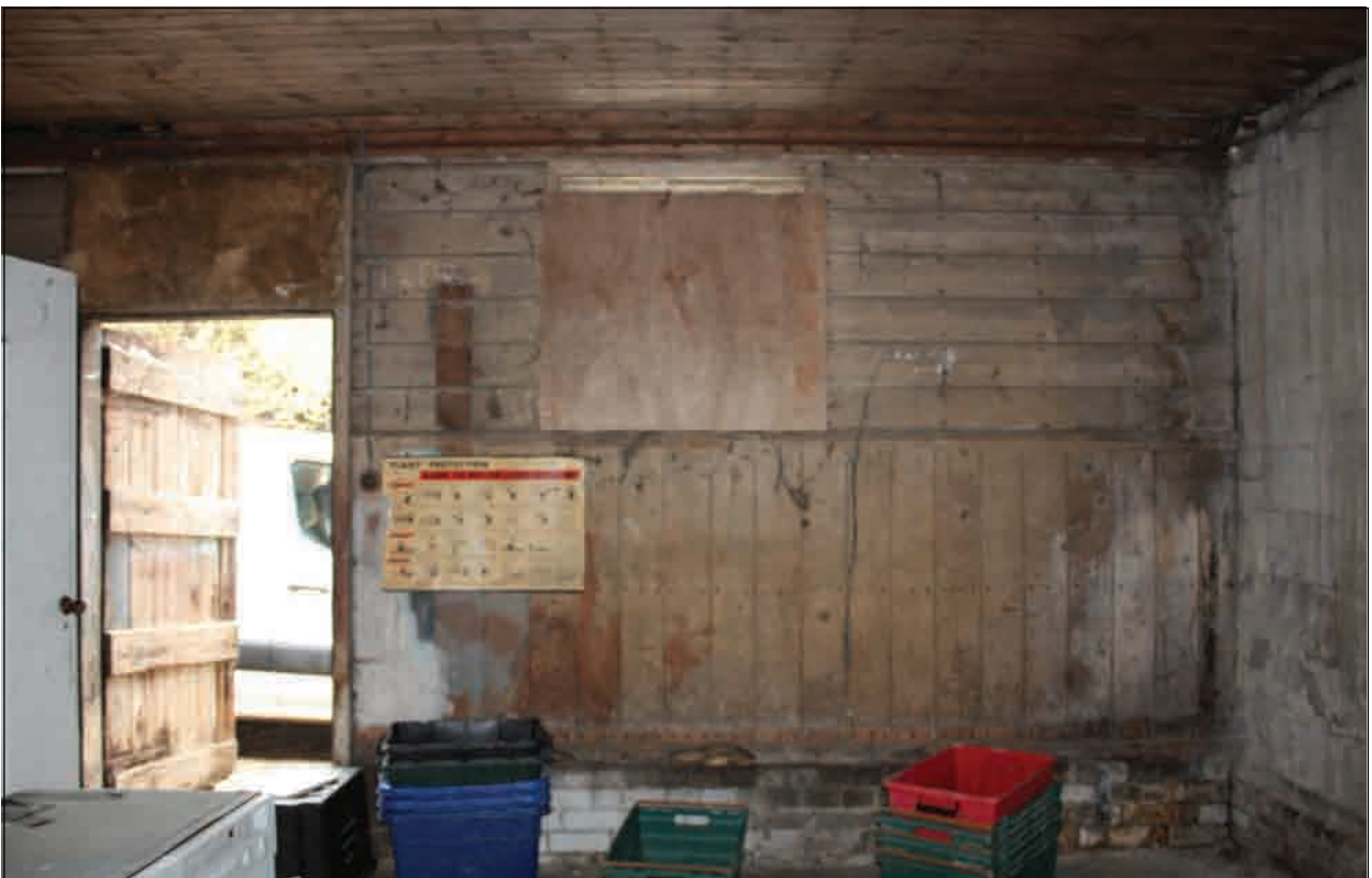
Plate 20: Room G1 interior, Building 2
