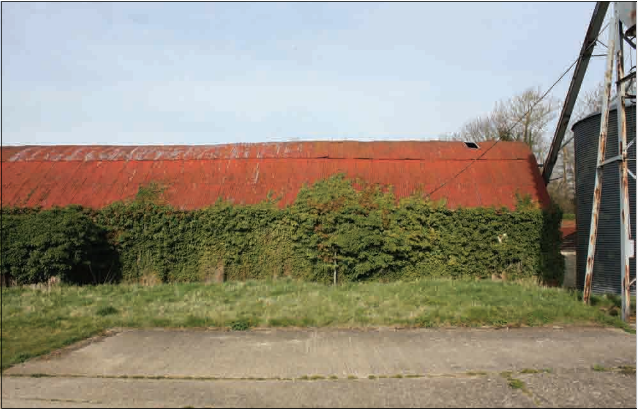
Plate 36: East-facing elevation, Building 3 (northern end)
