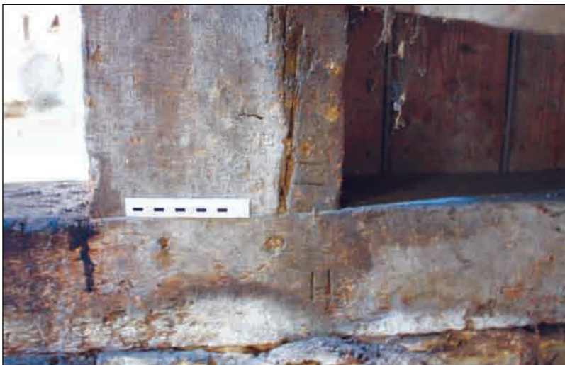
Plate 48: Carpenter's mark, Building 3
