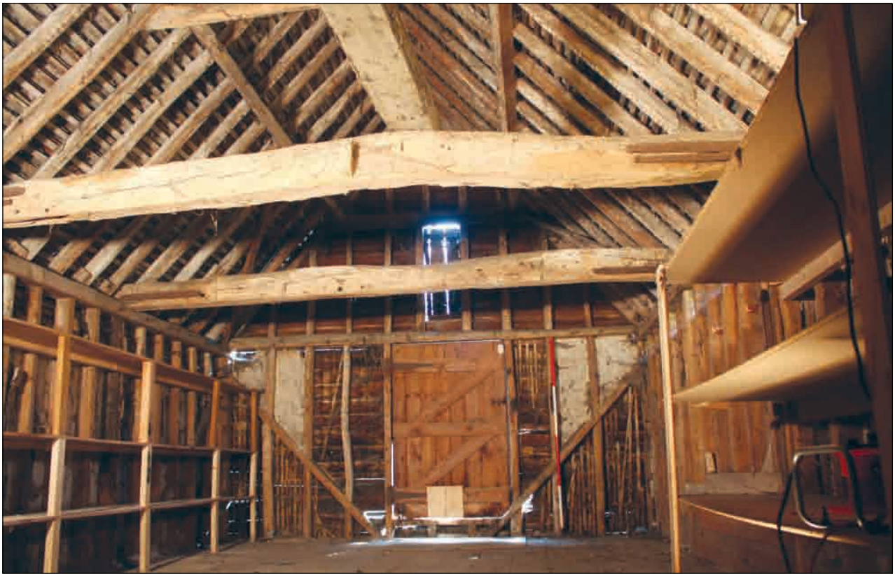
Plate 13: Interior of Building 1
