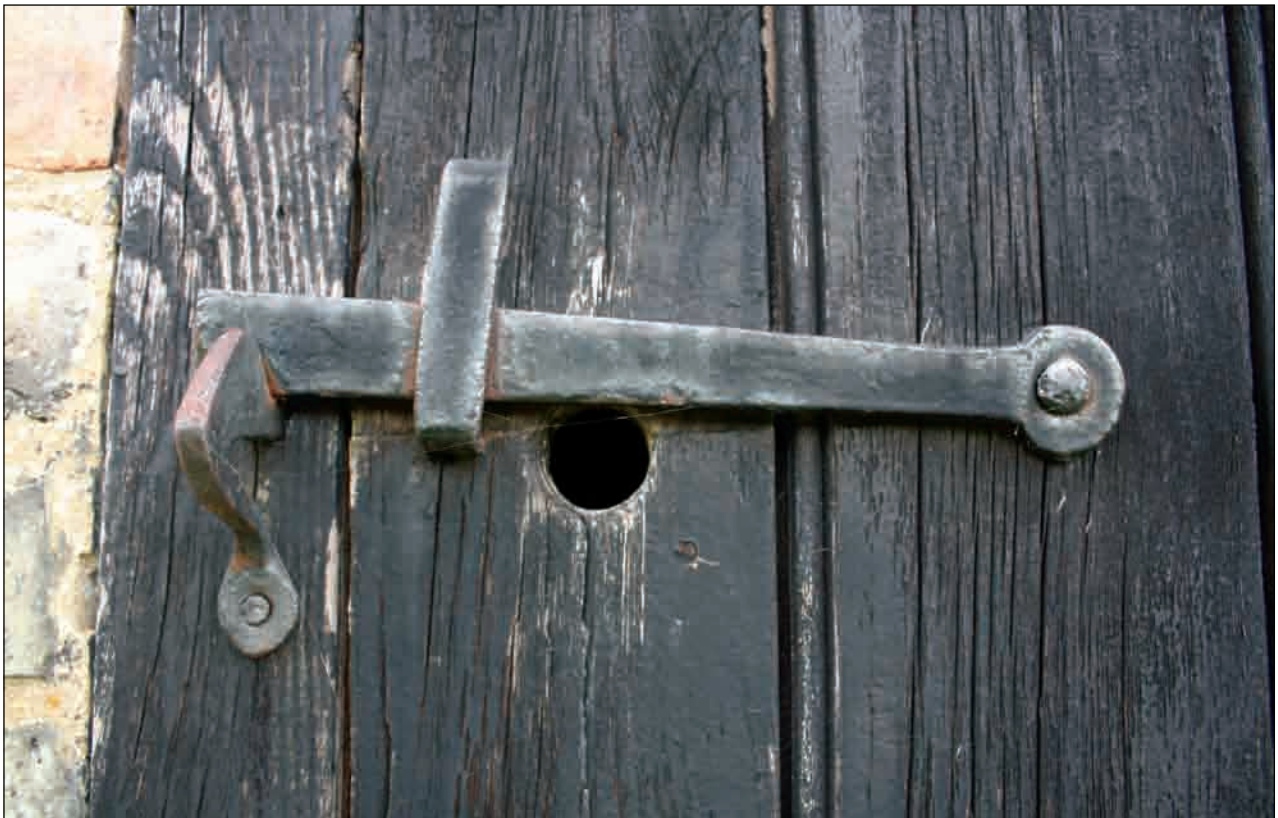
Plate 42: Detail of door latch on entrance door, Building 3
