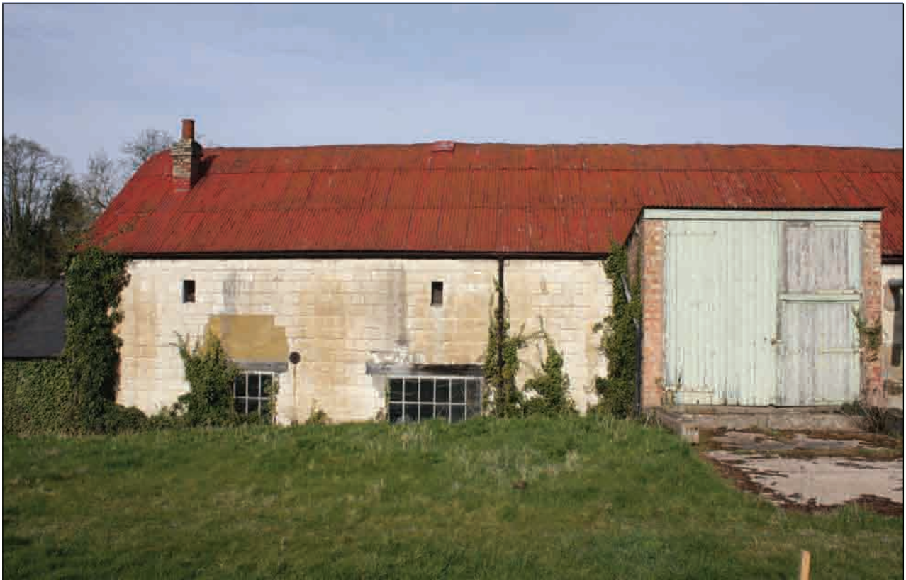
Plate 30: East-facing elevation, Building 3 (southern end)
