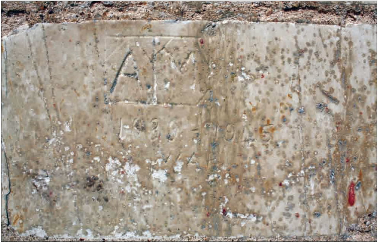
Plate 34: Graffiti on clunch block, east-facing elevation, Building 3
