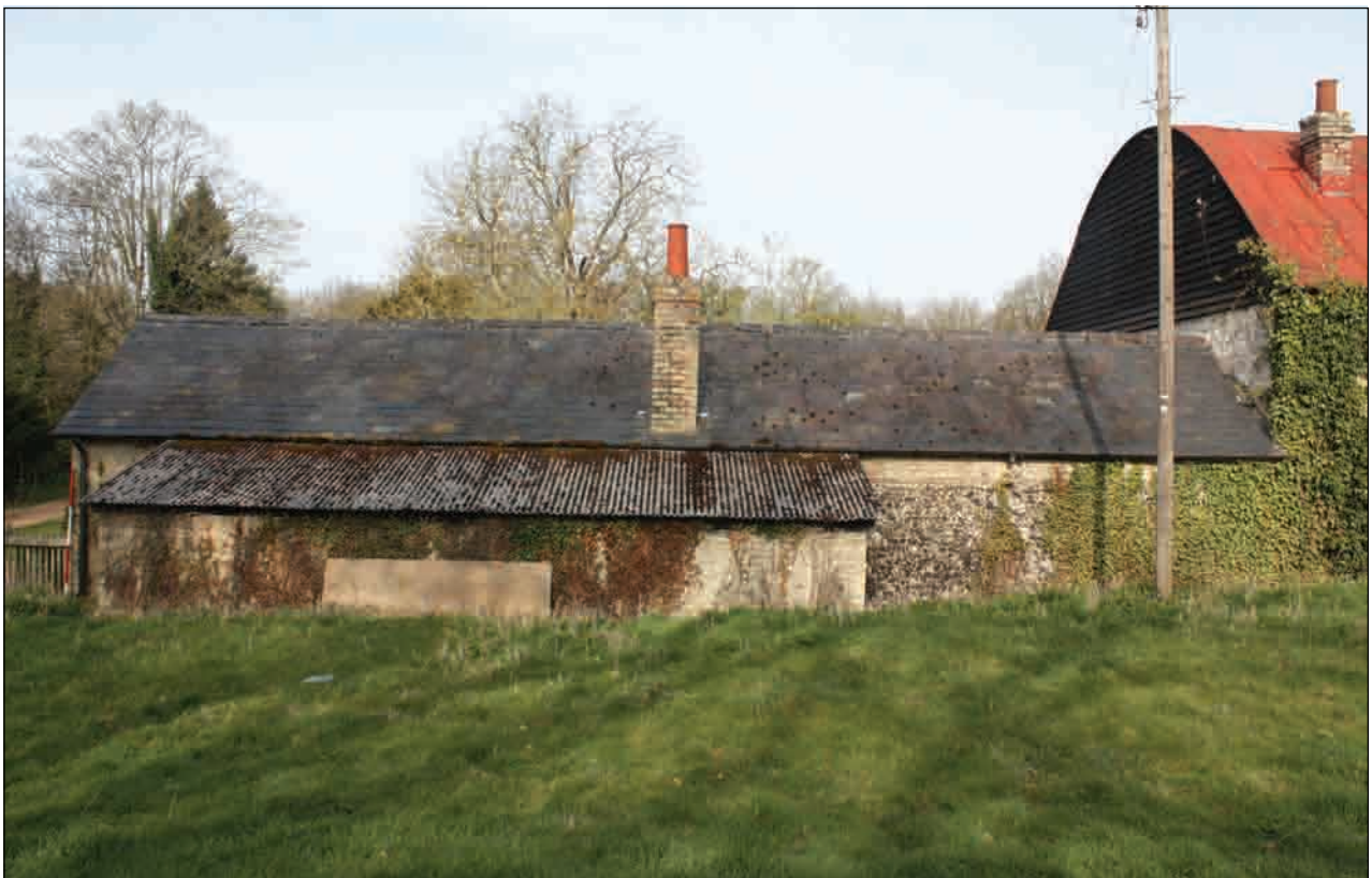
Plate 14: East-facing elevation, Building 2
