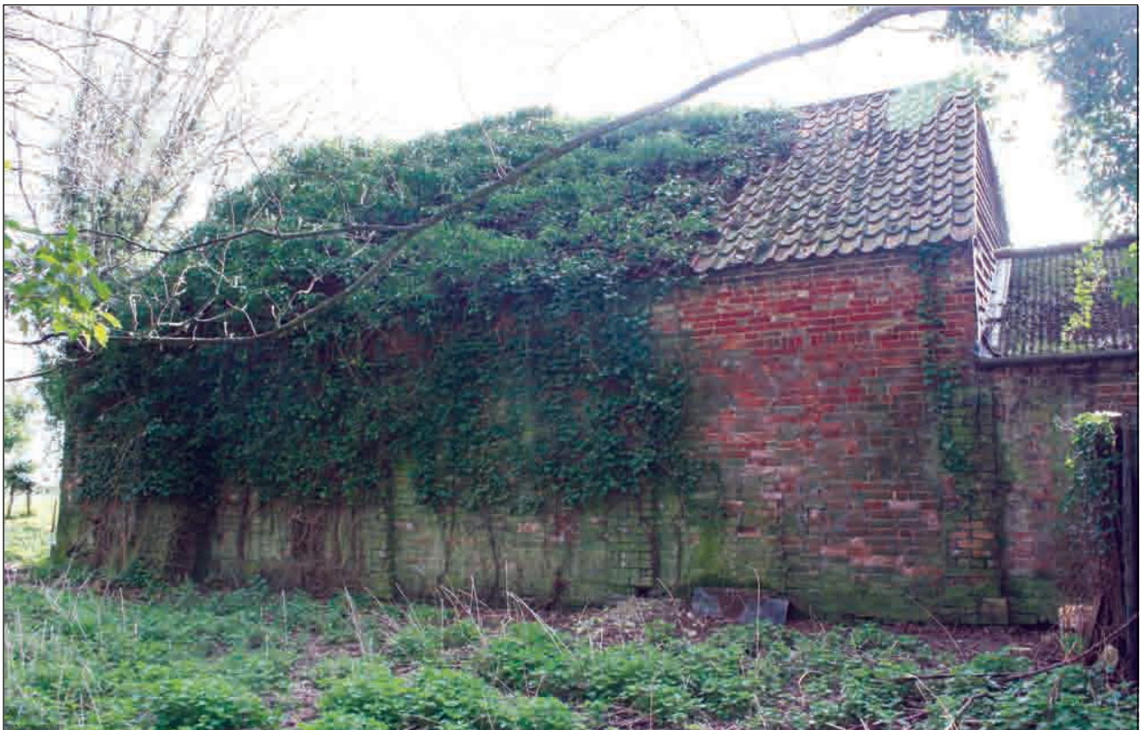
Plate 70: West-facing elevation, Building 5 (north)
