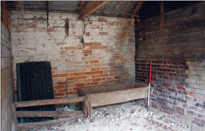
Plate 79: Troughs, Building 5 (south)
