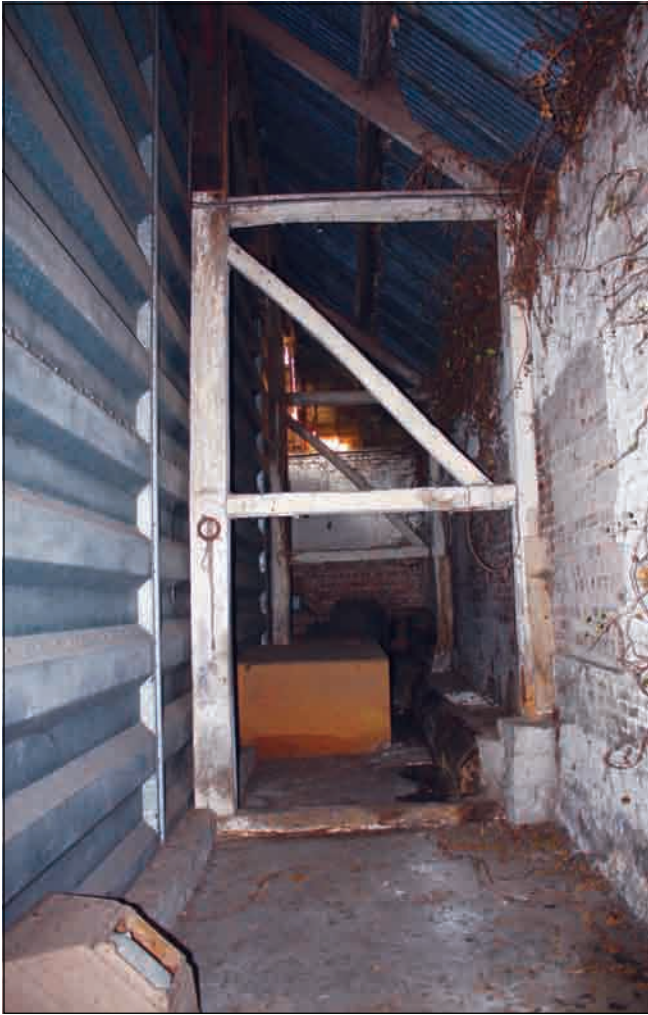
Plate 57: Remnants of aisled bay, Building 3, northern end
