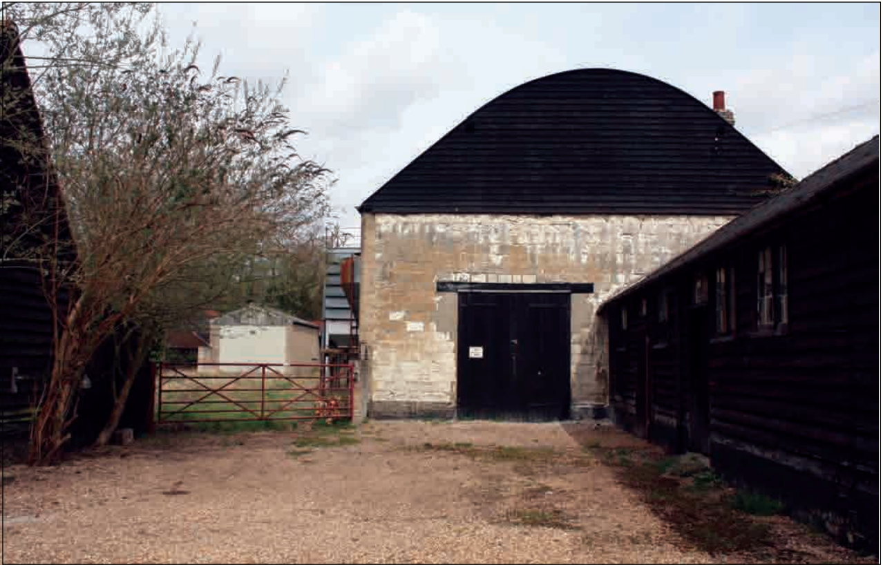
Plate 46: South-facing elevation, Building 3
