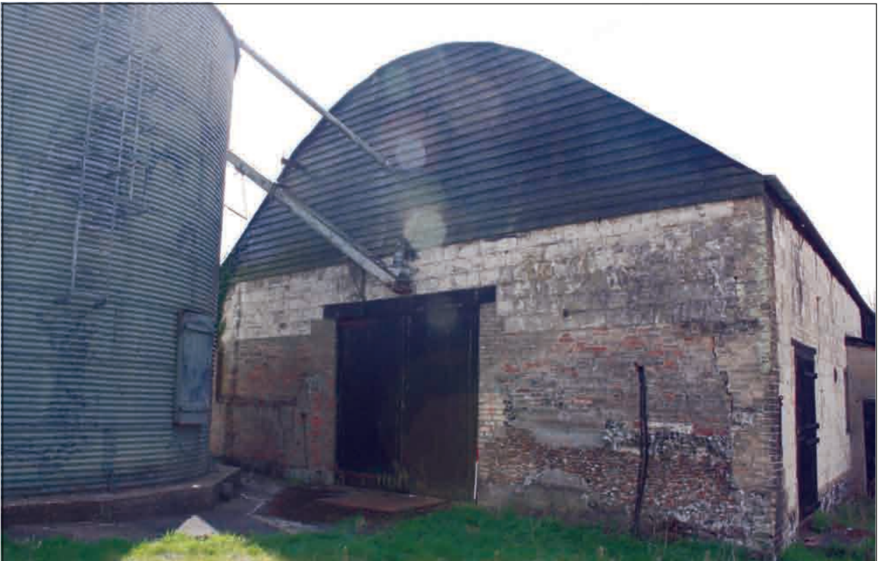
Plate 37: North-facing elevation, Building 3
