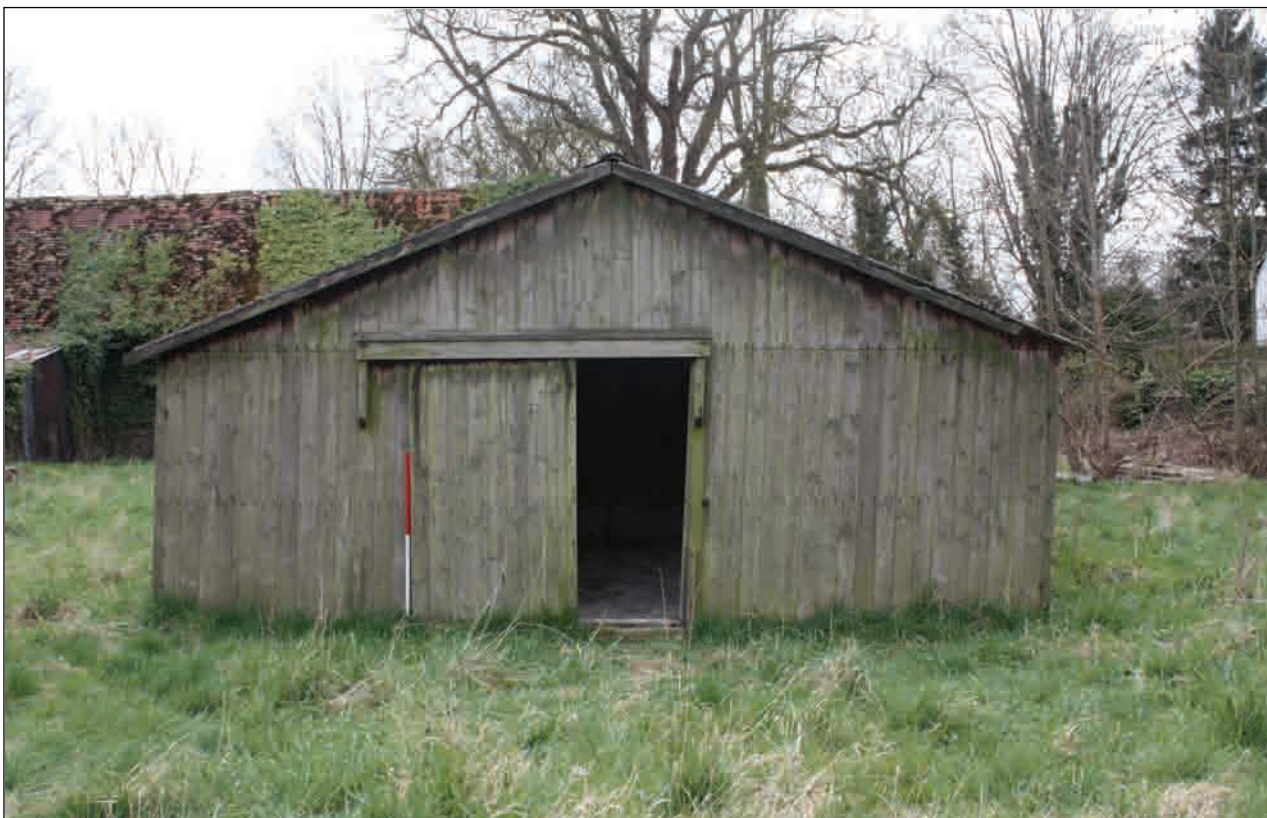
Plate 83: North-facing elevation, Building 6
