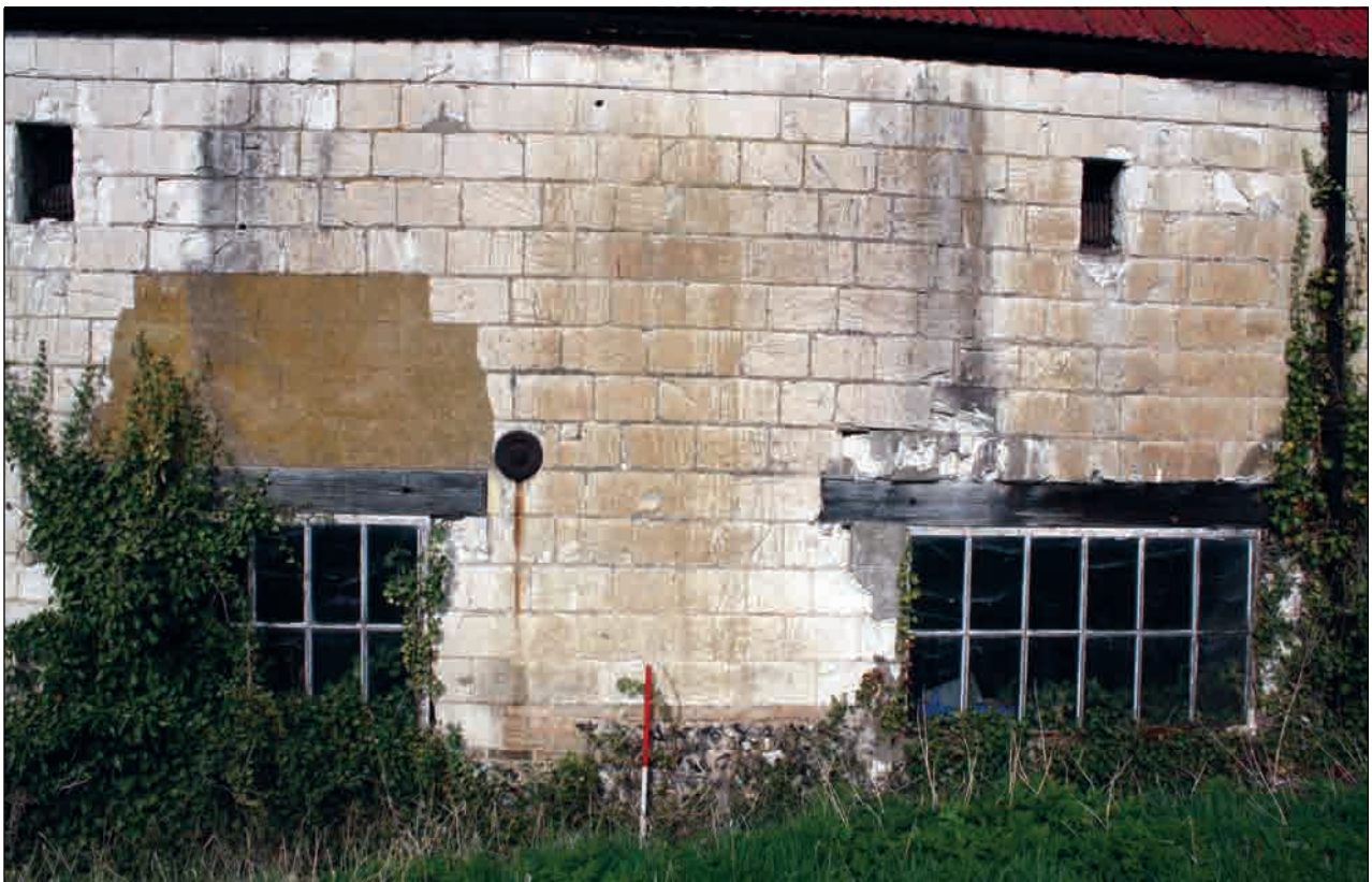
Plate 32: Windows on east-facing elevation, Building 3
