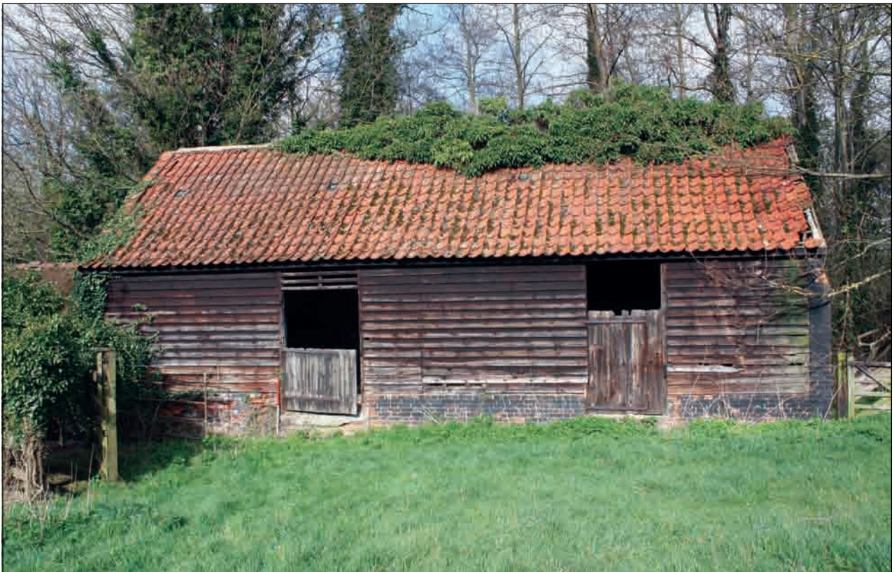
Plate 67: East-facing elevation, Building 5 (north)
