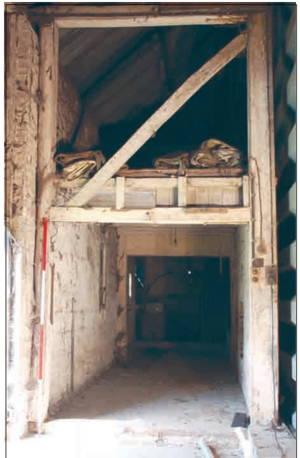
Plate 56: Remnants of aisled bay, building 3, northern end
