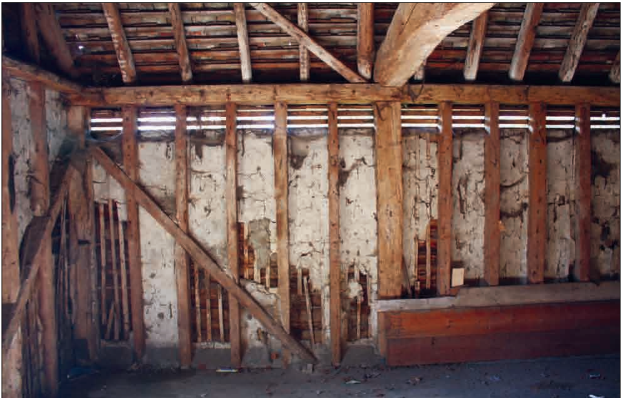
Plate 11: Lath and plaster between upright timbers, Building 1
