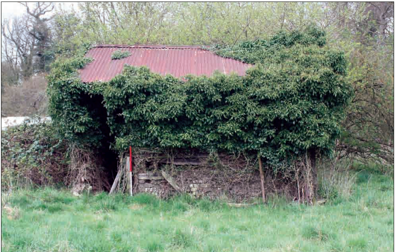
Plate 87: East-facing elevation, Building 7
