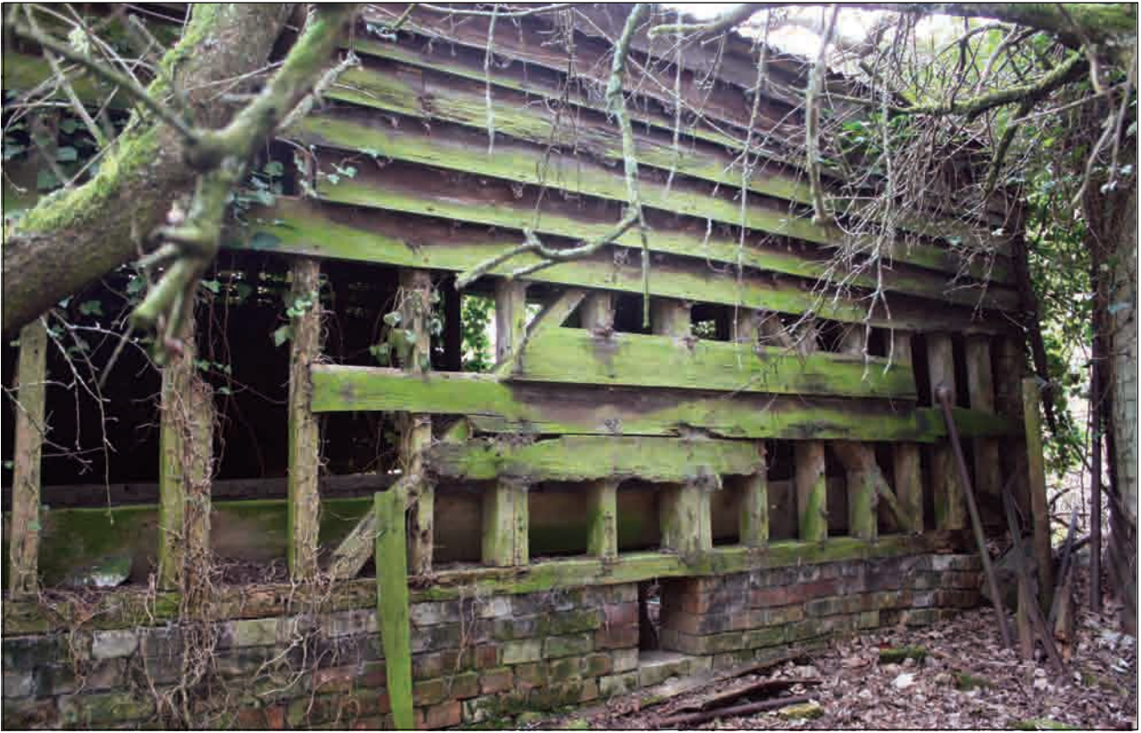
Plate 88: West-facing elevation, Building 7
