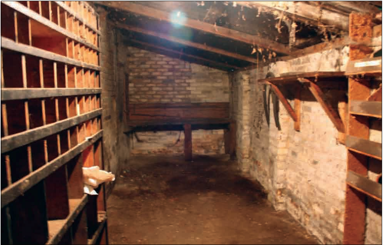
Plate 28: Room G4 interior, Building 2
