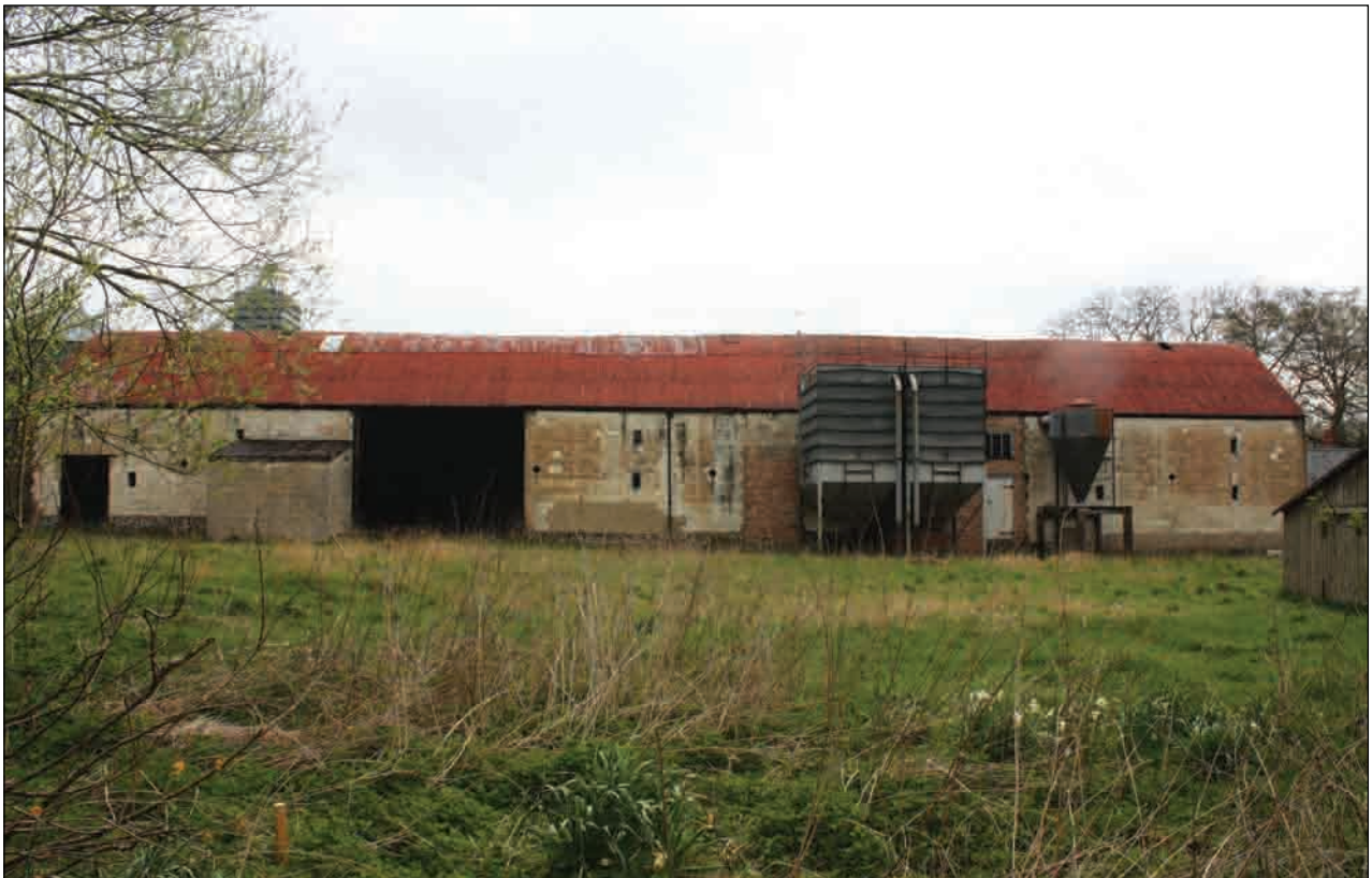
Plate 38: West-facing elevation, Building 3
