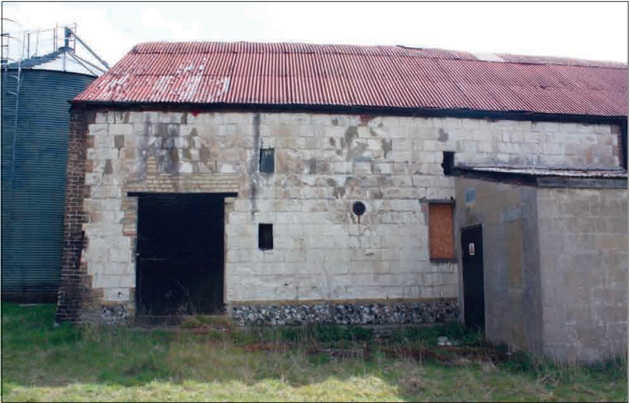
Plate 40: West-facing elevation, Building 3 (northern end)
