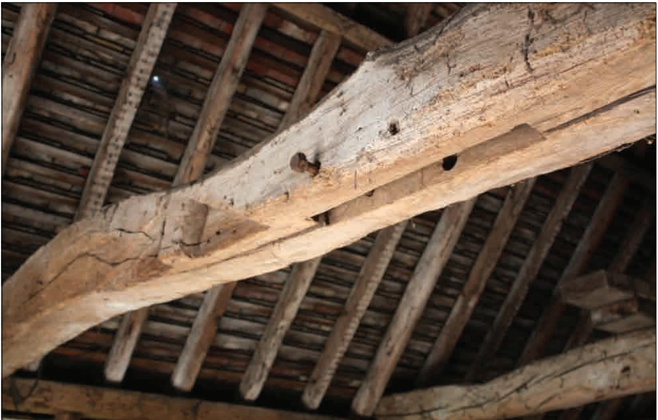
Plate 12: Detail of re-used tie-beam, Building 1
