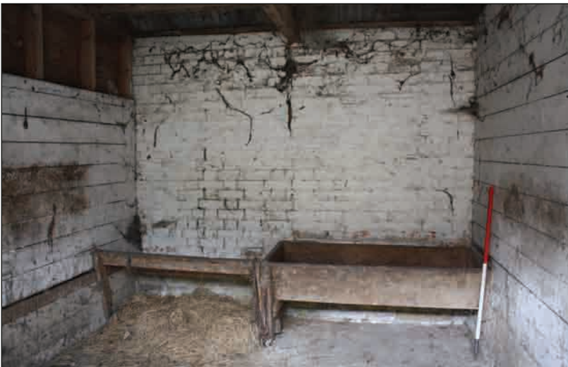
Plate 81: Troughs, Building 5 (south)
