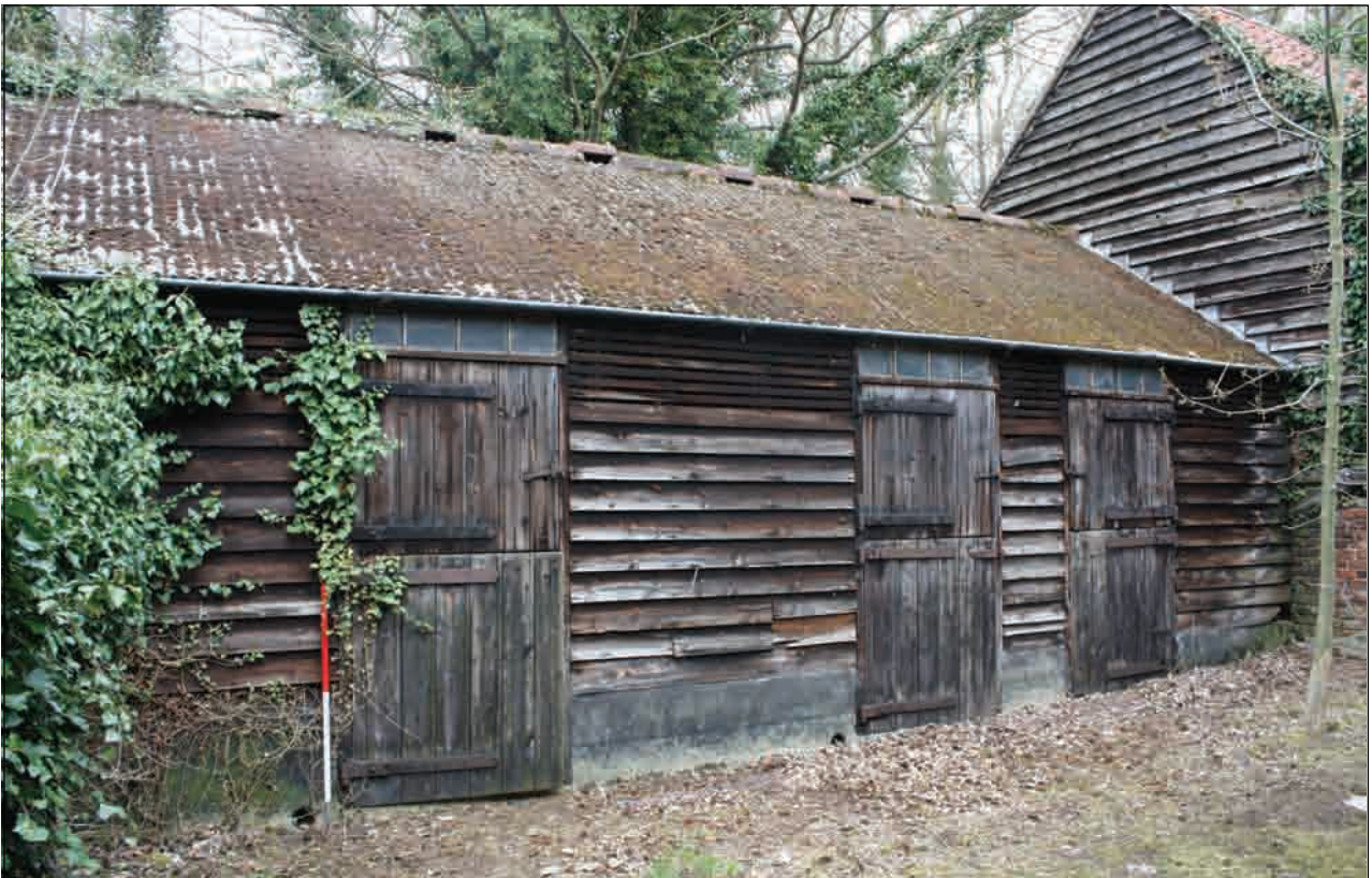
Plate 71: East-facing elevation, Building 5 (south)
