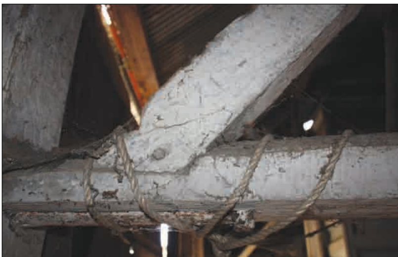
Plate 50: Carpenter's mark, Building 3
