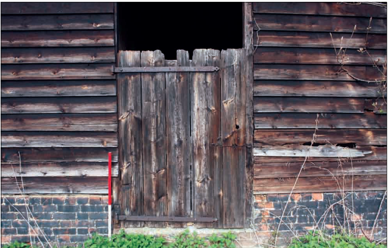
Plate 68: Two-part stable door, Building 5 (north)
