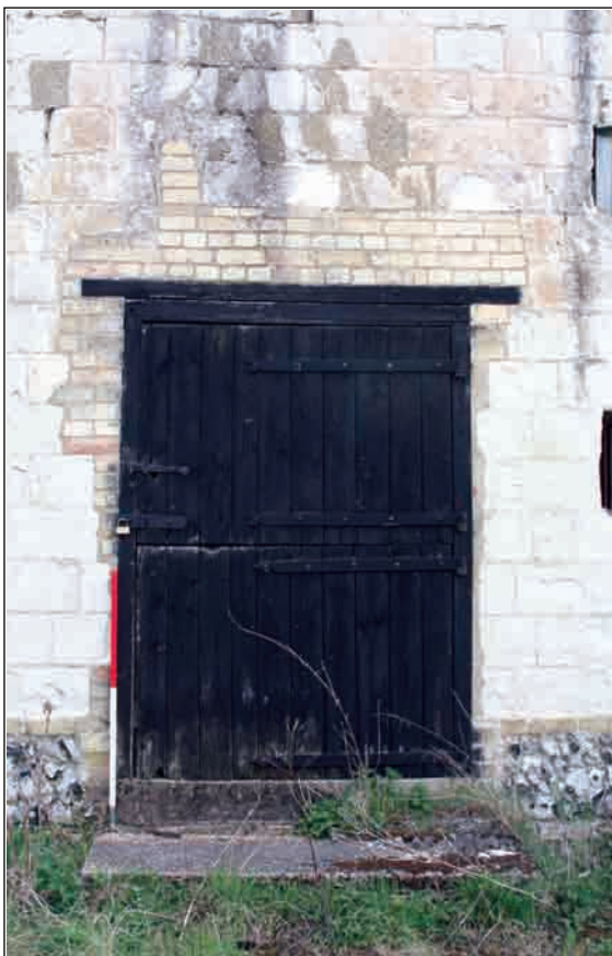
Plate 39: Door on west-facing elevation, Building 3
