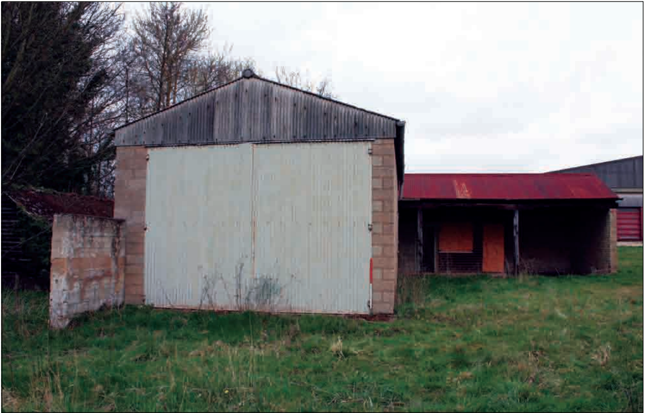
Plate 59: South-facing elevation, Building 4
