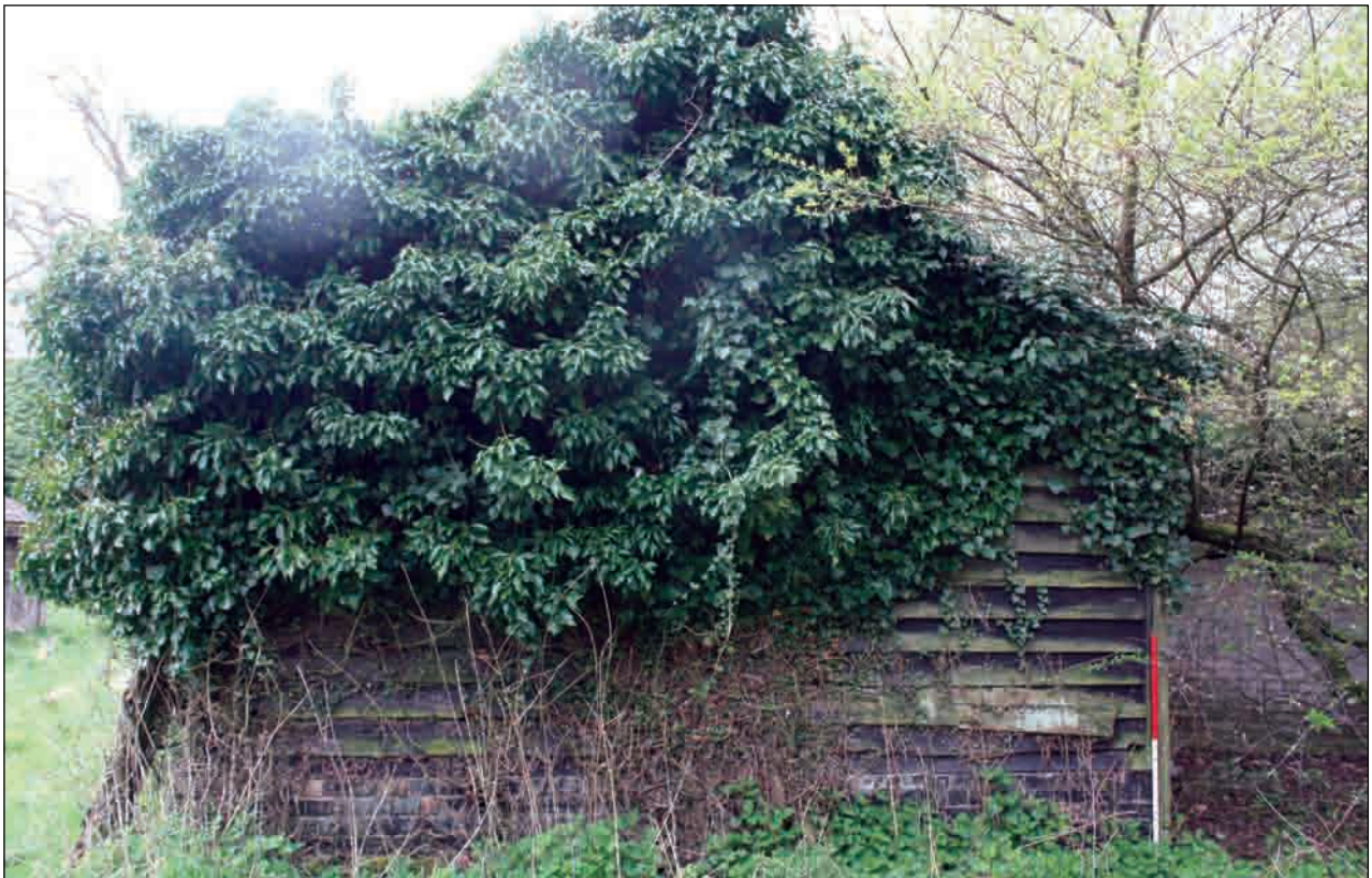
Plate 86: North-facing elevation, Building 7
