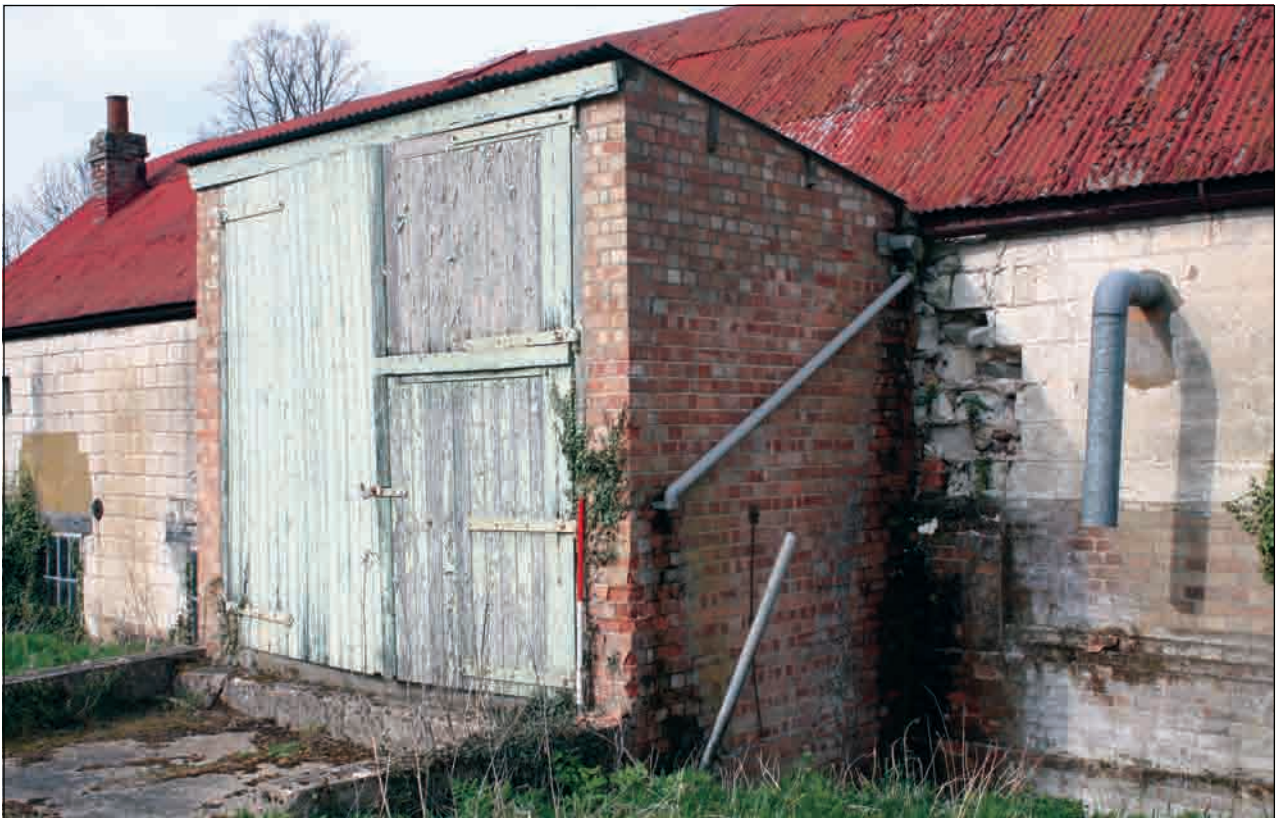
Plate 35: 20th century loading door, east-facing elevation, Building 3
