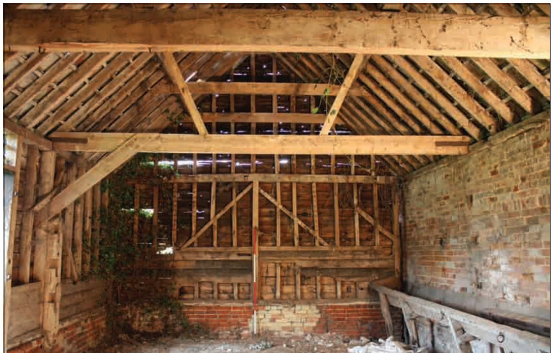
Plate 78: Interior view, Building 5 (north)
