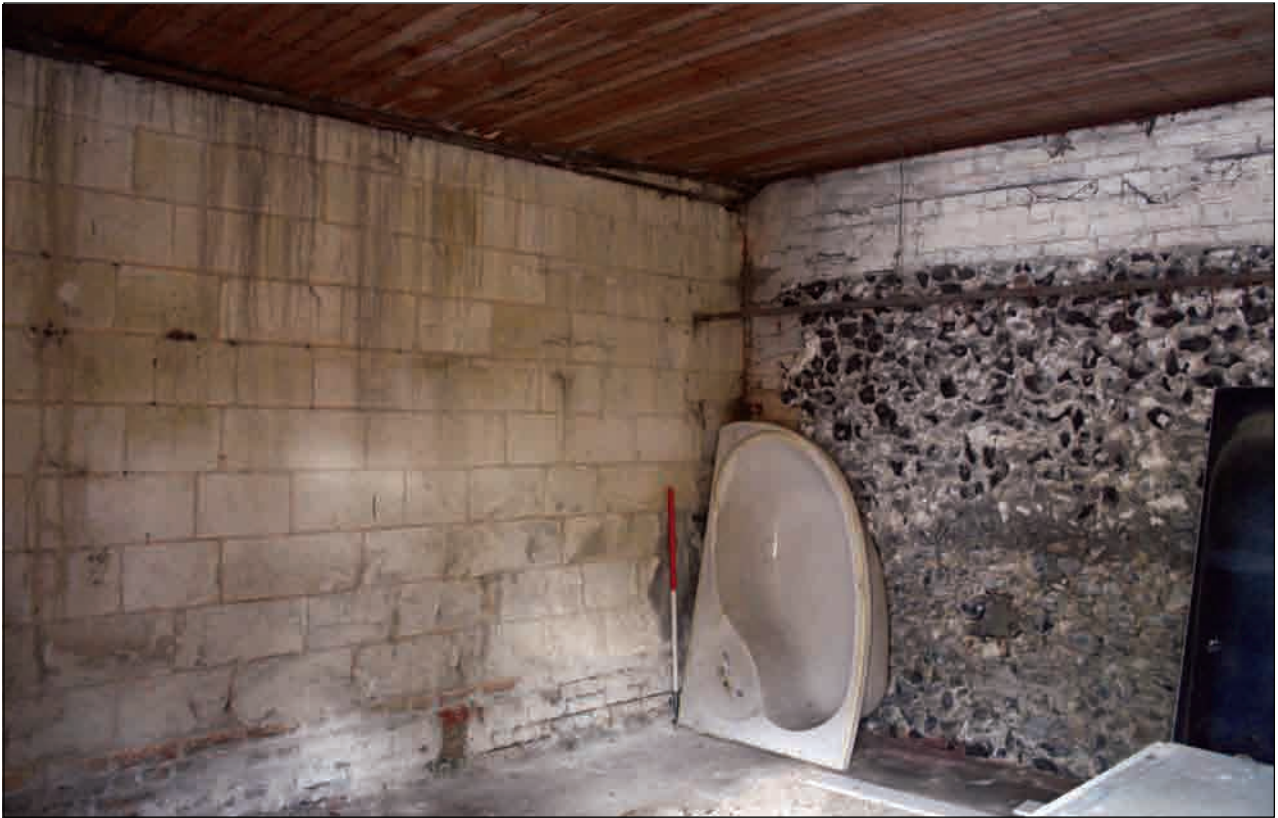
Plate 19: Room G1 interior, Building 2
