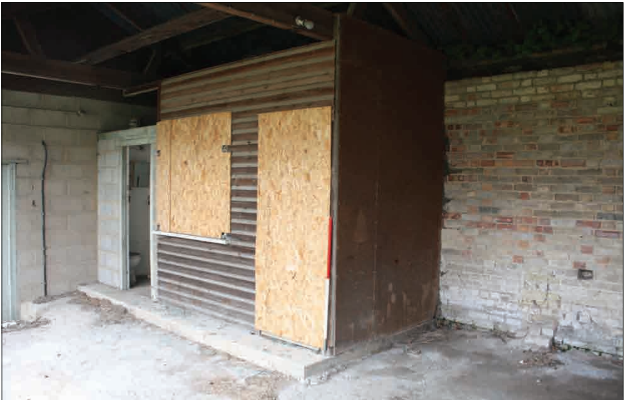
Plate 65: Modern internal facilities, Building 4
