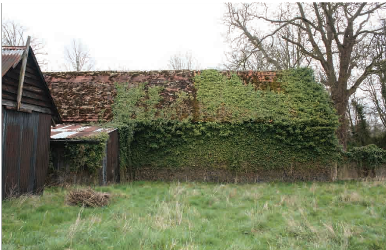
Plate 7: North-facing elevation, Building 1
