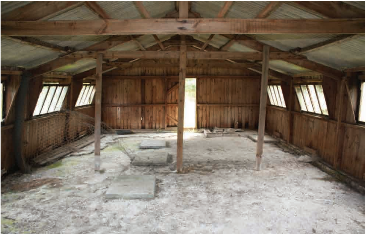
Plate 84: Interior view, Building 6
