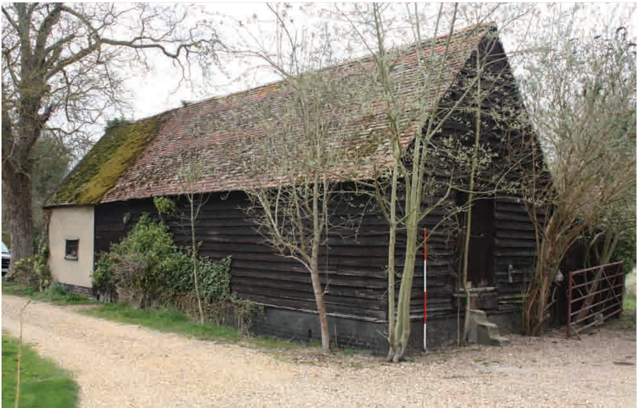
Plate 2: Building 1, from south-east
