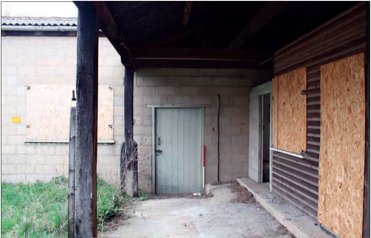
Plate 62: East-facing elevation, Building 4
