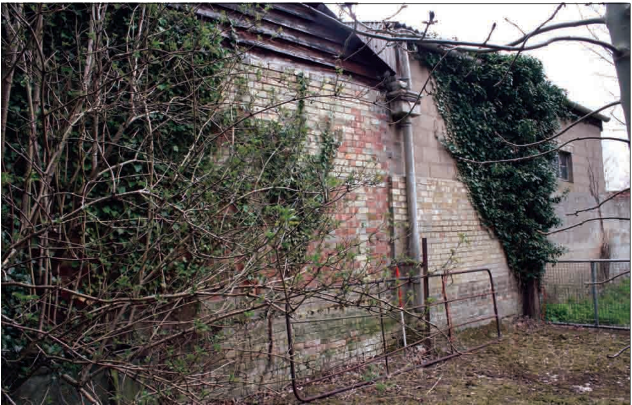
Plate 64: West-facing elevation, Building 4
