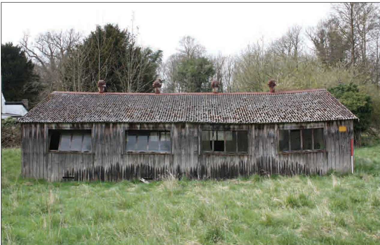
Plate 82: West-facing elevation, Building 6
