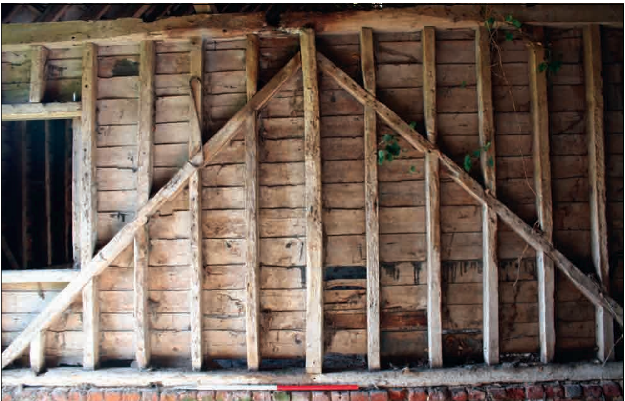
Plate 74: Internal partition, Building 5 (north)
