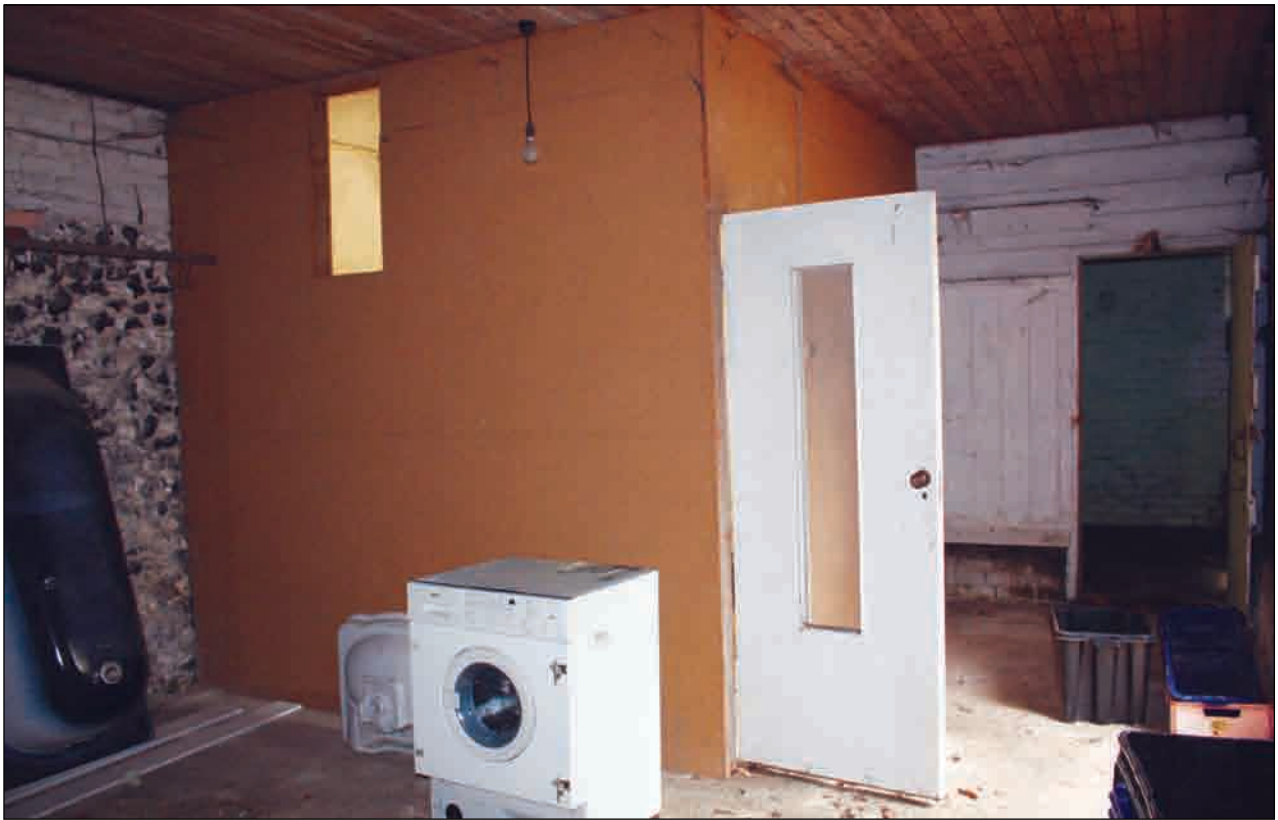
Plate 21: Room G1 interior, Building 2
