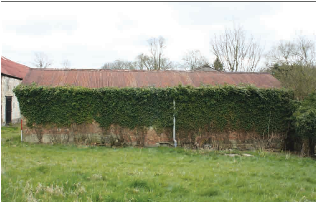
Plate 60: North-facing elevation, Building 4
