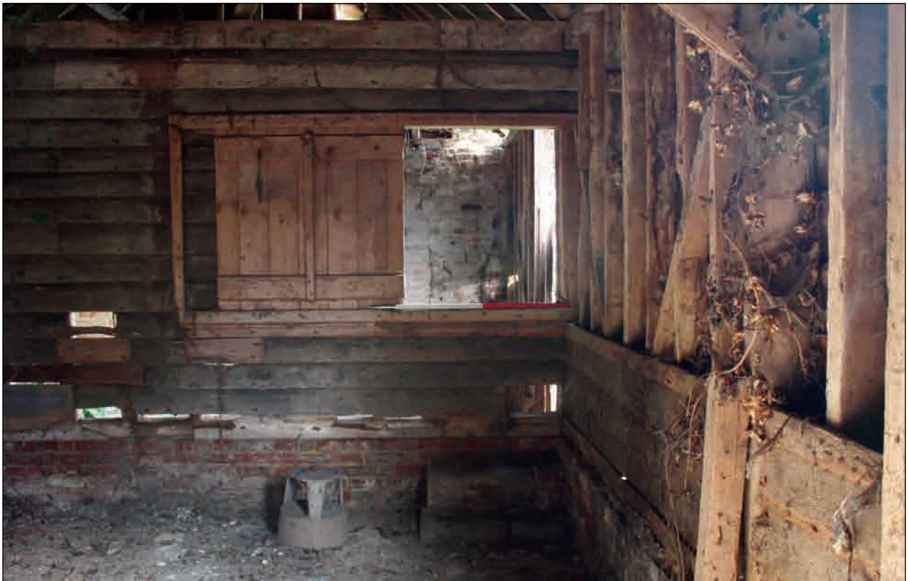
Plate 75: Detail of internal opening, Building 5 (north)
