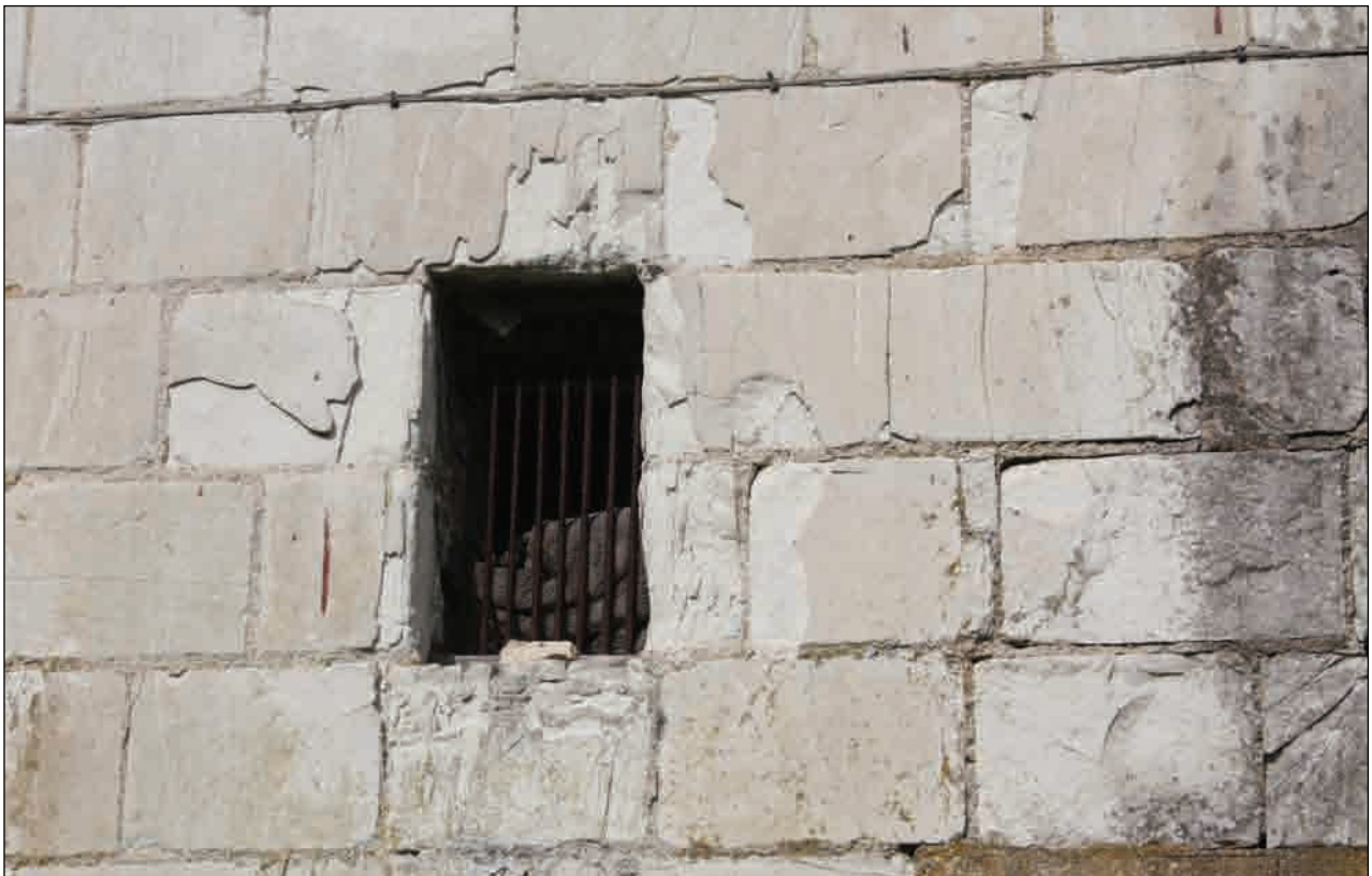
Plate 31: Ventilation opening on east-facing elevation, Building 3
