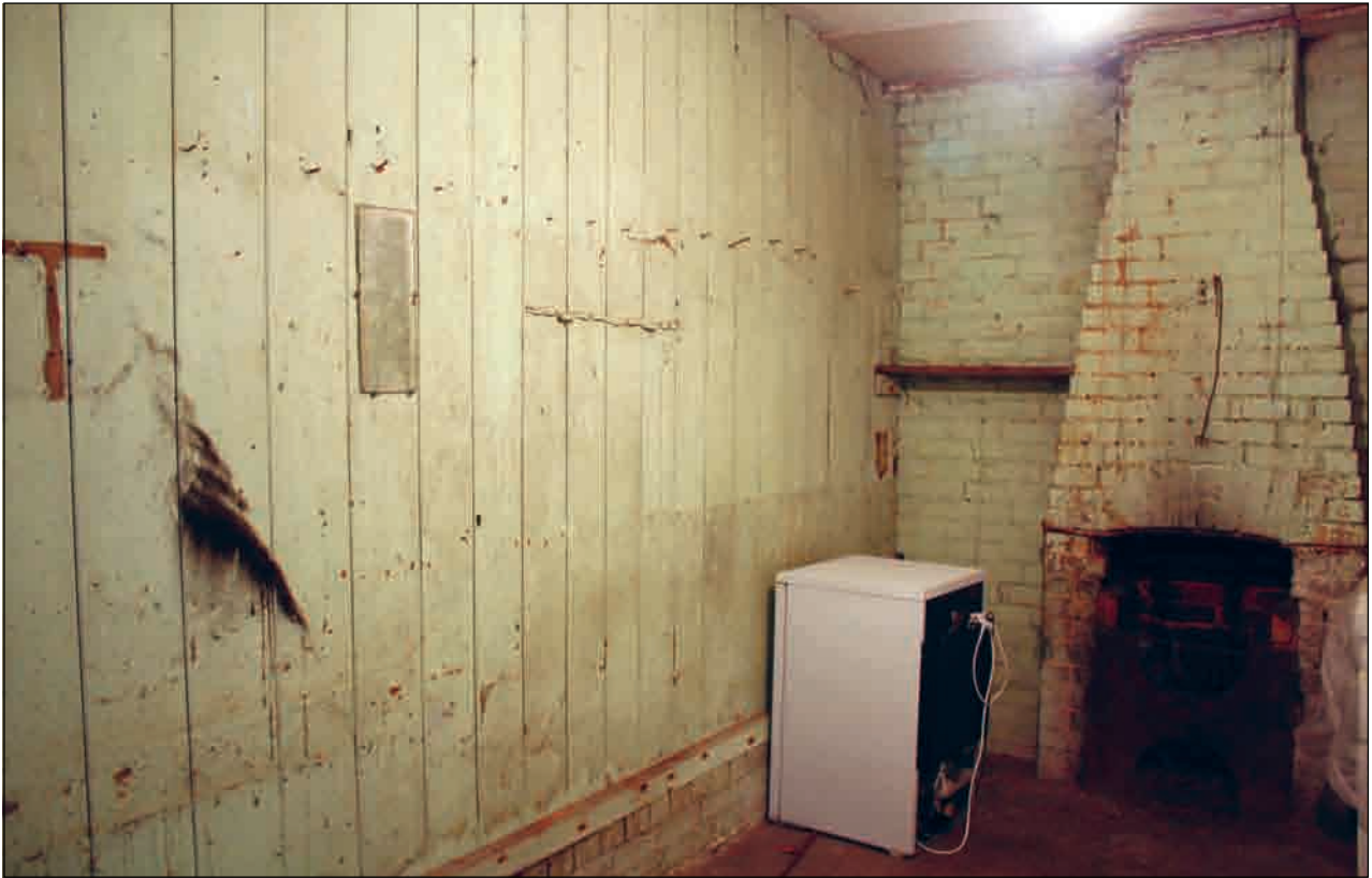
Plate 24: Room G2 interior, Building 2
