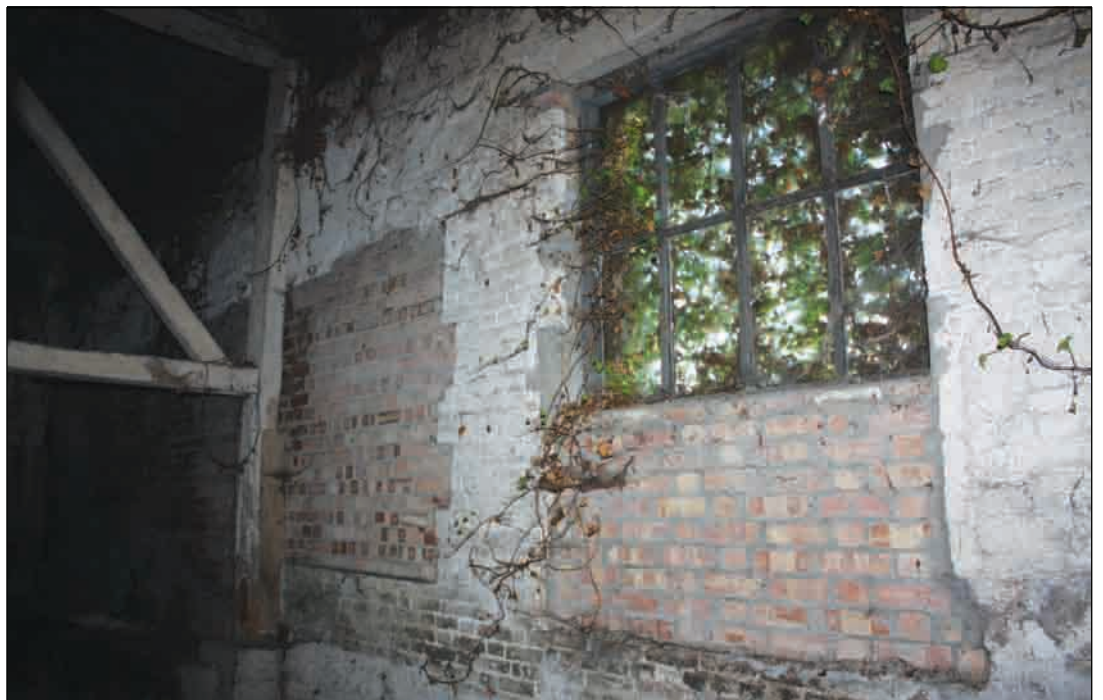
Plate 58: Blocked-up windows, eastern elevation, Building 3
