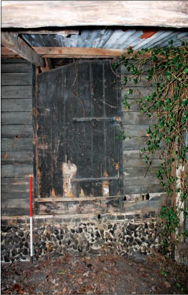
Plate 9: Door on north-facing elevation, Building 1
