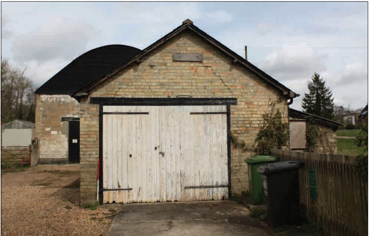
Plate 15: South-facing elevation, Building 2
