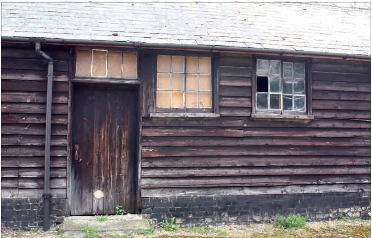
Plate 18: Entrance on west-facing elevation, Building 2
