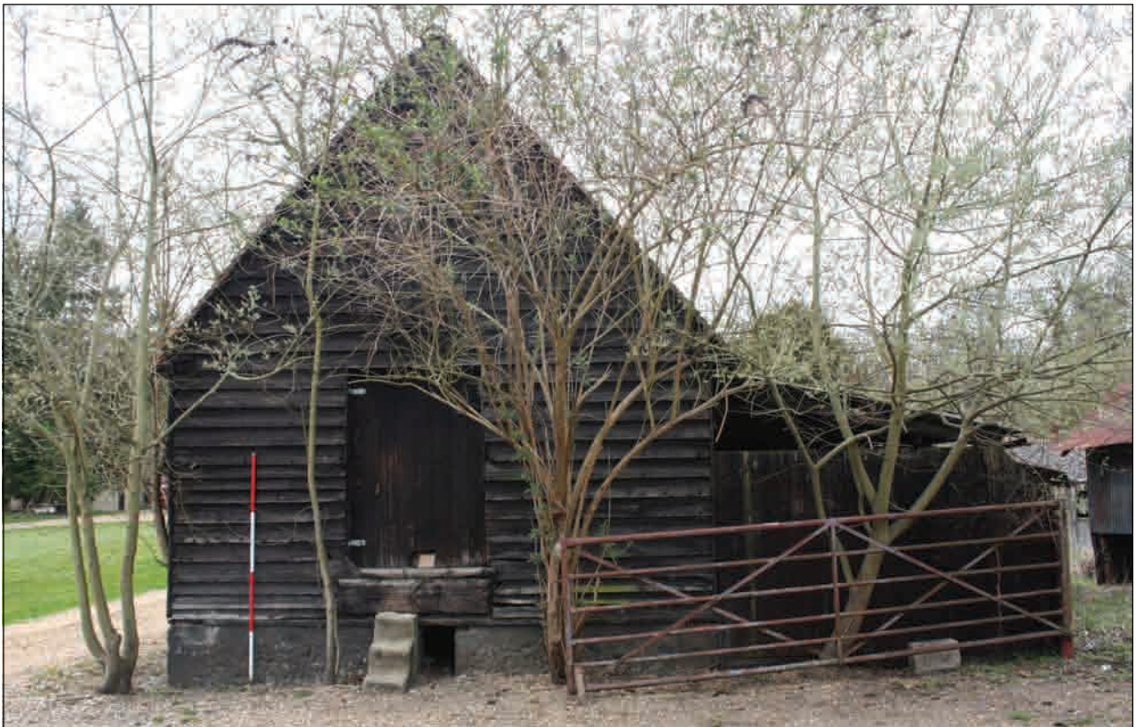
Plate 3: East-facing elevation, Building 1
