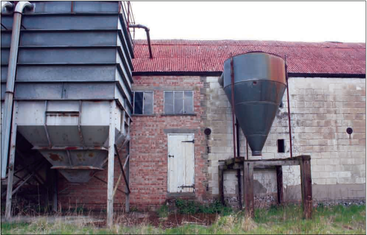
Plate 44: Blocked-up opening, west-facing elevation, Building 3
