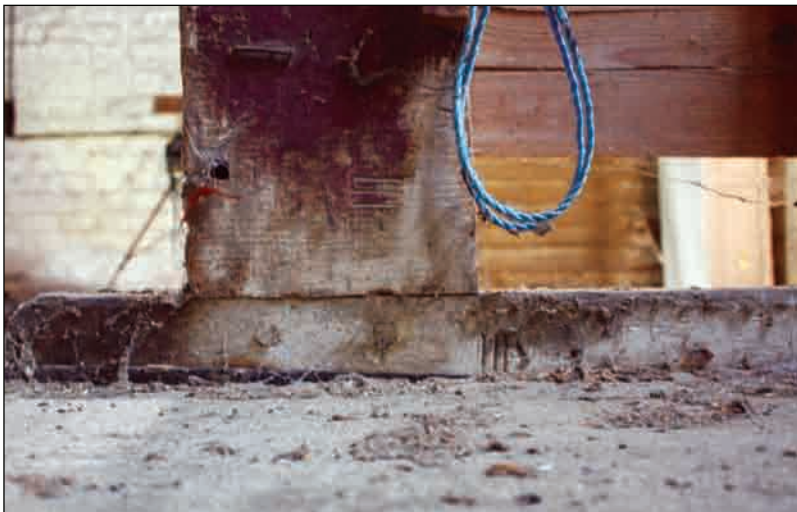
Plate 49: Carpenter's mark, Building 3
