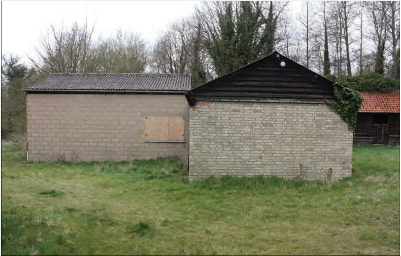
Plate 61: East-facing elevation, Building 4
