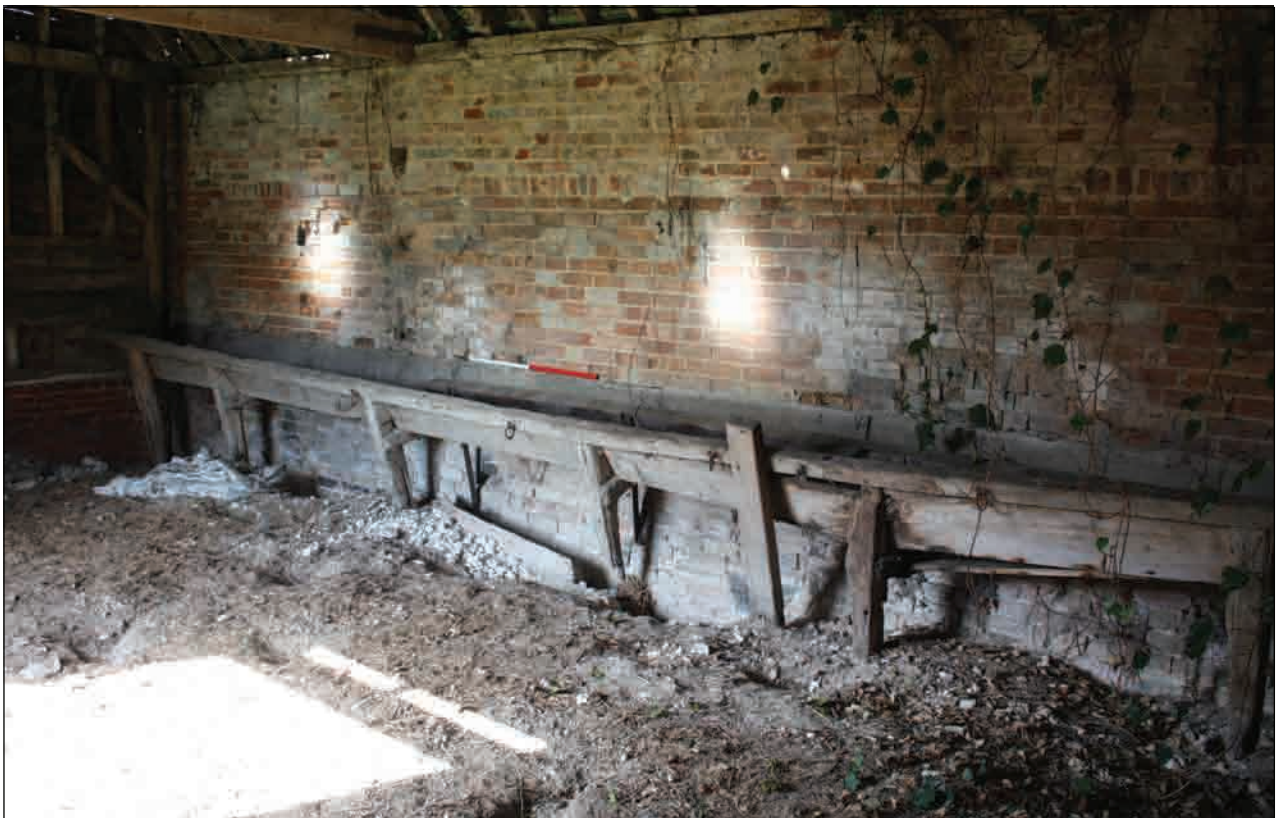
Plate 76: Troughs, Building 5 (north)
