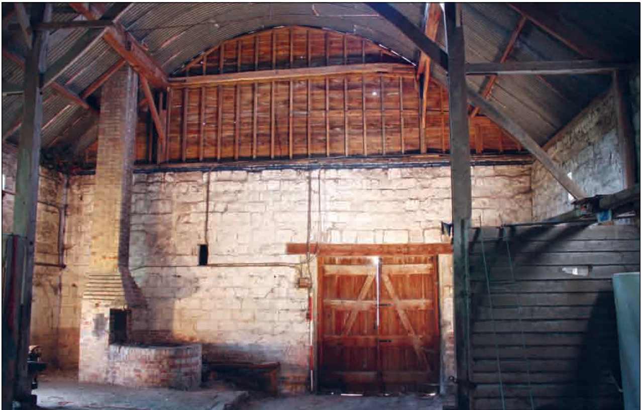
Plate 47: Southern gable end and brick forge, Building 3
