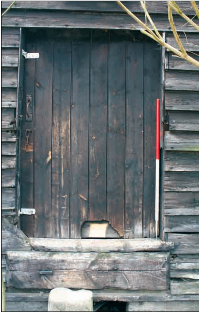
Plate 5: Entrance door on eastern elevation, Building 1
