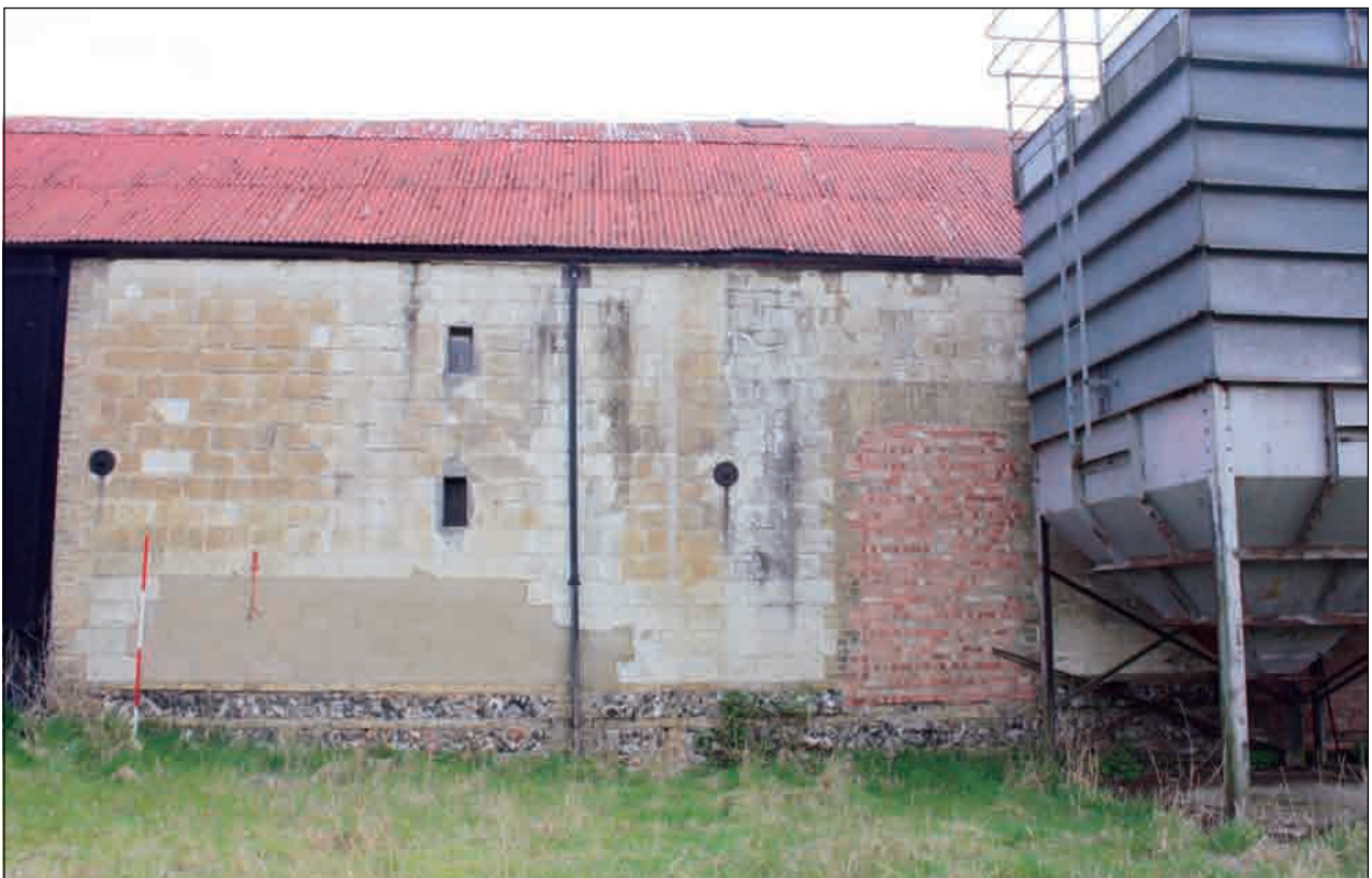
Plate 43: Ventilation openings, structural tie and blocked-up door, west-facing elevation, Building 3
