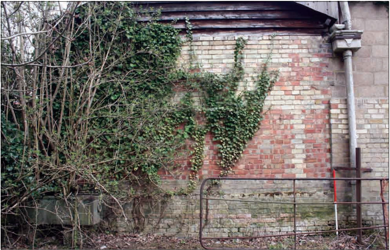
Plate 63: West-facing elevation, Building 4
