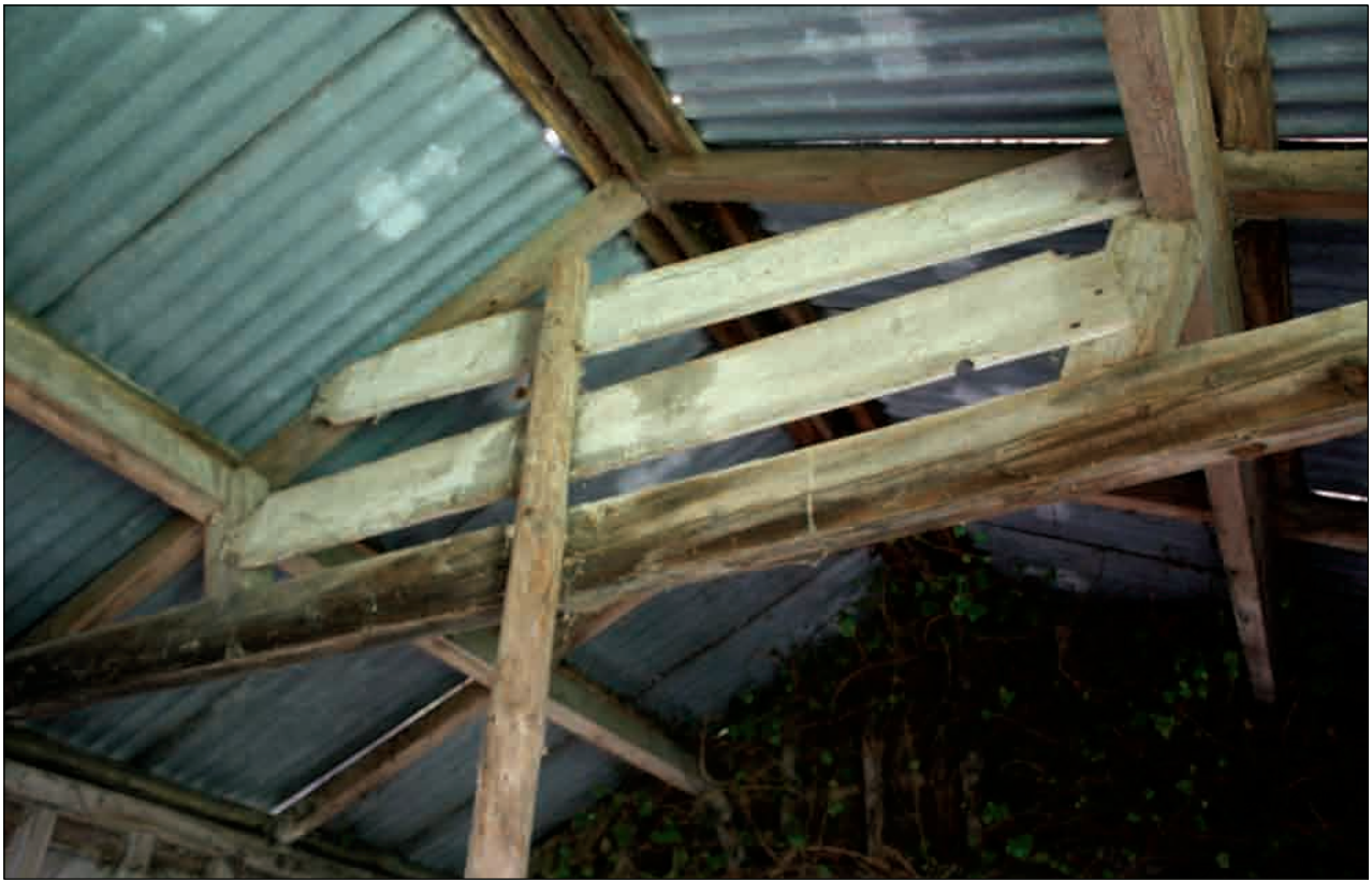
Plate 90: Modern/repaired roof structure, Building 7
