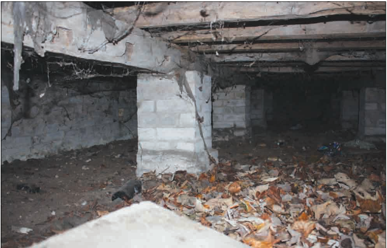
Plate 4: Brick plinths beneath Building 1
