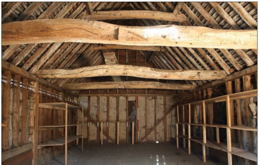
Plate 10: Interior of Building 1
