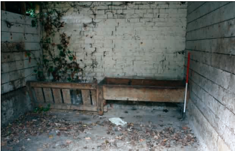
Plate 80: Troughs, Building 5 (south)
