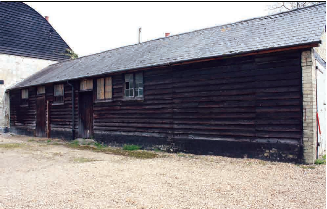
Plate 16: West-facing elevation, Building 2
