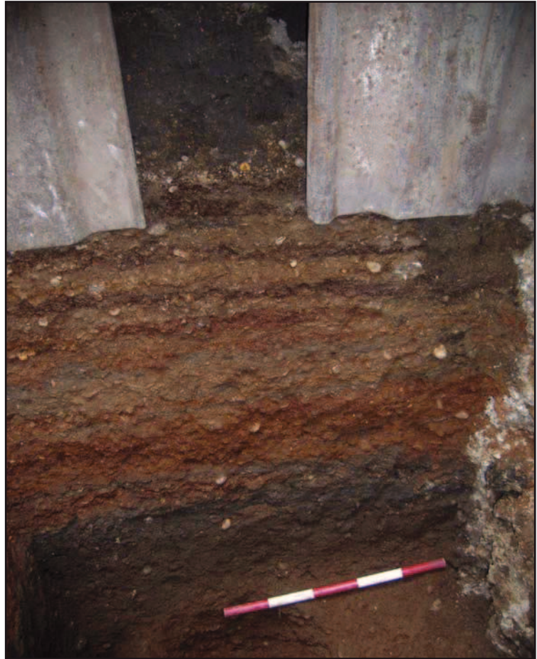
Plate 1: Testpit A; south facing section through metallised road surfaces
