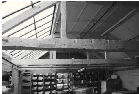
Plate 6: Block K details of roof timbers
