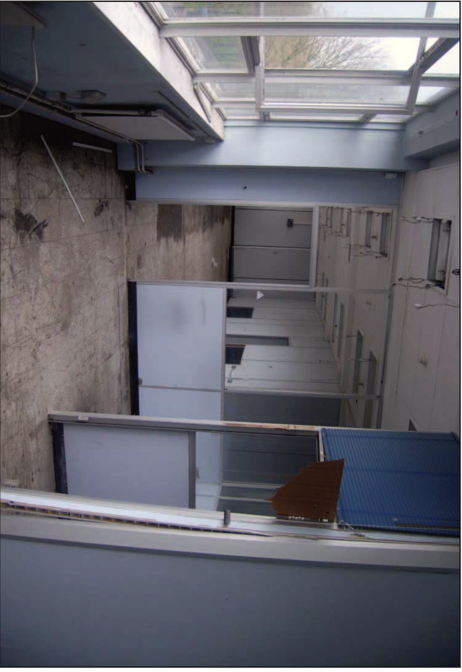
Plate 30: Offices at south end of Second Floor (Block A)
