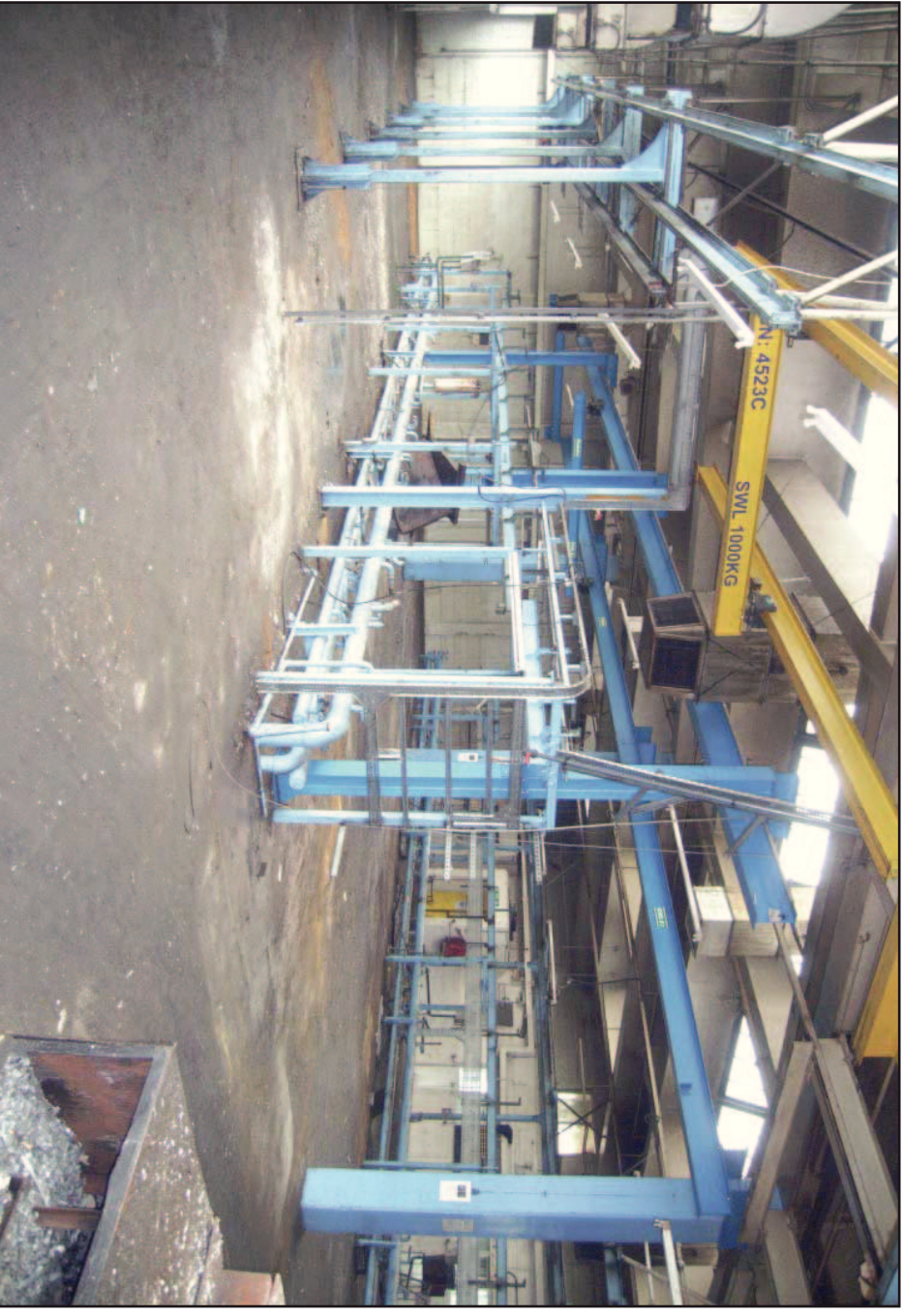
Plate 26: Foundry (1st floor Block C)
