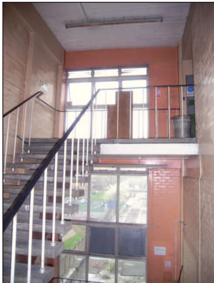
Plate 12: Staircase to north of clocking-in area
