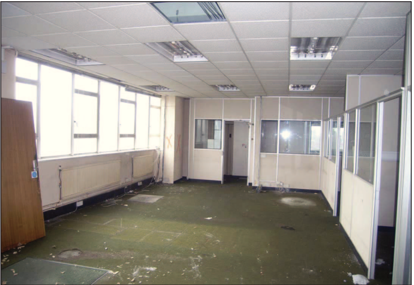
Plate 31: Offices in Block A (third floor)
