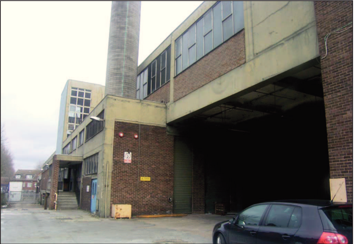
Plate 5: West elevation showing opening beneath Block B
