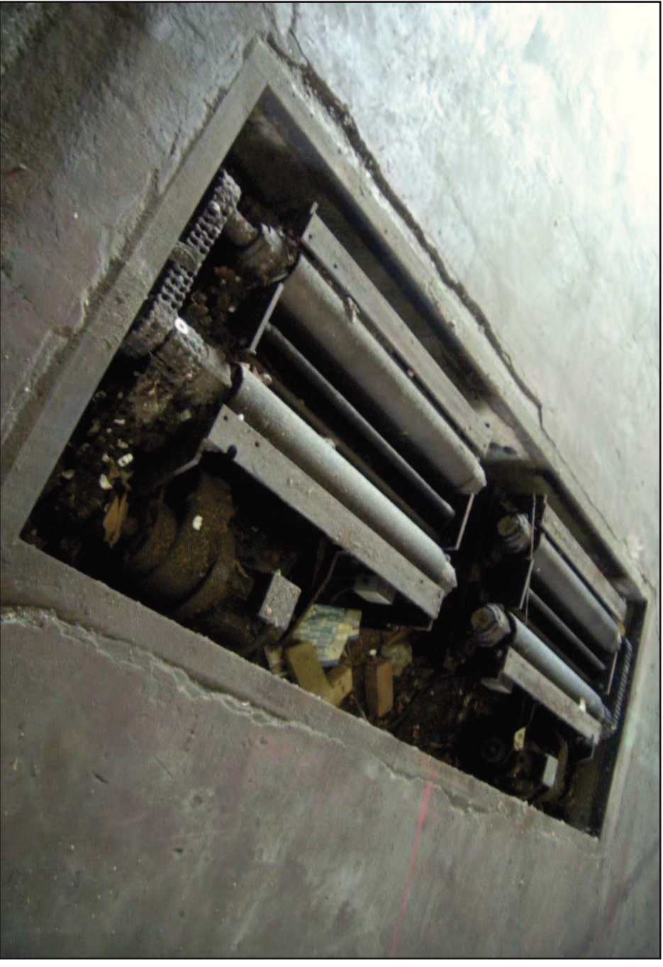
Plate 16: Rollers in floor of Block D
