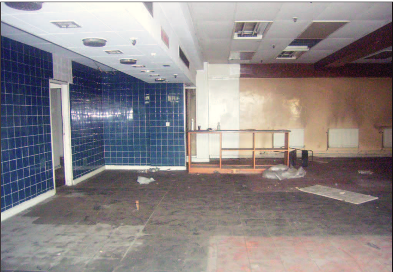
Plate 32: Canteen (Block A mezzanine between ground and first floor)
