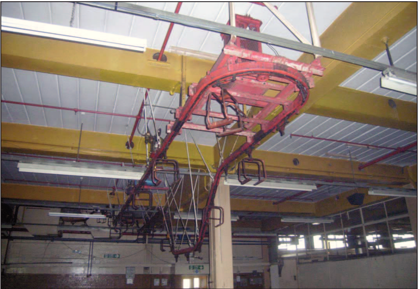
Plate 9: Overhead conveyor track in ground floor despatch area (Block B)
