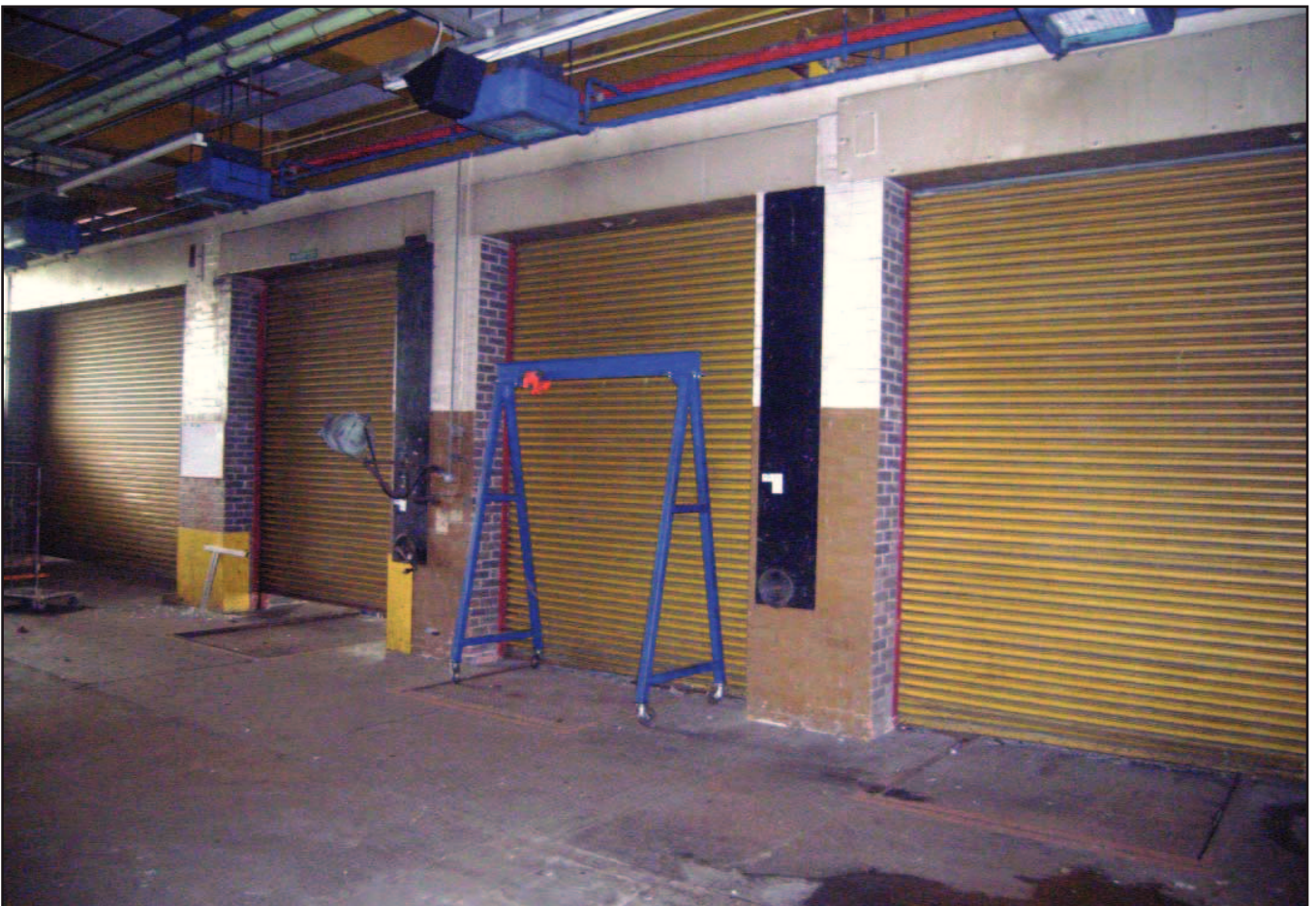
Plate 10: Loading bay at south end of ground floor despatch area (Block B)
