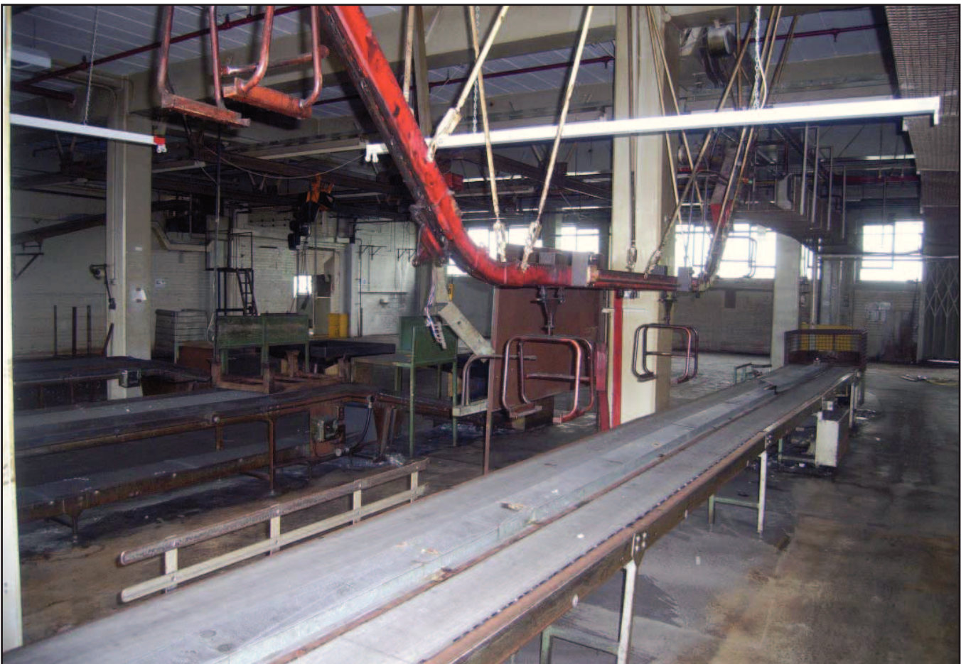
Plate 20: Conveyor and overhead track in Fetting Dept
