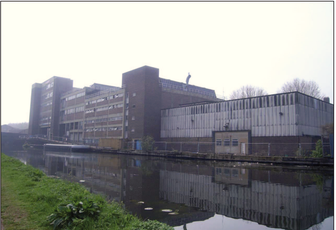
Plate 4: View of whole complex from north-east
