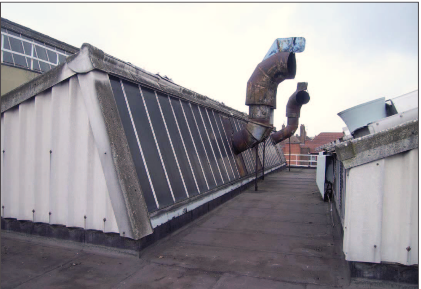
Plate 6: Roof lights above foundry showing extract ducts from zinc pots
