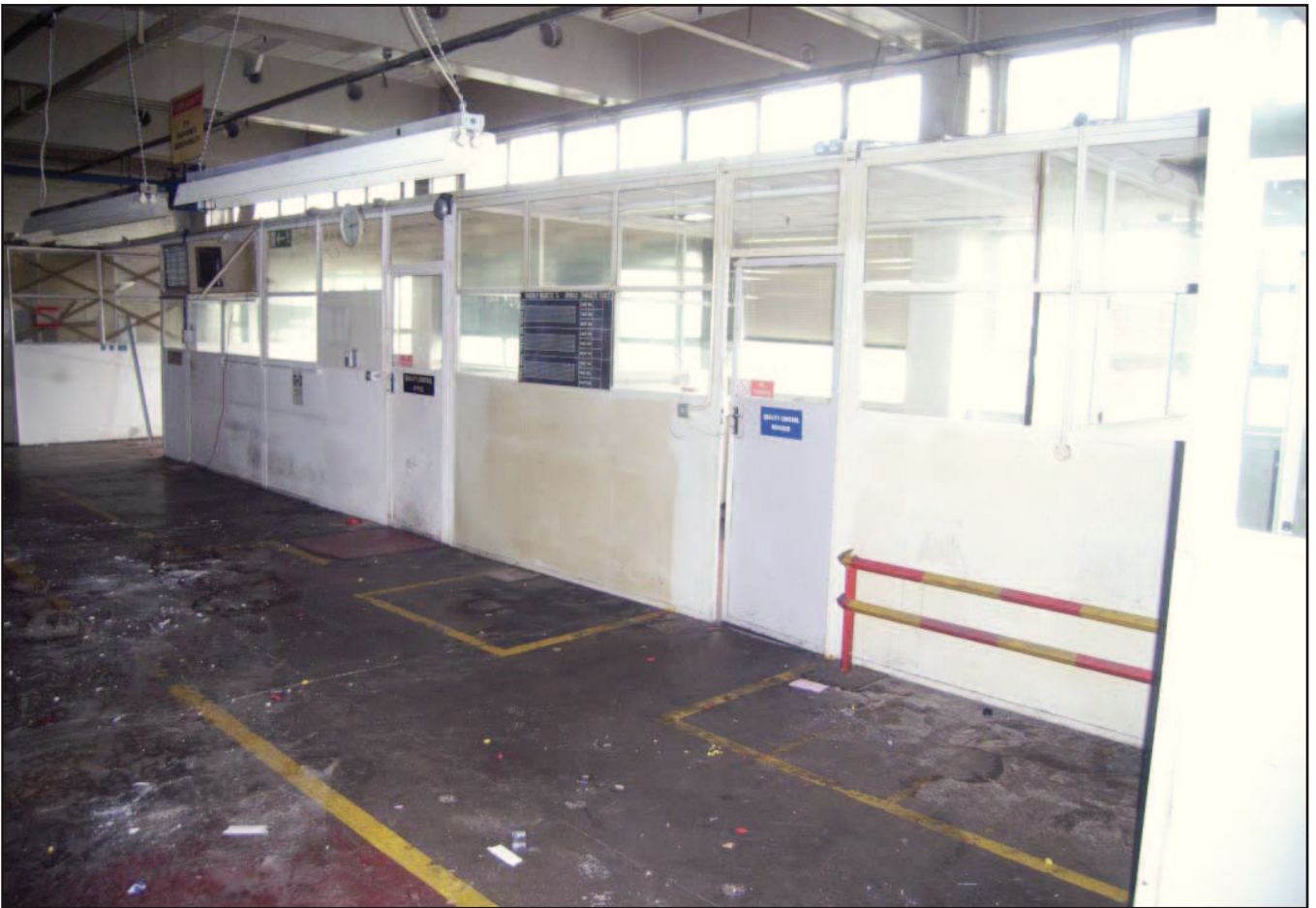
Plate 23: Offices at south end of Machining Dept (1st floor Block A)
