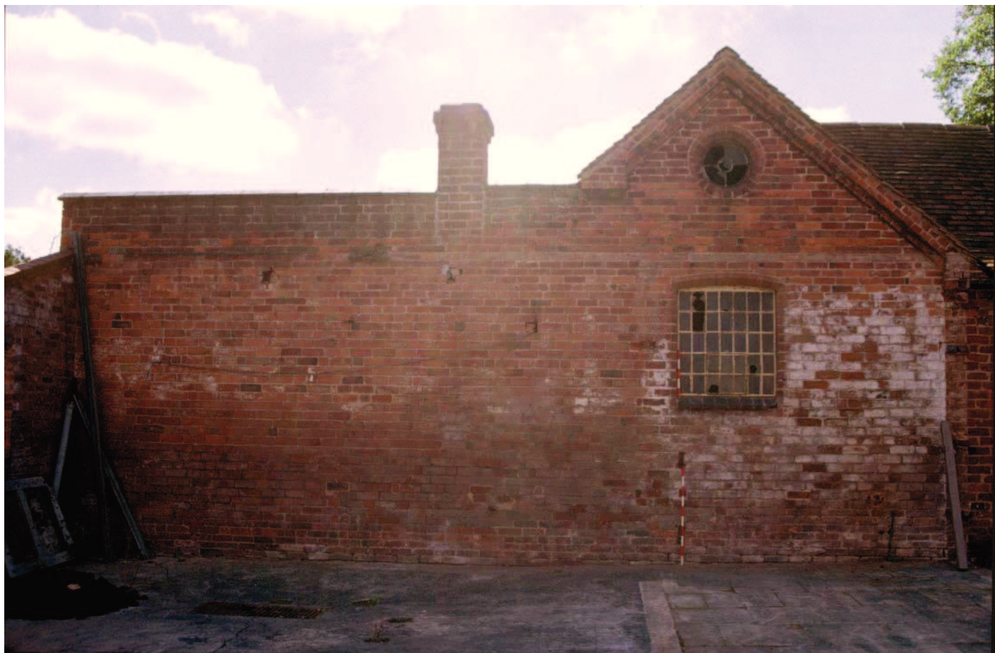
Plate 5: Park Attwood Farm, north elevation - amended gable height to accommodate high wall of extension (01/03)
