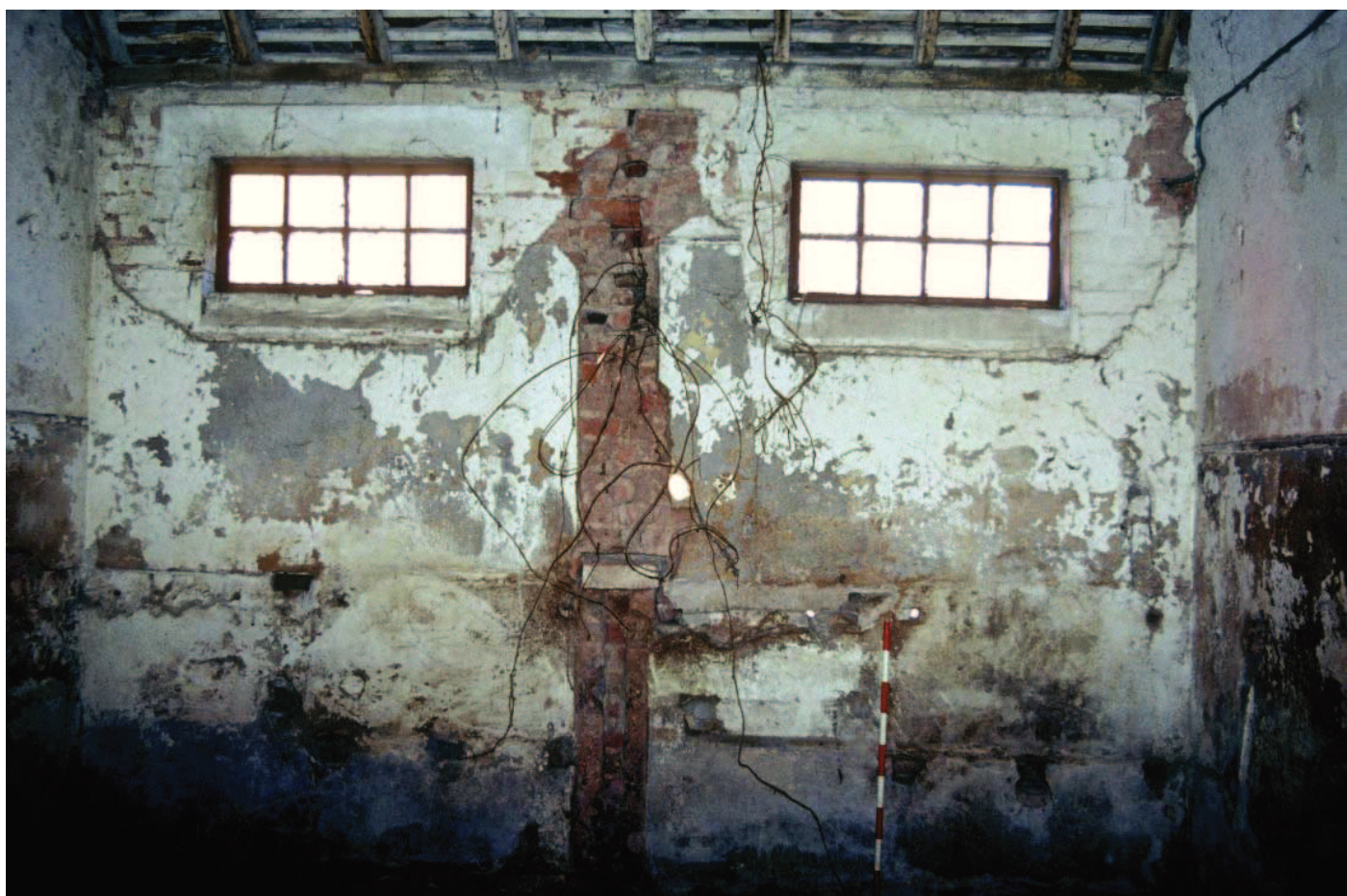
Plate 12: Park Attwood Farm, interior of Room 2 - location of stalls and manger fixtures (02/19)
