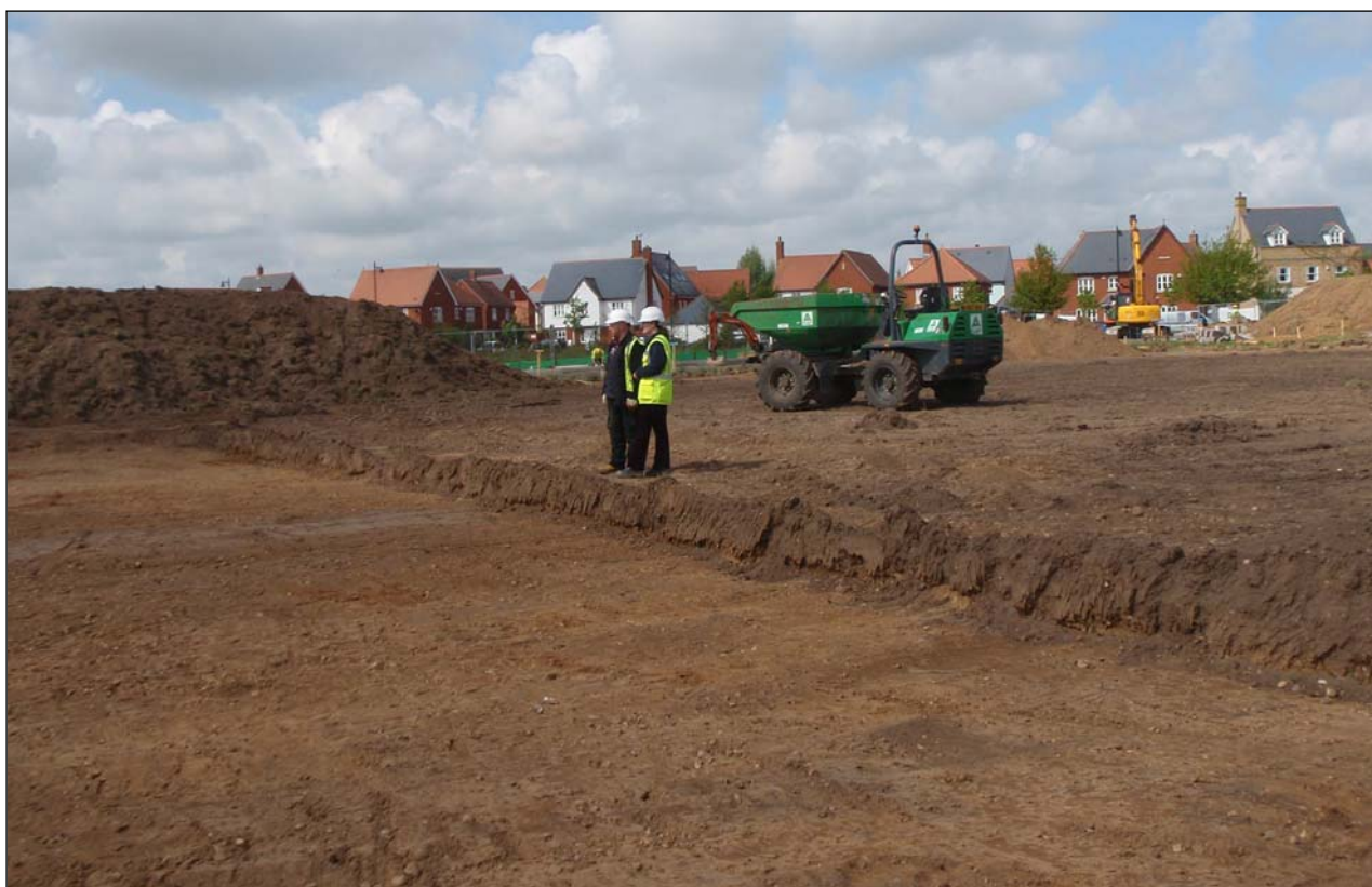
Plate 1: Site shot during machine stripping. Site 1a in the background. View from the east
