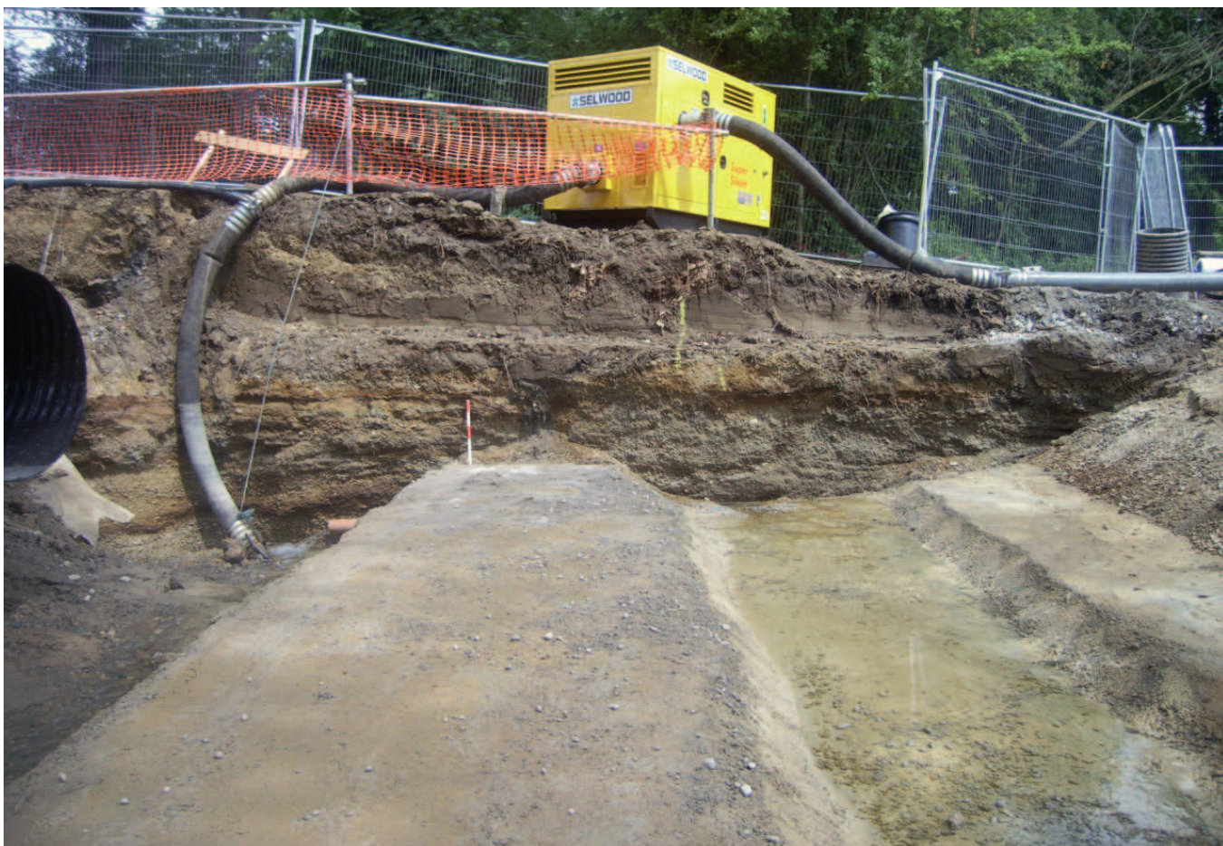
Plate 4: Culvert 2: south part of section, looking north-east
