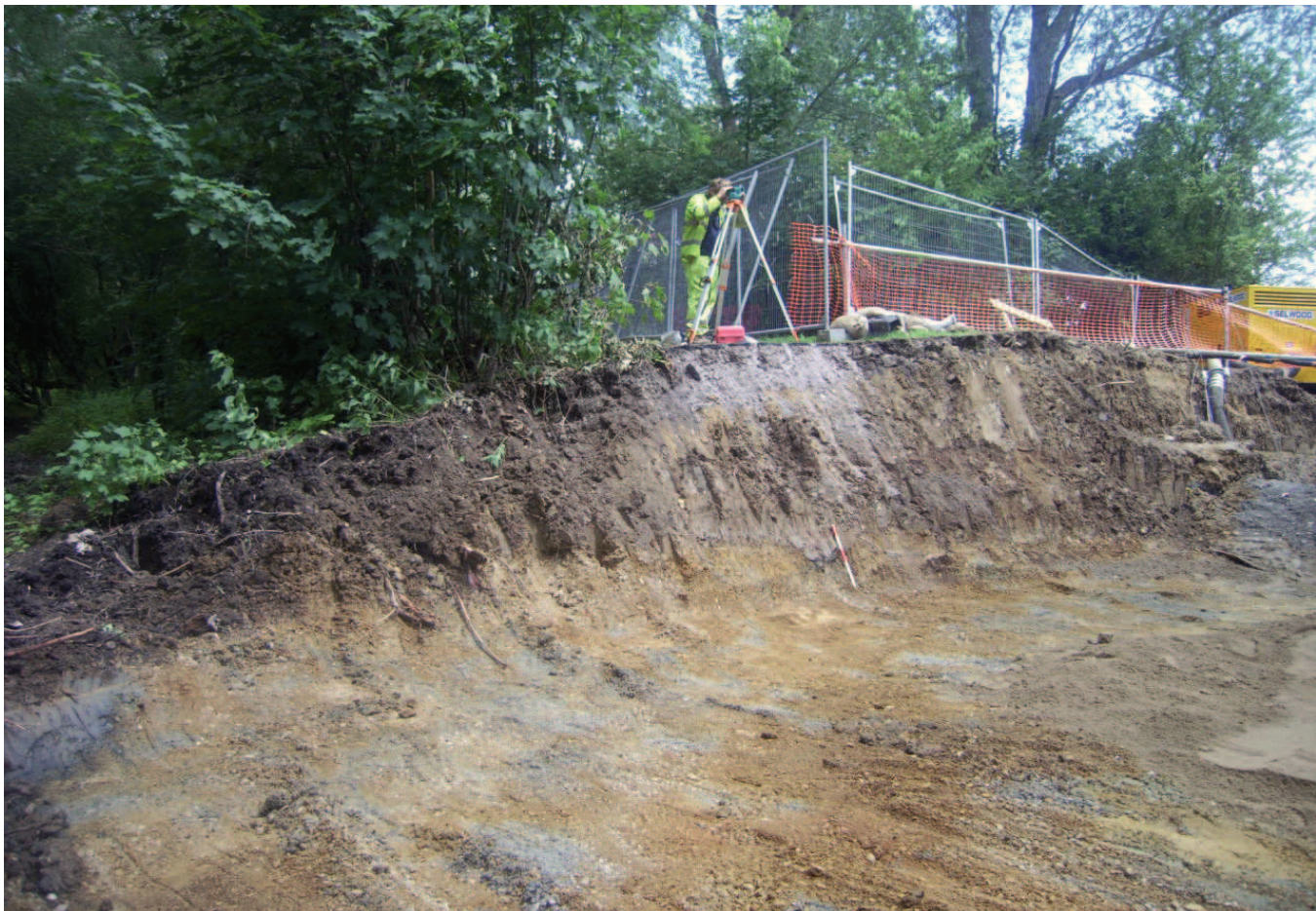
Plate 3: Culvert 2: north part of section, looking east
