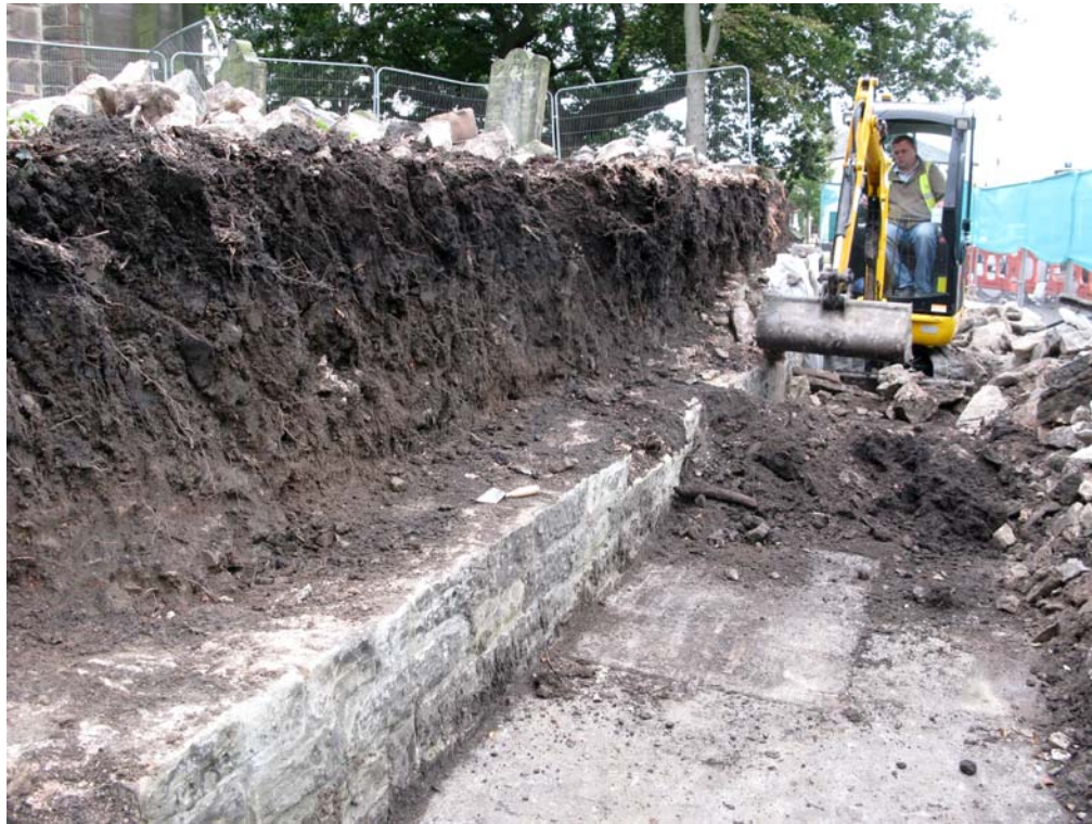
Plate 3: Excavation using a mechanical excavator
