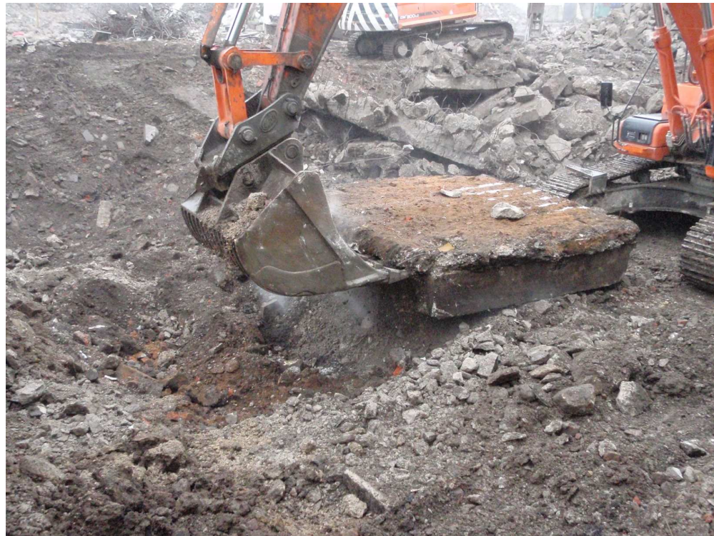
Plate 2: Removal of one of the foundation pads
