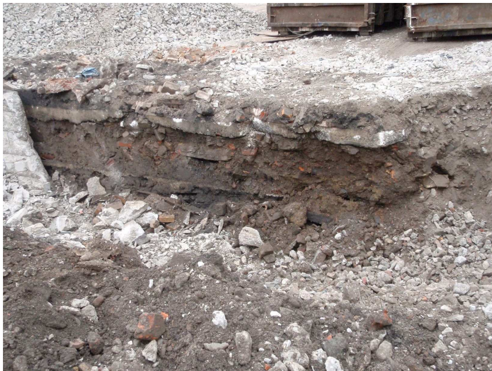
Plate1: Section through the demolition rubble under the concrete floor slab
