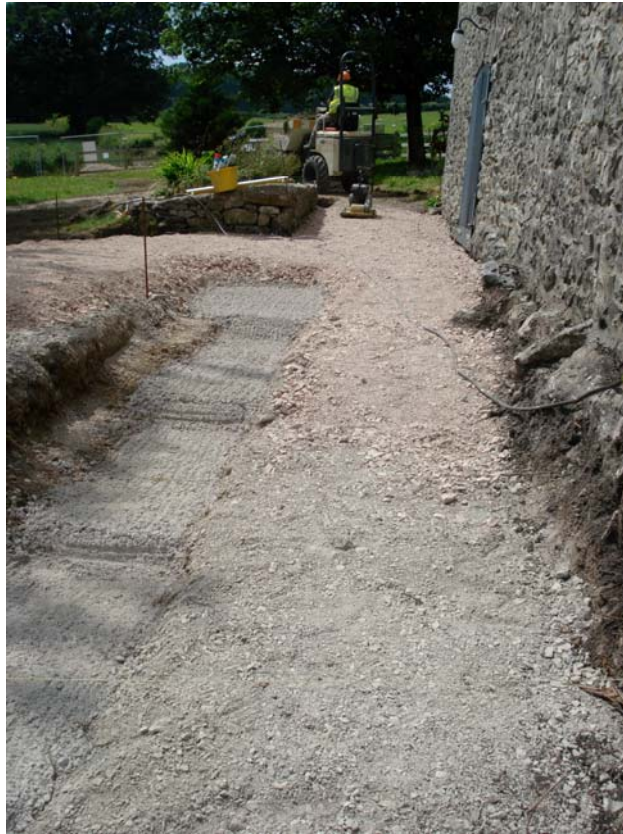
Plate 5: New path alongside south-east wall of the barn, looking west
