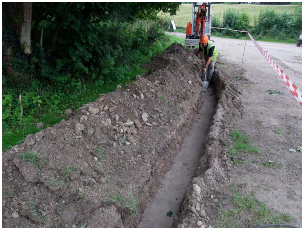
Plate 7: Cable trench excavation on the south side of the car park to the east of the barn, looking west
