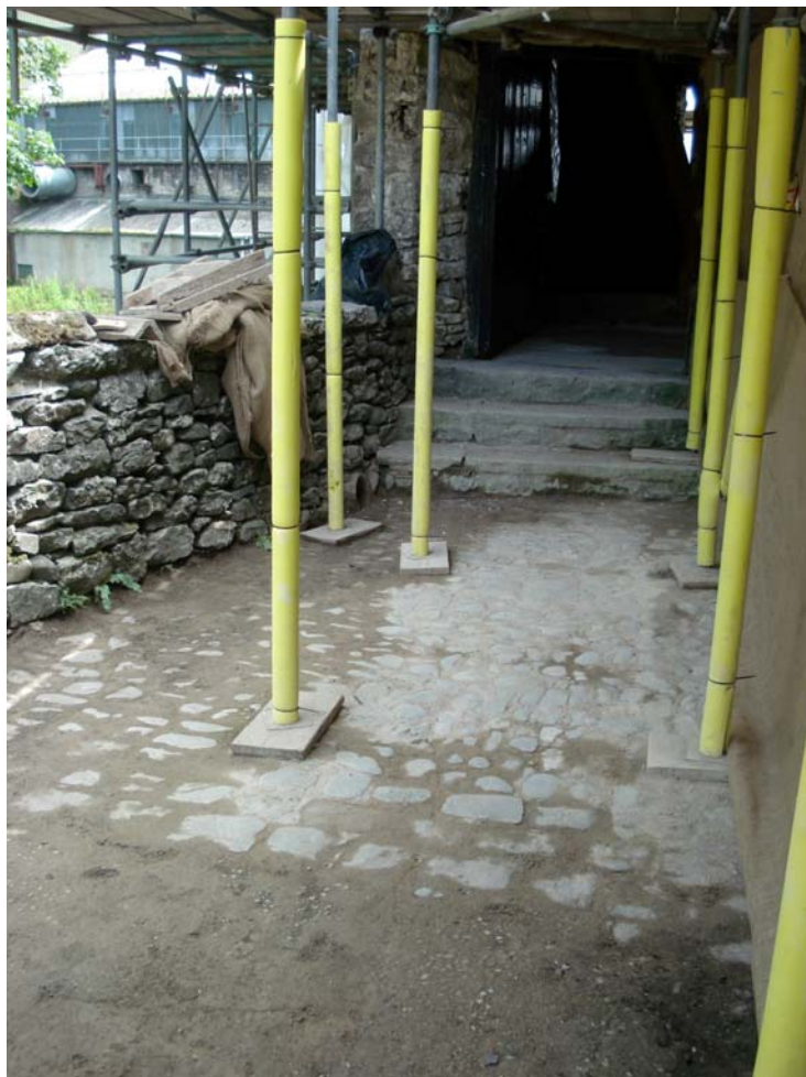
Plate 2: Path to north-east of mill, looking south-east
