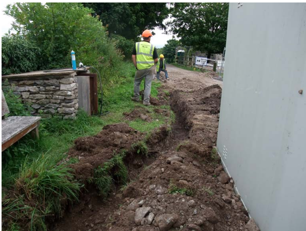
Plate 9: Cable trench at the north edge of the site, looking east
