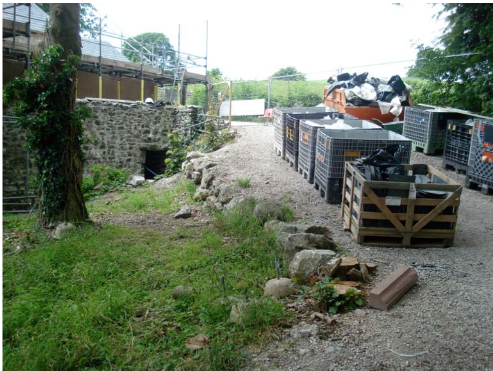
Plate 1: Path to be re-laid on the east side of the mill, looking west
