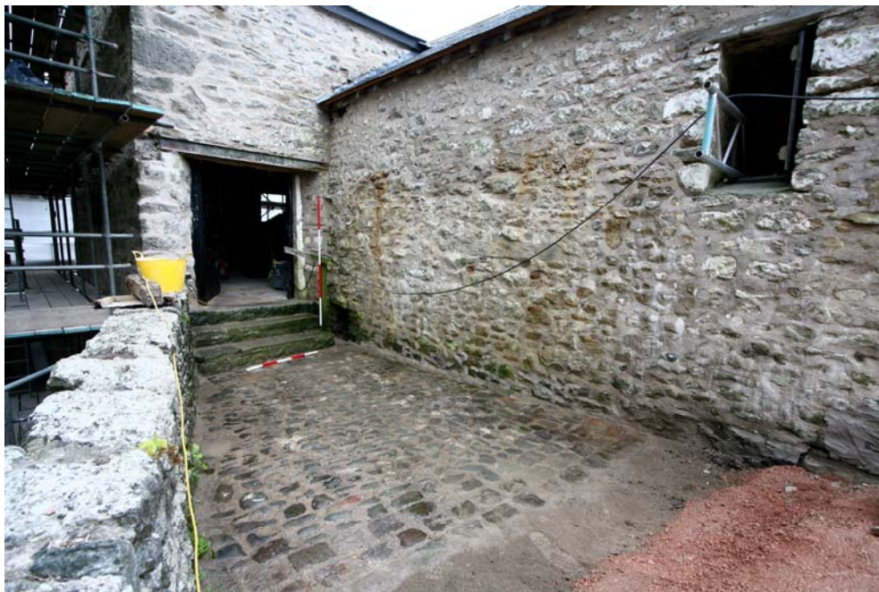
Plate 10: Cobbled area at the north-east side of the mill, looking south
