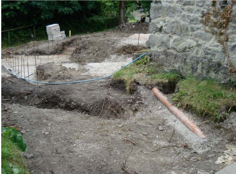
Plate 4: Excavations to the north-east of the barn, showing modern pipe, looking south
