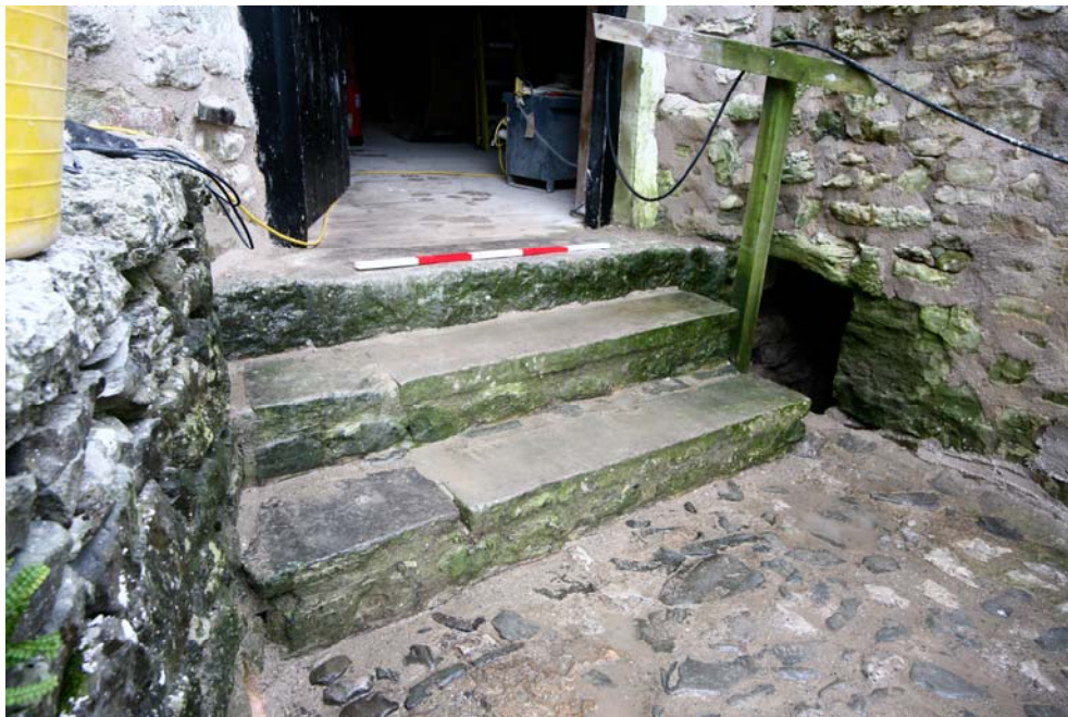
Plate 12: Steps leading to the mill door on the north-east side, looking south
