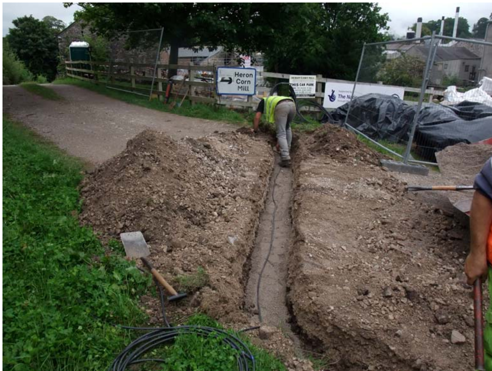
Plate 8: Cable trench excavation on the north side of the car park, looking east
