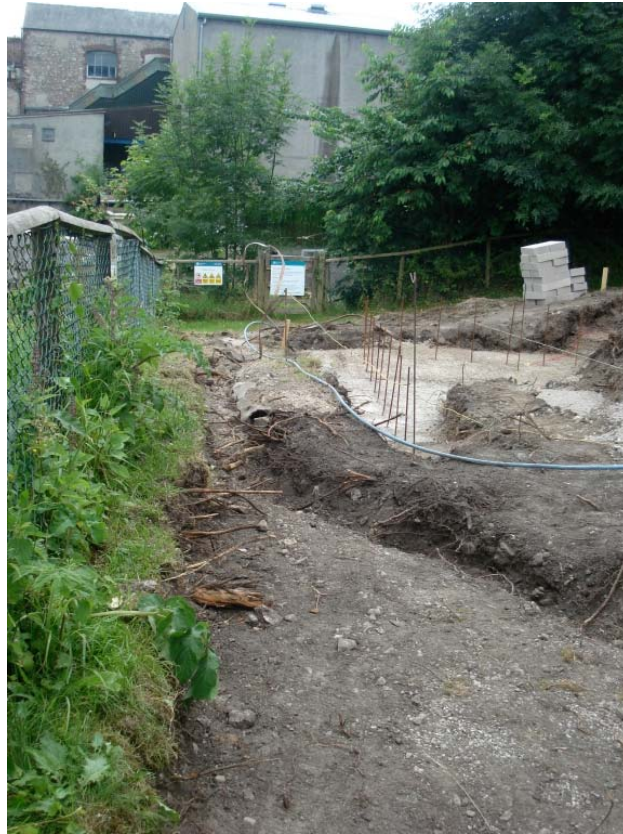
Plate 3: Excavations to the north-east of the barn, looking south
