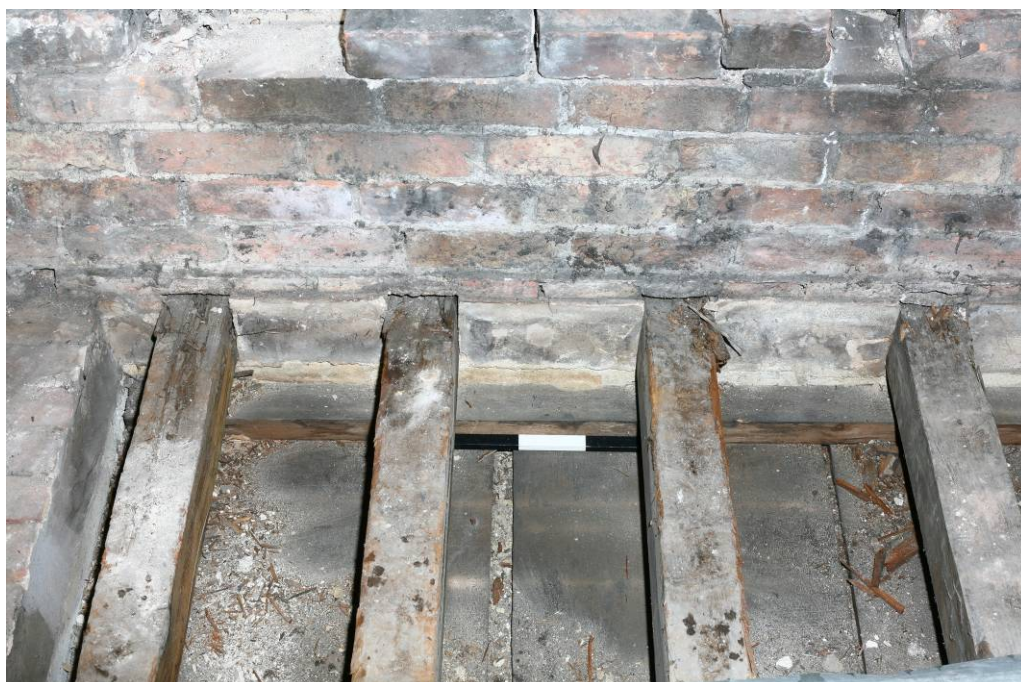
Plate 9: Plaster in-between the decorative beams at the base of the eastern section of wall indicating a former ceiling
