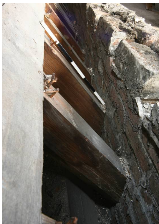
Plate 10: Rear of the wall showing the rafters entering the wall
