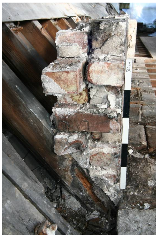
Plate 11: Relationship between the brick wall and rafter
