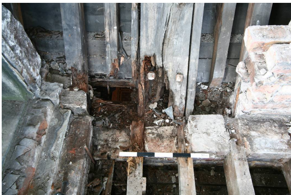
Plate 3: West end of the wall showing rotted rafters and low wall below floor level
