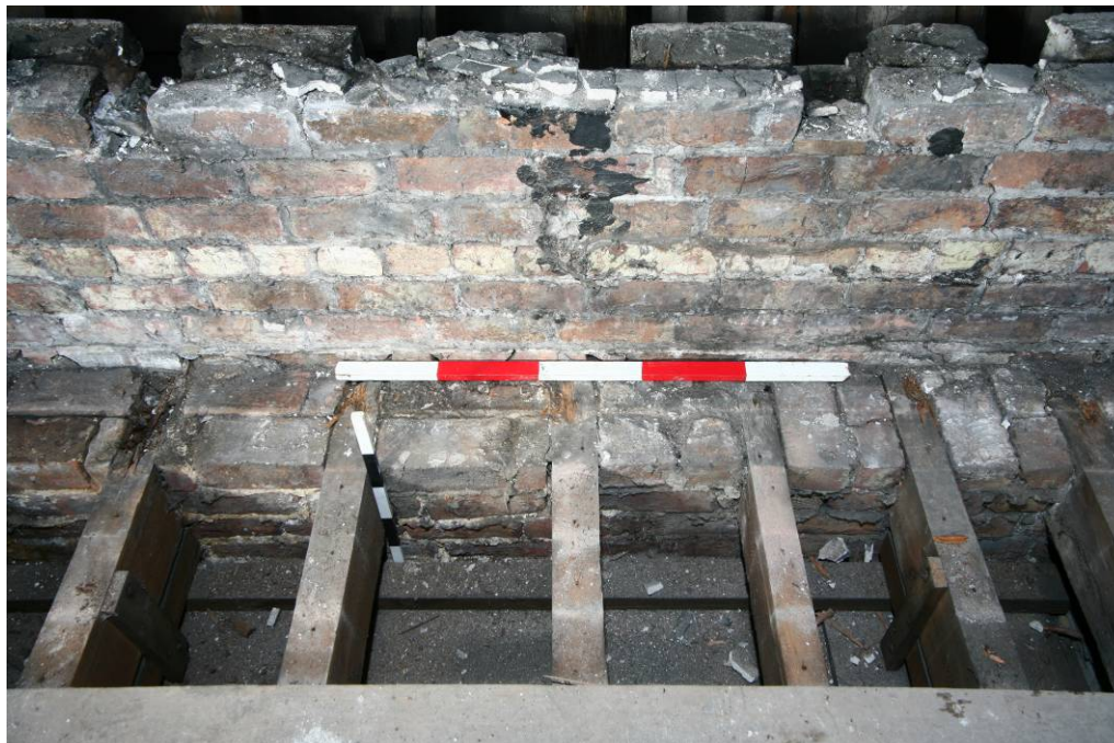
Plate 8: Low section of wall showing how the joists are fitted
