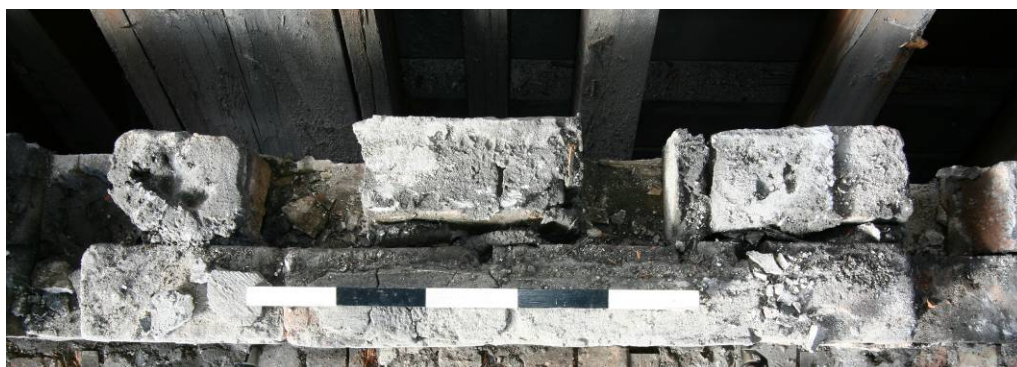
Plate 7: Gaps in the wall for the spurs forming the support structure of the lead lined gutter/channel
