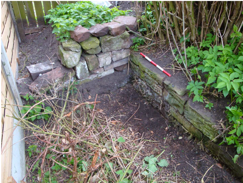
Plate 4: Stone walls, in north-east of application area – reused masonry from early post medieval building?
