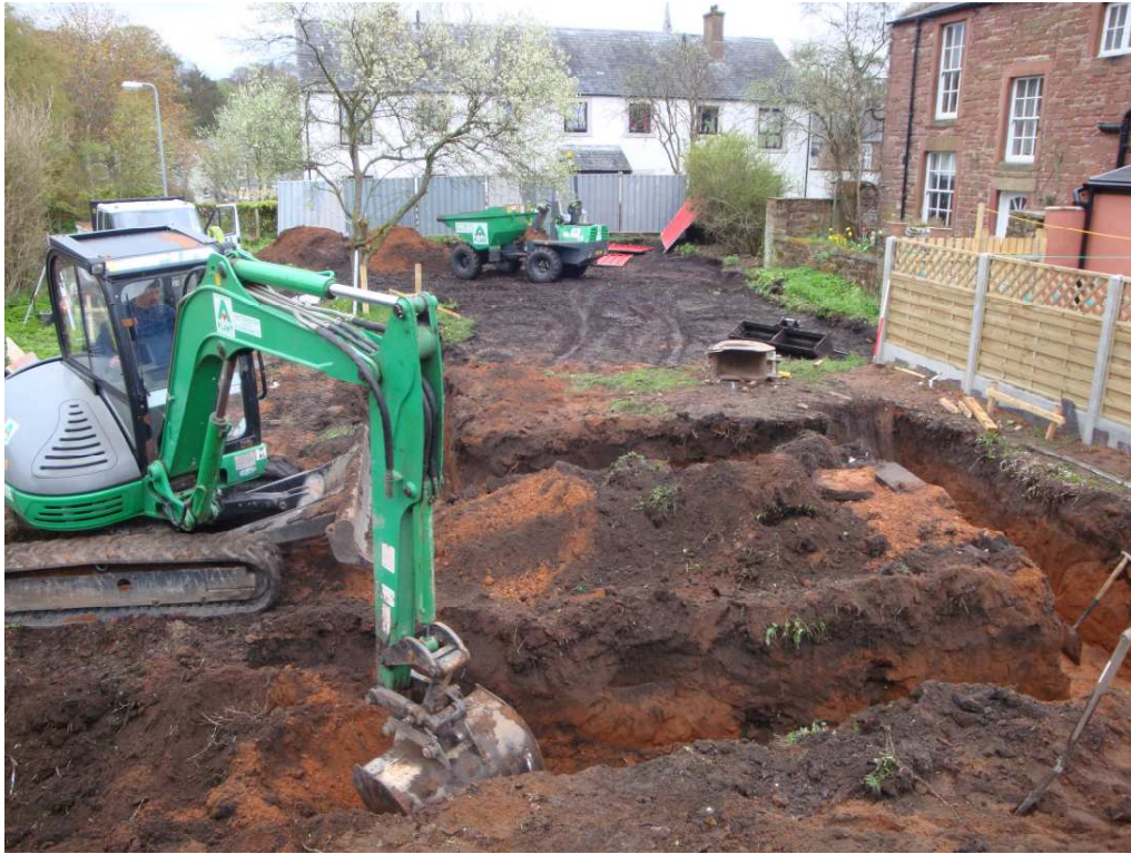
Plate 3: Continuation of foundation trench
