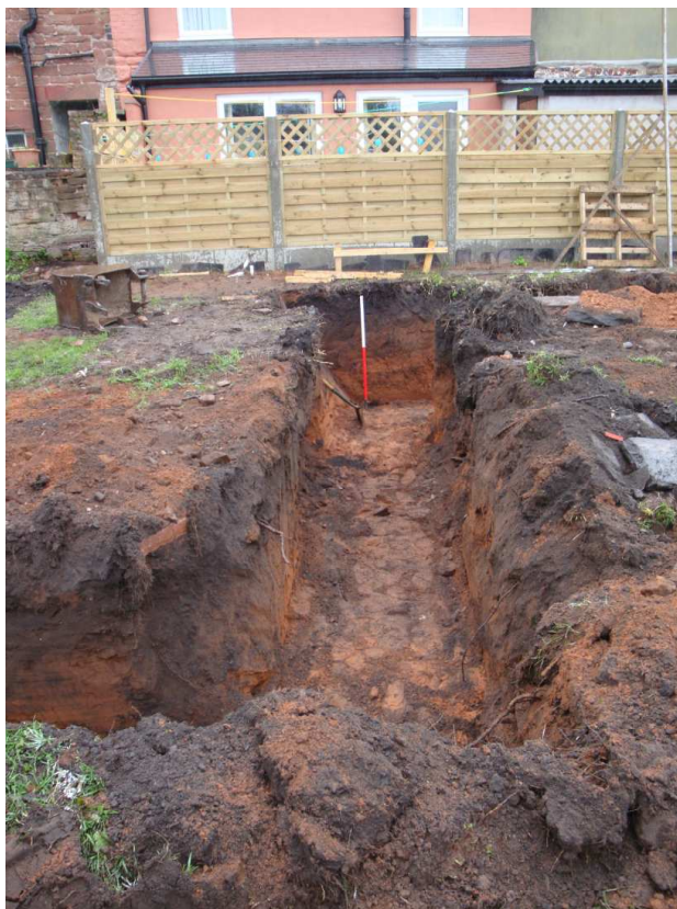
Plate 2: Section of the foundation trench at the northern end of the plot
