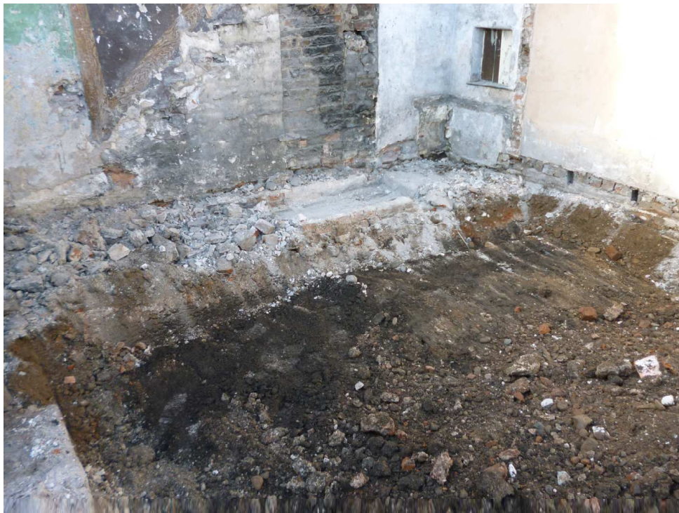
Plate 2: the excavated trench, through the centre of the site, showing the buried soil horizon
