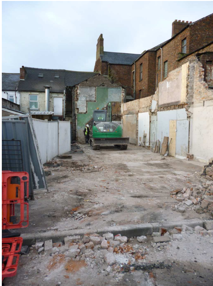
Plate 1: the development area before the start of groundworks
