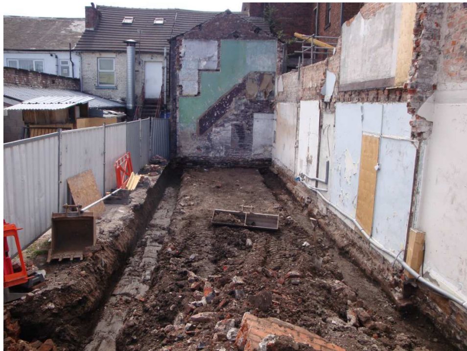
Plate 4: the fully excavated foundation trench
