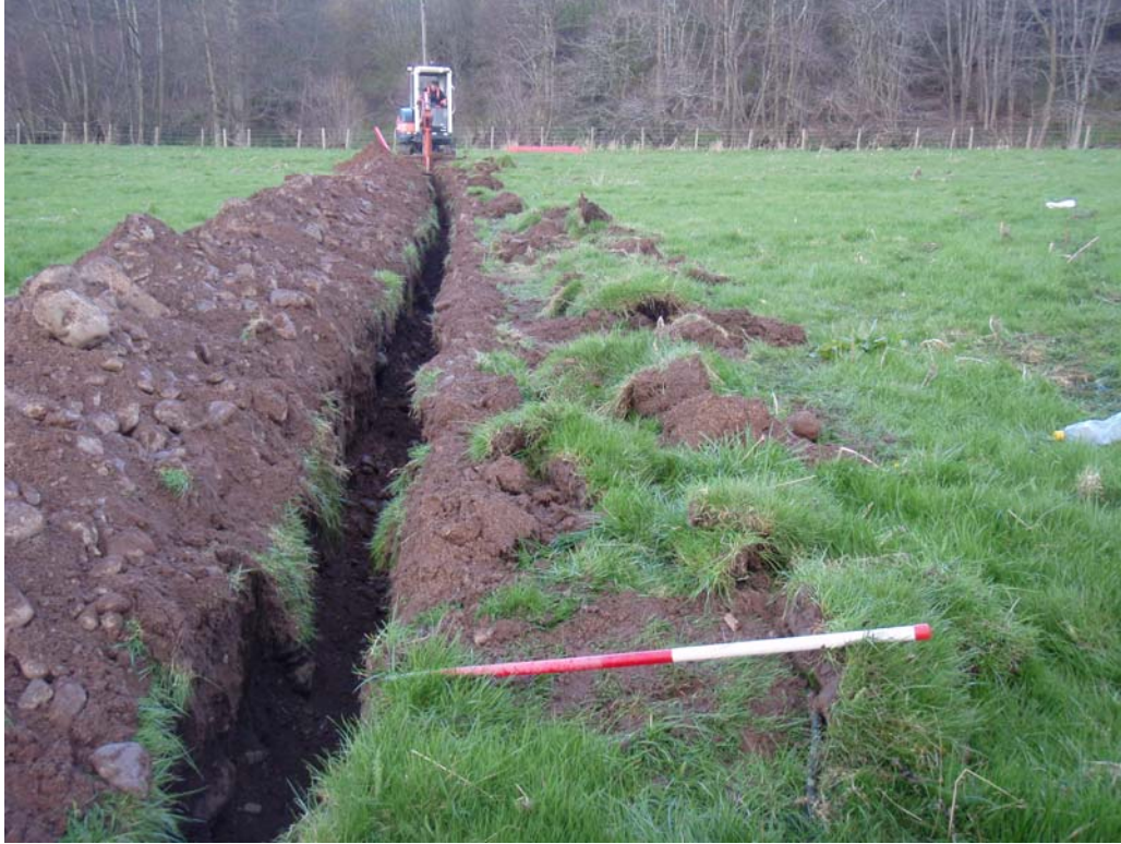
Plate 3: Excavation of cable trench recorded during the watching brief
