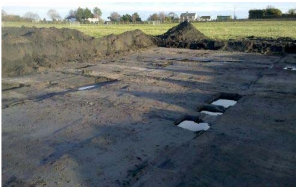
Plate 29: Overall, post-excitation view of Trench 16 Extension, looking east
