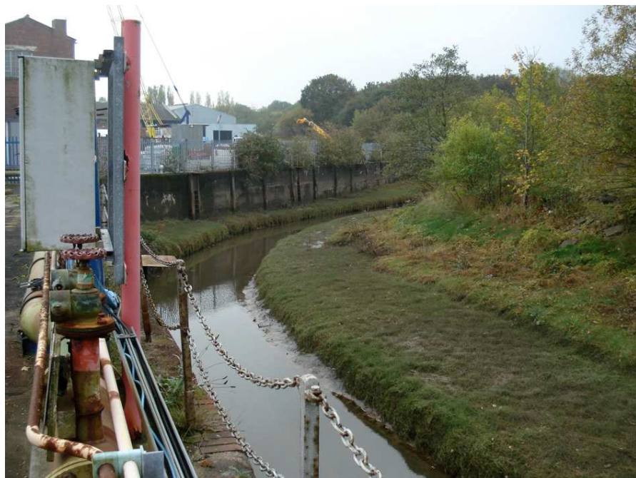
Plate 12: Sea wall (Site 31), looking south-east
