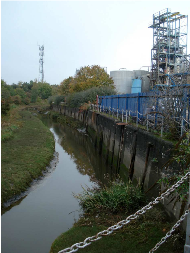
Plate 11: Sea wall (Site 31), looking north-west
