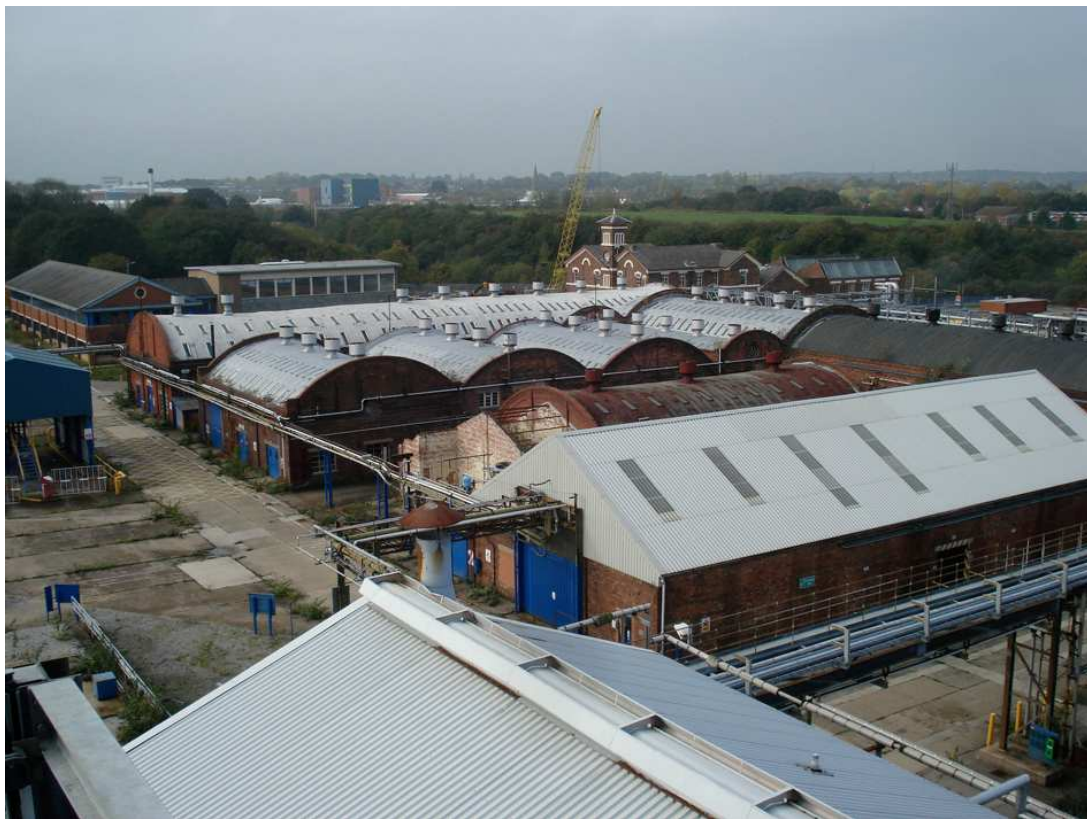
Plate 20: General view across site to the listed building (LB no 215551), looking west
