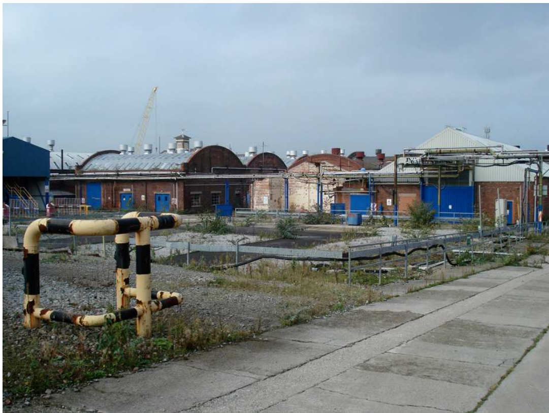
Plate 18: General view from eastern extent of site, looking north
