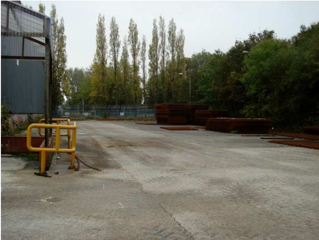
Plate 6: South-west boundary of the proposed development area, looking south-east
