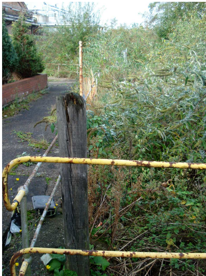
Plate 16: Timber bollard on former edge of sea wall (Site 31), looking west
