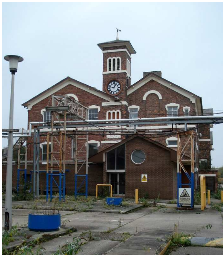
Plate 9: Listed building (LB no 21551), looking north-west
