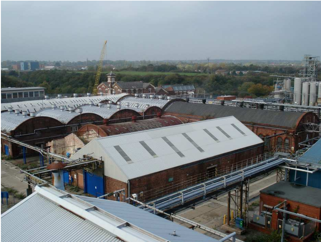
Plate 19: General view across site, looking north-west
