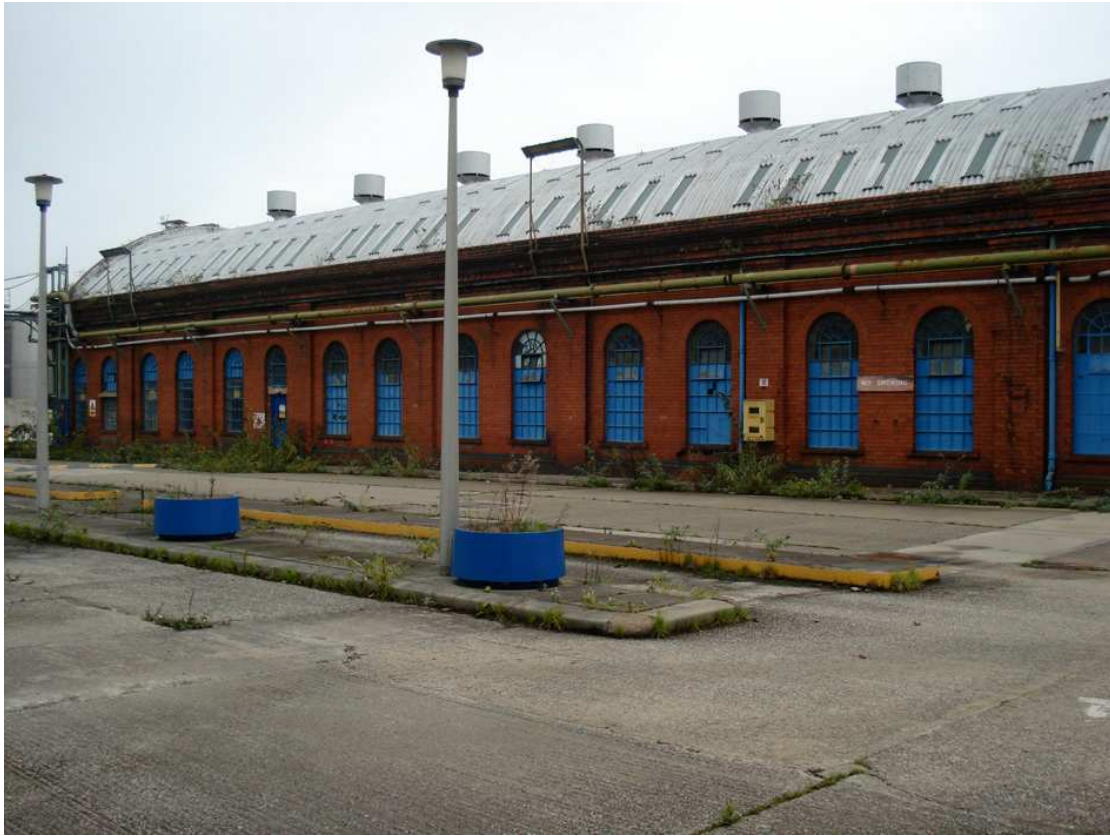
Plate 10: Late nineteenth century buildings, looking north
