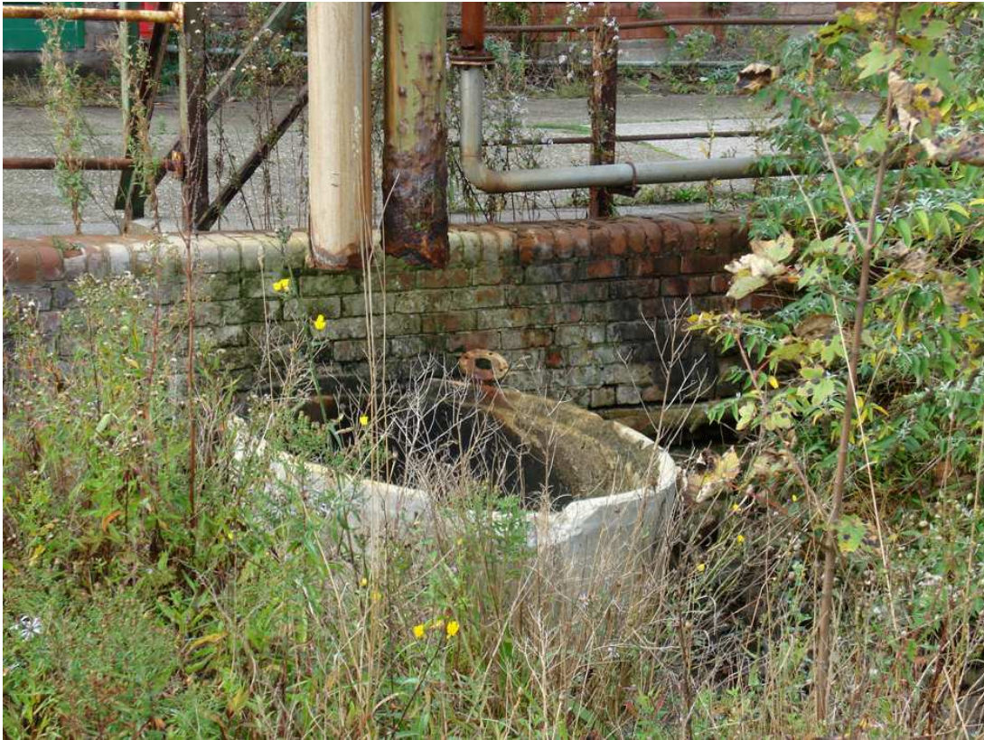
Plate 13: Remains of brick sea wall (Site 31), looking south
