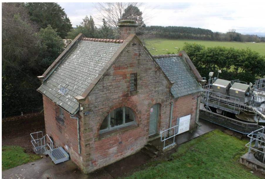
Plate 1: General view of the admin building facing south-west
