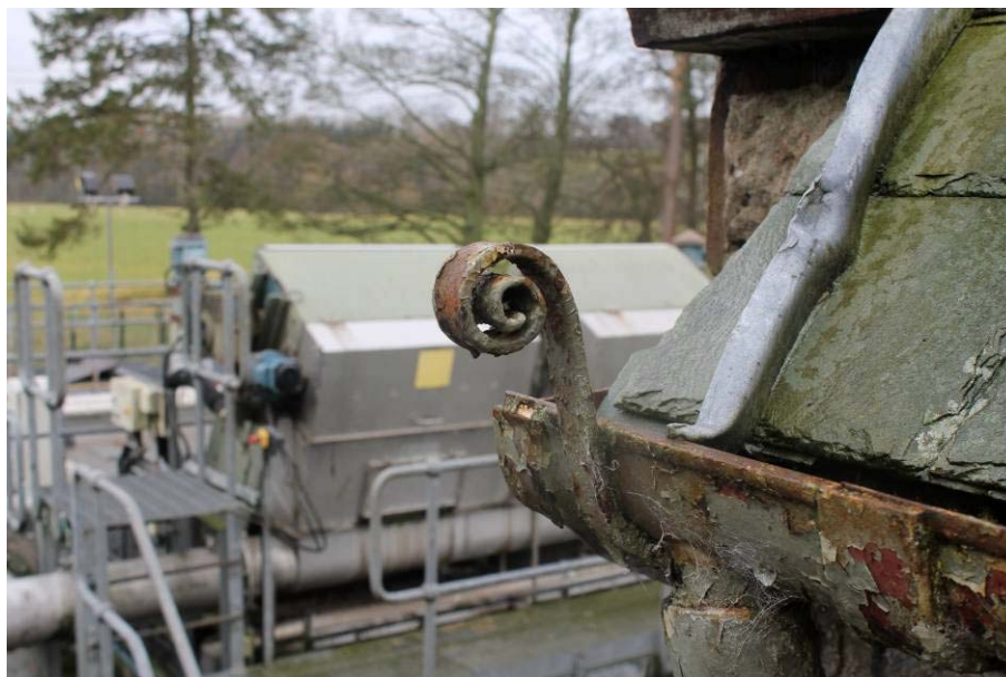
Plate 8: Detail view of a wrought iron scroll attached to the cast iron gutter on the west-side of the south-facing elevation.
