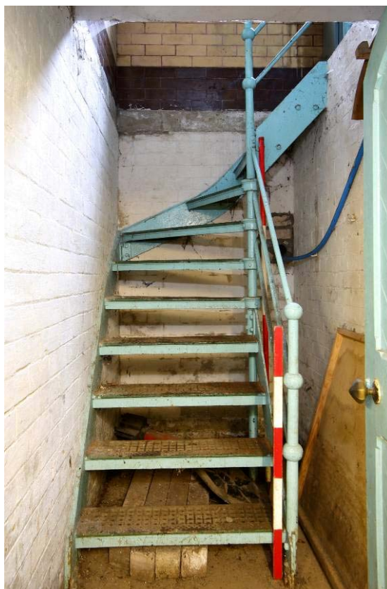
Plate 9: General appearance of the staircase.
