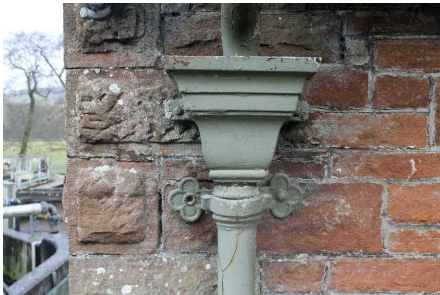
Plate 7: Detail view of the hopper and decorative brackets on the west side of the south-facing elevation
