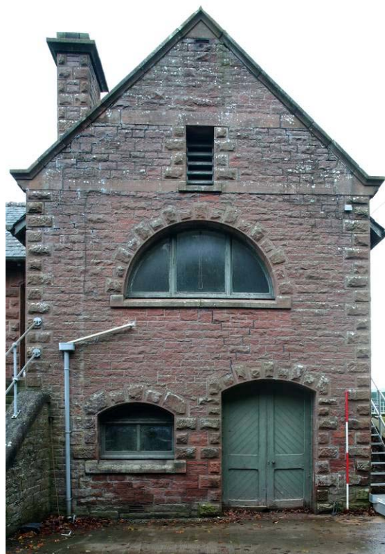
Plate 5: The south-facing elevation facing north
