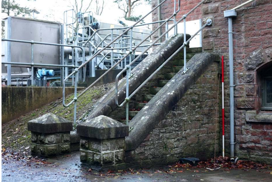
Plate 6: View of the flight of steps leading to the west part of the south-facing elevation
