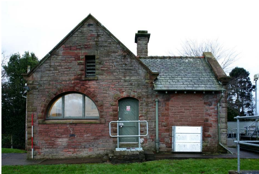
Plate 4: The north-facing elevation facing south
