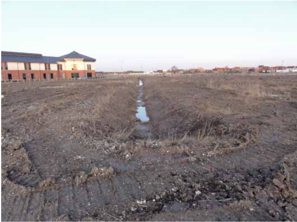
Plate 13: A pipe trench dug through the northern portion of the site
