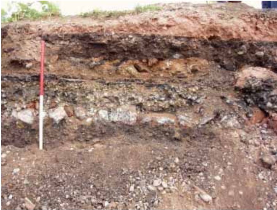
Plate 7: Former road surface 1002 beneath the present surface 1014
