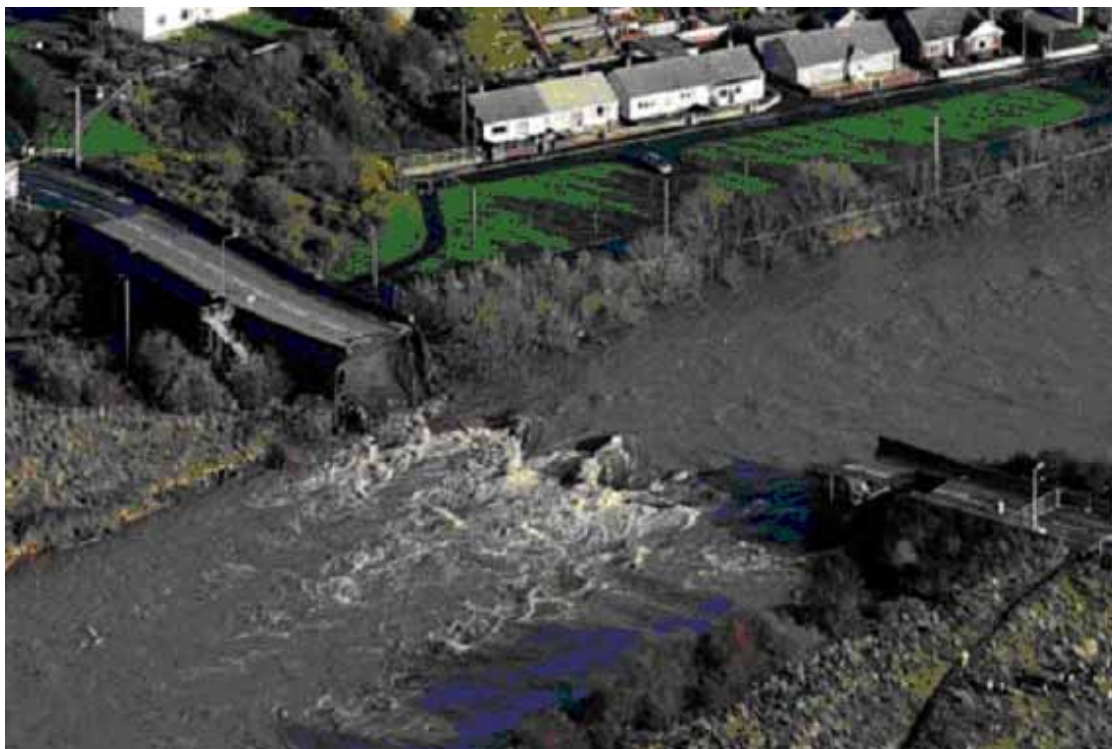
Plate 2: View of Northside Bridge following its collapse in November 2009
