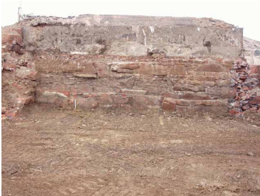
Plate 5: The south-facing concrete slab 1004 and inner wall 1016
