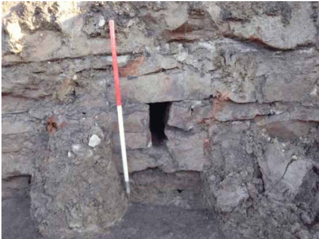
Plate 3: Drain 1024 in wall 1016 and construction cut 1050
