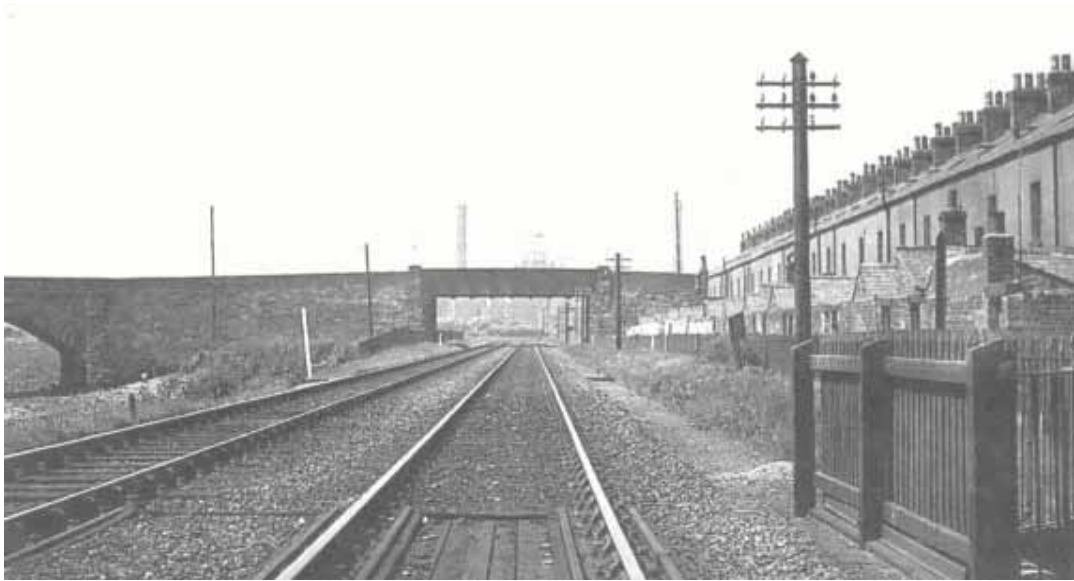
Plate 1: View of Northside Bridge looking west
