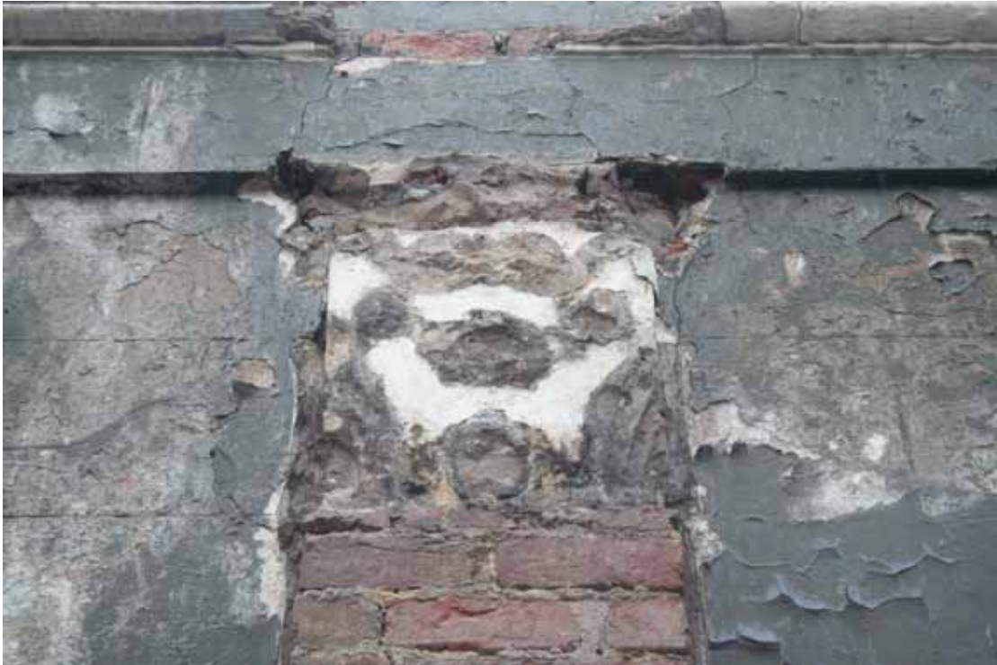
Plate 27: Close up of brick pilaster showing surrounding stucco and remnants of plaster capital
