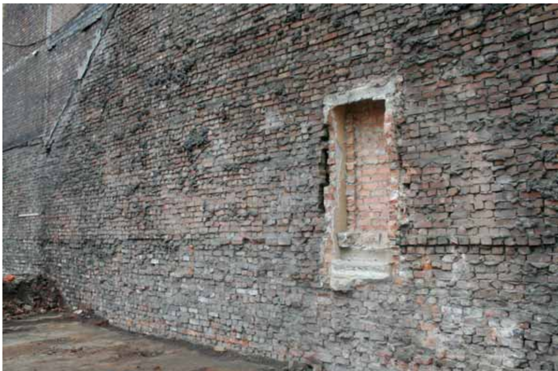
Plate 32: Blocked doorway and steps in the north-facing elevation of 13 Hope Street
