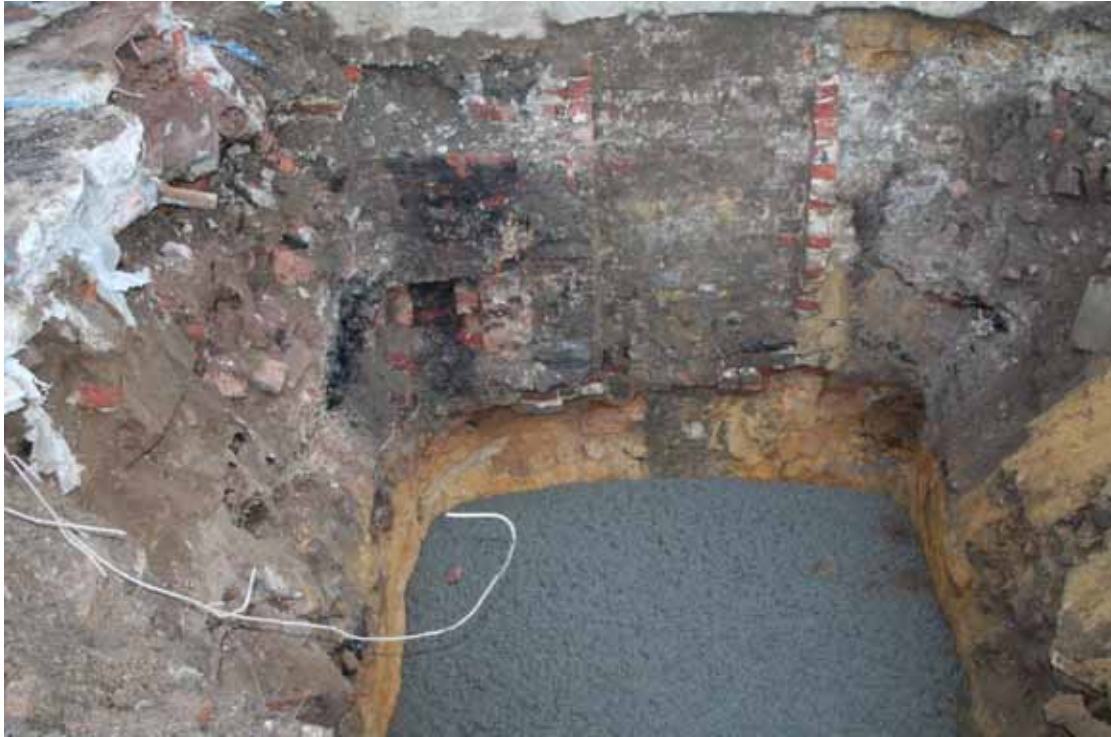
Plate 41: Pad 10 (south-facing view) showing truncated cellar walls situated directly onto yellow sandstone bedrock
