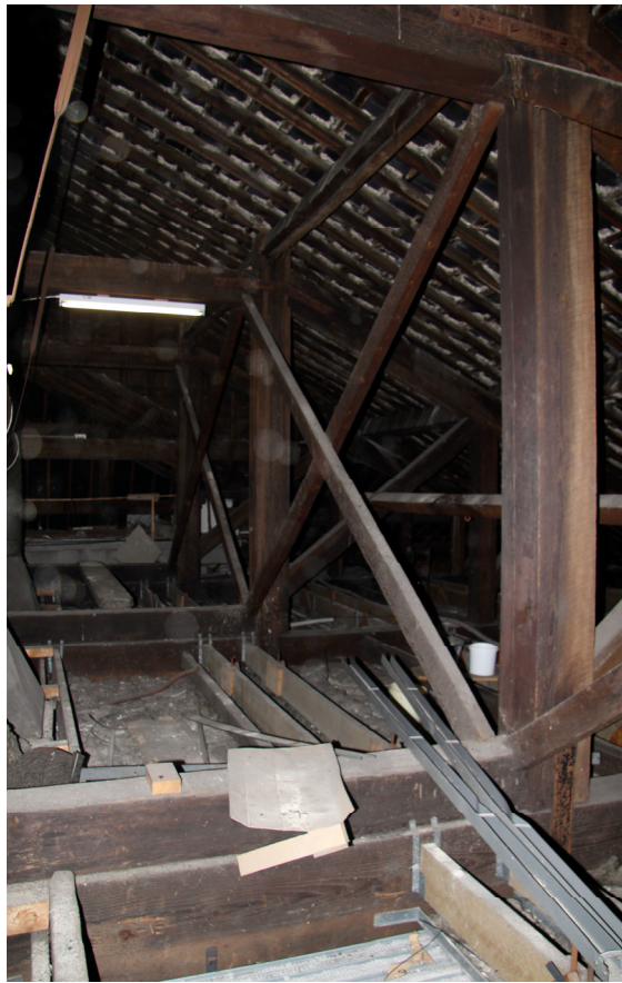
Plate 23: Central section of the Queen post truss
