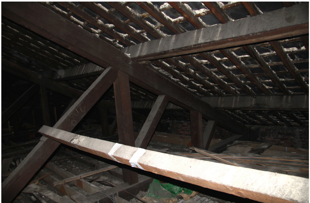
Plate 22: Part of the Queen truss in the Hope Hall roof space
