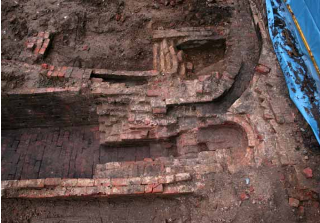
Plate 39: Southern end of Wagon Boiler base showing flues
