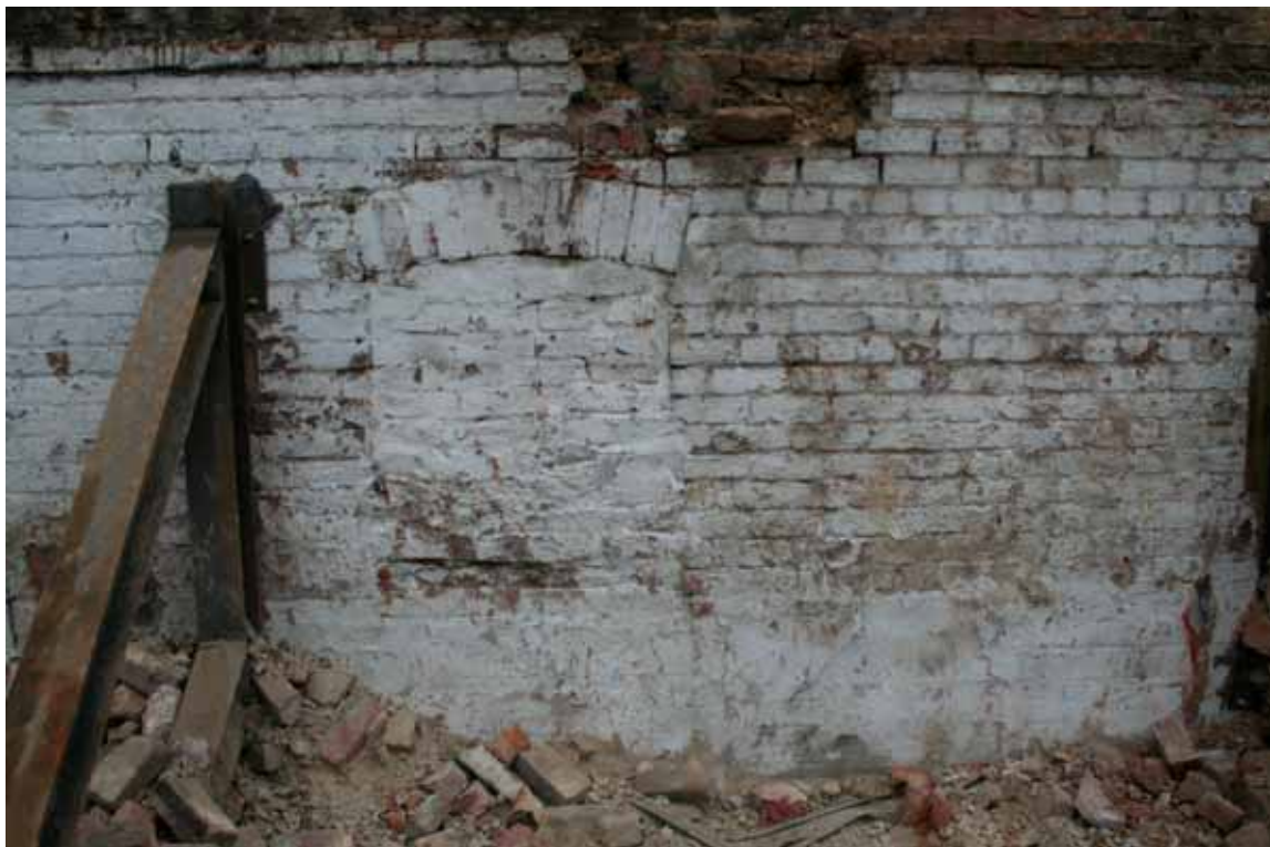
Plate 34: Blocked window with segmental brick arch in northern basement wall of 9 Hope Street
