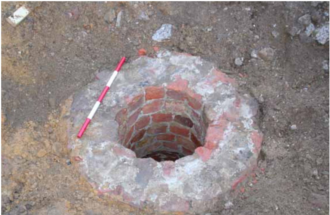
Plate 40: Narrow brick funnel well cap
