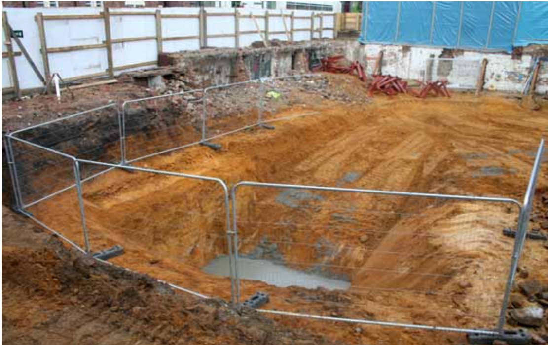
Plate 42: Section C showing the natural yellow sandstone bedrock
