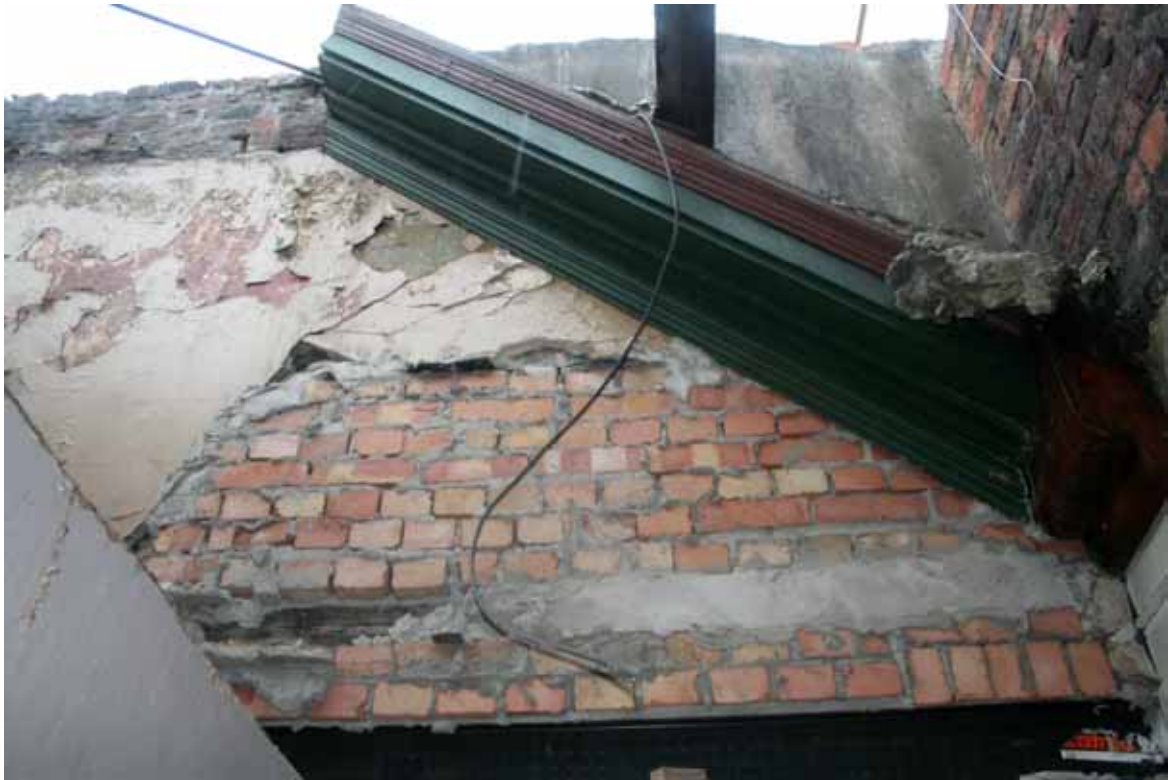
Plate 29: Timber gable frame with rounded corbel and bolection moulding
