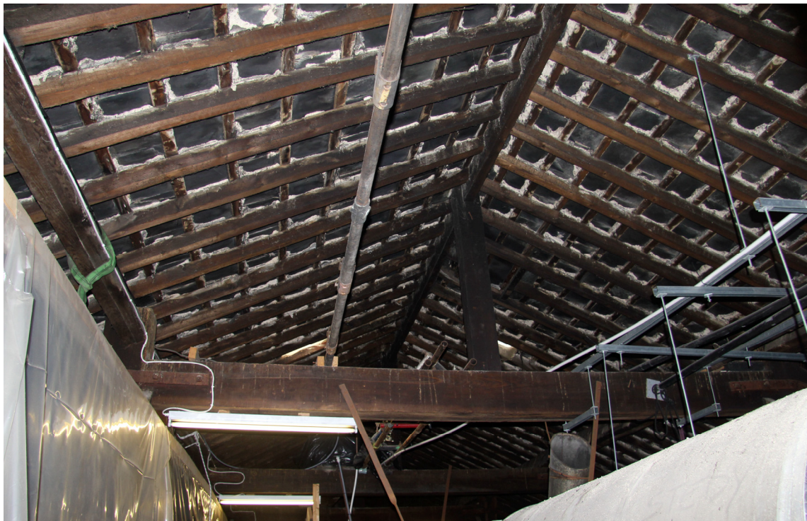
Plate 24: Central top post of the Queen post truss
