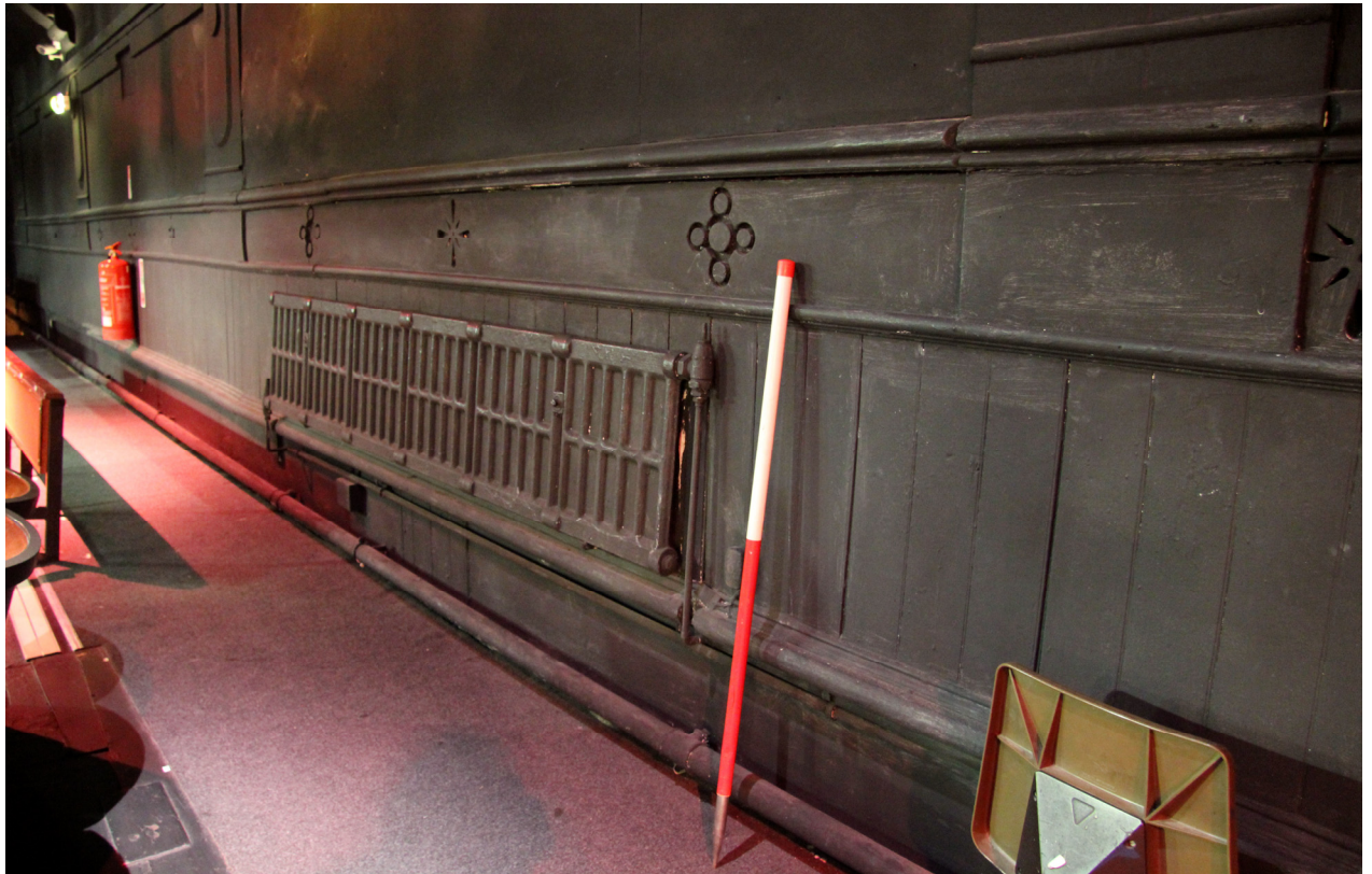
Plate 21: Early radiator on the south side of the auditorium (Room 67)
