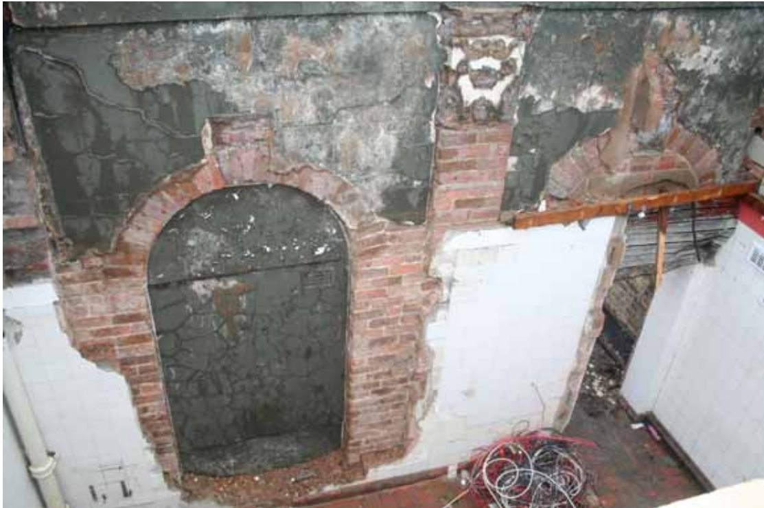
Plate 25: Southern bay of principal elevation, 9 Hope Street showing blocked windows and central pilaster
