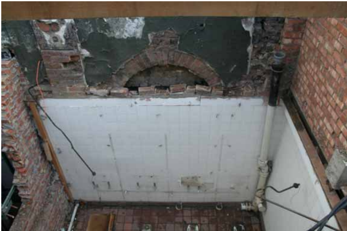
Plate 26: Northern bay of principal elevation showing blocked arched window and to the left, truncation by the insertion of modern lift shaft wall
