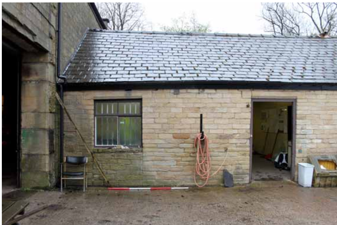
Plate 23: North-west external elevation of Building B
