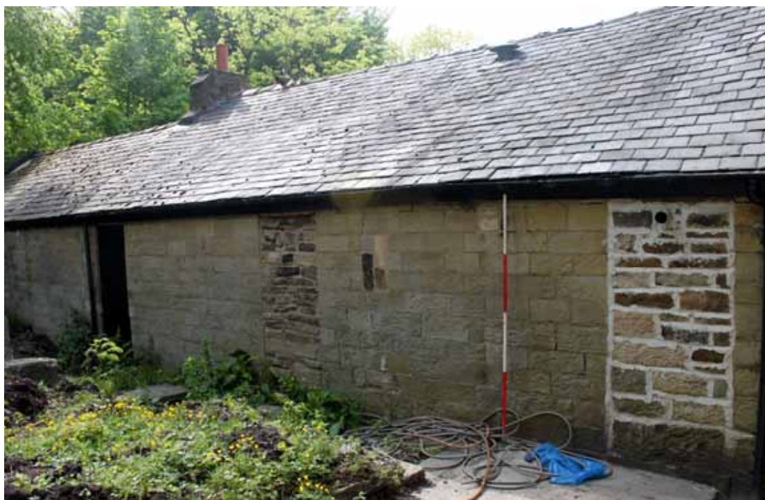
Plate 25: South-east elevation of buildings B and C
