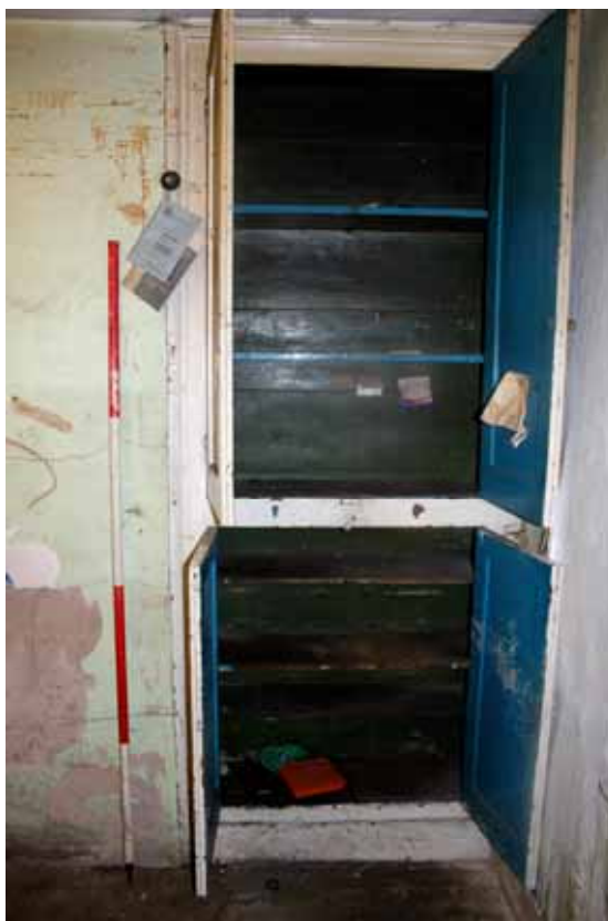
Plate 19: Cupboards in the north-west elevation of Room G3 of the cottage
