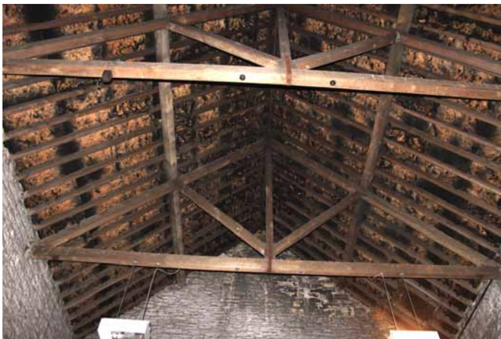
Plate 4: The barn roof structure
