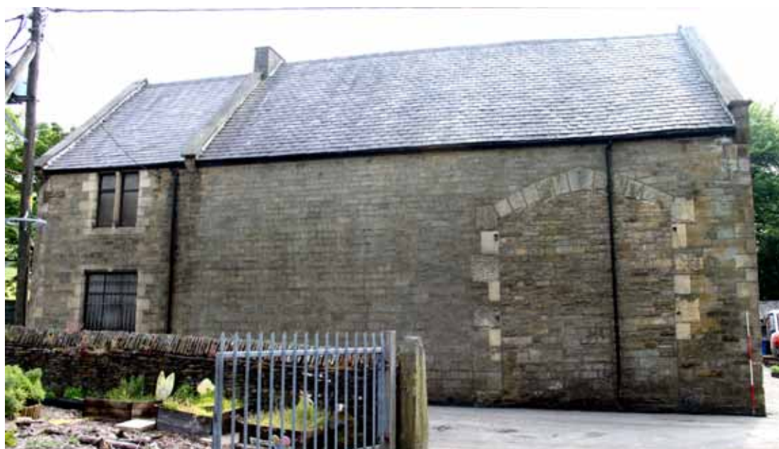
Plate 11: North-eastern elevation of Building A showing blocked coach doorway
