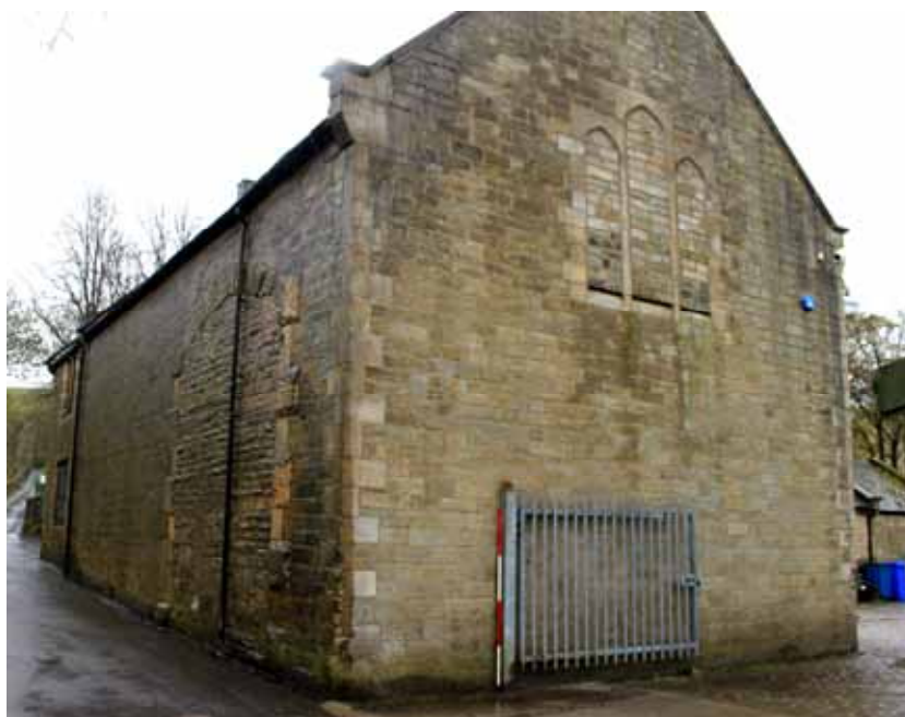
Plate 2: North-west gable elevation of the barn showing the blocked lancet window
