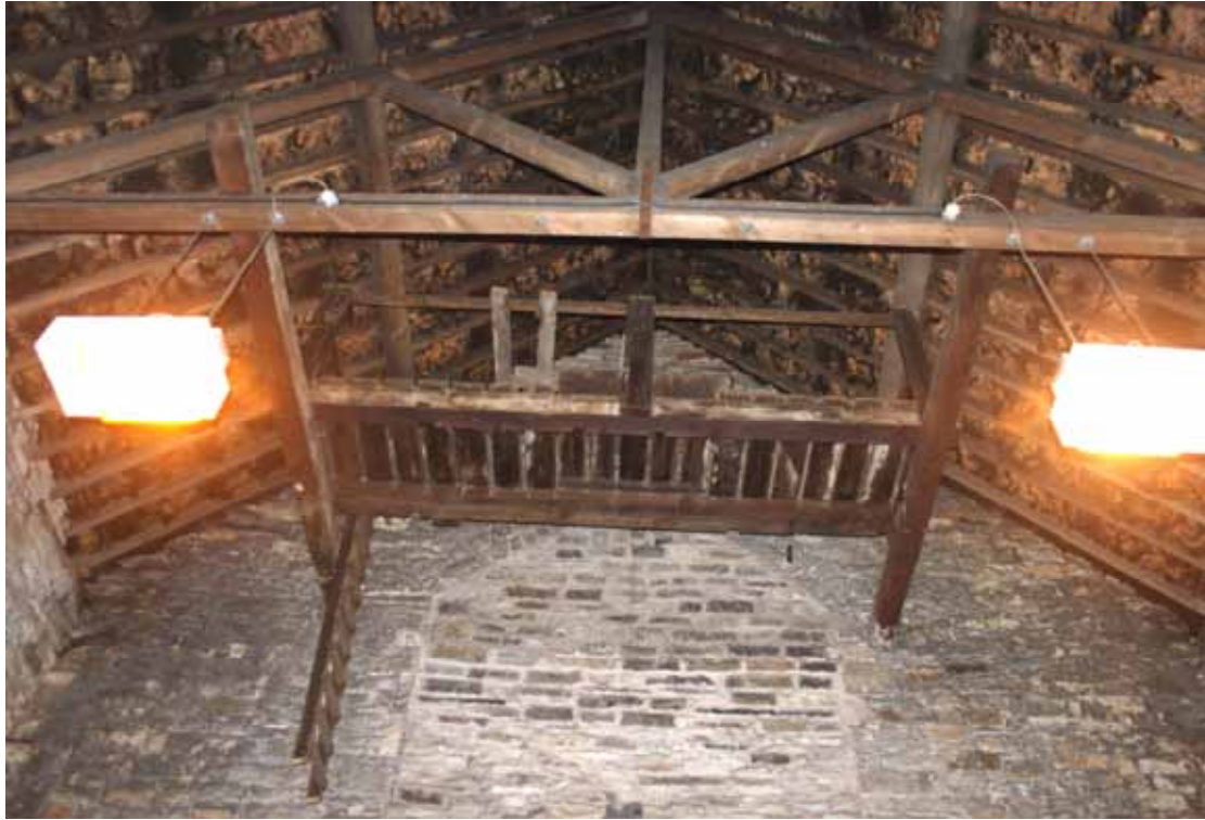
Plate 17: Wooden gantry set into the roof space of the north-western end of the barn
