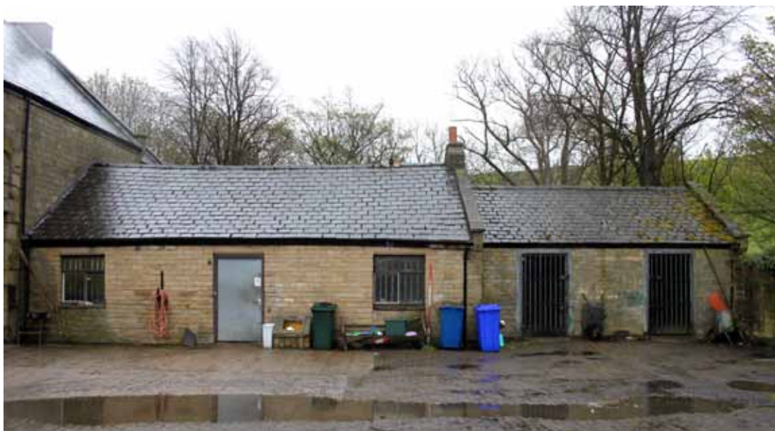
Plate 9: North-west elevation of Buildings B and C
