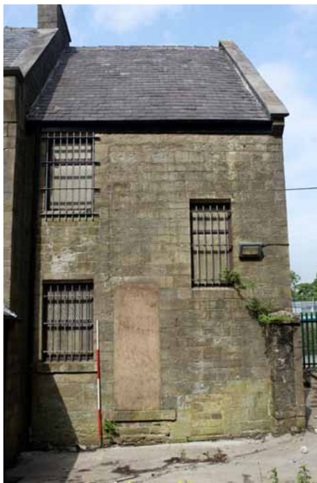
Plate 6: South-western elevation of the cottage
