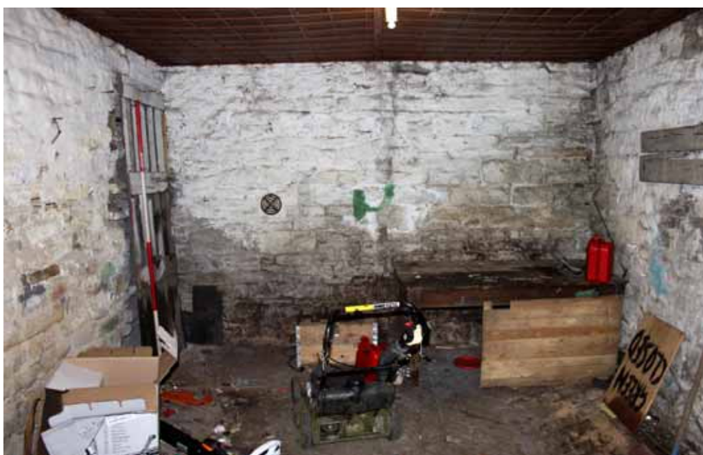
Plate 10: The south-western room of Building C looking south-east
