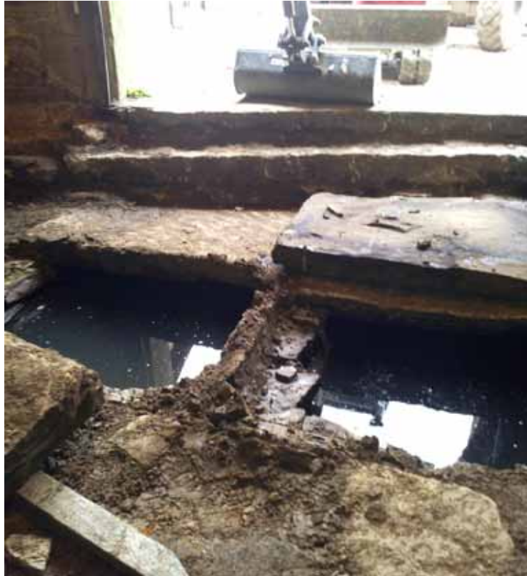
Plate 27: Water-filled voids discovered beneath the floor in front of the south-western carriage entrance of Buildings A
