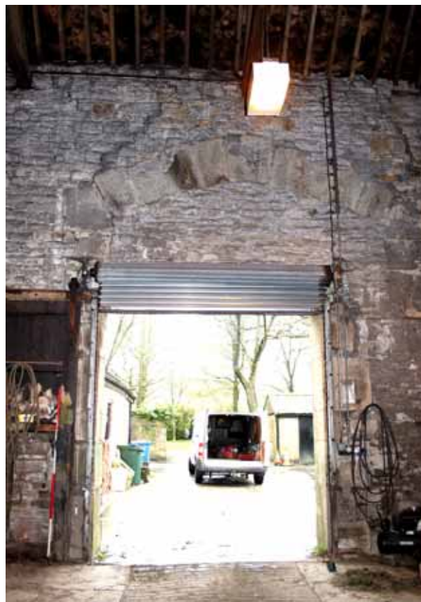
Plate 14: Internal face of the partially blocked south-western carriage entrance of the barn
