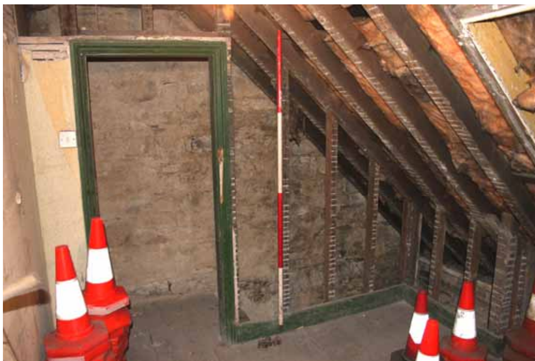
Plate 8: Attic interior looking south-west
