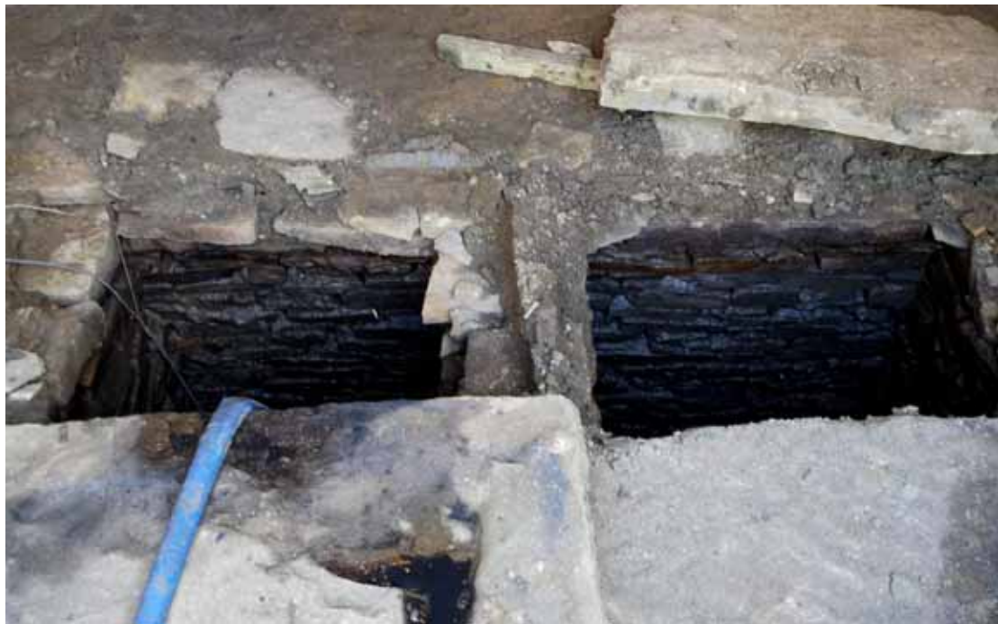
Plate 28: The voids looking north-east following removal of water
