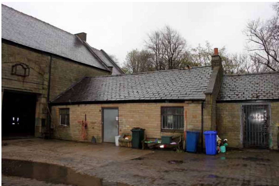
Plate 22: North-west elevation of Buildings B and C
