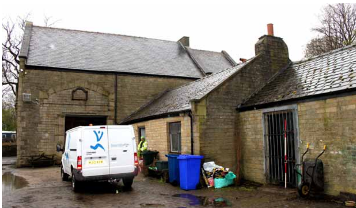
Plate 26: Buildings A, B and C looking North-East
