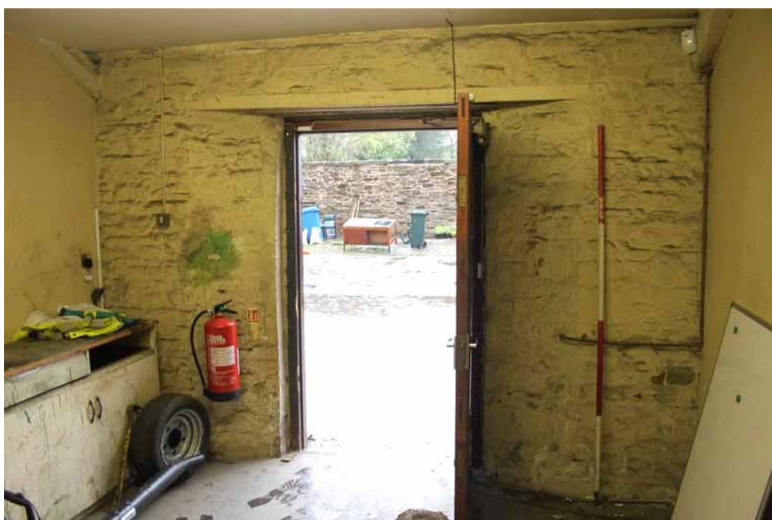
Plate 24: Central room of building B looking north-west
