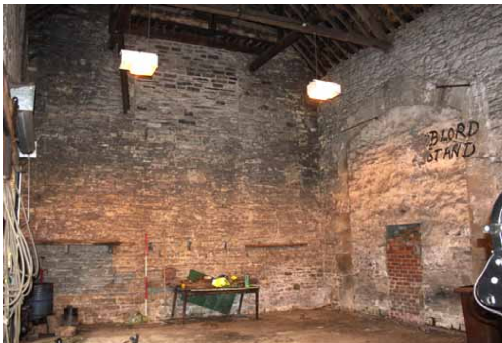
Plate 3: The north-west internal elevation of the barn, and the blocked north-eastern carriage entrance
