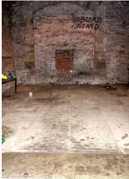
Plate 13: internal face of the blocked north-eastern carriage entrance of the barn
