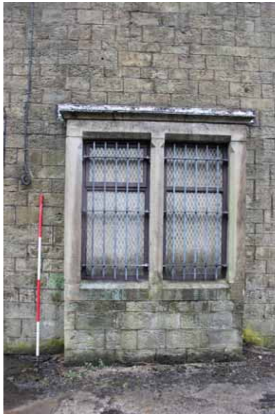
Plate 18: Mullioned window in protruding bay in the south-eastern elevation of the cottage
