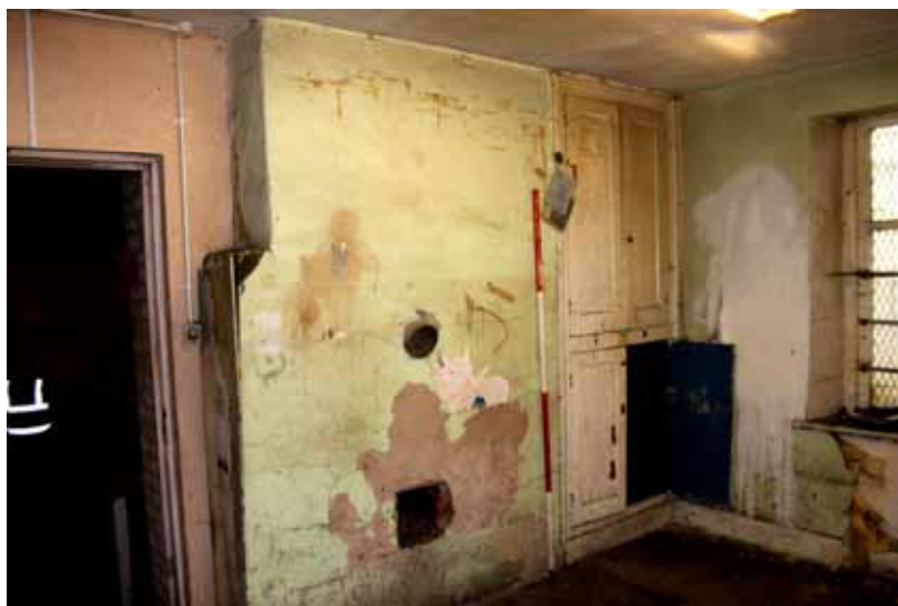
Plate 7: Room G3 of the cottage looking north
