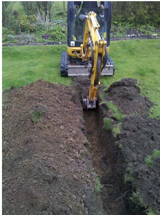
Plate 3: North-facing view of cable trench within garden of Camp Farm House
