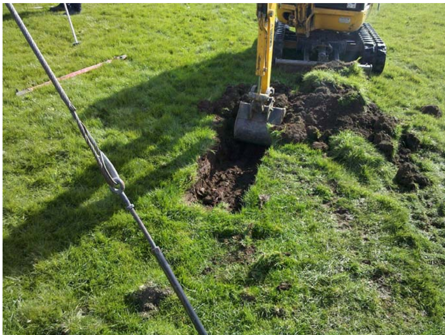
Plate 4: South-west-facing view of trench for stay wire for pole 073206
