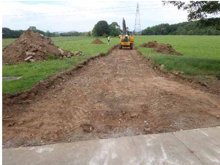
Plate 2: Topsoil stripping along the access track adjacent to the sewage works, looking west, showing limited exposure of natural clay and cobble subsoil
