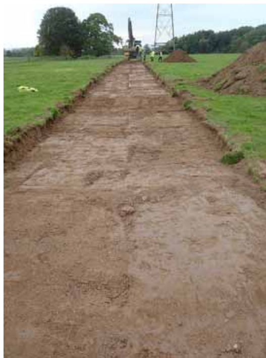
Plate 1: Topsoil stripping along the route of the access track, looking west
