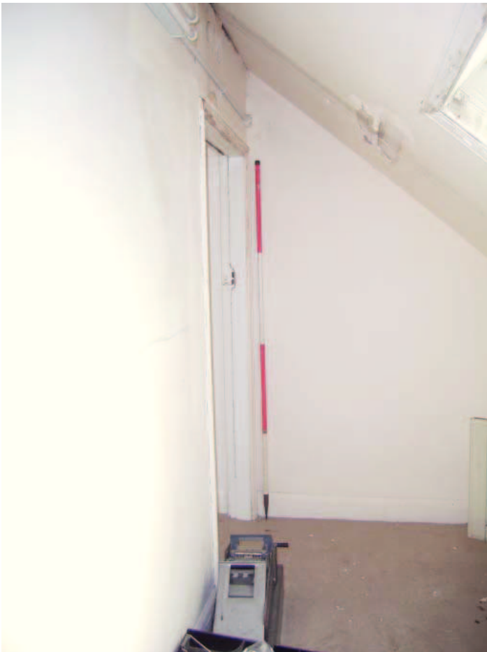
Plate 20: Detail of storage room on second floor
