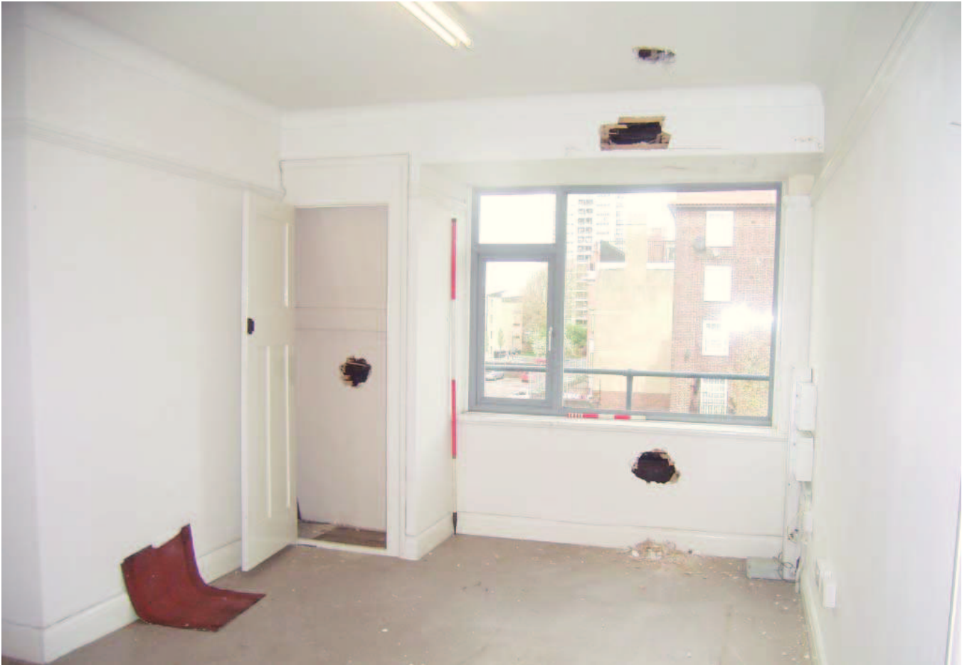
Plate 19: View of south east room on second floor
