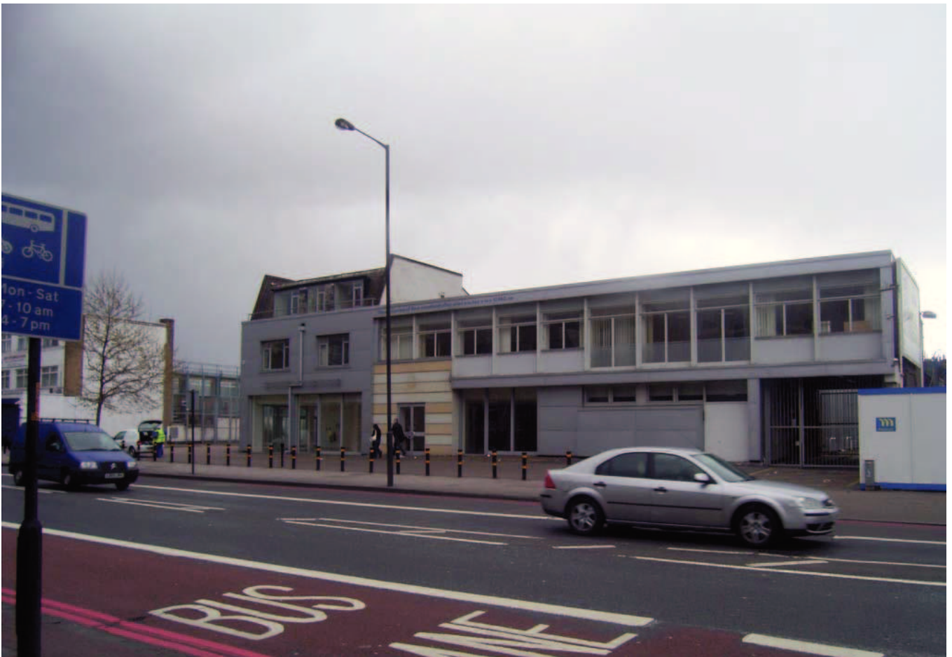
Plate 1: View of south elevation
