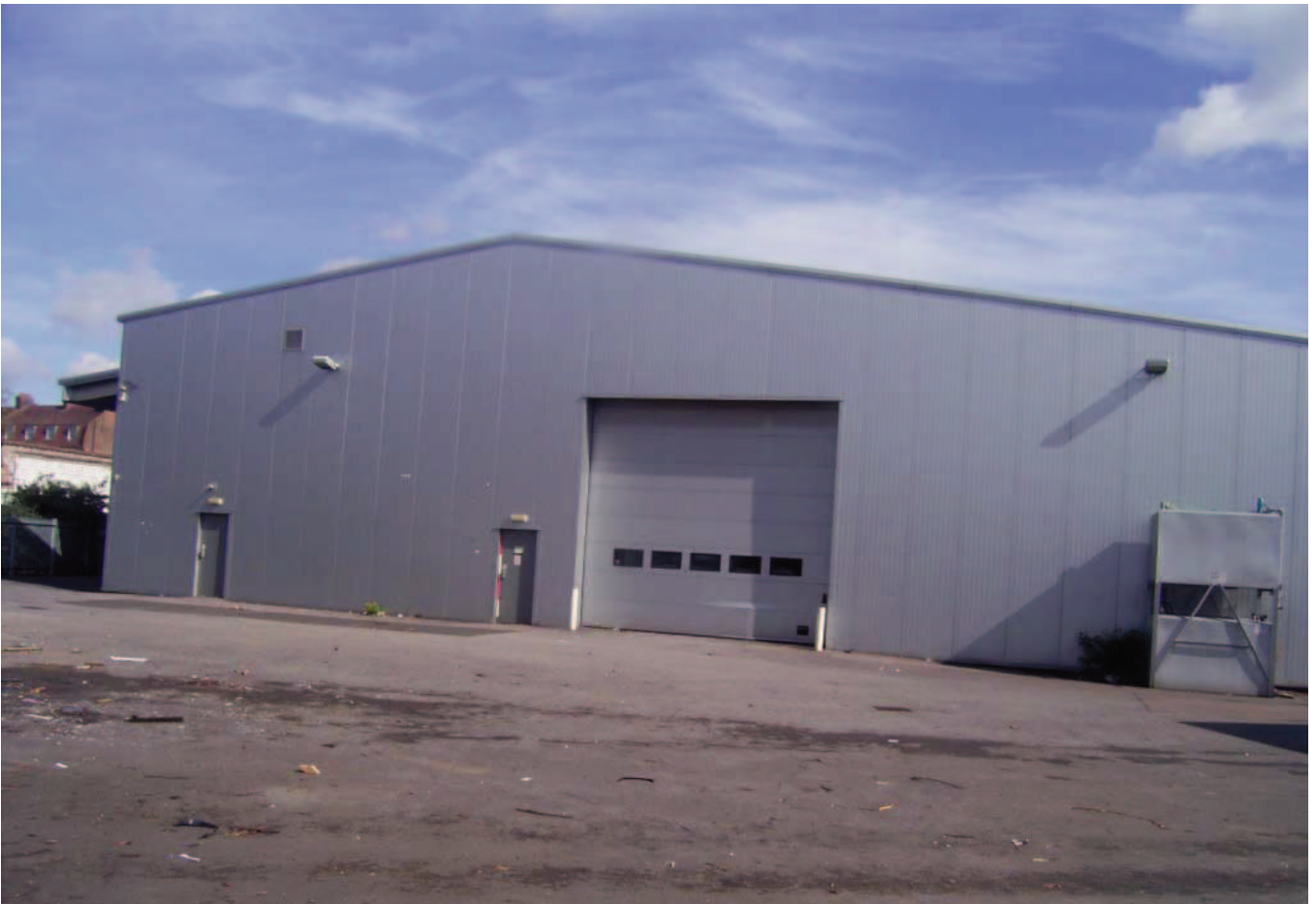
Plate 6: View of modern workshop to rear of showroom
