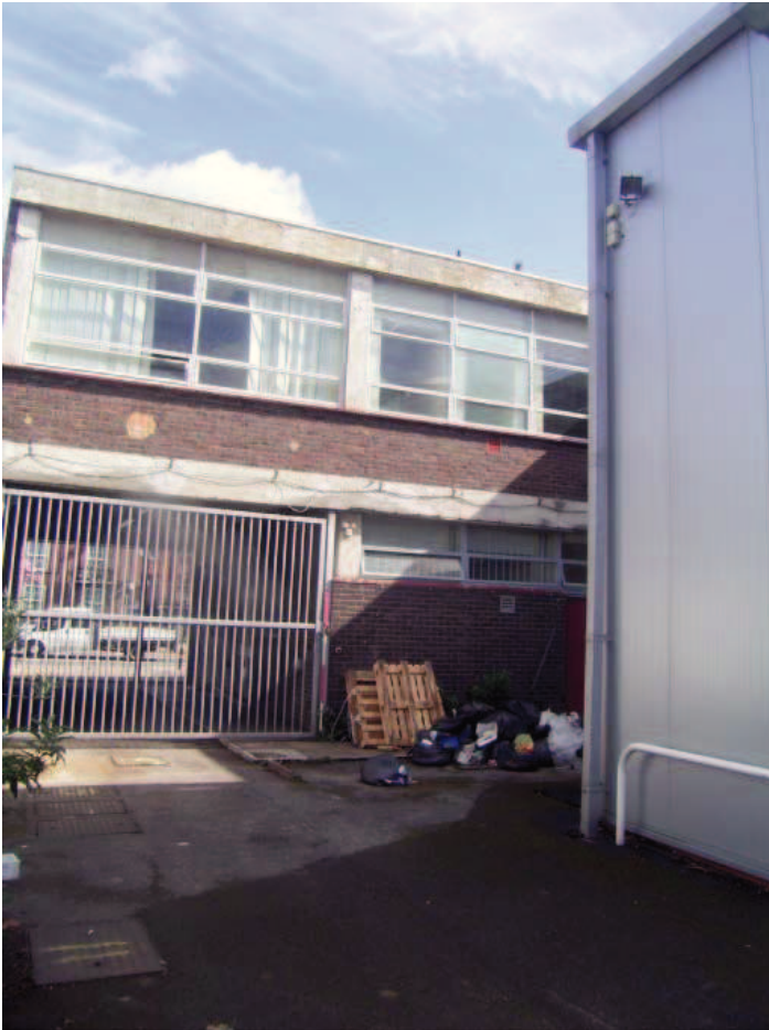
Plate 7: View of 1970s extension north elevation
