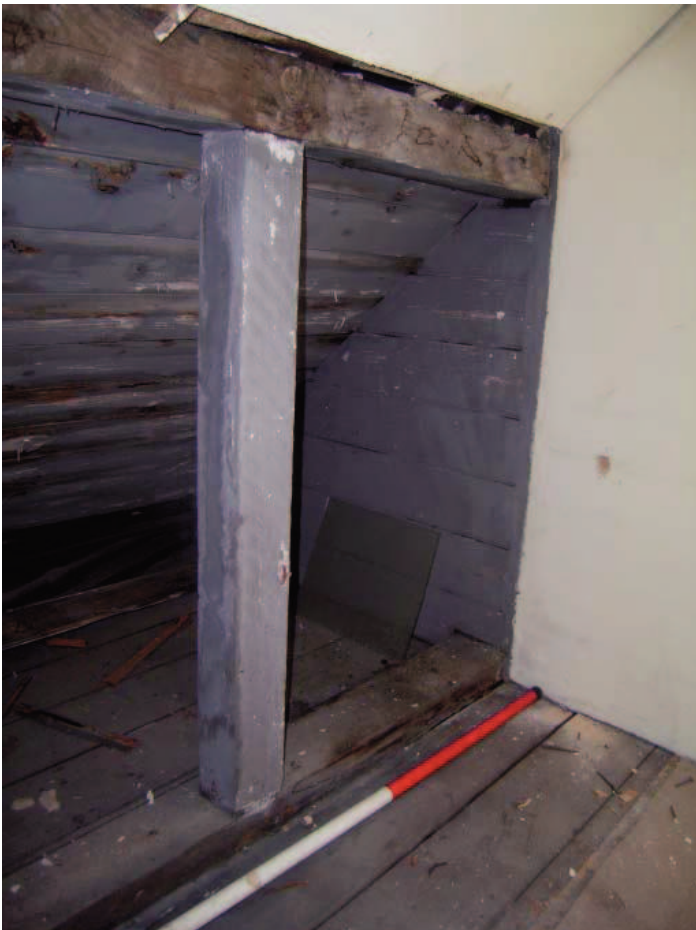
Plate 22: View of boarded storage area on second floor
