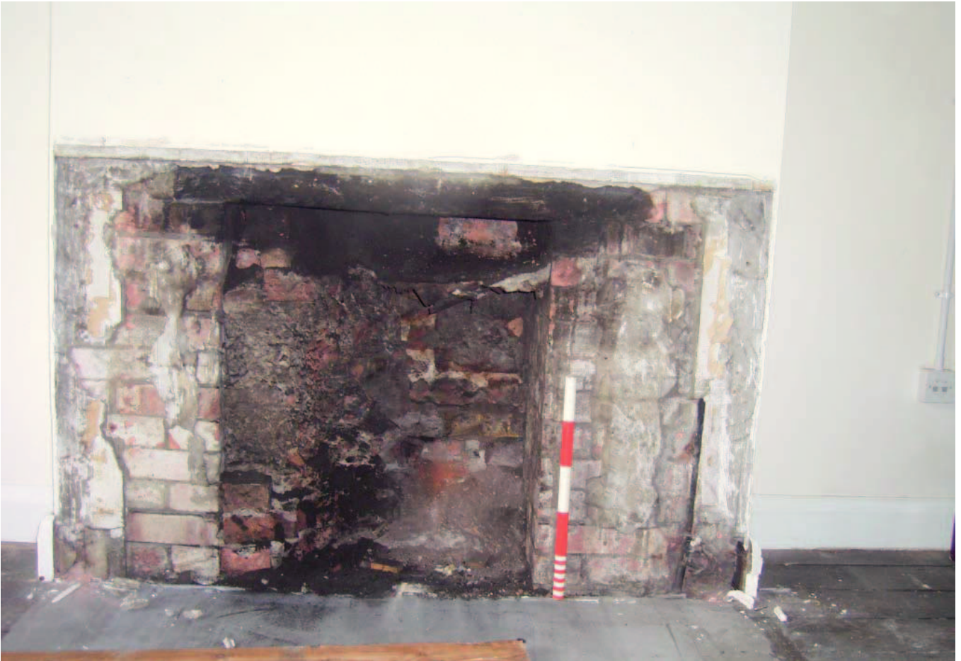
Plate 13: Detail of former hearth within first floor training room
