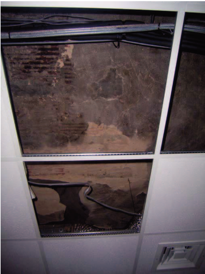
Plate 16: Exposed fragment of lath and plaster ceiling on first floor
