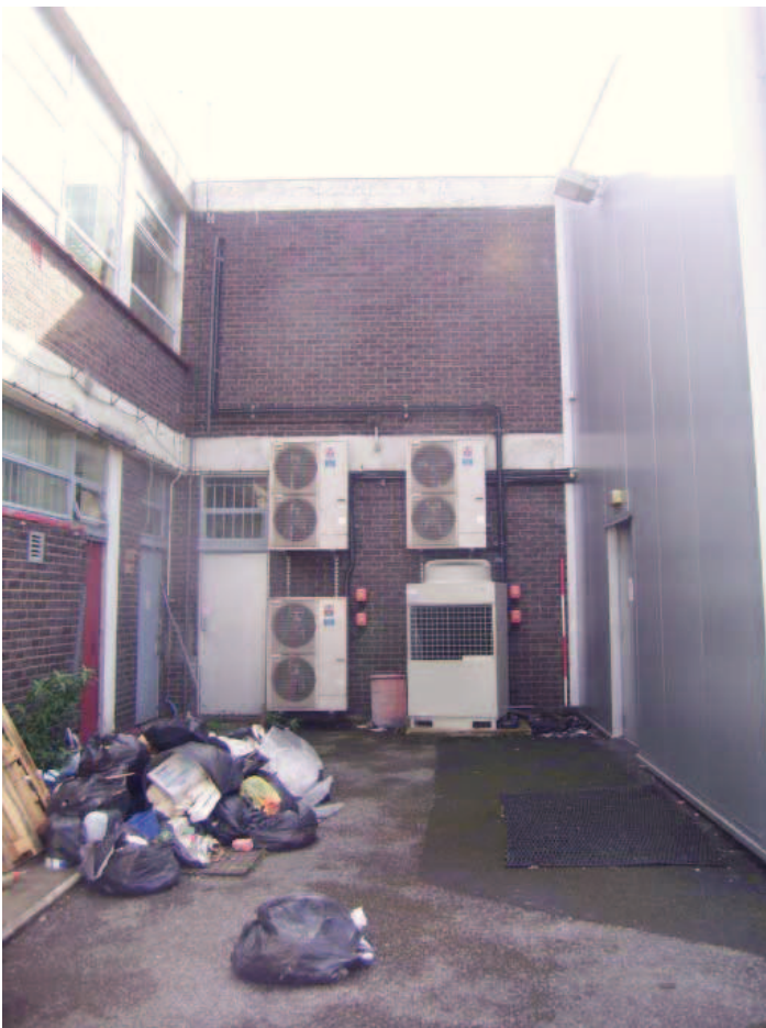
Plate 8: View of east elevation showing join between 1970s extension and workshop
