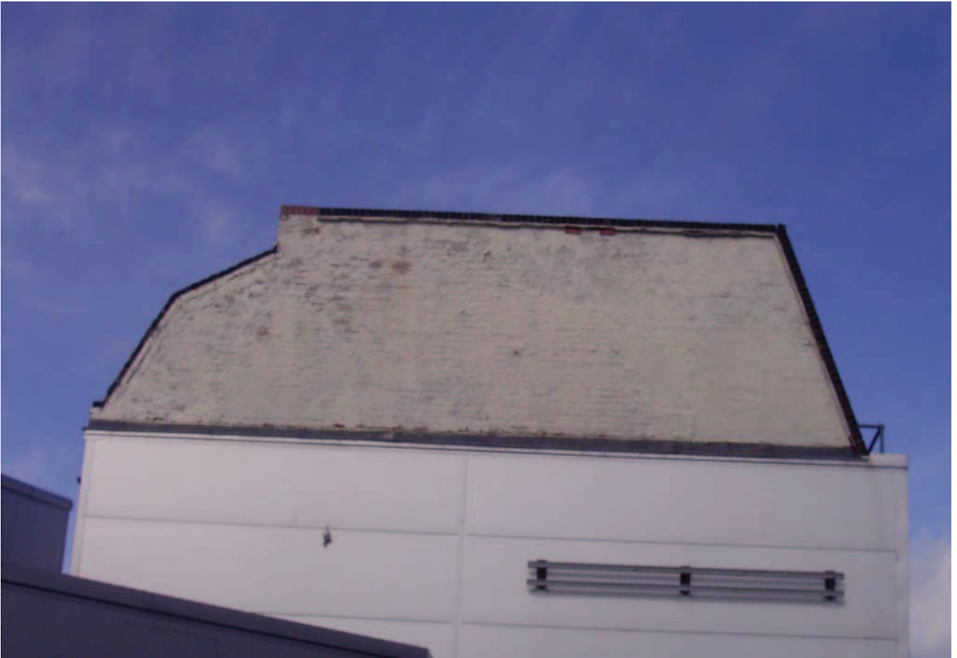
Plate 5: Detail of west elevation of brick gable
