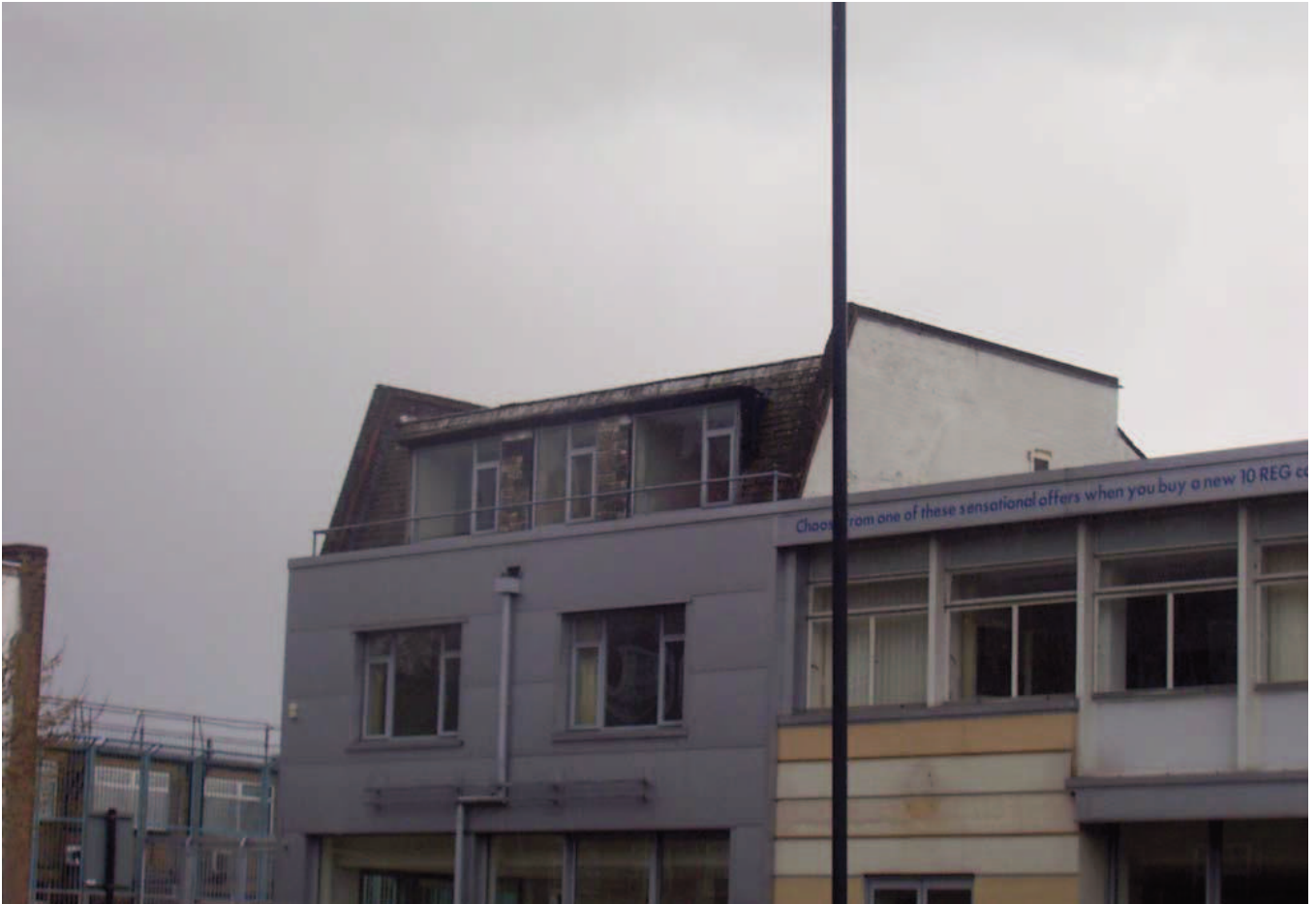
Plate 3: Detail of mansard roof
