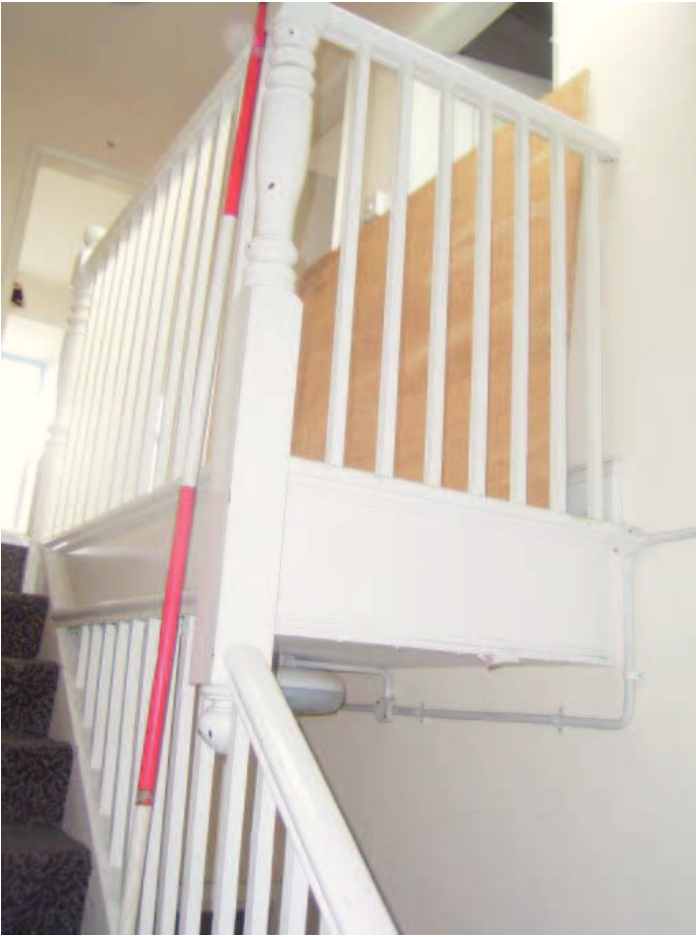
Plate 17: View of stairwell to second floor
