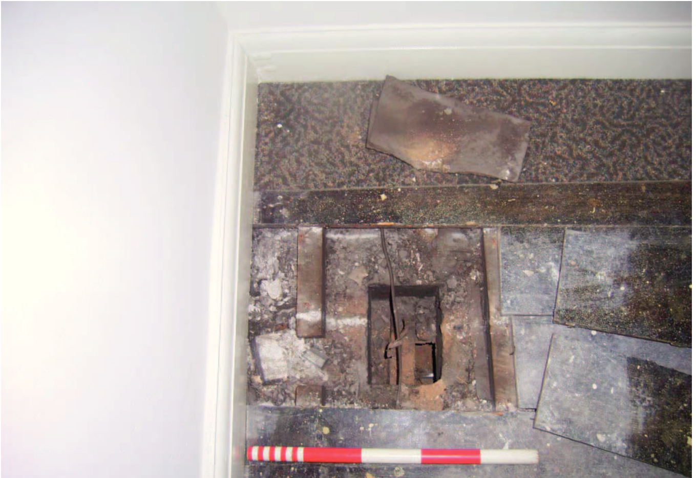
Plate 15: Detail of removed floor boards within rest room
