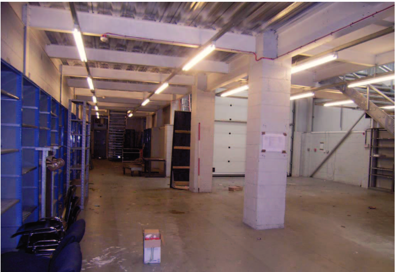
Plate 10: Internal view of ground floor store room
