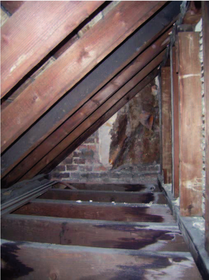
Plate 21: View within roof space on second floor
