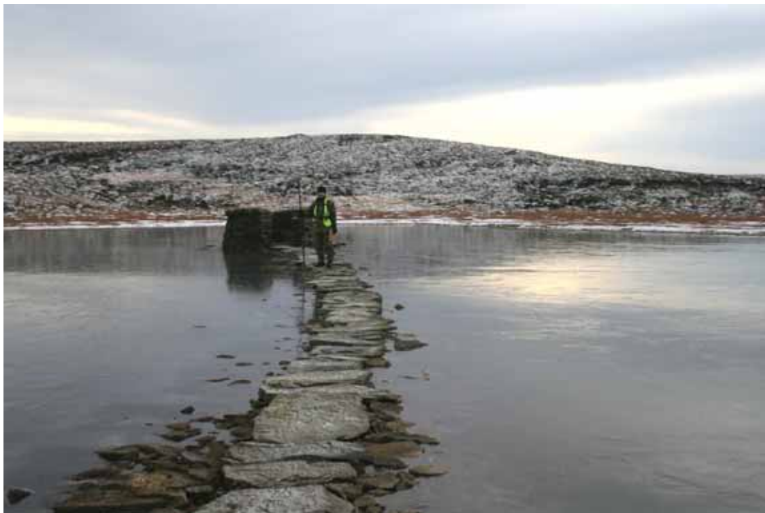
Plate 12: Looking southwards along the stone causeway (Site 22)
