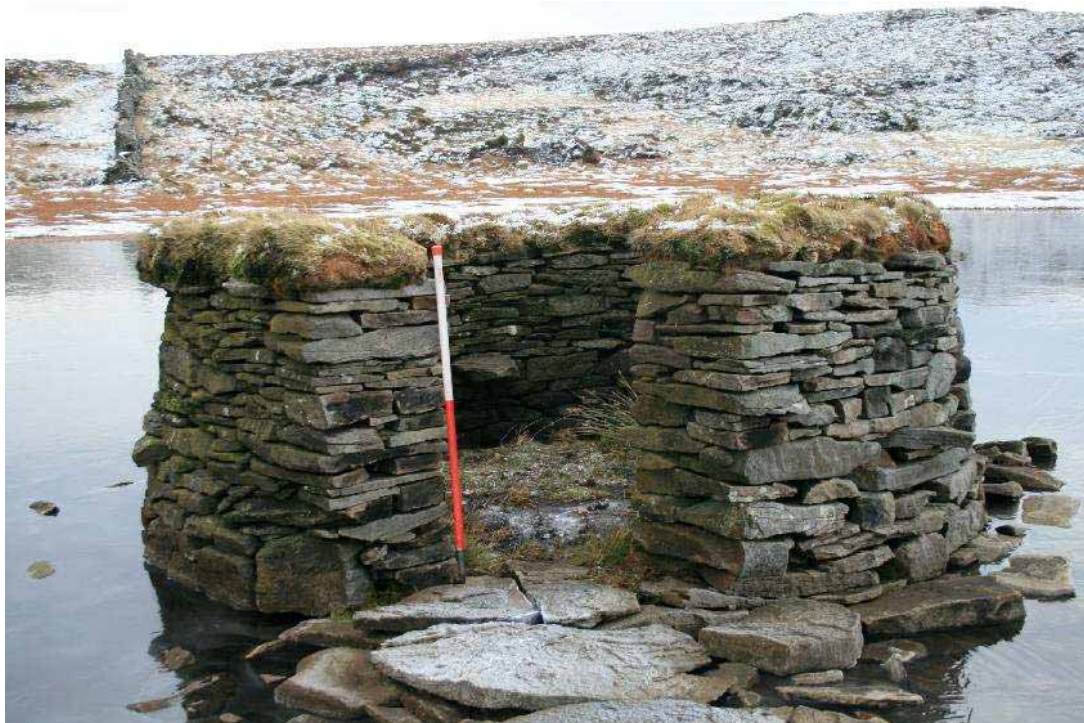
Plate 13: A view through the entrance of the shooting butt (Site 22) with a through-stone seat visible in the rear part of the wall
