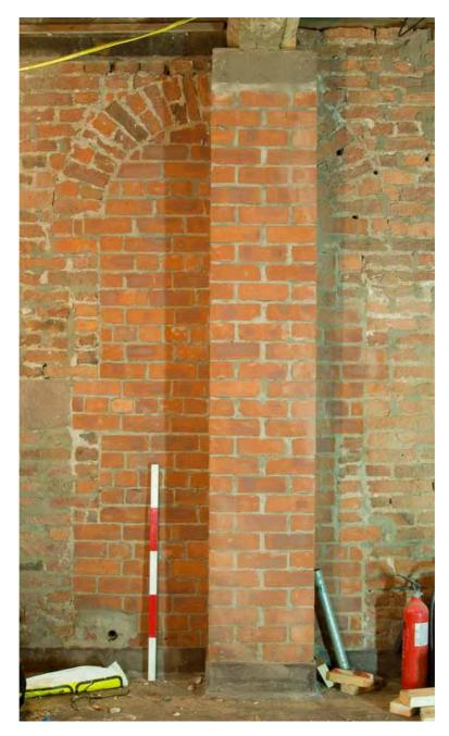
Plate 18: Blocked doorway into Stair Tower (G13)
