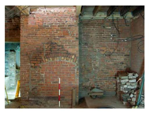
Plate 20: Blocked and remodelled fireplace, south wall, the Radclyffe Room
