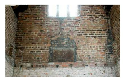
Plate 29: Inserted wall plaque, and window in Stair Tower gable
