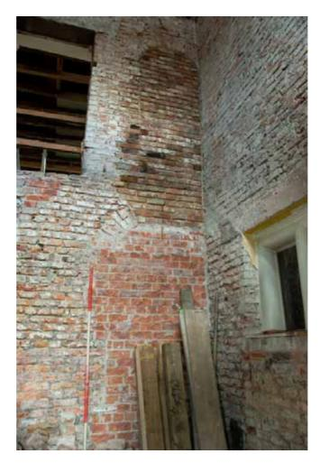
Plate 24: Blocked doorways in the Stair Tower, at ground and first floor level
