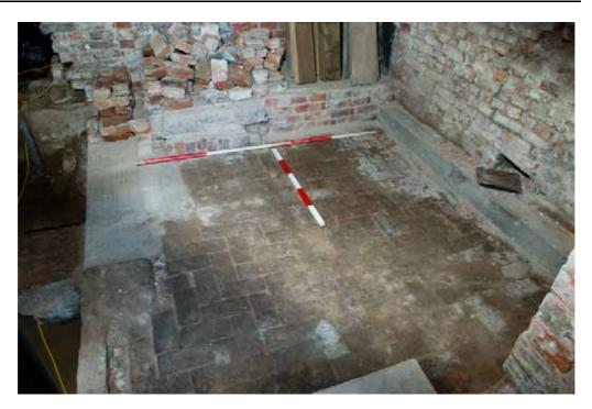
Plate 27: Herring-bone brick floor of Stair Tower
