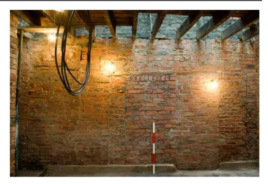
Plate 31: Blocked apertures in west wall of the annexe
