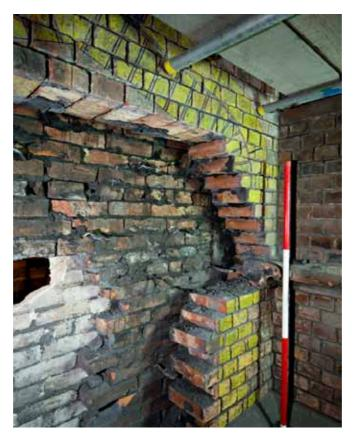
Plate 7: Detail of cavity wall construction
