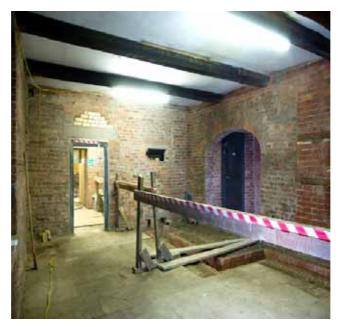
Plate 13: View of the Kitchen (G10), showing flue aperture and re-modelled doorway
