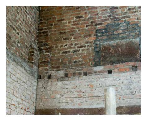
Plate 22: Reduced wall thickness at second-floor level of the stair tower
