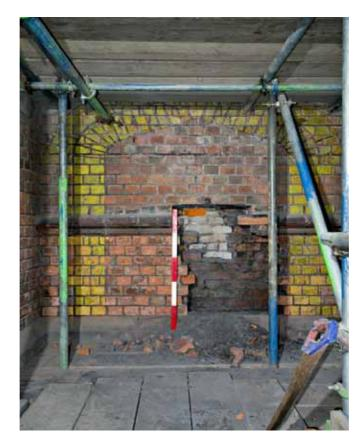
*Plate 6: South external wall of the Great Hall (G4), showing the position of the new doorway*
