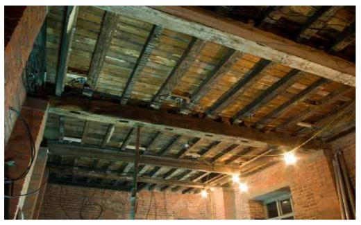
Plate 17: Ceiling within the Radclyffe Room (G11B), showing re-used beams
