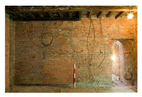
Plate 19: Blocked fireplace and remodelled doorway, the Radcylffe Room
