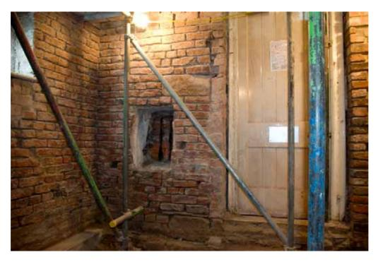
Plate 26: Small window with wrought-iron bars revealed at ground-floor level
